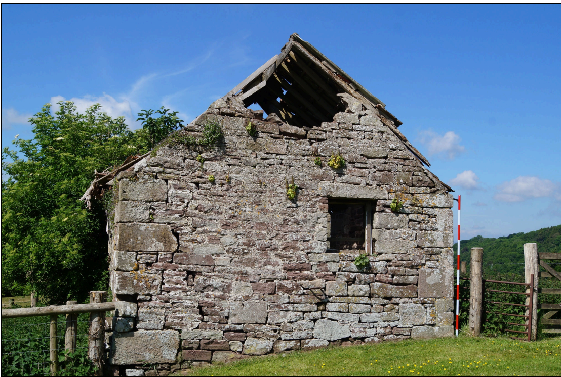
Plate 12: BGT2020_012, view of the eastern wall, looking west-northwest
