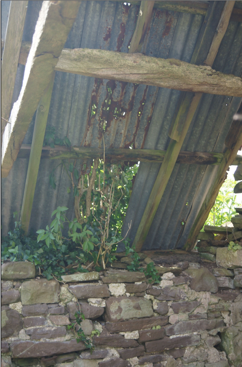
Plate 53: BGT2020_053, view of the roof in southwest corner.
