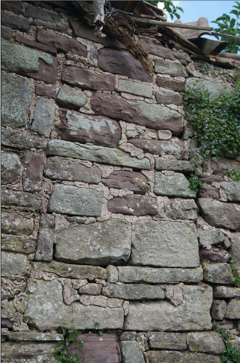
Plate 60: BGT2020_060, external view of detail of infilled window on southern wall.
