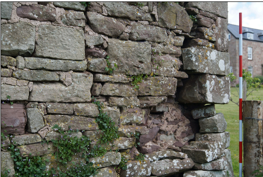
Plate 59: BGT2020_059, external view of southeast corner facing northeast.
