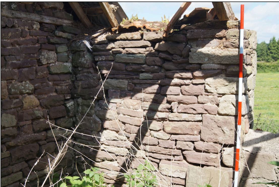
Plate 31: BGT2020_031, internal view of north-western corner, looking north-northwest.
