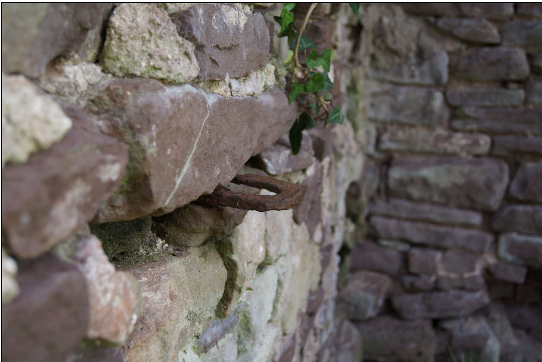
Plate 72: BGT2020_072, detail of internal horseshoe in wall.
