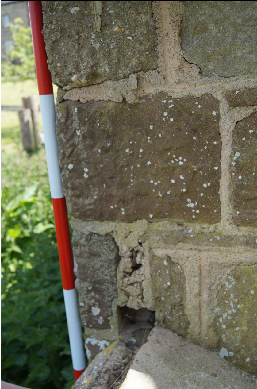
Plate 46: BGT2020_046, internal detail of window on northern wall looking east.
