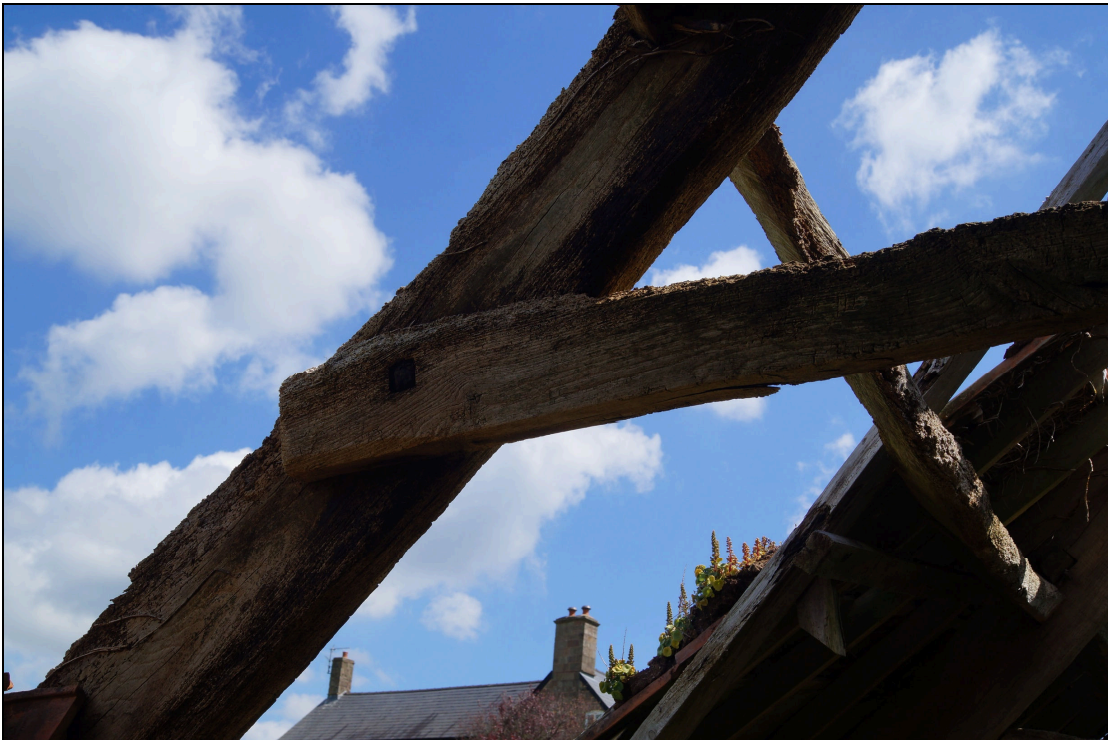
Plate 50: BGT2020_050, details of roof timbers facing northeast.
