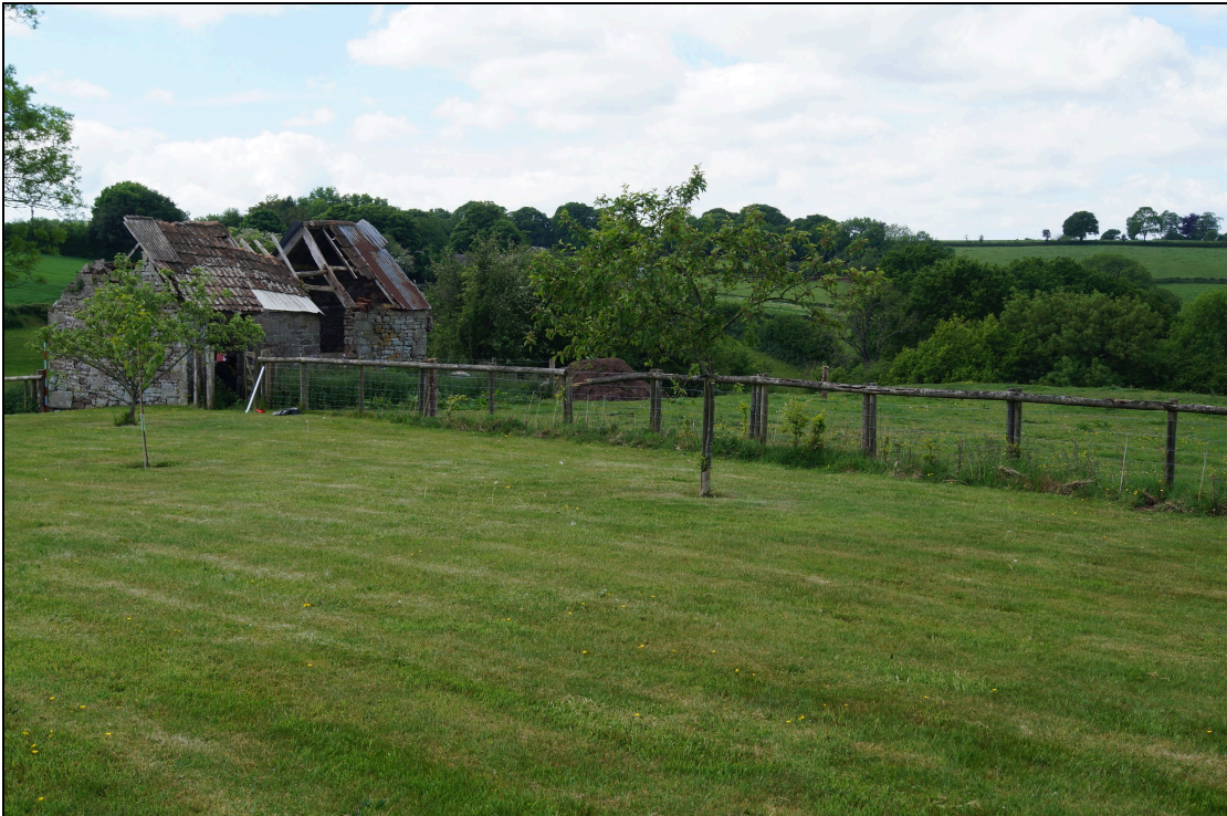
Plate 6: BGT2020_006, general outside view of Chapel Barn looking southwest.
