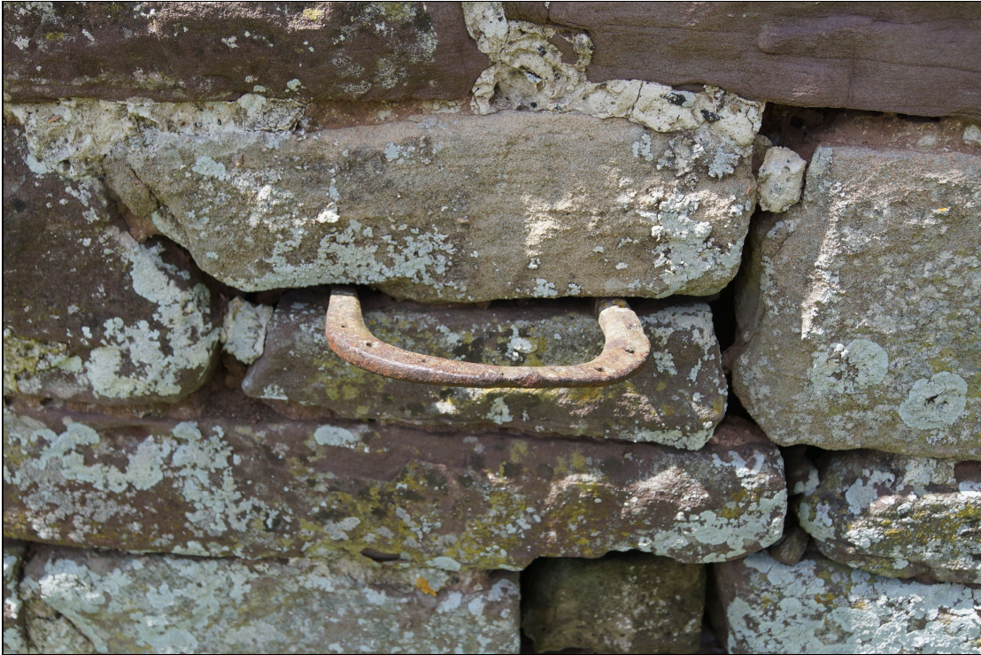
Plate 71: BGT2020_071, detail of horseshoe tied into external eastern wall.
