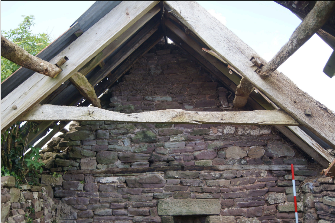
Plate 35: BGT2020_035, internal view of roof and western wall, looking west.
