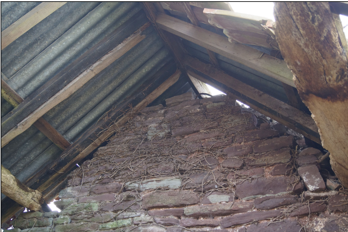
Plate 36: BGT2020_036, internal view of the roof and western gable.
