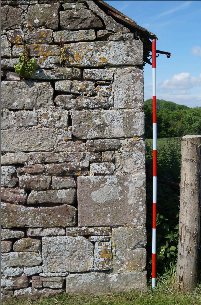
Plate 13: BGT2020_013, View of the northeastern corner of eastern wall, looking west.
