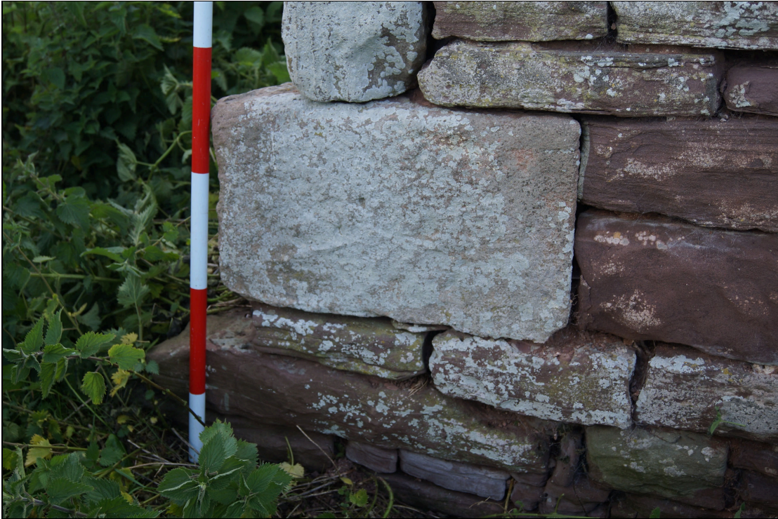
Plate 56: BGT2020_056, external view of bottom of north west corner.
