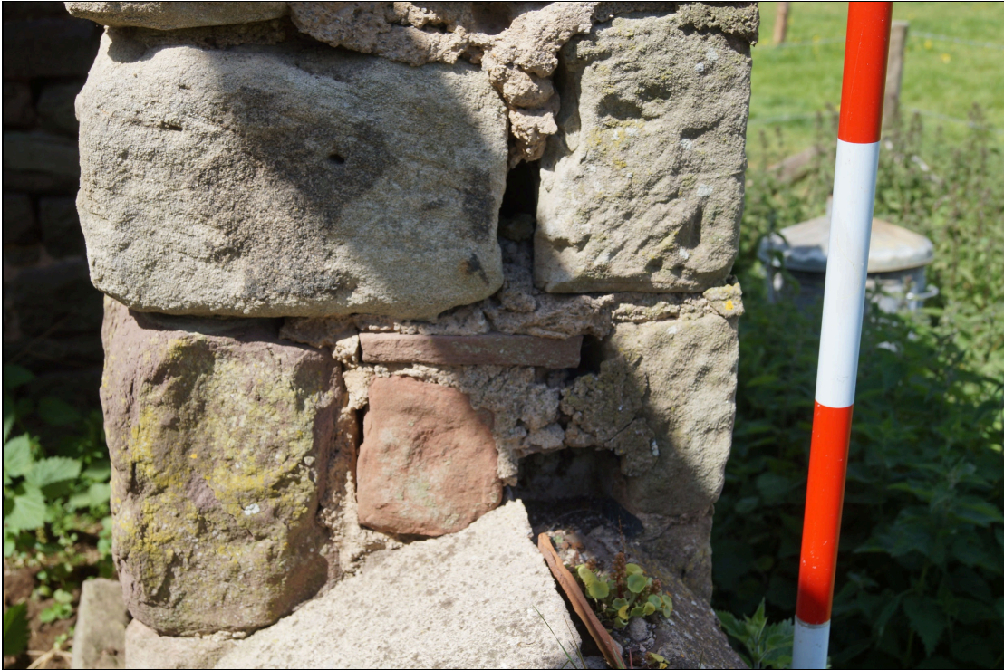
Plate 45: BGT2020_045, internal view of window in northern wall looking west.
