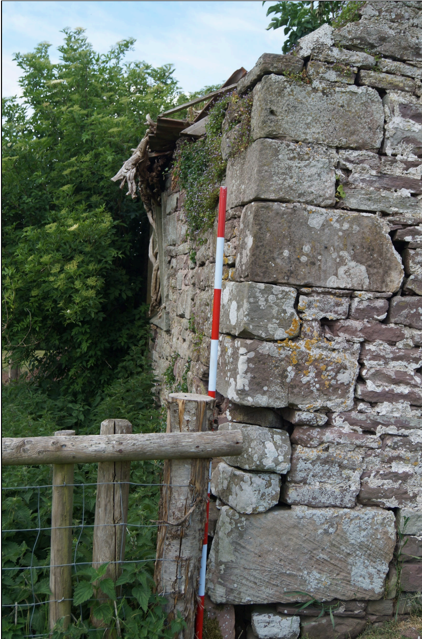
Plate 62: BGT2020_062, external view of south-eastern corner facing west.
