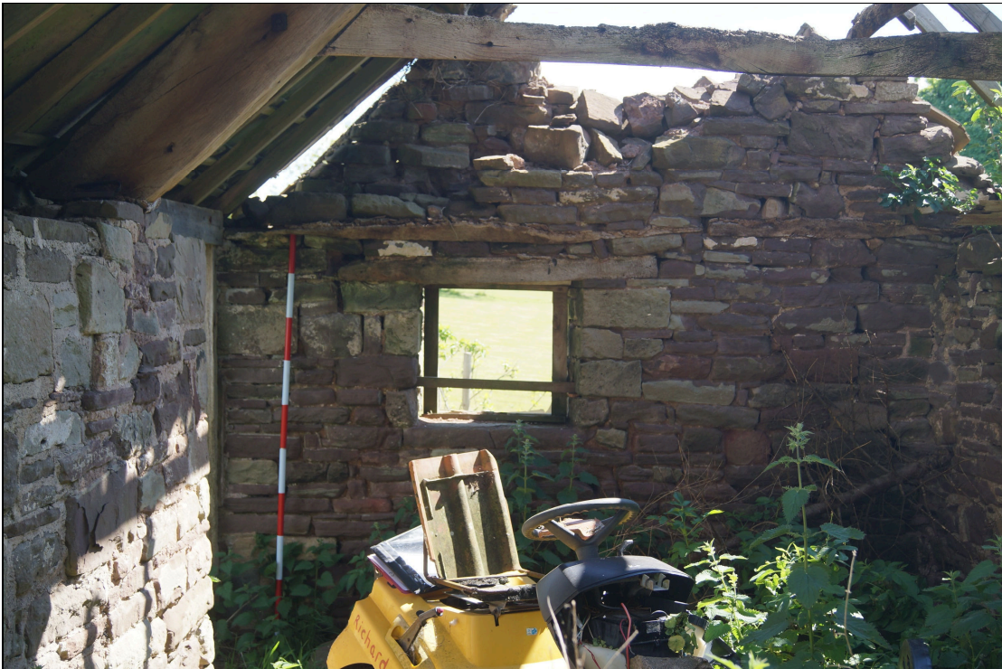
Plate 22: BGT2020_022, internal view of eastern wall, looking east
