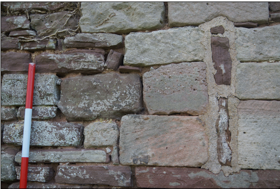
Plate 57: BGT2020_057, external view of blocked in window niche facing east.
