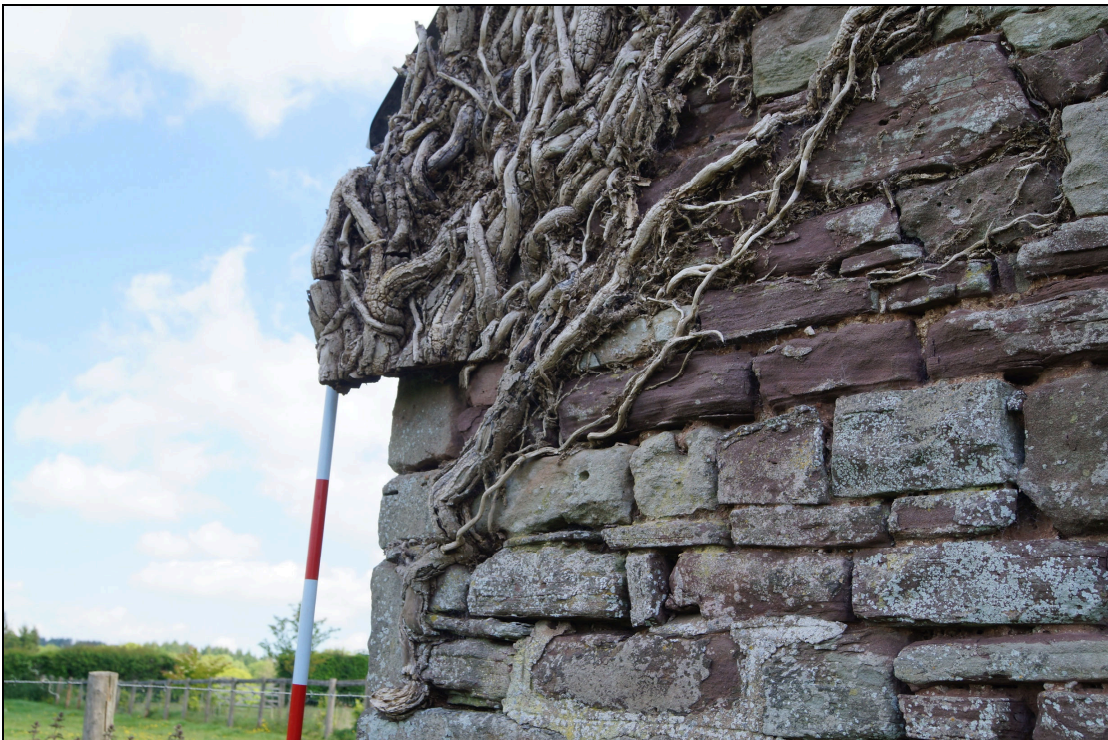
Plate 55: BGT2020_055, external view of north western corner facing northeast.
