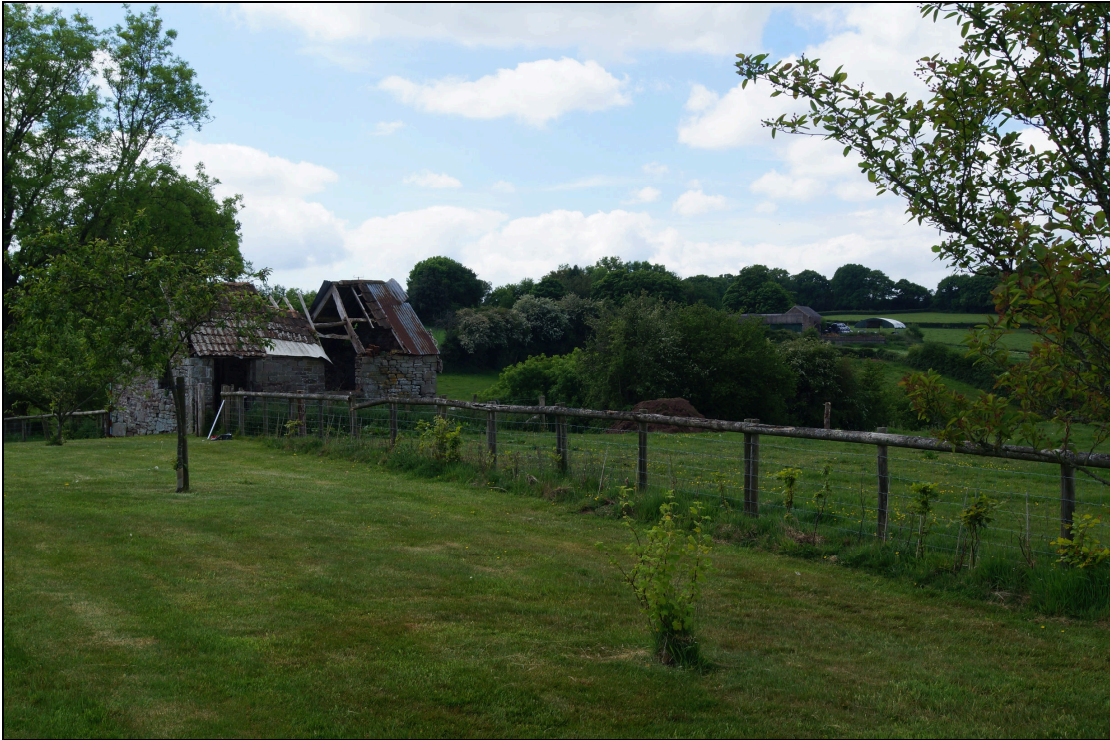
Plate 3: BGT2020_003, general outside view of Chapel Barn looking southwest.
