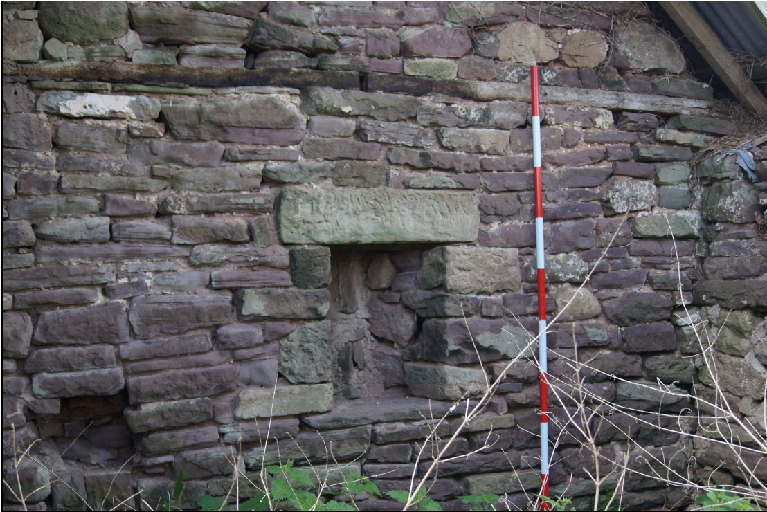
Plate 43: BGT2020_043, view of blocked-in window niche on western wall looking northwest.
