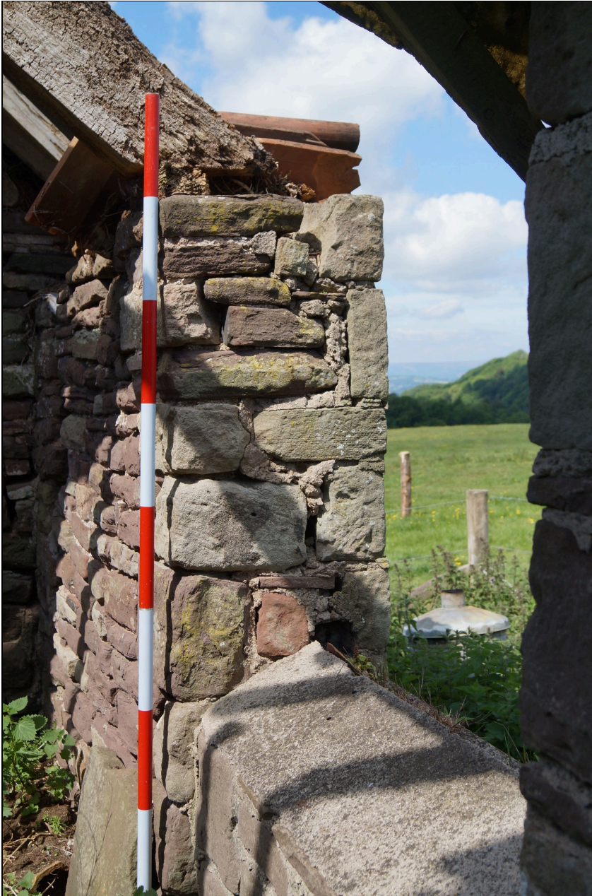
Plate 32: BGT2020_032, internal view of northern window facing west-northwest.
