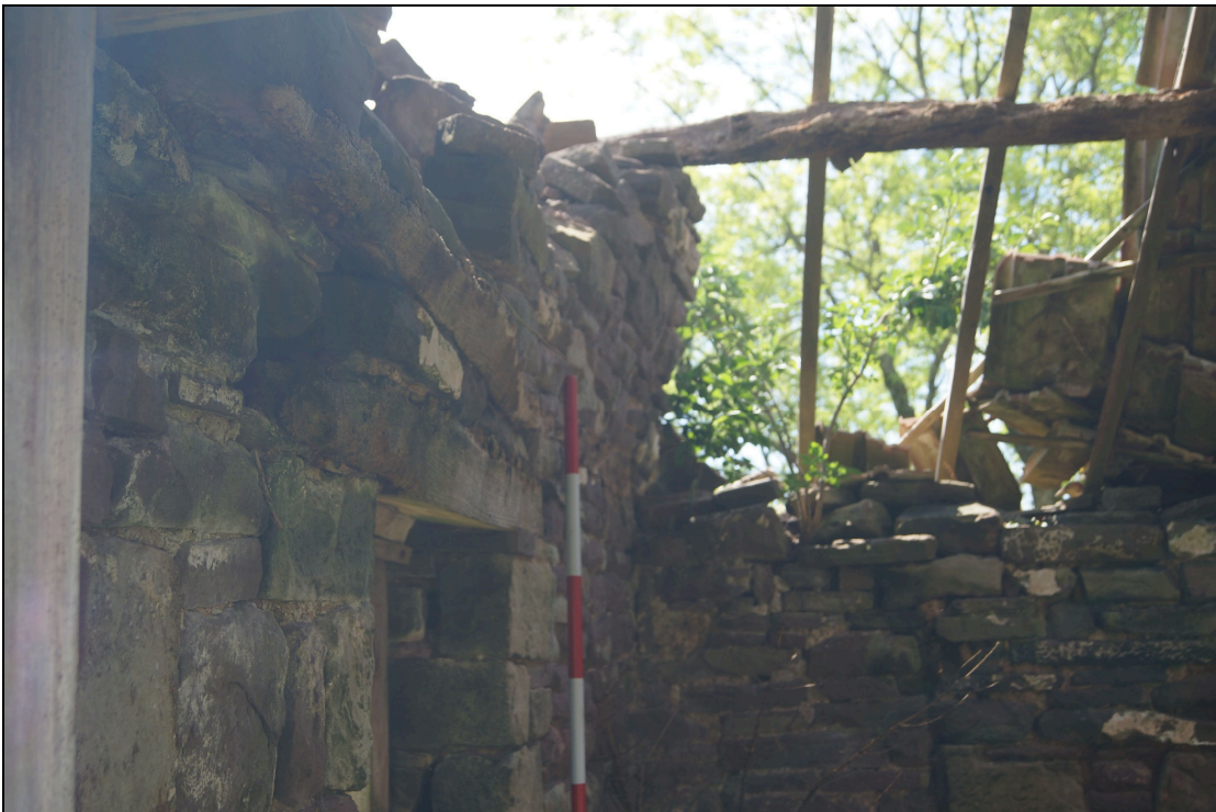
Plate 27: BGT2020_027, view of southeastern internal corner from doorway, looking south-southeast.
