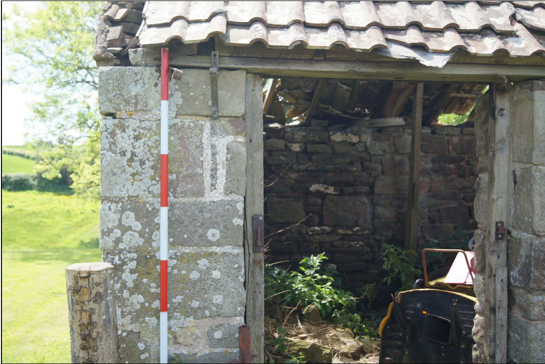
Plate 65: BTC2017_065, external view of doorway facing south.
