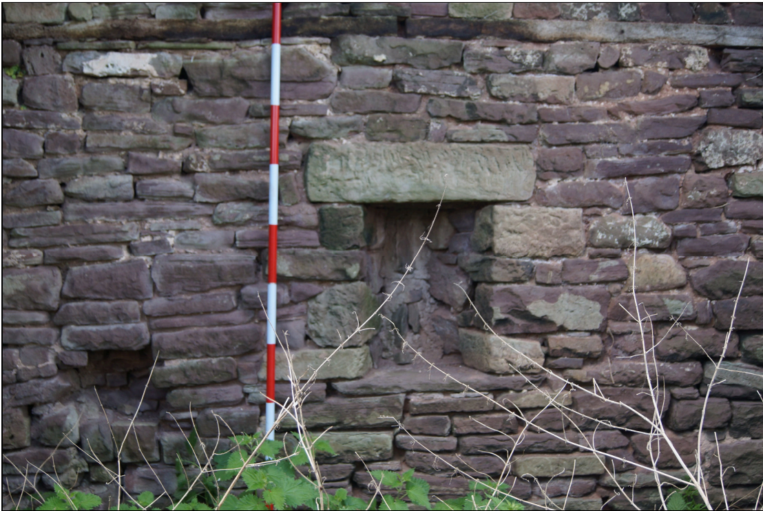
Plate 41: BGT2020_041, view of blocked-in window niche on western wall, looking west-northwest.
