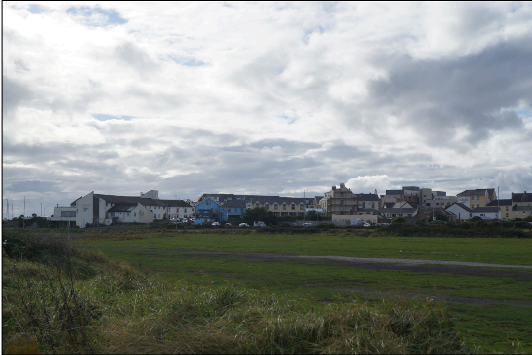
Plate 1: Looking west-southwest across the filled in dock area, now in use as a car park/open space but may be developed in the future under regeneration plans. The Glamorgan Holiday Hotel is on the left.
