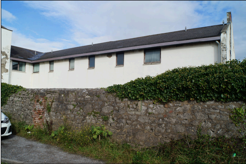
Plate 23: Looking northeast to the western side of the Glamorgan Holiday Hotel over the stone retaining wall. This wall has been patched and repaired but appears to be one of the few remaining features of the early development to the west of the harbour.
