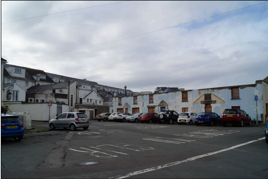
Plate 31: Looking northeast across "The Square" from outside the Glamorgan Holiday Hotel towards the partially demolished Knights Arms and the rear of 4 storey buildings along the Esplanade
