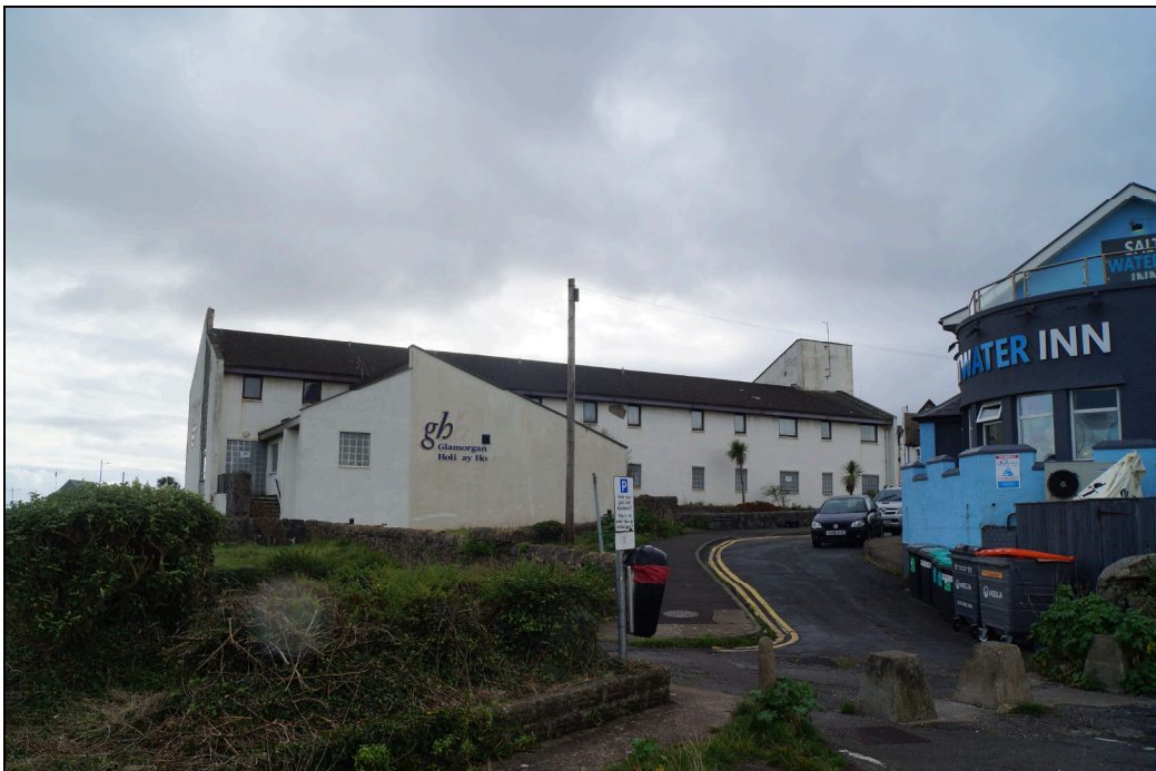
Plate 20: Looking south at the Glamorgan Holiday Hotel with the Saltwater Inn (formerly the Ship and Castle) to the right.
