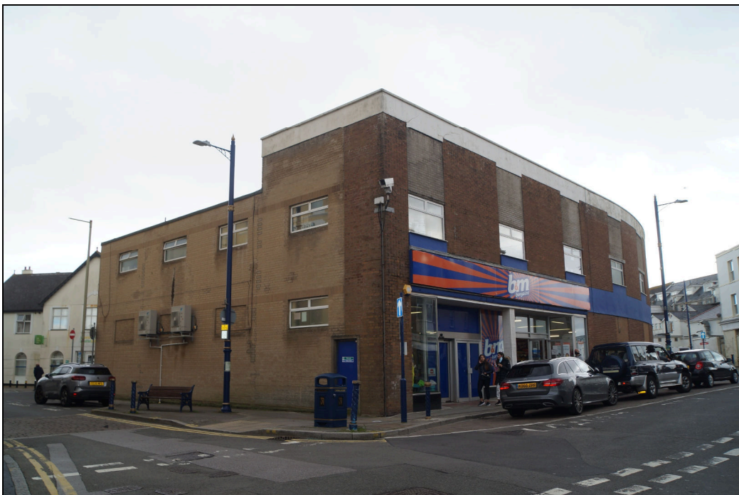
Plate 16: Looking southeast at the junction of Dock Street and John Street.
