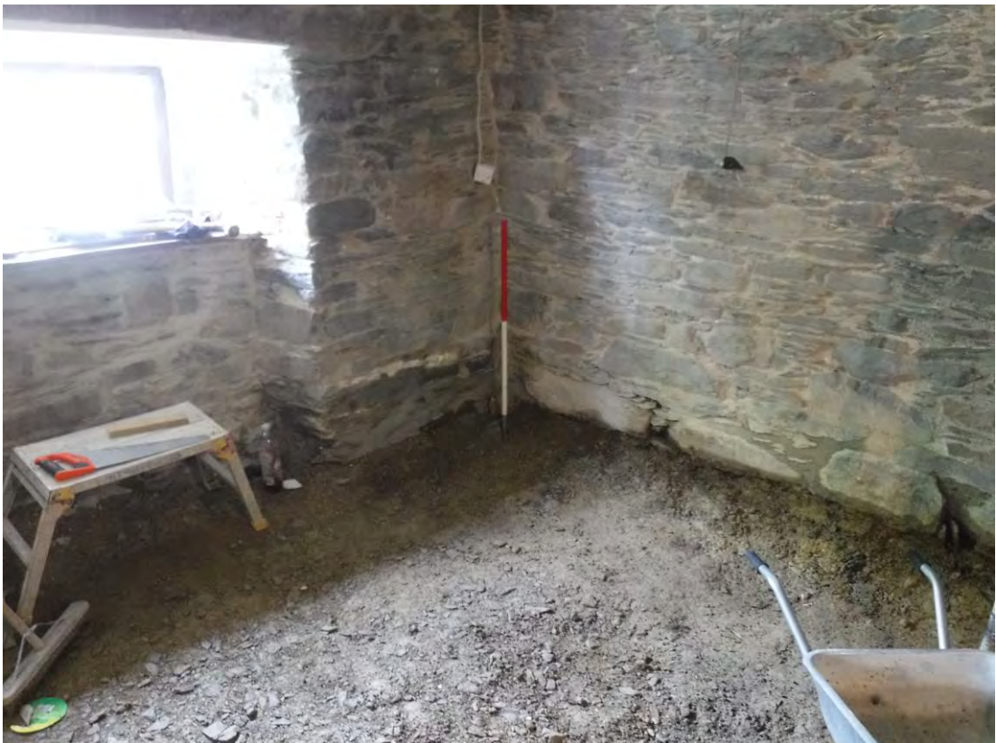
Plate 6: South-western corner of development area (Dining Room) after the lowering of the floor. 1m scale.
