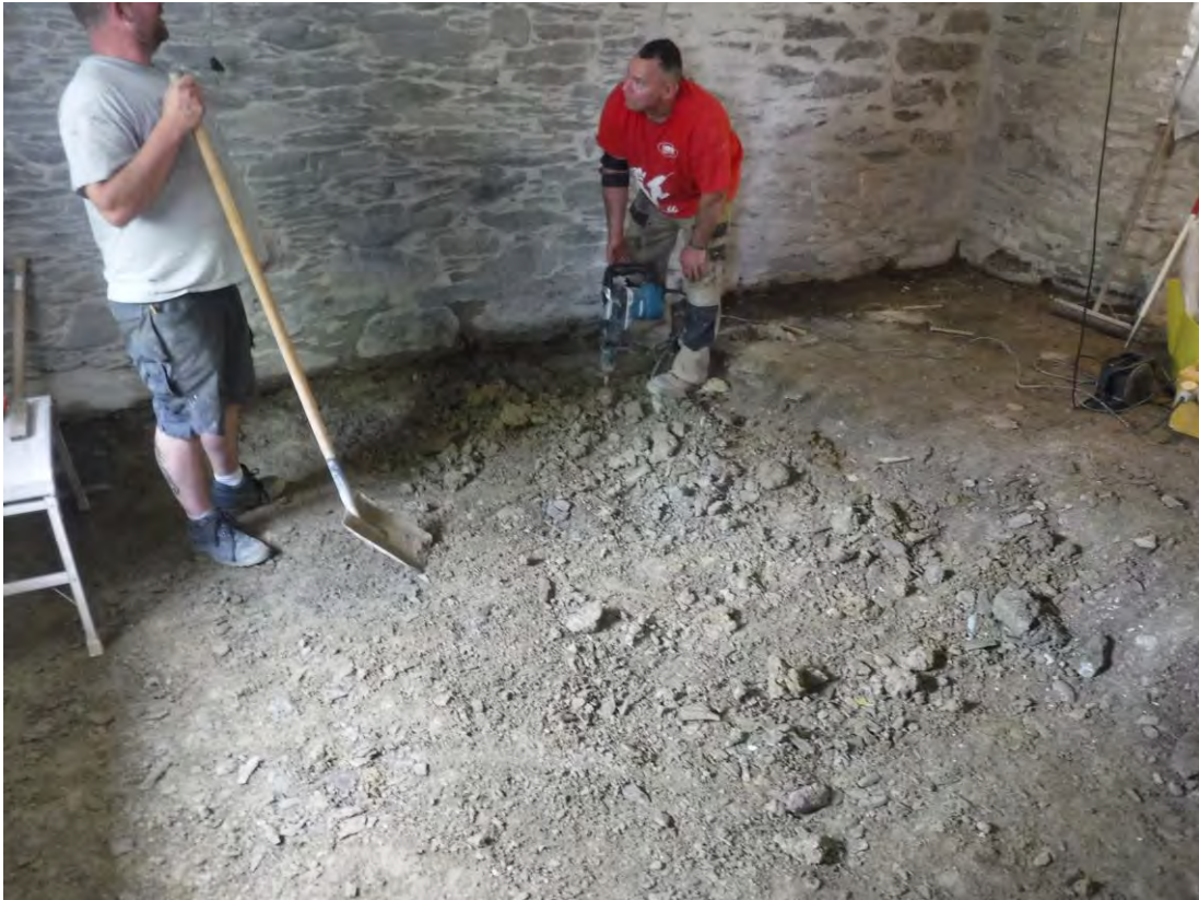
Plate 3: Working photograph of the floor being lowered.
