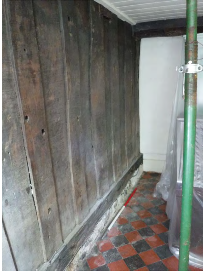
Plate 1: Post and panel partition viewed from lounge. 1m scale.
