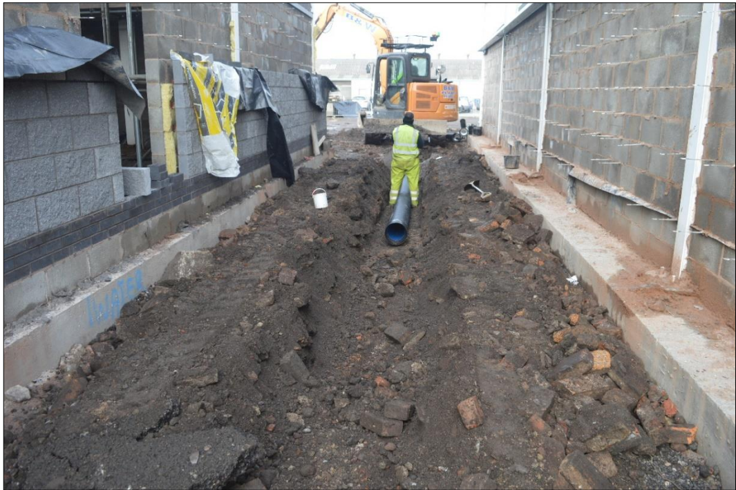
Fig. 5 Pipe-laying in Trench 1
