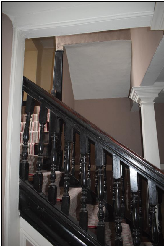
Fig. 9 Detail of staircase ceiling indicating earlier arrangement Photo CPAT 4992-011
