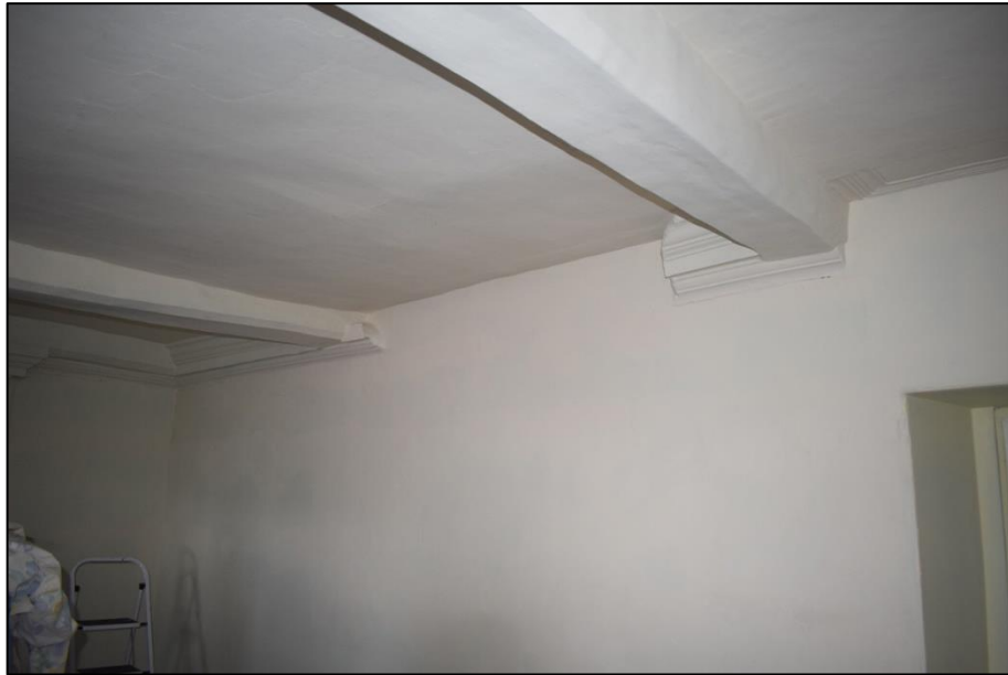
Fig. 23 Cutout in the cornicing in the first floor room on the north elevation Photo CPAT 4992-141
