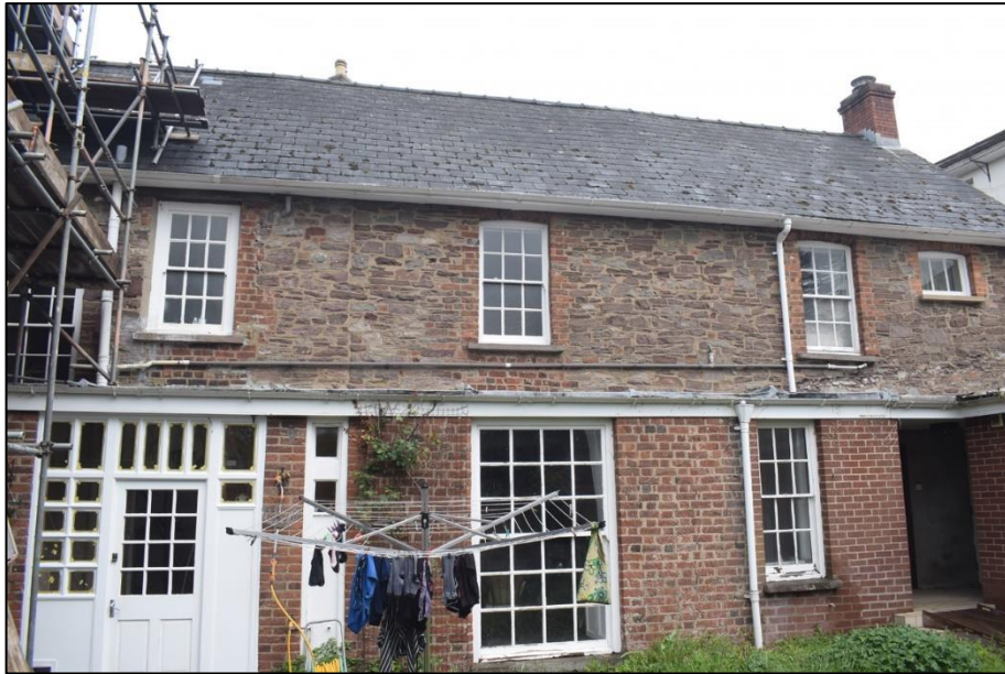
Fig. 18 Extension to former entrance block to the south-east Photo CPAT 4992-041
