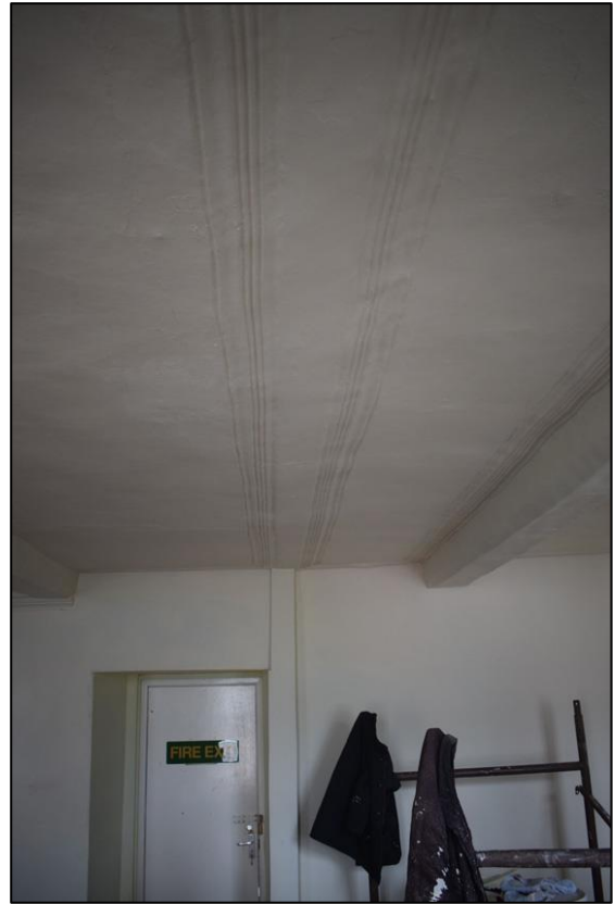
Fig. 13 Decorative plasterwork on first floor ceiling Photo CPAT 4992-087
