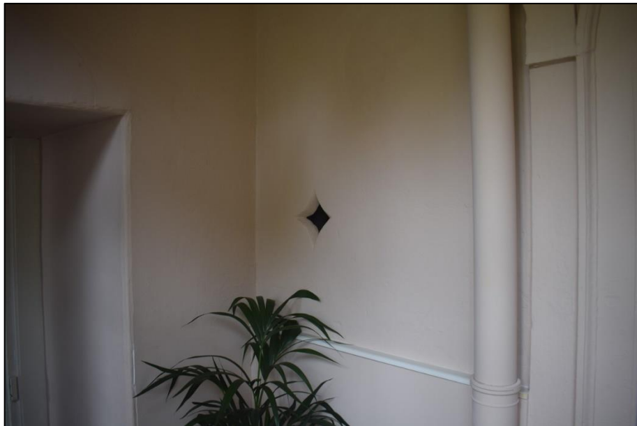
Fig. 7 Look out window adjacent to doorway Photo CPAT 4992-030
