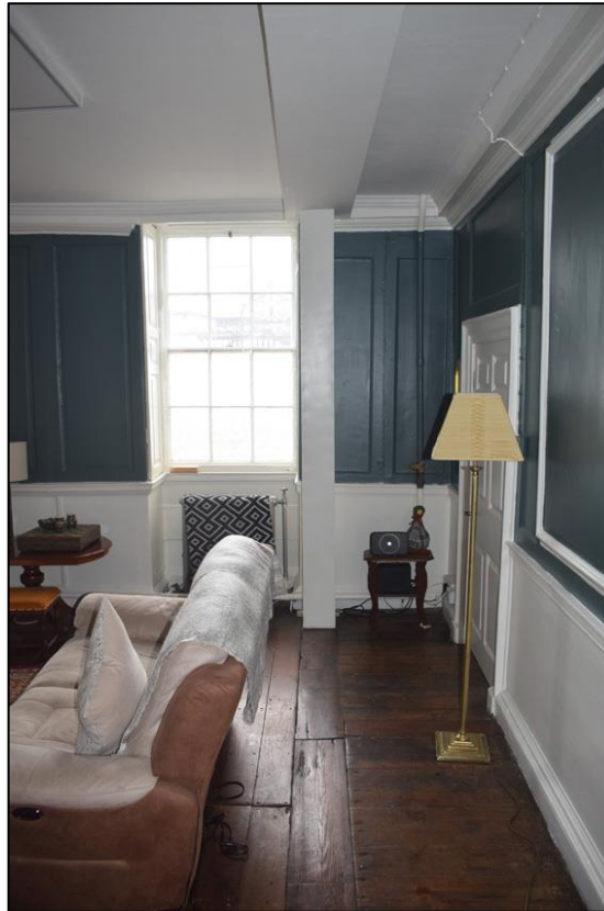
Fig. 20 Former line of partition between parlour and hallway Photo CPAT 4992-007
