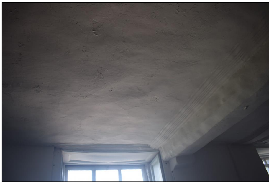
Fig. 22 Hand formed plaster detail in the first floor room on the north elevation Photo CPAT 4992-140
