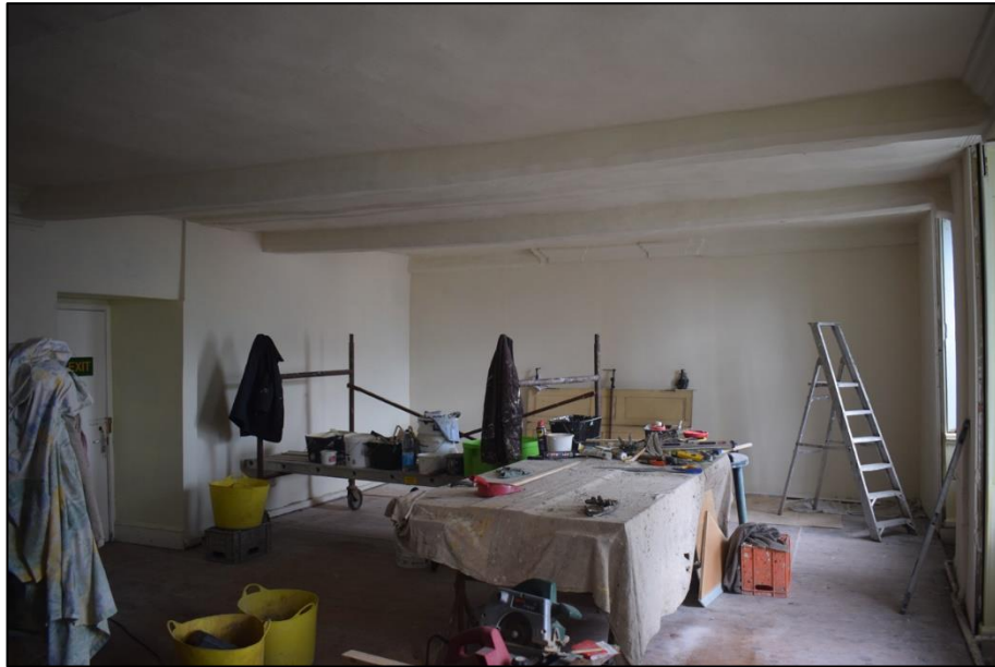
Fig. 8 First floor room within the main block Photo CPAT 4992-084
