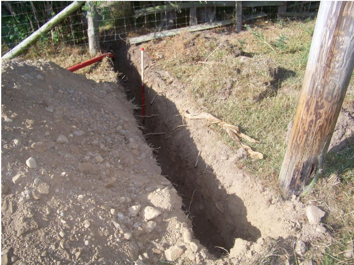
Fig. 3 Trench for pole 2. View to west. Photo CPAT 5030-6
