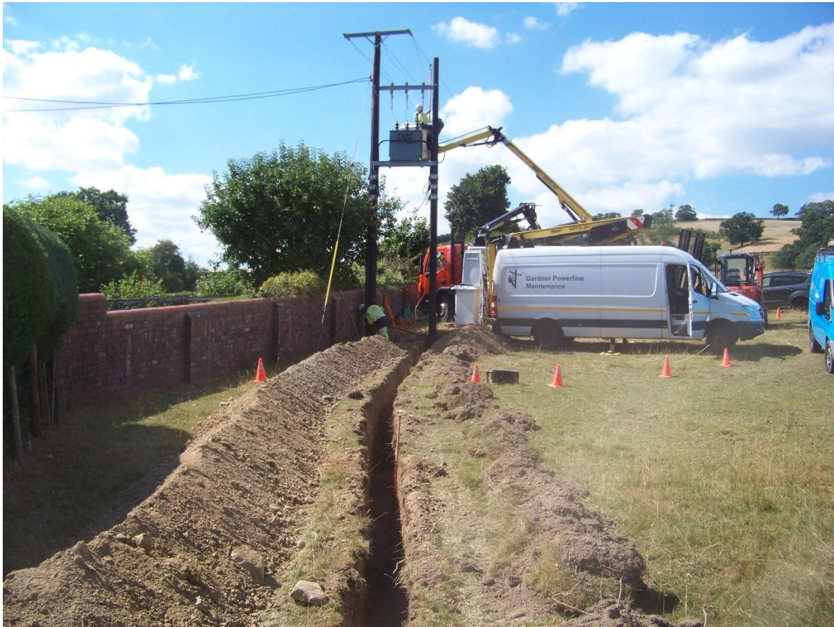
Fig. 4. Cable trench for pole 3. View to north-west. Photo CPAT 5030-2
