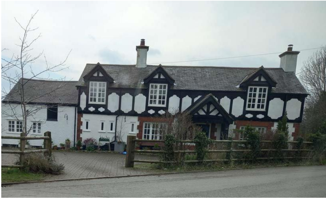
Fig. 4 The former Plough Inn looking east
