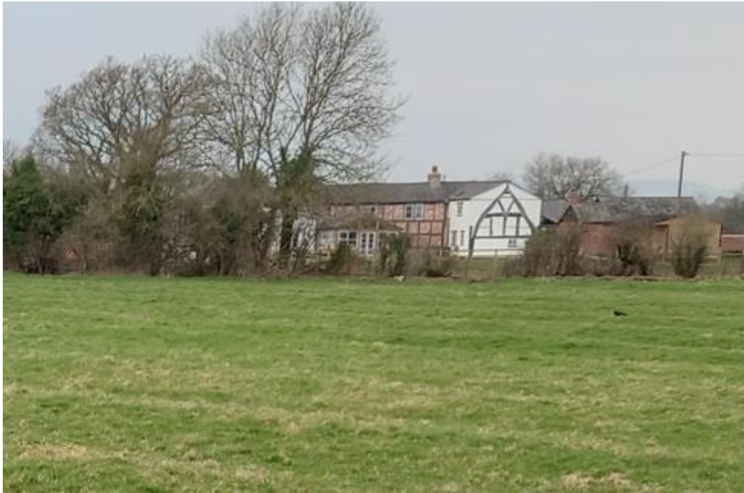
Fig. 2 The cruck- and timber-frame house at Chapel House Farm with ridge and furrow in field to east of it
