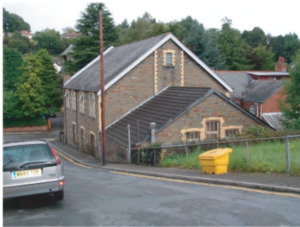
Reason for image General view of south and east elevations.
