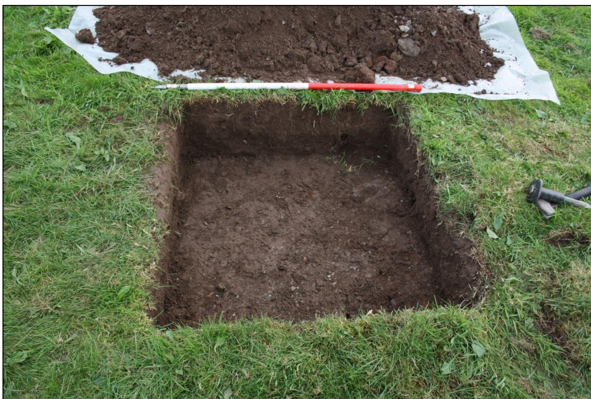
Figure 9: Site for new panel after excavation, facing S
