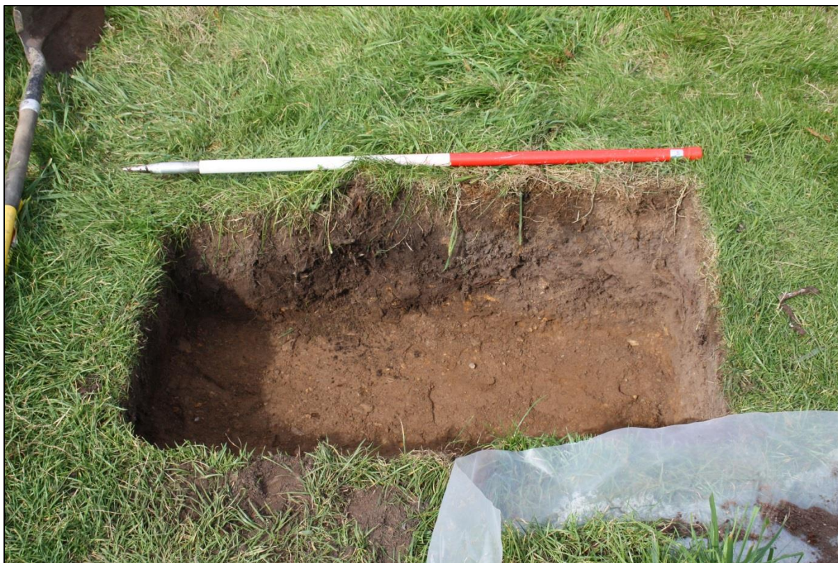
Figure 10: Trench for new panel, I after excavation, facing NW
