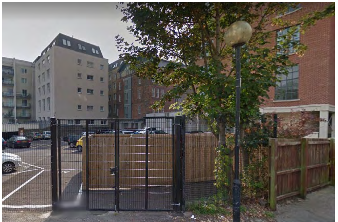
Plate 17: View of the rear of Empire House in the context of twentieth-century development
