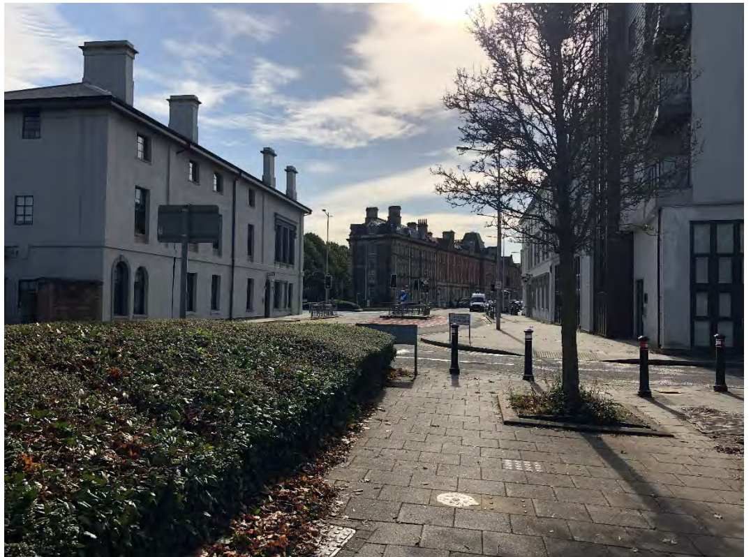
Plate 16: View of Cardiff Bay Station in the context of the Mount Stuart Conservation Area, looking south
