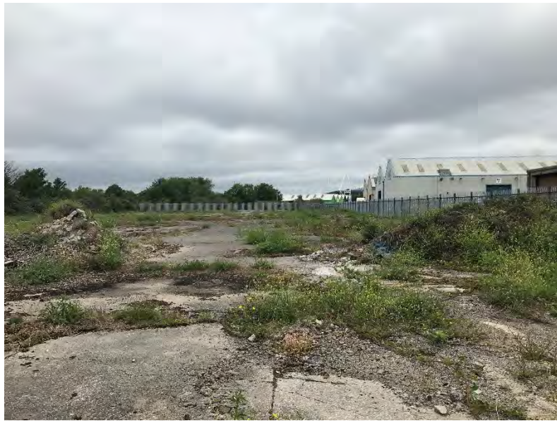
Plate 8: Hardstanding associated with the former foundry site adjacent to the embankment (looking north)
