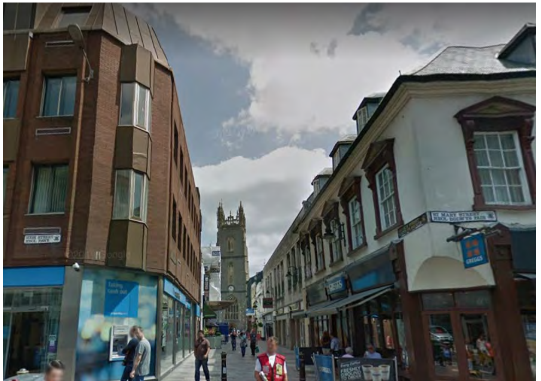
Plate 11: View of the Church of St John the Baptist from St Mary's Street
