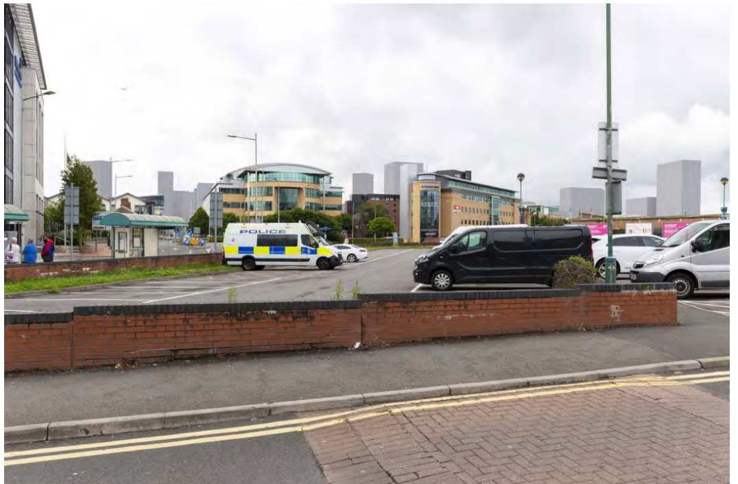
Plate 21: View from Cardiff Central looking south (Axis and Mason TVIA image No 6)
