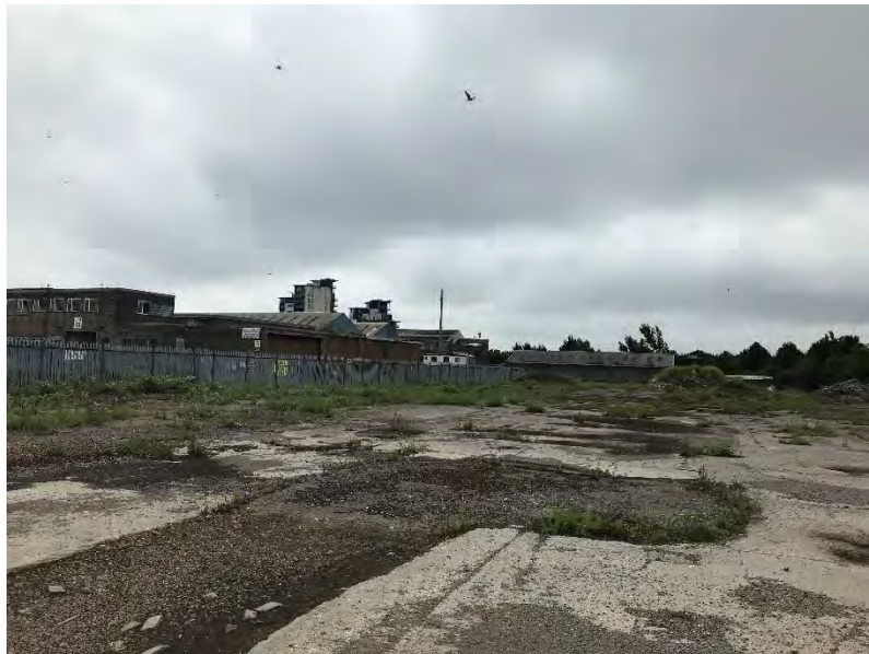
Plate 7: Hardstanding associated with the former foundry site adjacent to the embankment (looking south)
