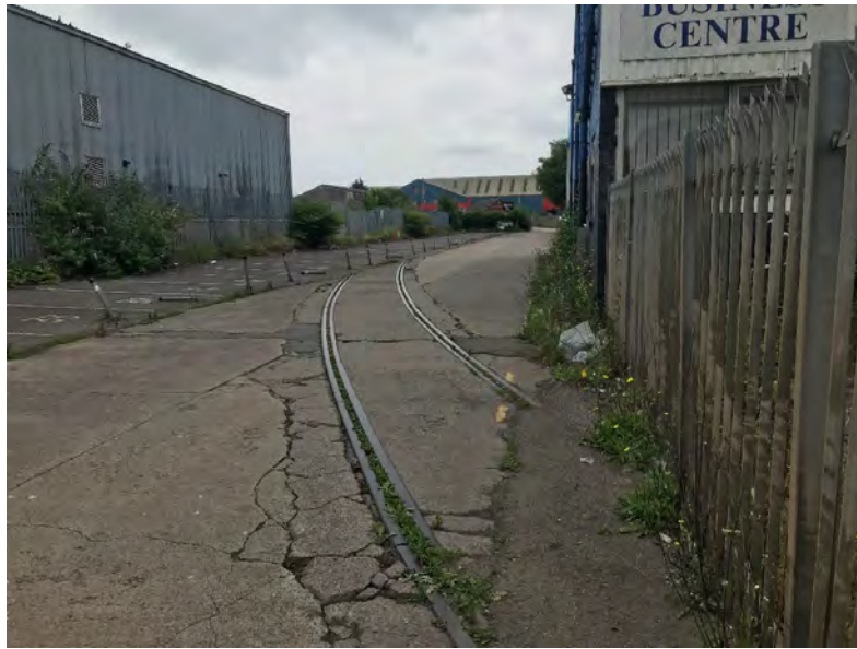
Plate 6: Surface evidence associated with the GWR (Riverside Branch) along Curran Road in the north-east of the study site (looking south)
