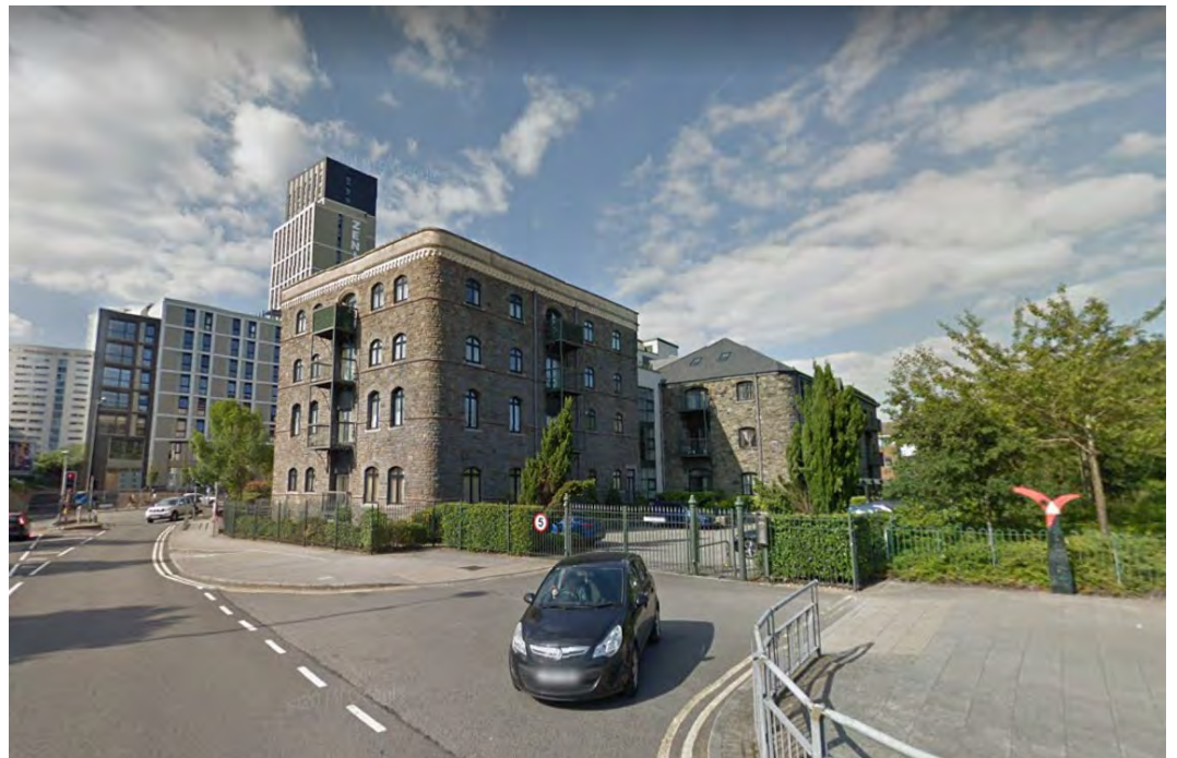
Plate 23: View of Grade II historic warehouses in the context of twenty-first century development in their vicinity, looking north-west
