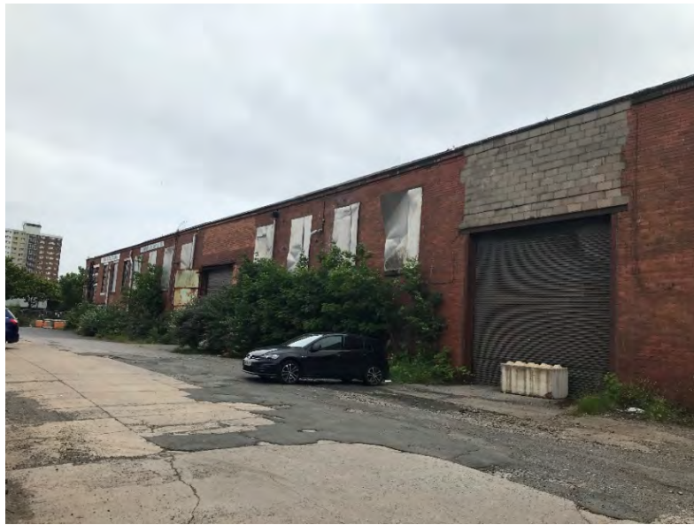
Plate 4: Northern elevation of mid-20 th century industrial unit associated with the Curran Engineering Works (looking south east)
