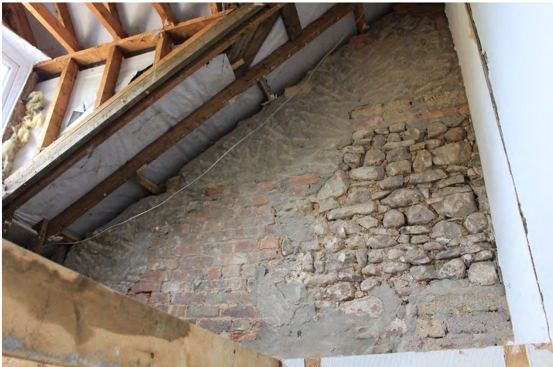
Image EDP A1.20: Upper part of the gable end in G2, looking south, showing brickwork rebuilding/extension here. Also showing the 20 th century roof.
