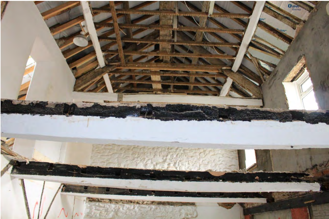
Image EDP A1.7: View of the 19 th century timber joists of the upper floor in G1, looking south.
