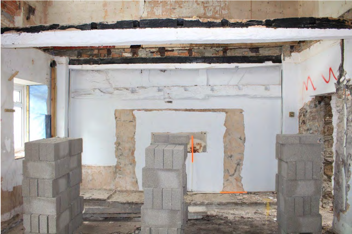
Image EDP A1.12: View of the northern gable, looking north and showing the earlier, lower timber beam and the later raised floor above.
