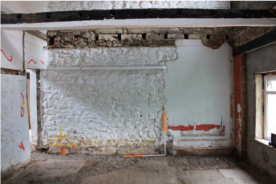
Image EDP A1.10: View of the lower part of the southern gable in G1, looking south. Showing the inserted joist holes to take the later floor.
