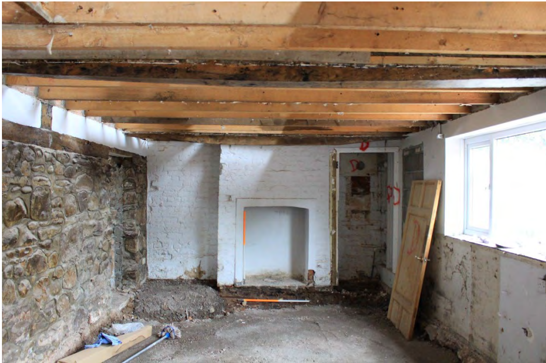
Image EDP A1.16: General view of room G2 looking north, showing the stone spine wall with timber frame on top to the left and brick fireplace on the northern wall. The right-hand wall is rendered blockwork.
