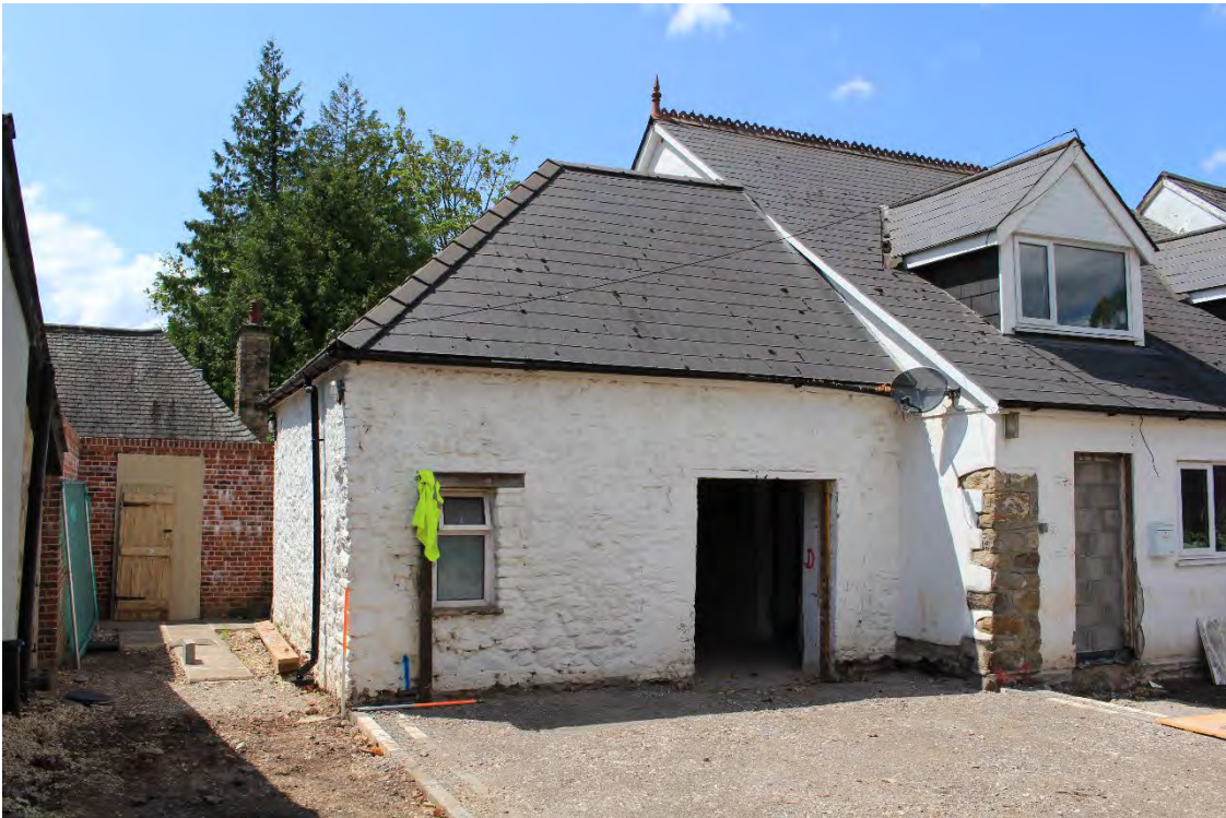
Image EDP A1.25: Eastern and western elevations of the 'coach house' section, looking west, showing the two openings in the eastern wall and the plain southern wall.
