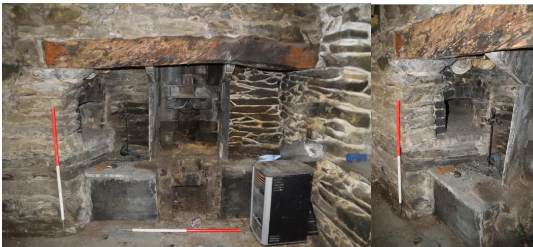
Figure 9: Inglenook style Fireplace (left) and bread oven in room 1B (right) (CPAT photo 5079-023 and 24).
