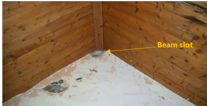
Figure 13: West facing internal gable wall showing beam slot at the apex of the roof. (CPAT Photo 5079-075)
