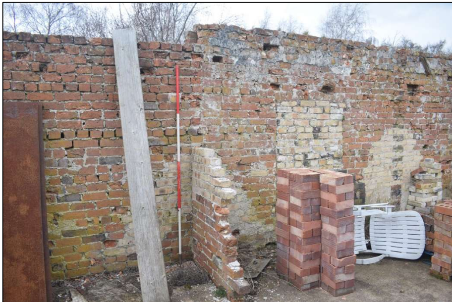
Fig. 7 Internal partition within the northern section of the building Photo CPAT 5040_024
