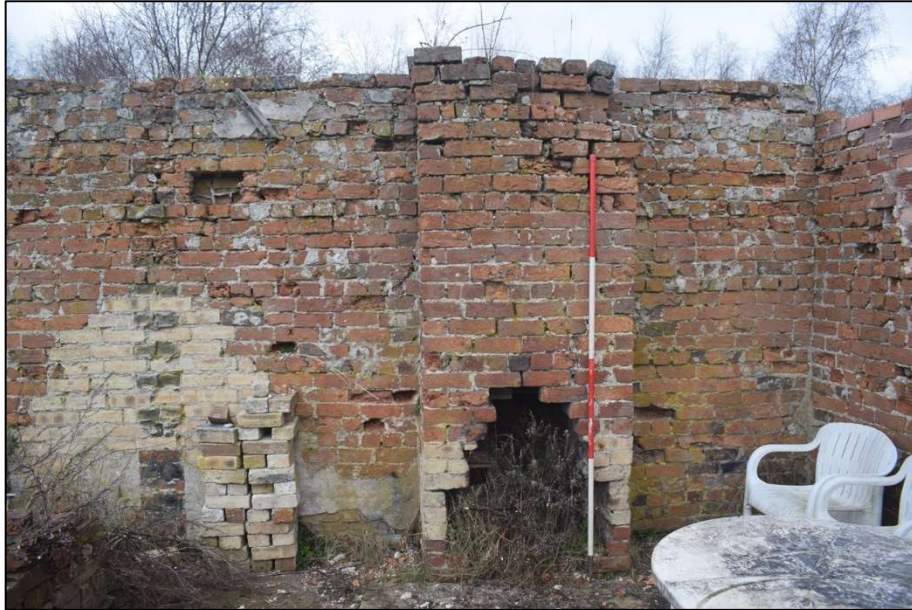
Fig. 8 Chimney stack at northern extent of the building Photo CPAT 5040_028
