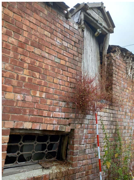
Fig. 12 West elevation of Barn and Cart Shed showing change in brickwork, open and infilled ventilation slots, windows and first floor doorway (CPAT 5005-023 and 025)
