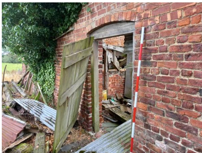
Fig. 9 Interior of southern gable to barn and old brickwork along walls (CPAT 5005-014); change in brickwork in west elevation around the inserted doorway (CPAT 5005-010 and 018)
