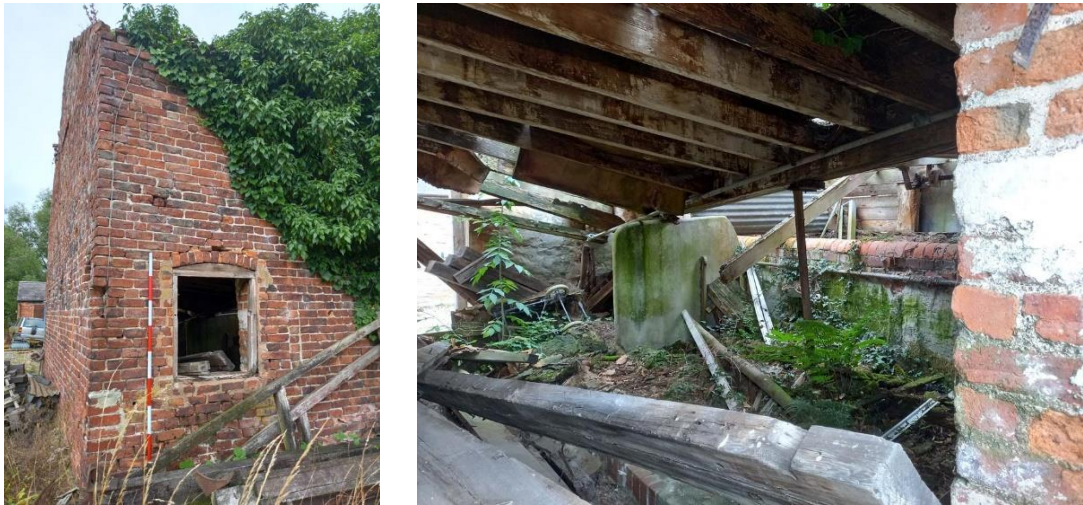
Fig. 5 Window at north-west corner and view through it to cow stall and plinth, with collapsed hay loft (CPAT 5005-007 and 008)
