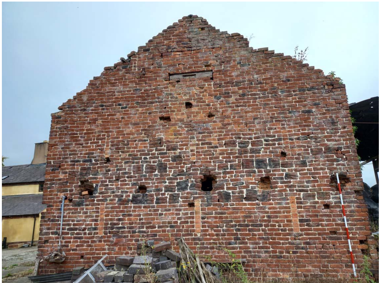
Fig. 4 North-facing gable end of cow house; note joist holes, infilled ventilation slots and window (CPAT 5005-006)
