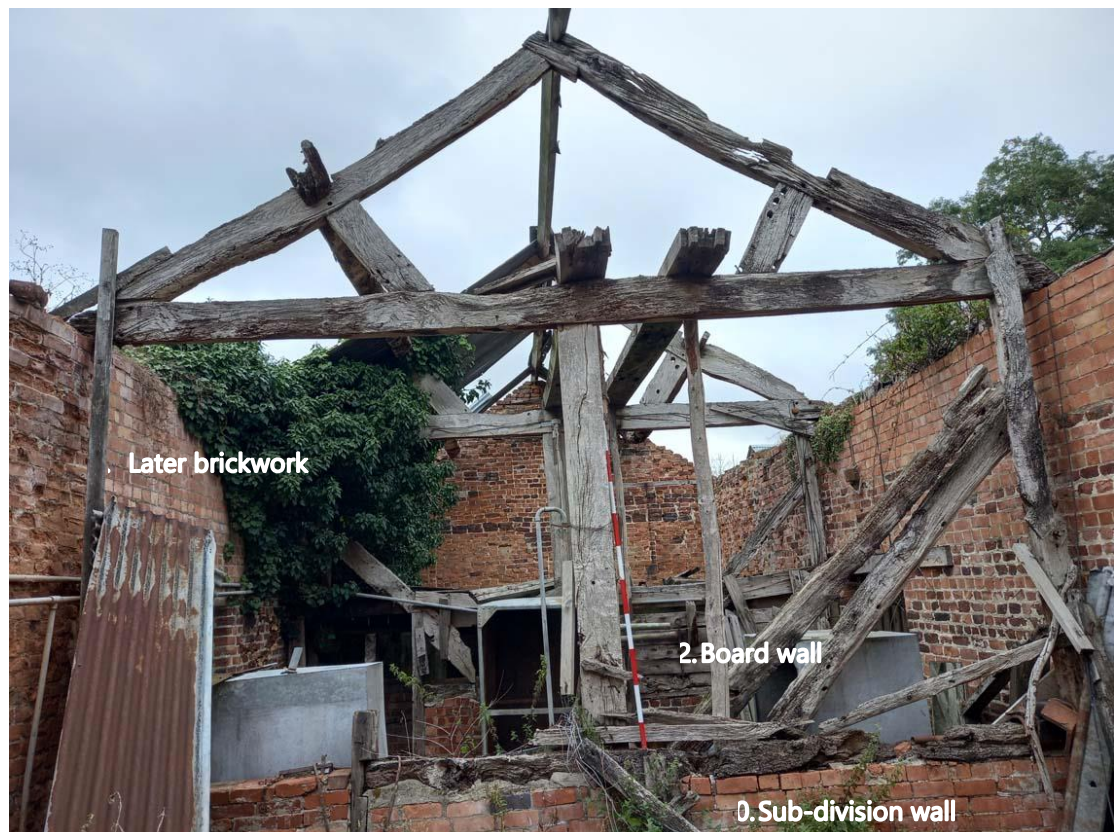
Fig. 10 Interior of barn showing raking Queen Post roof trusses (CPAT 5005-039)
