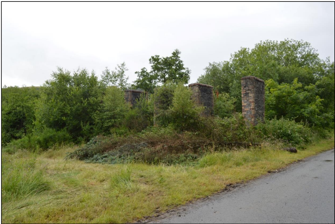
Fig. 8: The piers (PRN 214949) that once carried a tramway across the mine site, from the north. CPAT 4999-0001
