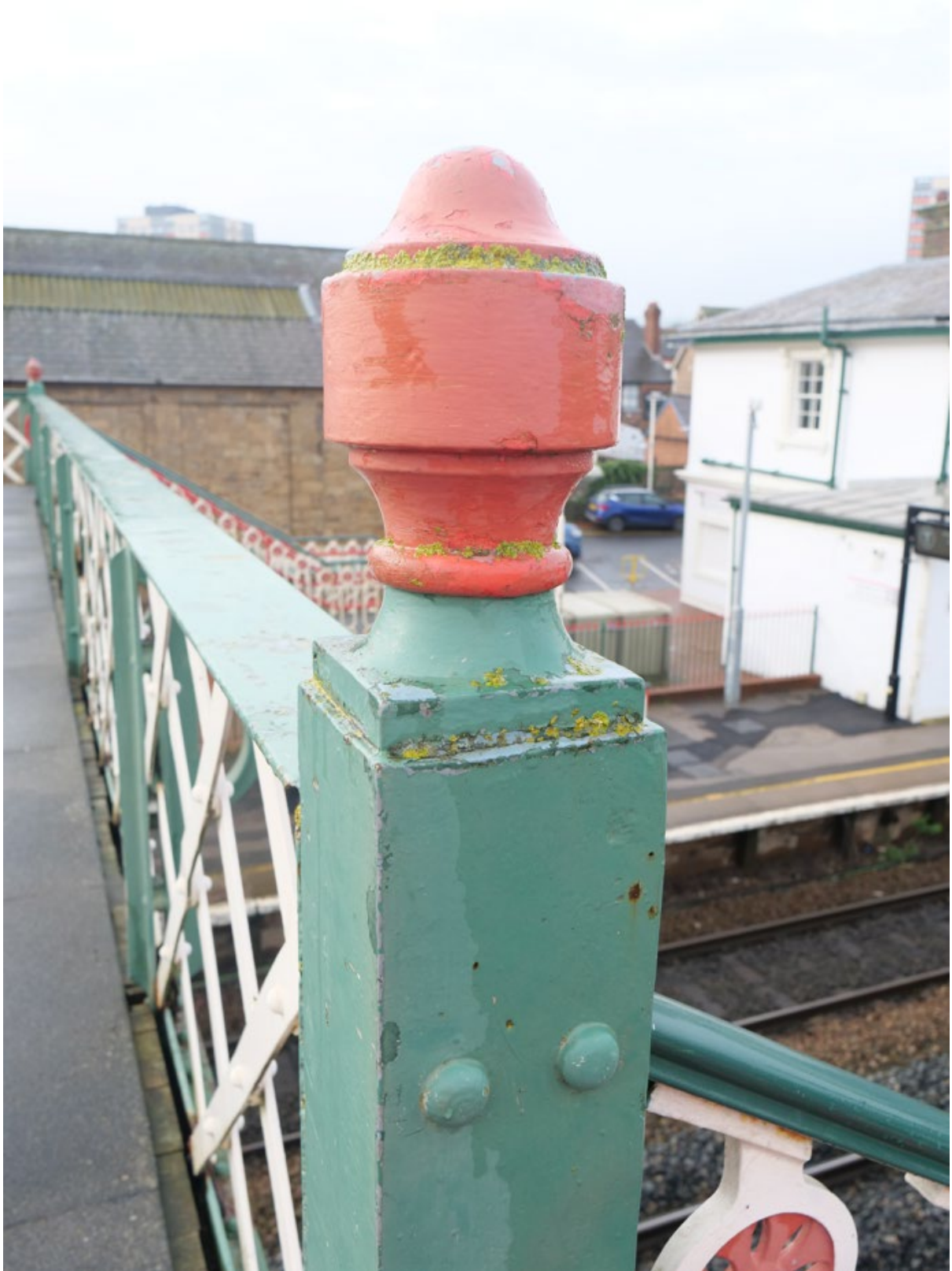
Plate 15: Detail of decorative cast iron parapet finial, looking southwest
