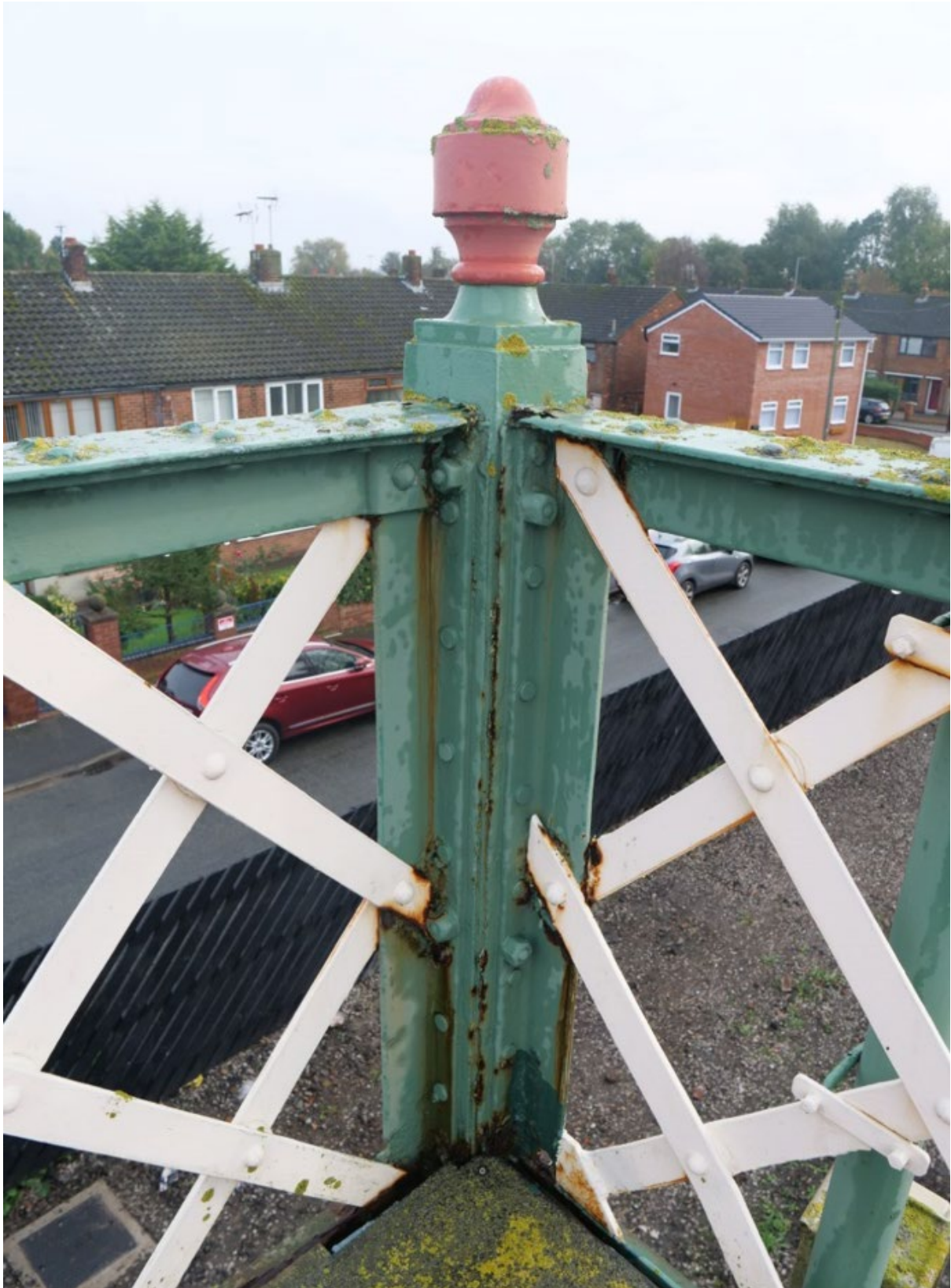
Plate 14: Decorative cast iron finial at the southeast corner of the parapet (Platform 1), looking southeast
