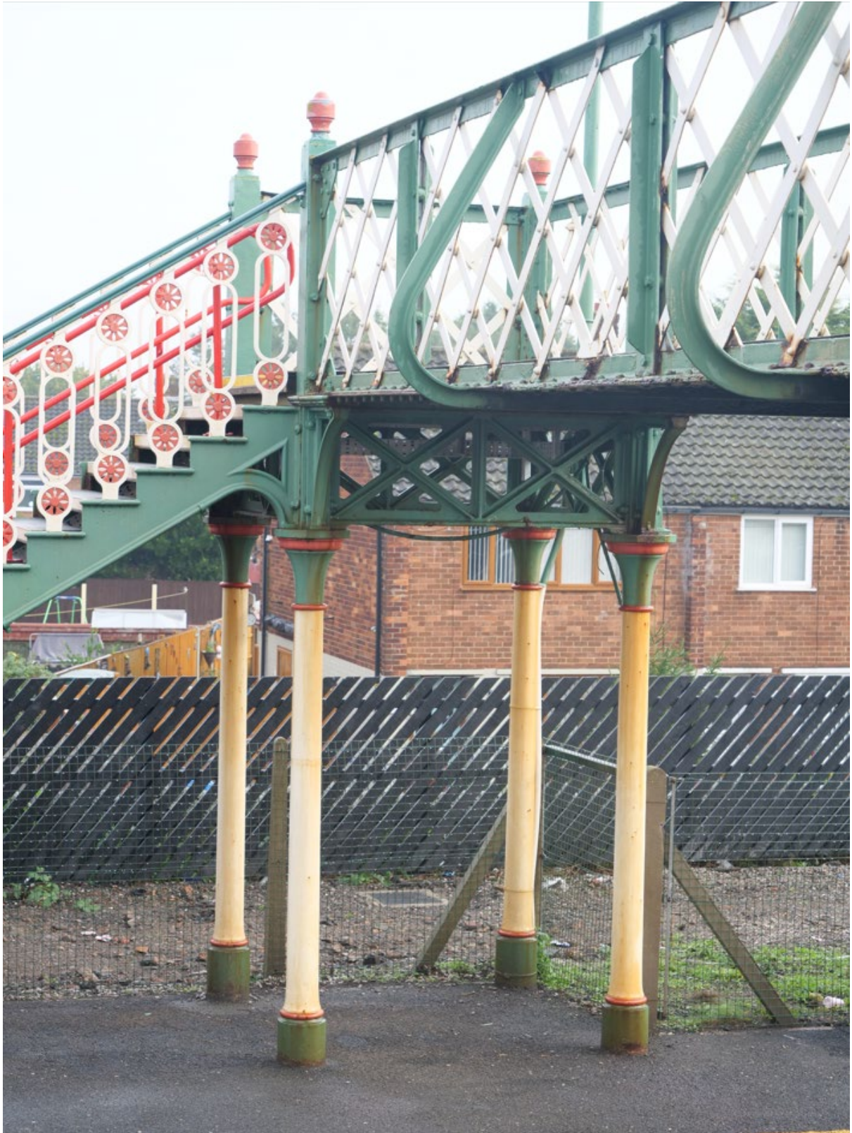
Plate 4: The northeast bridge pier and columns, looking northeast from Platform 2
