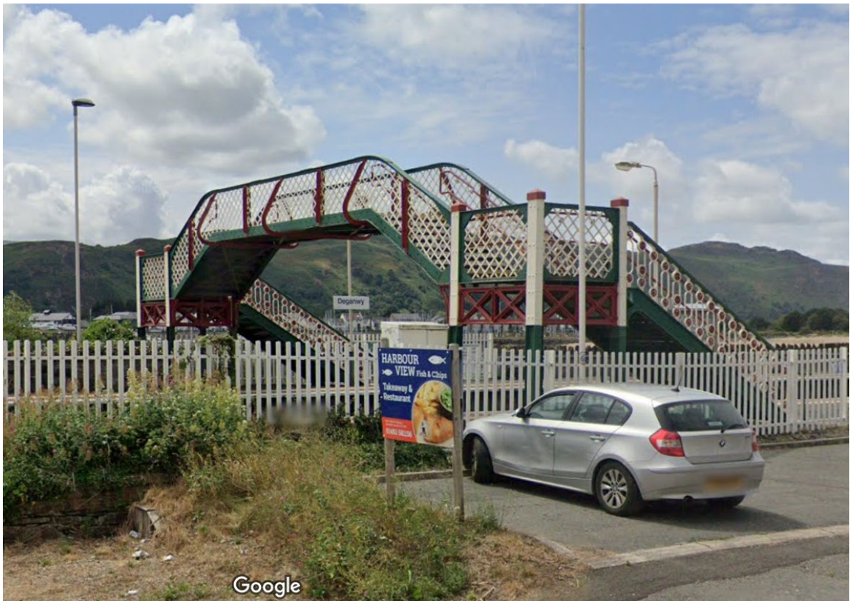
Historical Plate 6: Deganwy Station footbridge, view from Station Road, June 2023 © 2023 Google
