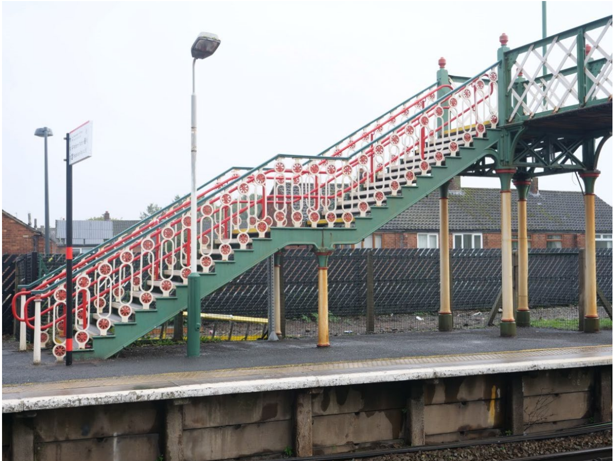
Plate 17: Northeast staircase (Platform 1), looking east from Platform 2
