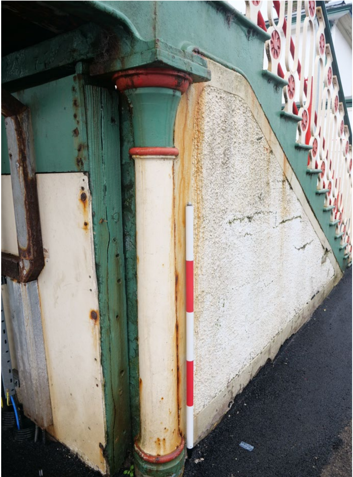
Plate 19: Cast iron column and enclosed void under southwest staircase (Platform 2), looking southwest
