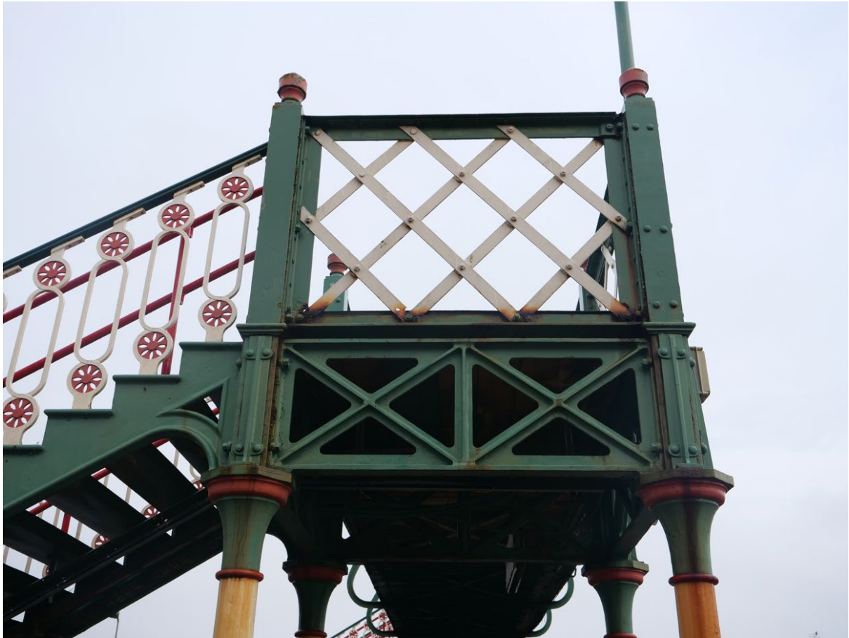
Plate 6: The southwest bridge pier/tower (Platform 2), showing the cross girders atop the cast iron column capitals, looking northeast
