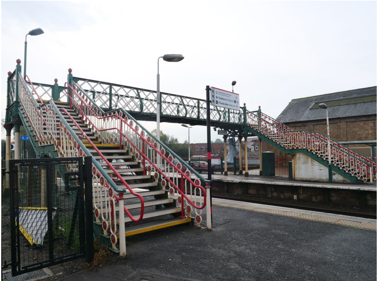
Plate 2: General view of the station footbridge, looking southwest from Platform 1
