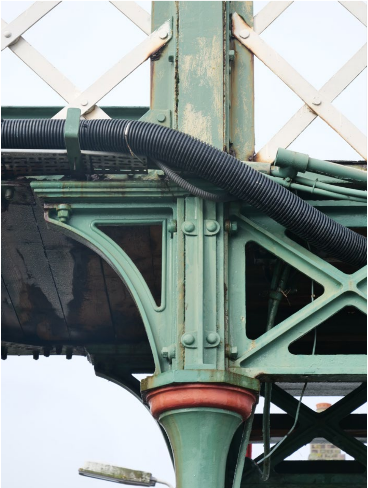
Plate 9: Detail of deck bracket on northeast bridge pier/tower (Platform 1), looking northwest
