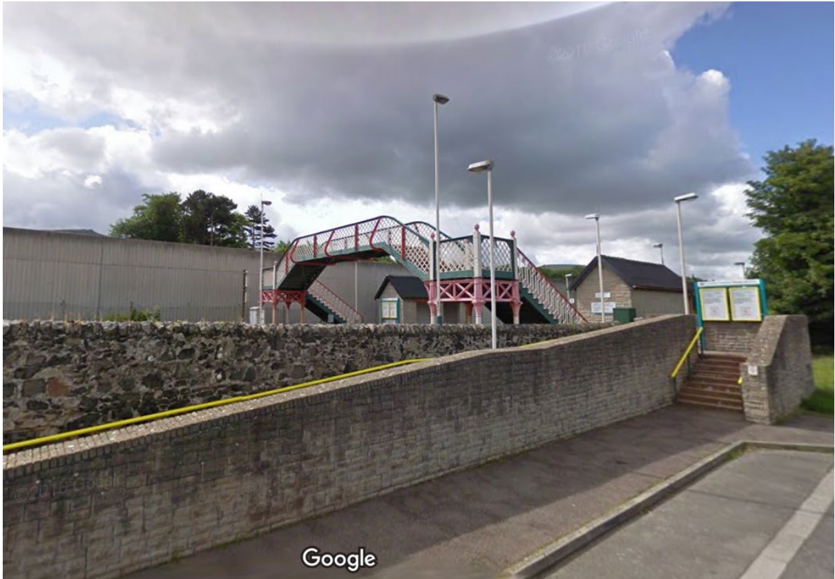
Historical Plate 5: Llanfairfechan Station footbridge, looking southwest from West Shore, June 2011 © 2023 Google
