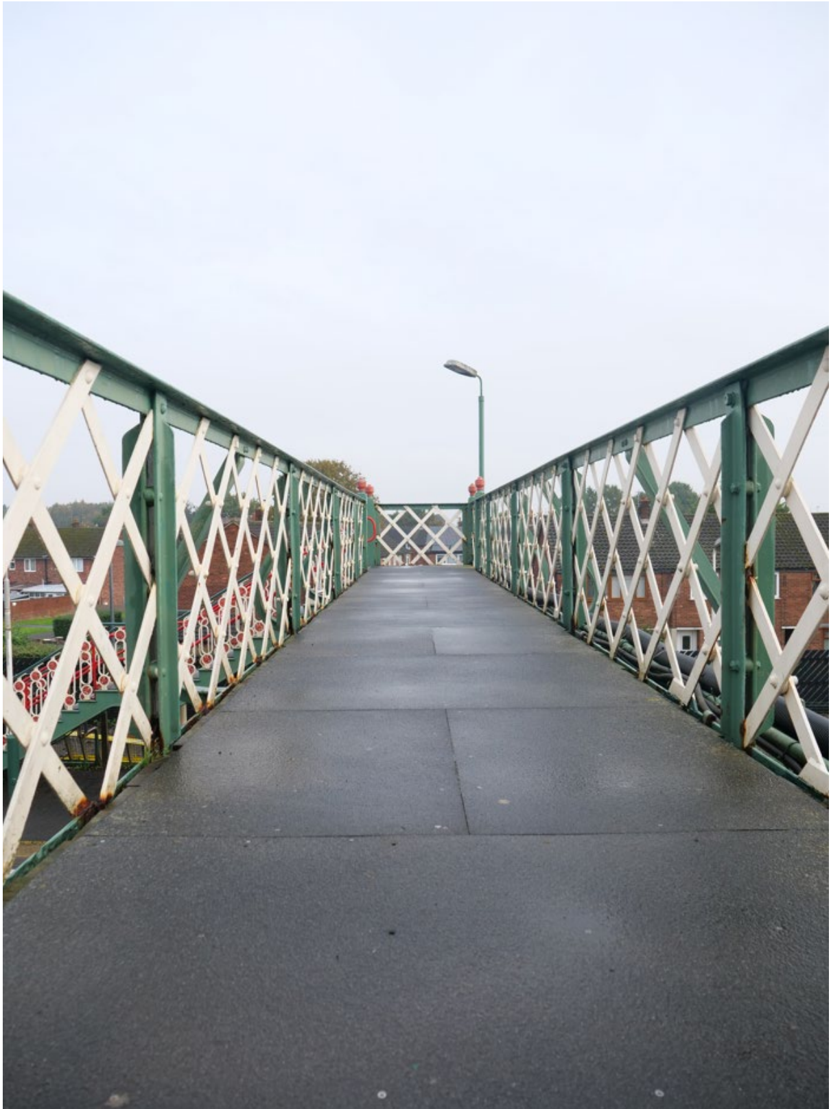
Plate 11: Top deck of the footbridge, looking northeast, showing modern surface
