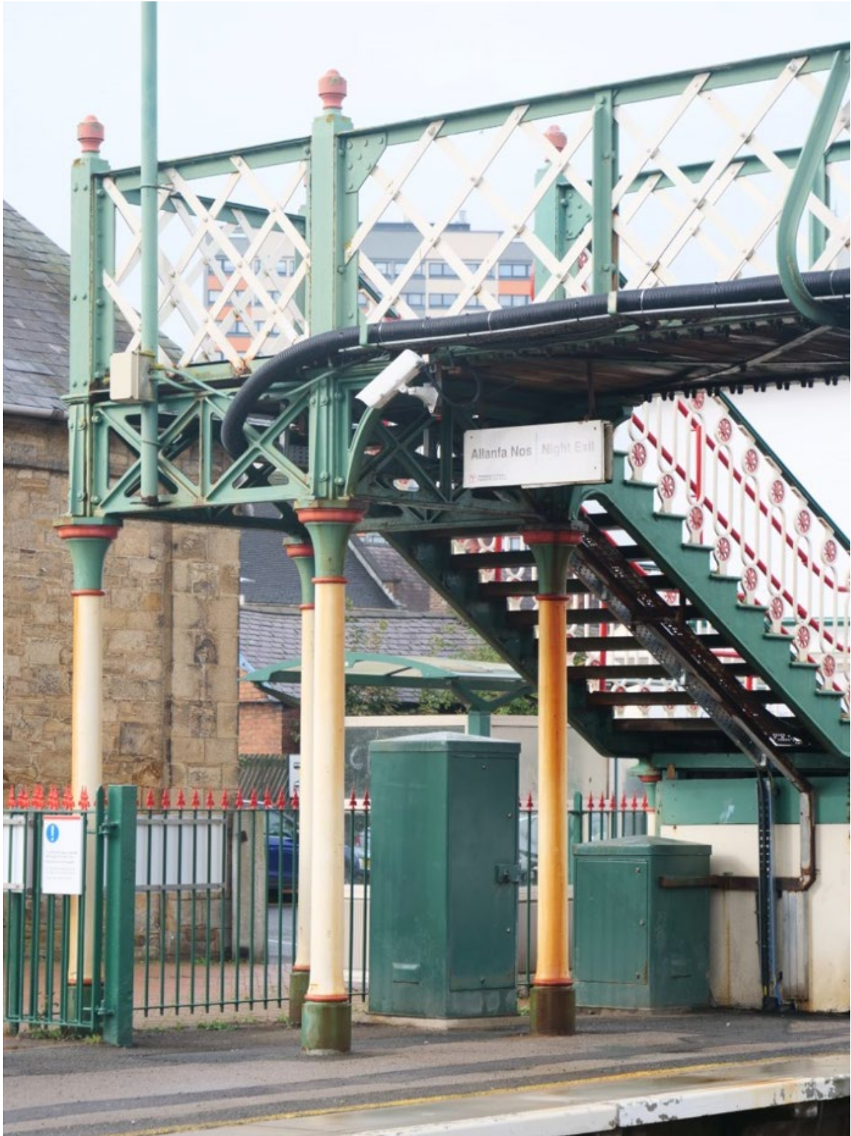
Plate 5: The southwest bridge pier and columns, looking southwest from Platform 1
