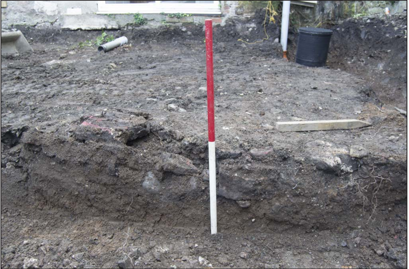
Plate 31: West facing section of drainage trench showing stones and cobbles of yard surface; scale 1x1m; view from W (archive reference: G2766_061).
