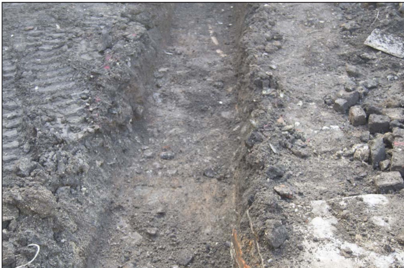
Plate 35: Central drainage trench; scale not used; view from N (archive reference: G2766_069).
