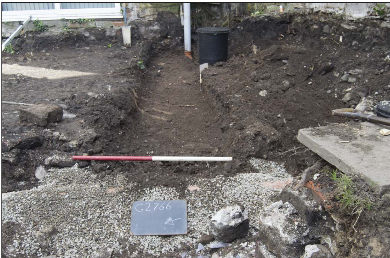
Plate 42: Southern foundation trench; scale 1x1m; view from W (archive reference: G2766_086).
