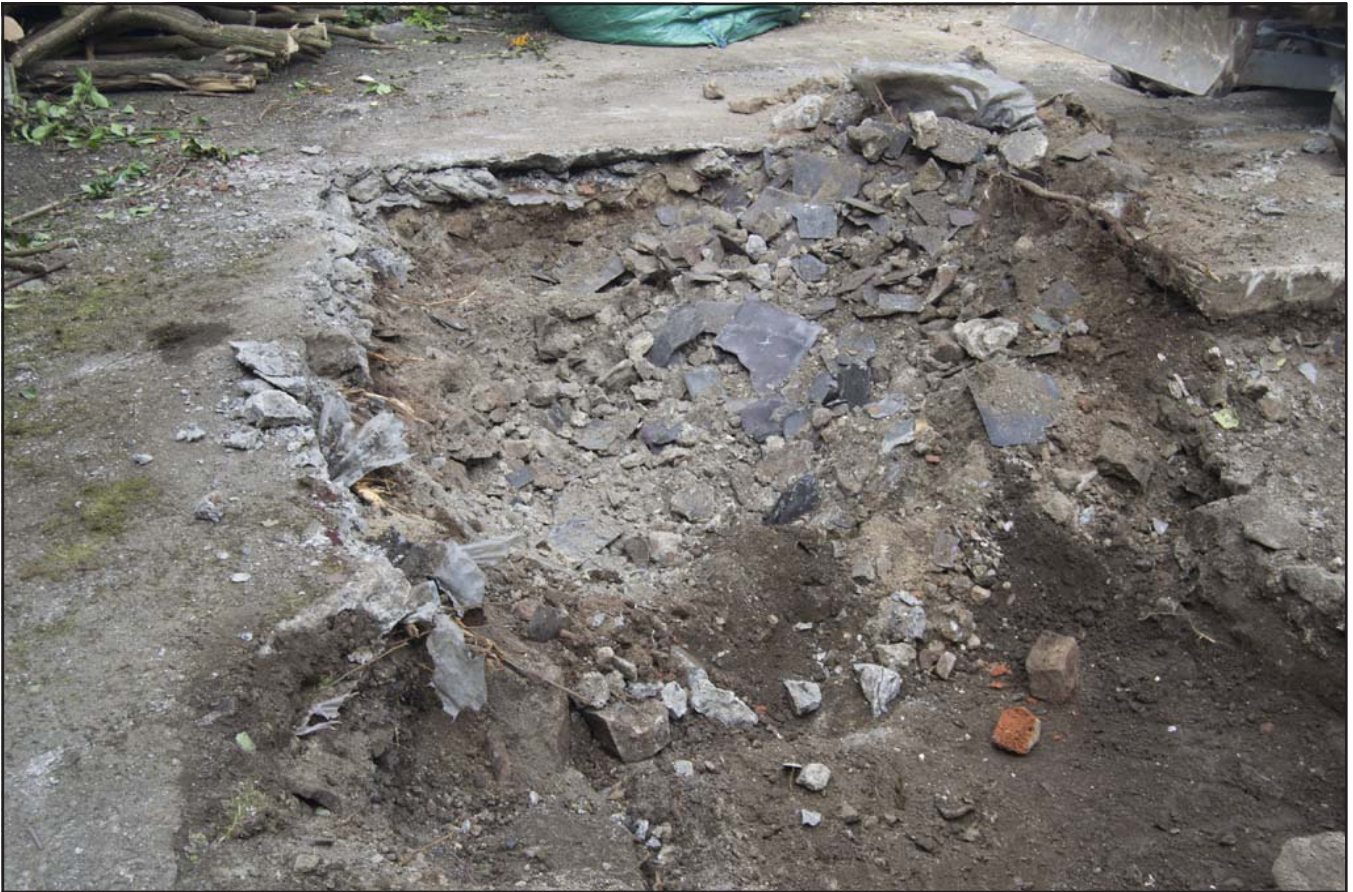
Plate 11: Working shot - view of demolition debris at west end of extension area; scale not used; view from E (archive reference: G2766_017).
