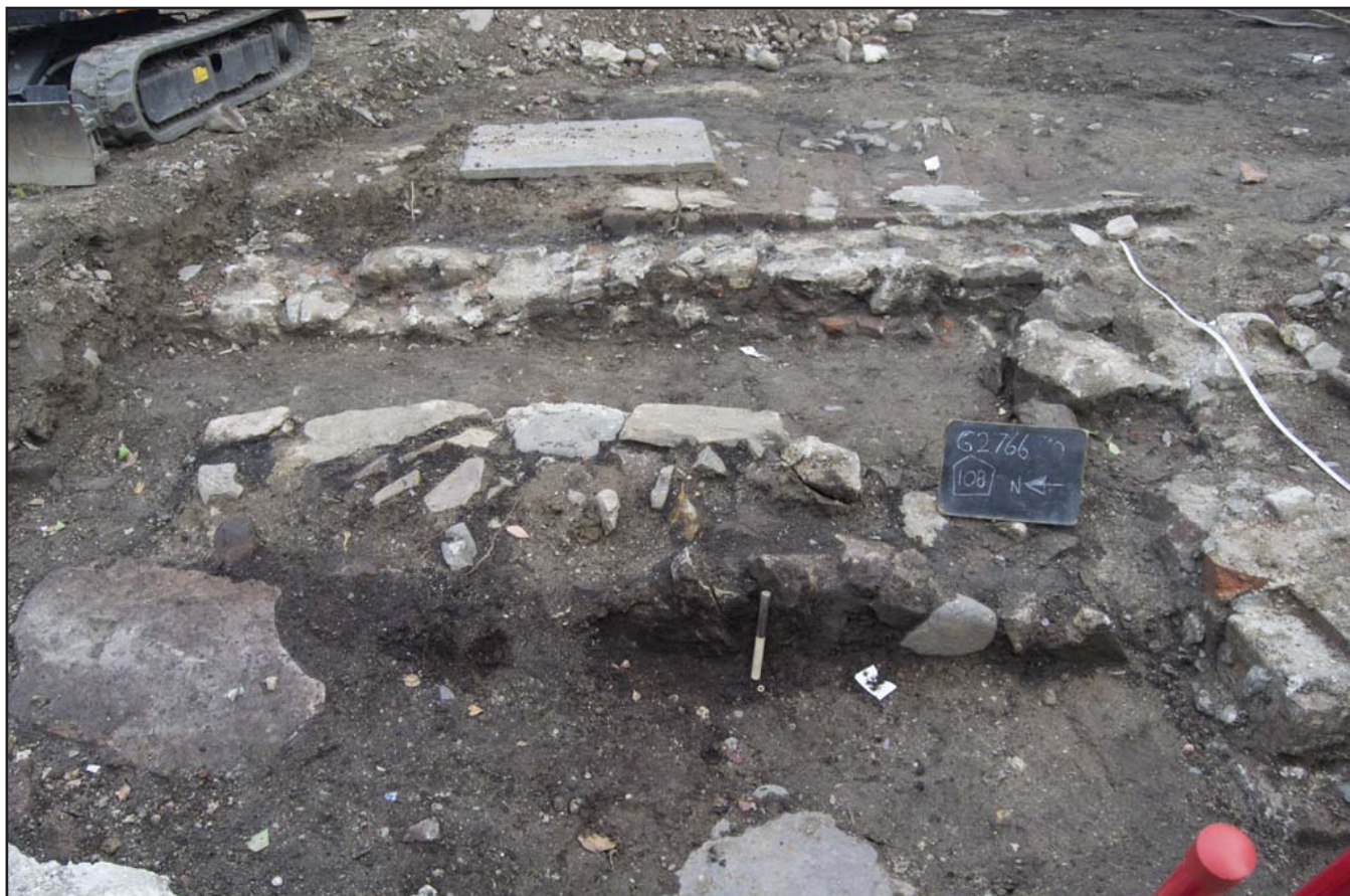
Plate 21: West facing elevation of wall 108; scale 1x0.3m; view from W (archive reference: G2766_040).
