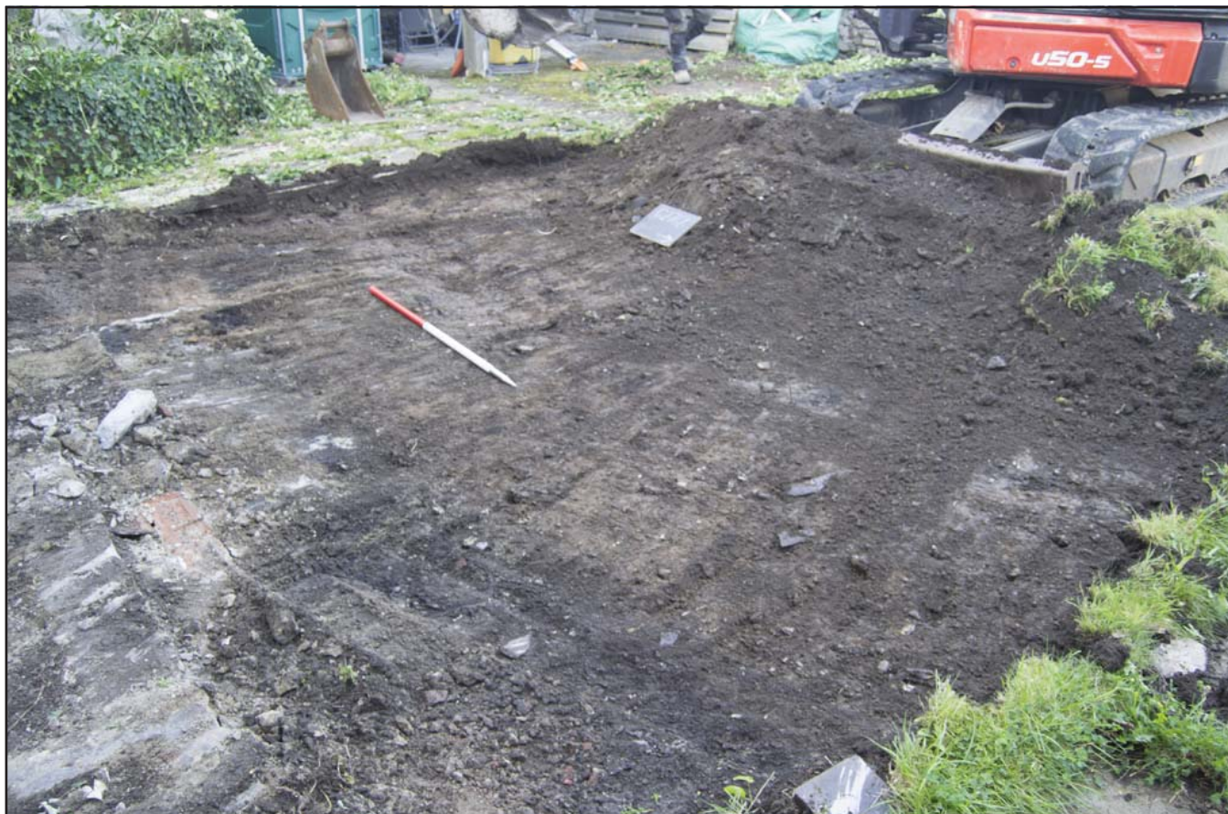
Plate 5: View of stripped area mid-excavation; scale 1x1m; view from NE (archive reference: G2766_005).
