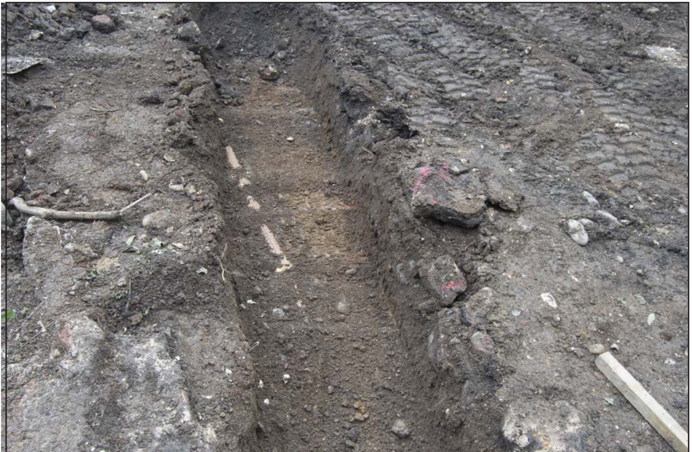
Plate 32: Length of central drainage trench showing modern waste pipe; scale not used; view from S (archive reference: G2766_063).
