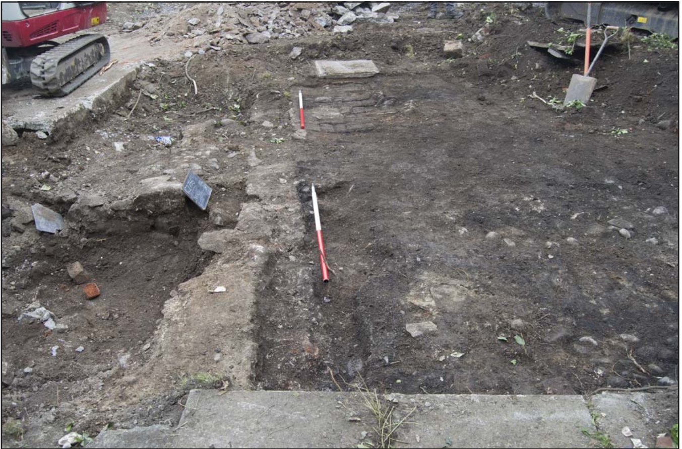
Plate 17: Mid-ex shot of western end of extension area showing wall and yard area; scale 2x1m; view from S (archive reference: G2766_024).
