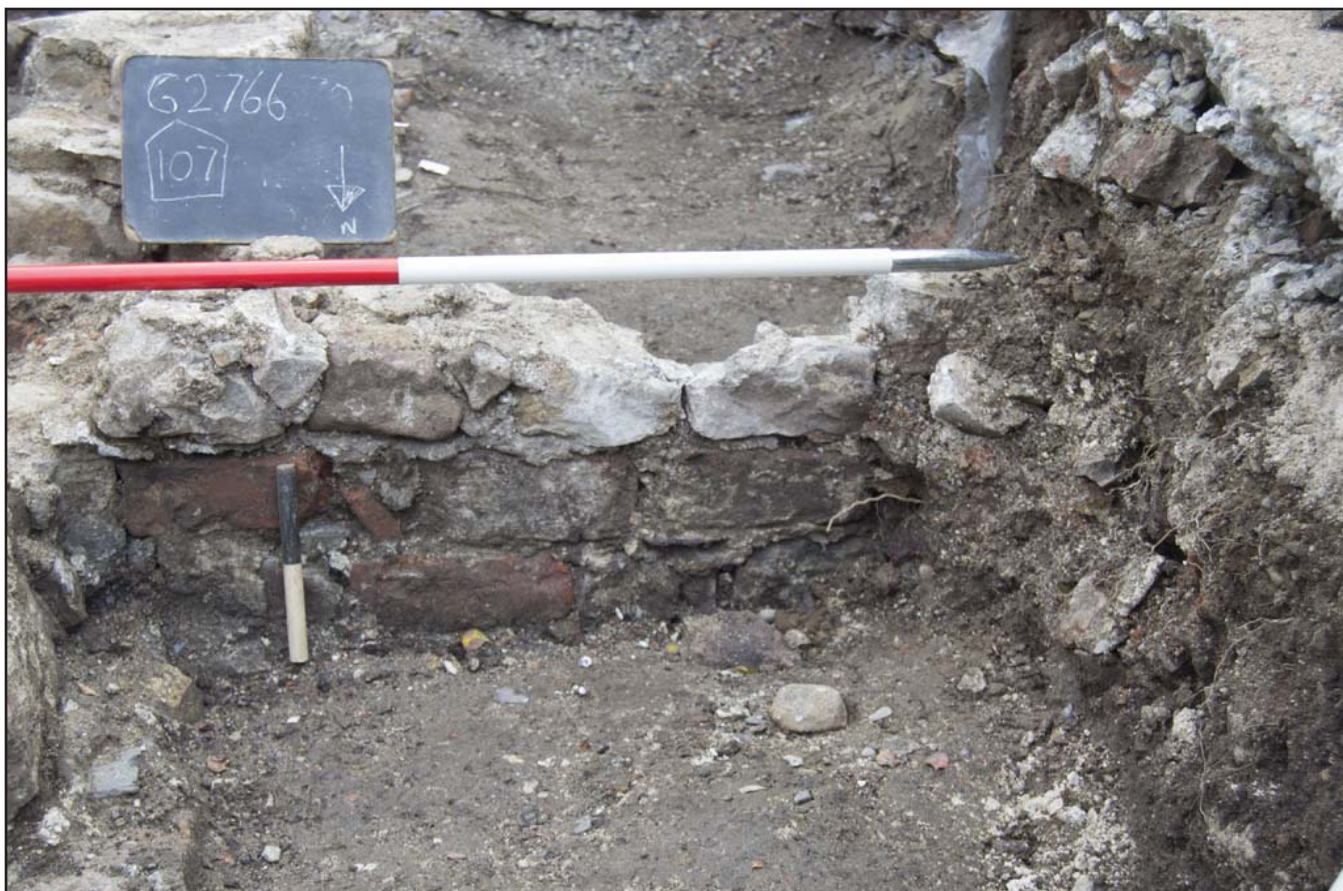
Plate 22: South facing elevation of wall 121 with 107 in the background; scale 1x0.3 & 1x1m; view from N (archive reference: G2766_041).
