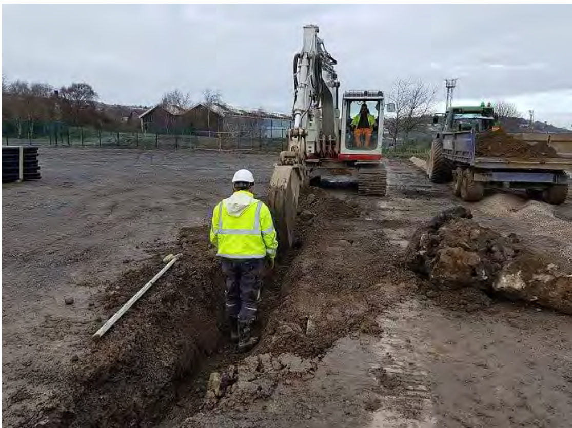
Photo 2: View north, excavation of drainage trenches in progress.
