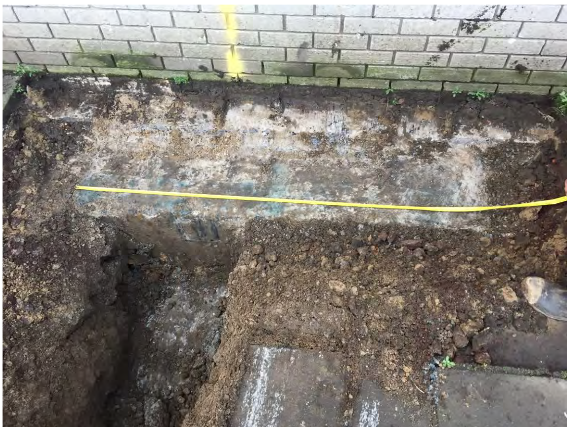
Photo 10: View south, foundation excavations on north side of the school, exposing pre-existing foundations.
