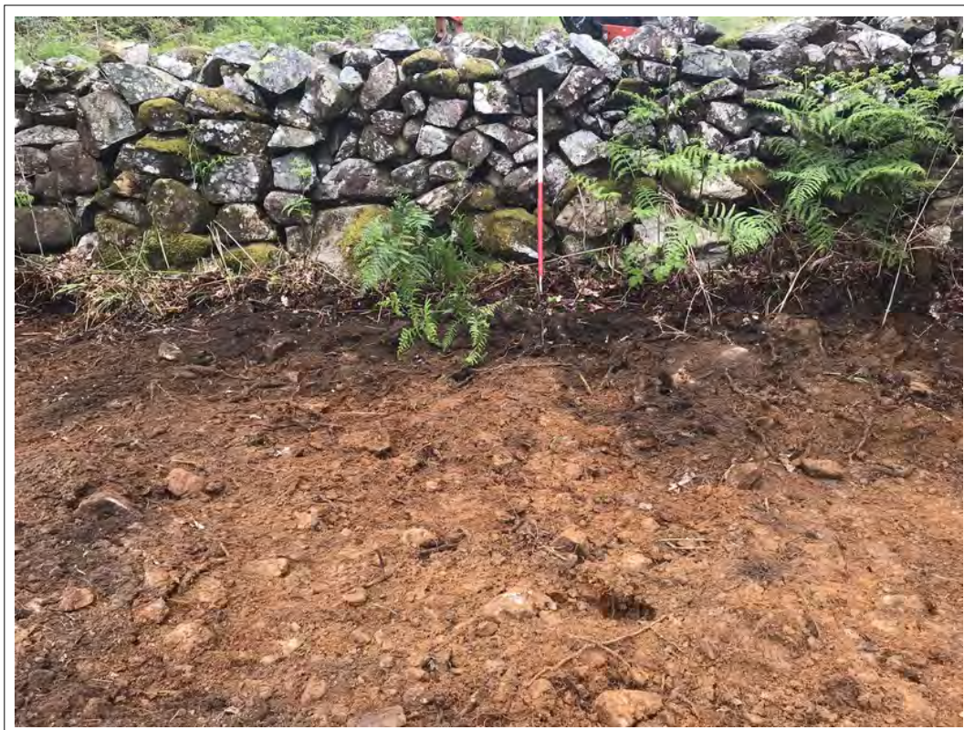
Plate 3. Dry-stone wall (103). View north. 1m scale
