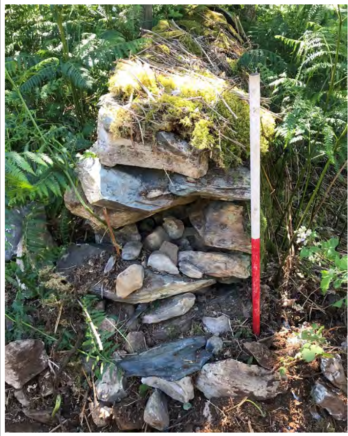
Plate 21. Dry-stone wall (203). View east. 1m scale
