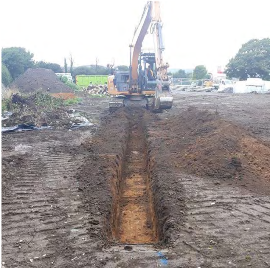
Photo 1: The initial trench, Trench 1 across plots 1 and 2, under excavation. Looking north.
