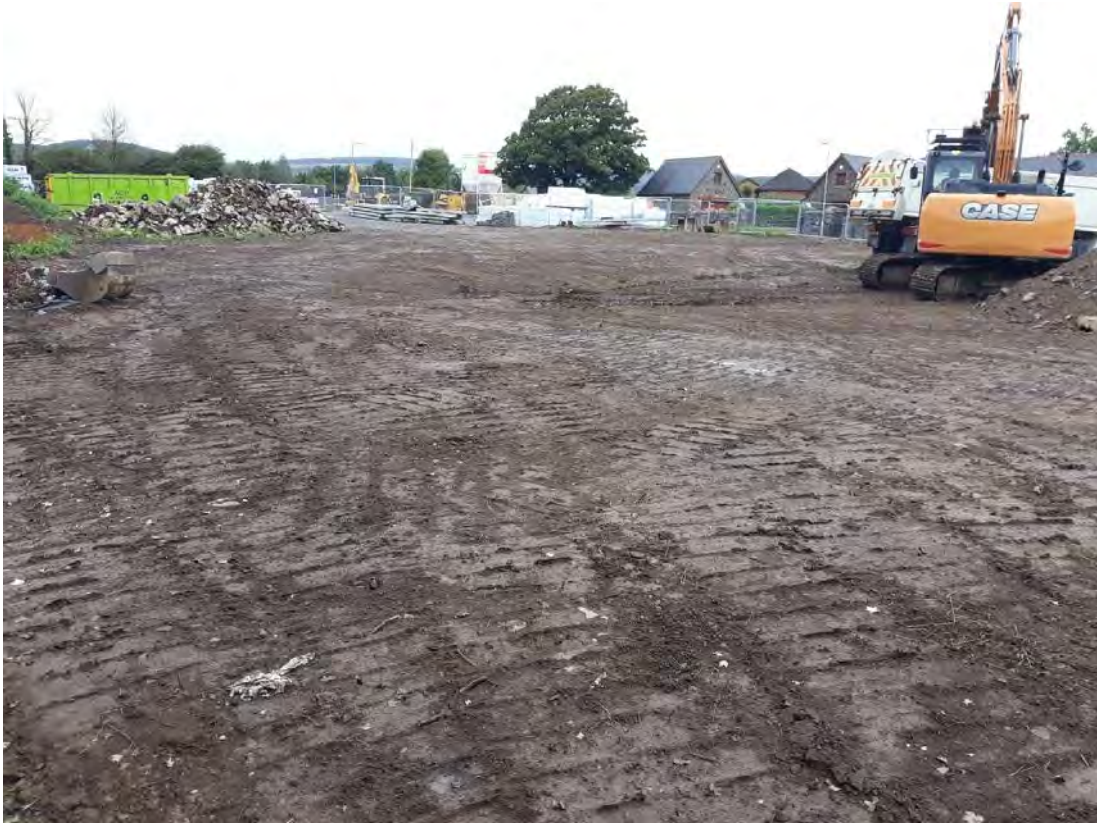
Photo 15: View across Plots 9 & 10, after initial topsoil strip, looking north.
