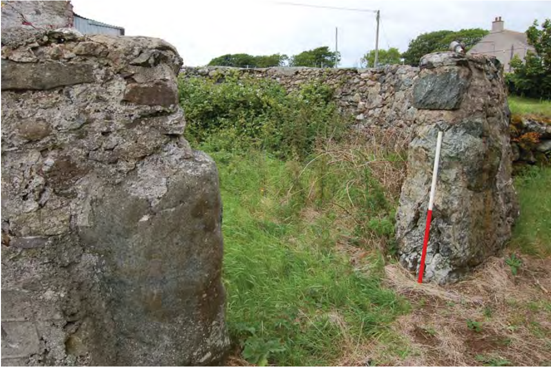
Plate 8. Stone enclosure entrance, view SW. 1m scale
