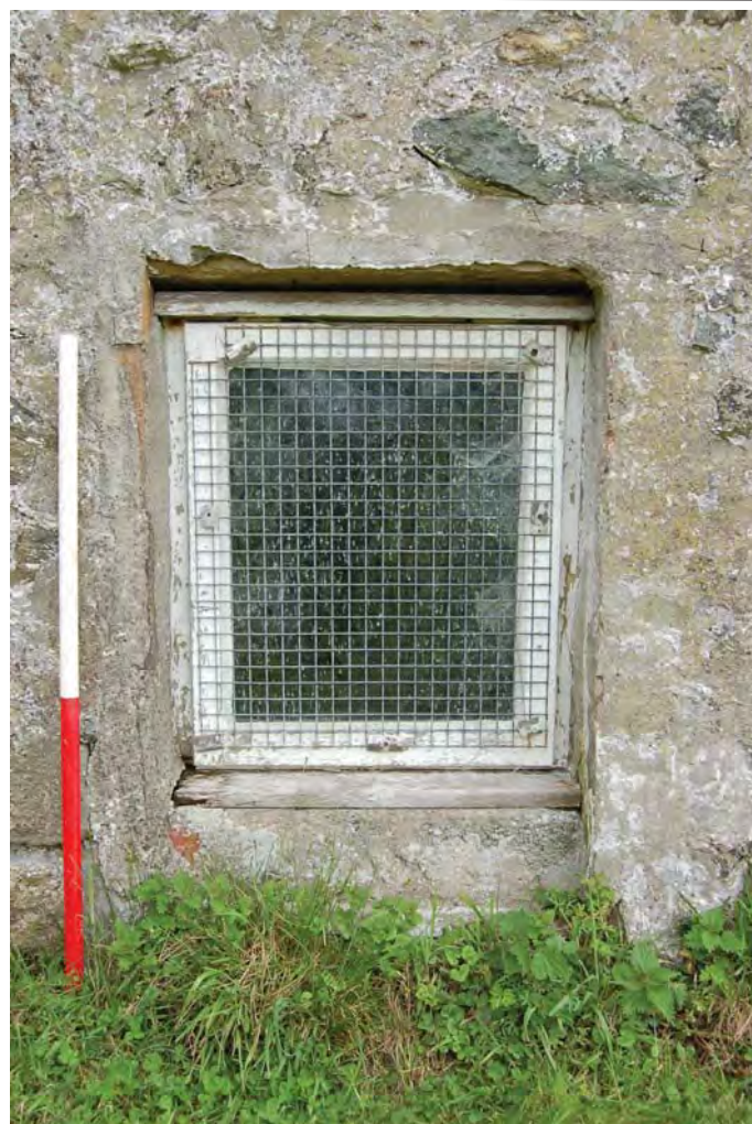
Plate 51. Main Range NW end window. View NE. 1m scale
