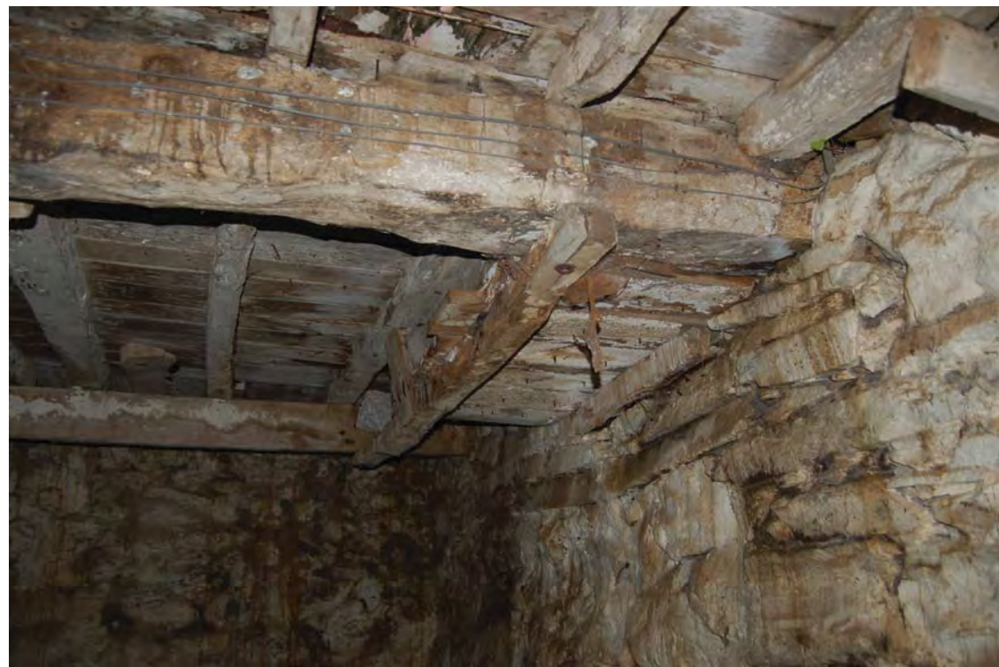
Plate 40. Interior of Room 2 of main range, stepped ceiling view S.
