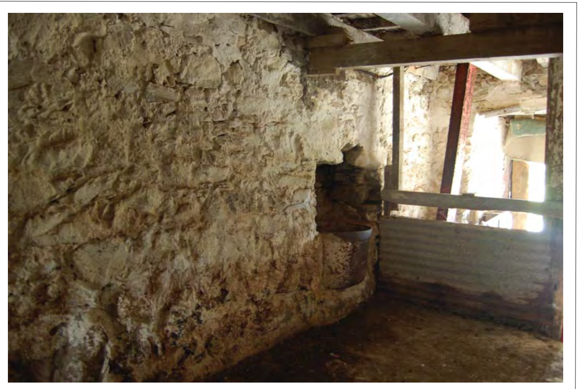
Plate 42. Interior of Room 3 of main range, iron trough, view NE.
