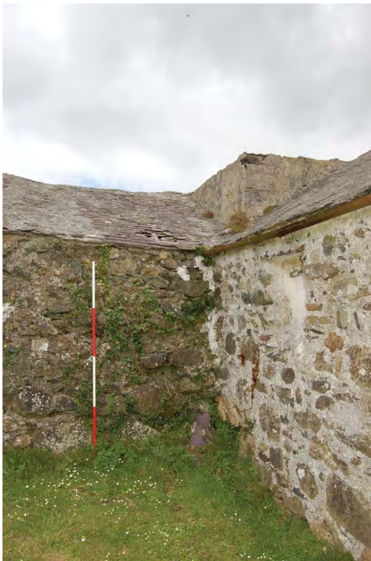
Plate 58. West Range join with Main Range. View NW. 2m scale
