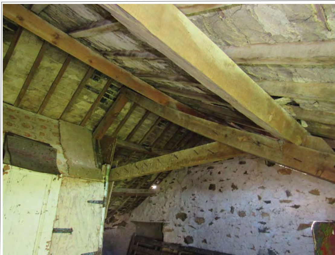
Plate 66. Room 8. Blocked door to Room 7 and roof structure. View SE
