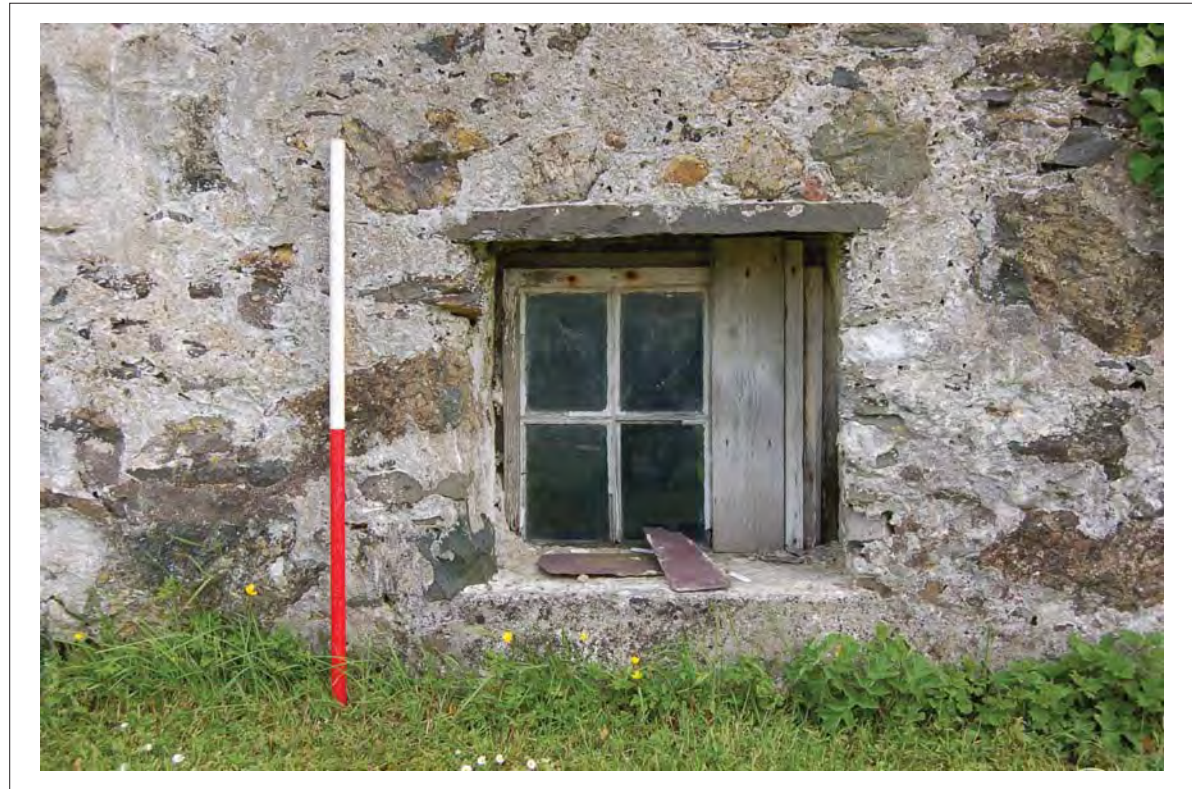
Plate 54. Main Range SE end window. View NE. 1m scale
