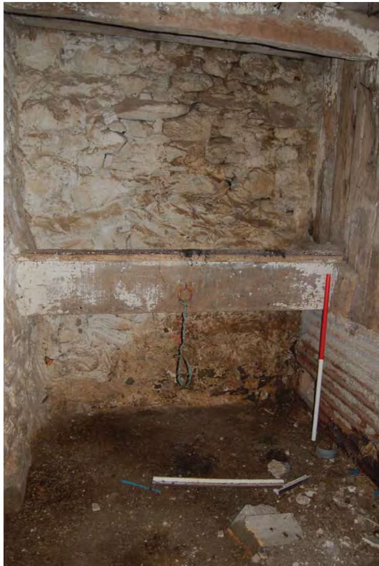
Plate 34. Interior of Room 2 of main range, manger, view SE. 1m scale
