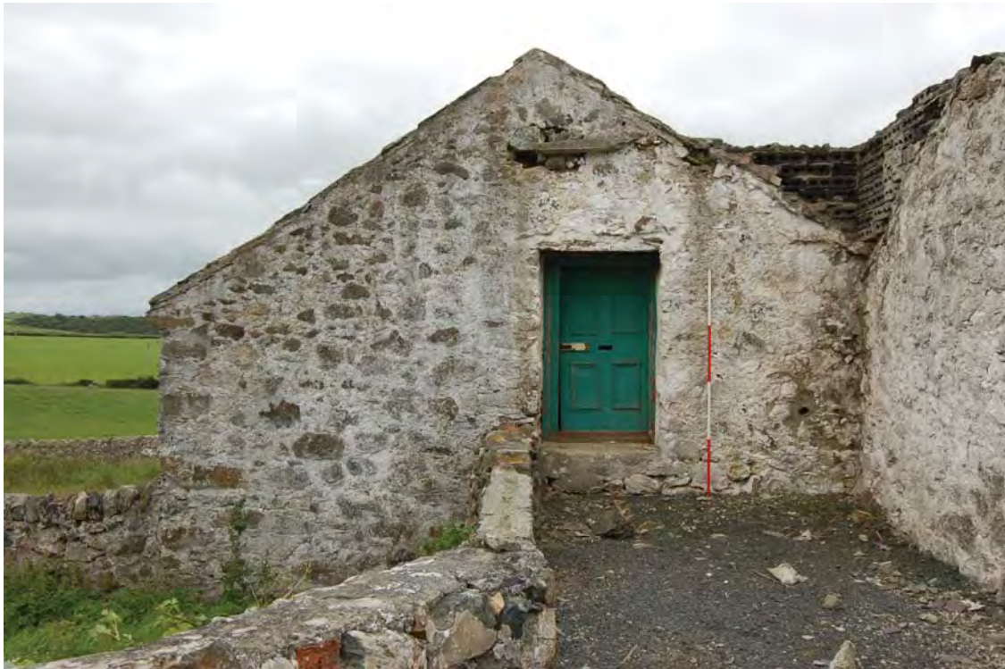
Plate 3. Main Range NW gable end, view SE. 2m scale
