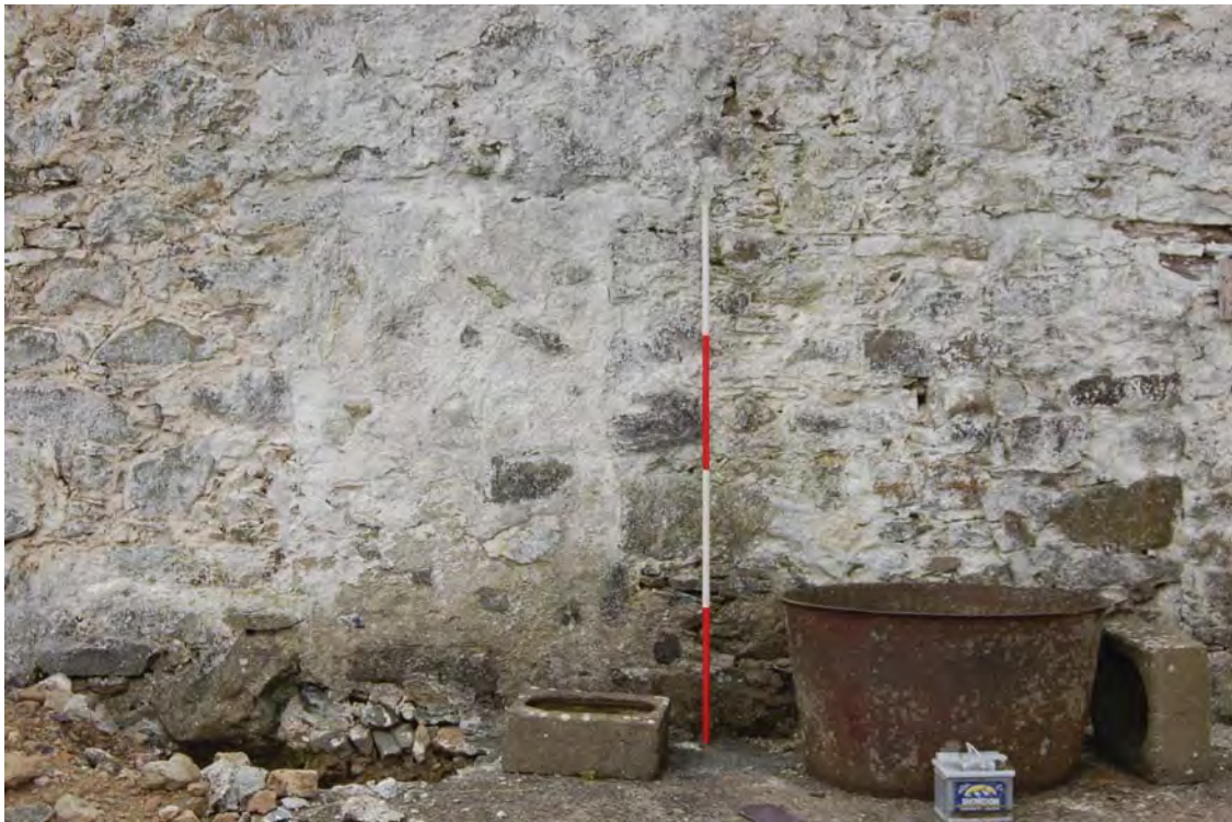
Plate 18. Main Range, central blocked doorway, view SW. 2m scale
