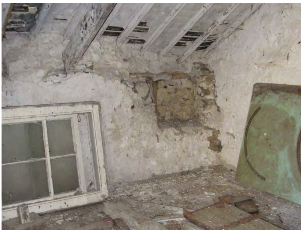
Plate 68. Room 9. Blocked Window. View SE
