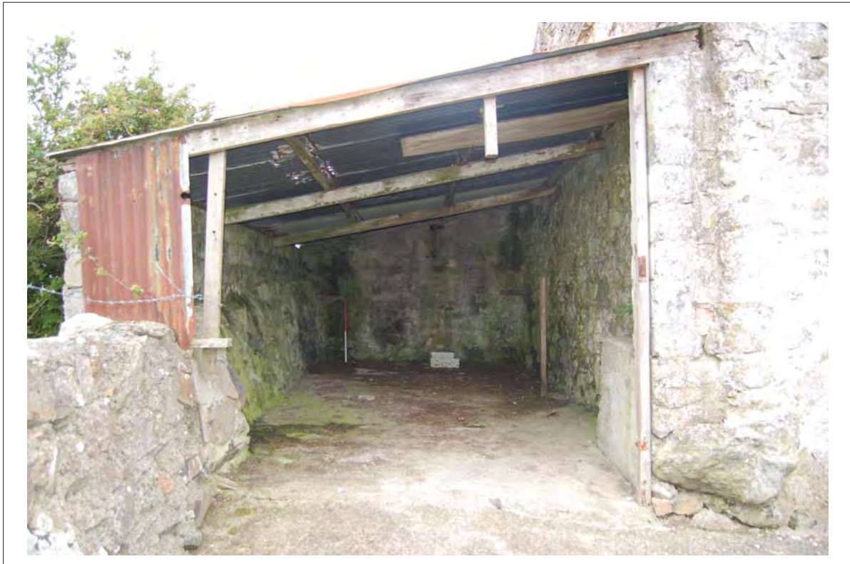
Plate 30. Extension to SE of main range, using enclosure wall, view SW. 1m scale
