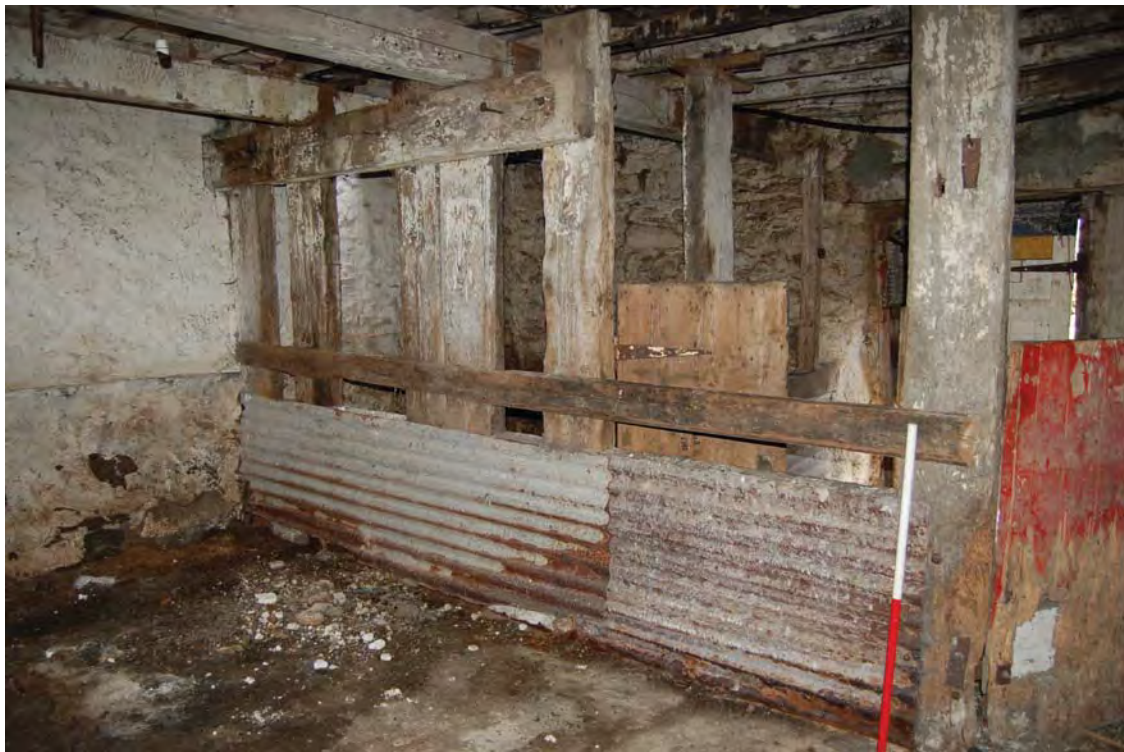
Plate 38. Interior of Room 2 of main range, stalls, view NE. 1m scale
