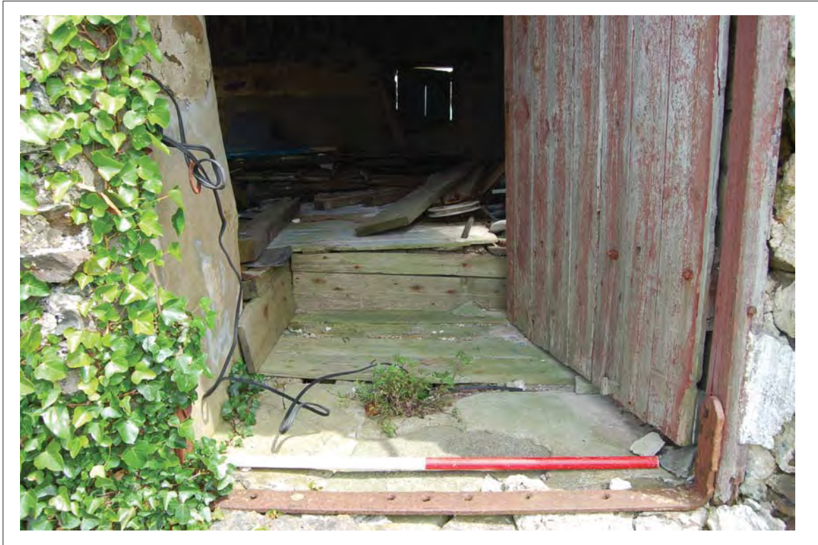
Plate 63. Room 7 recess for door. View NE.
