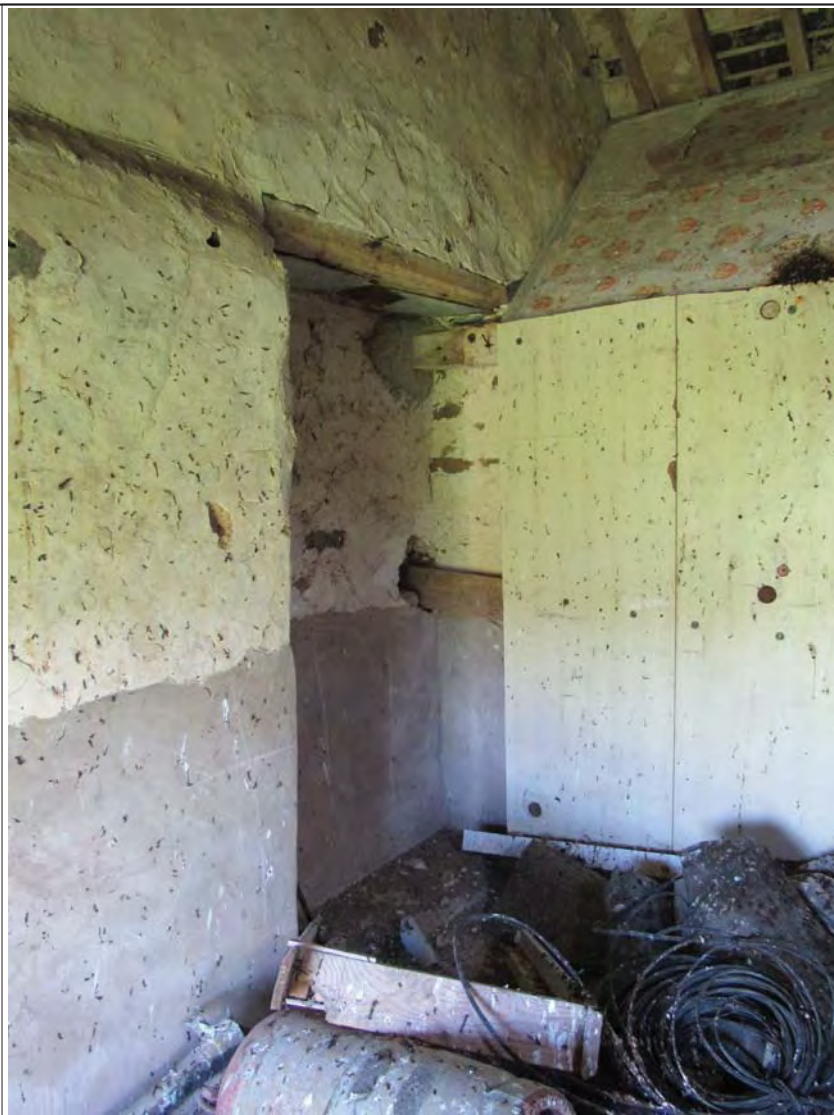
Plate 65. Room 8. Blocked door to Room 9. View N
