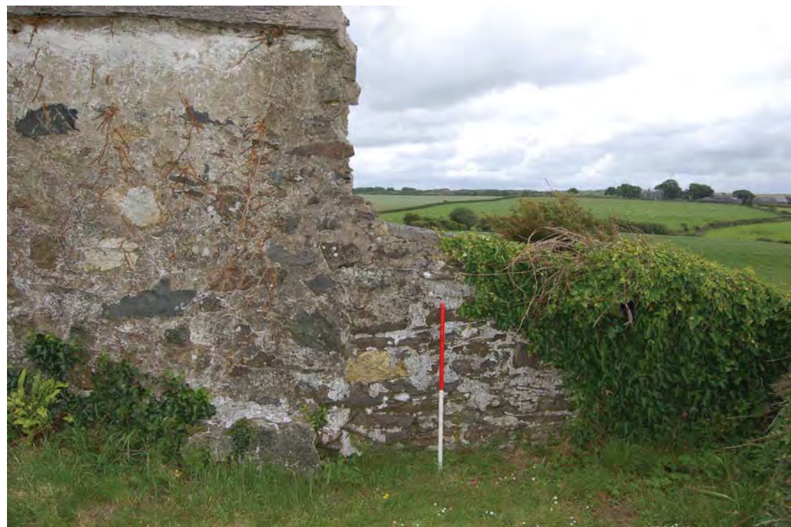
Plate 56. Main Range SE end extension. View NE. 1m scale
