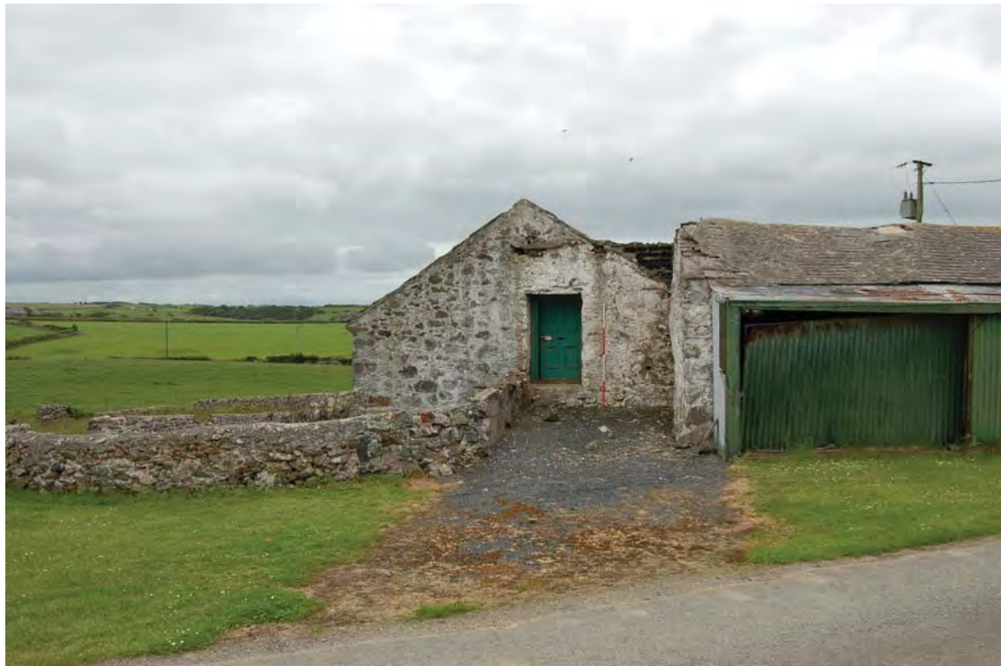
Plate 2. Main Range NW gable end, view SE. 2m scale
