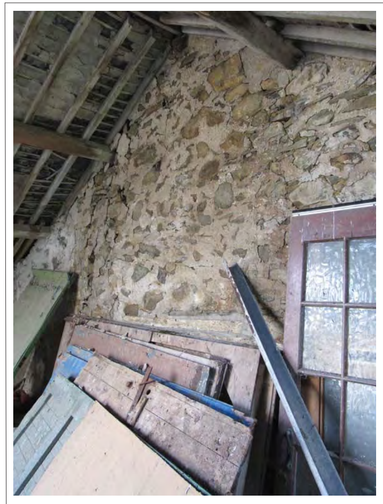
Plate 64. Room 7, with lintel of blocked up window. View SE.
