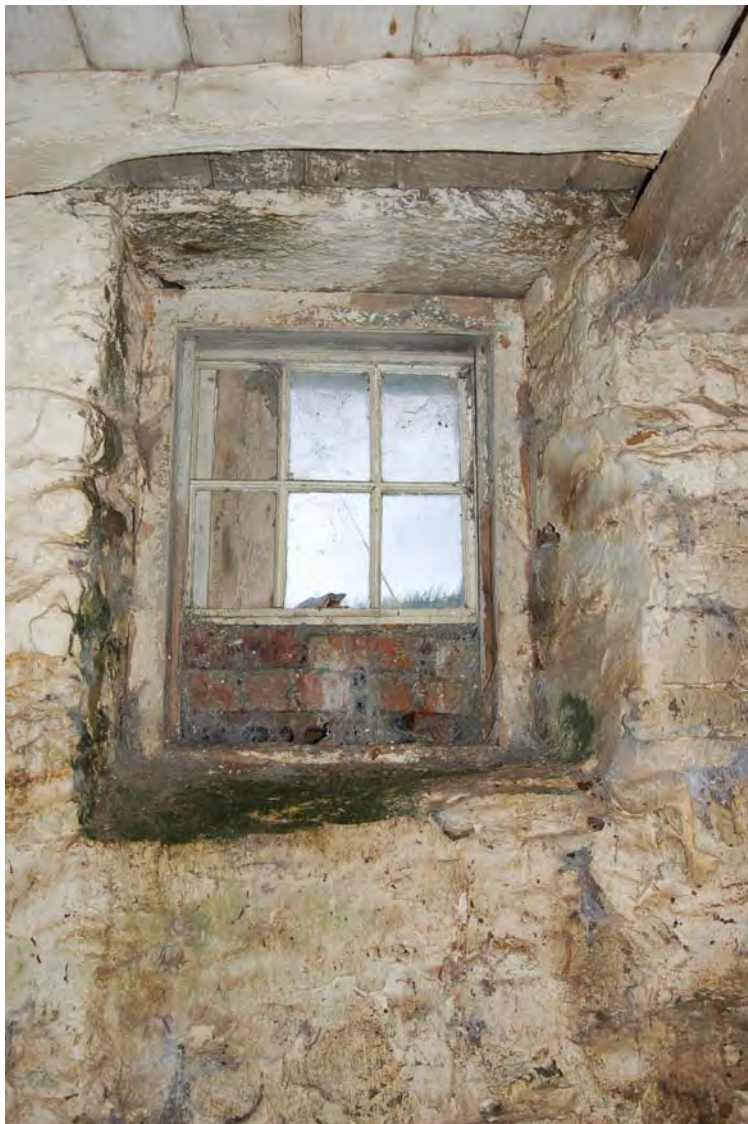
Plate 36. Interior of Room 2 of main range, window, view SW.
