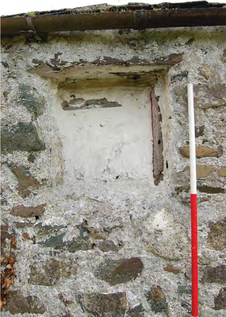
Plate 50. Main Range NW end window. View NE. 1m scale
