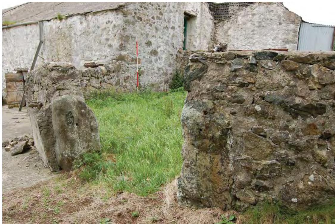
Plate 8. Stone enclosure entrance, view SW. 2m scale
