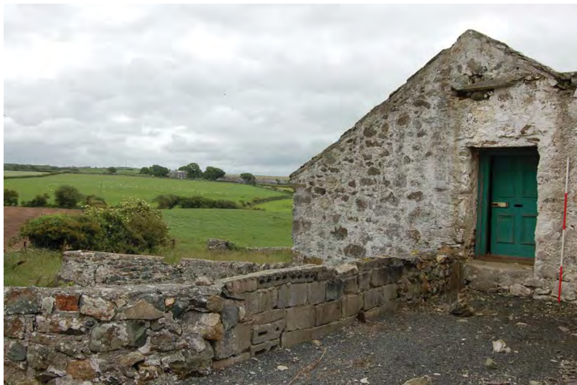
Plate 4. Main Range NW gable end and enclosure, view SE. 2m scale
