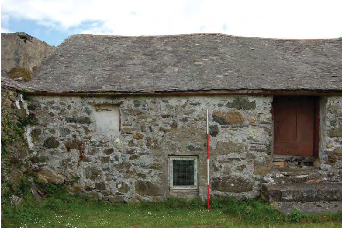
Plate 49. Main Range NW end detail. View NE. 2m scale
