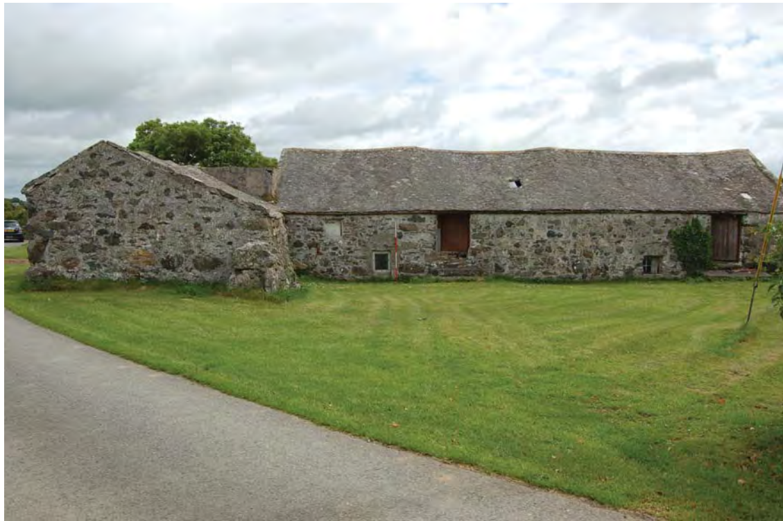
Plate 48. Main Range and West Range gable end. View NE. 2m scale
