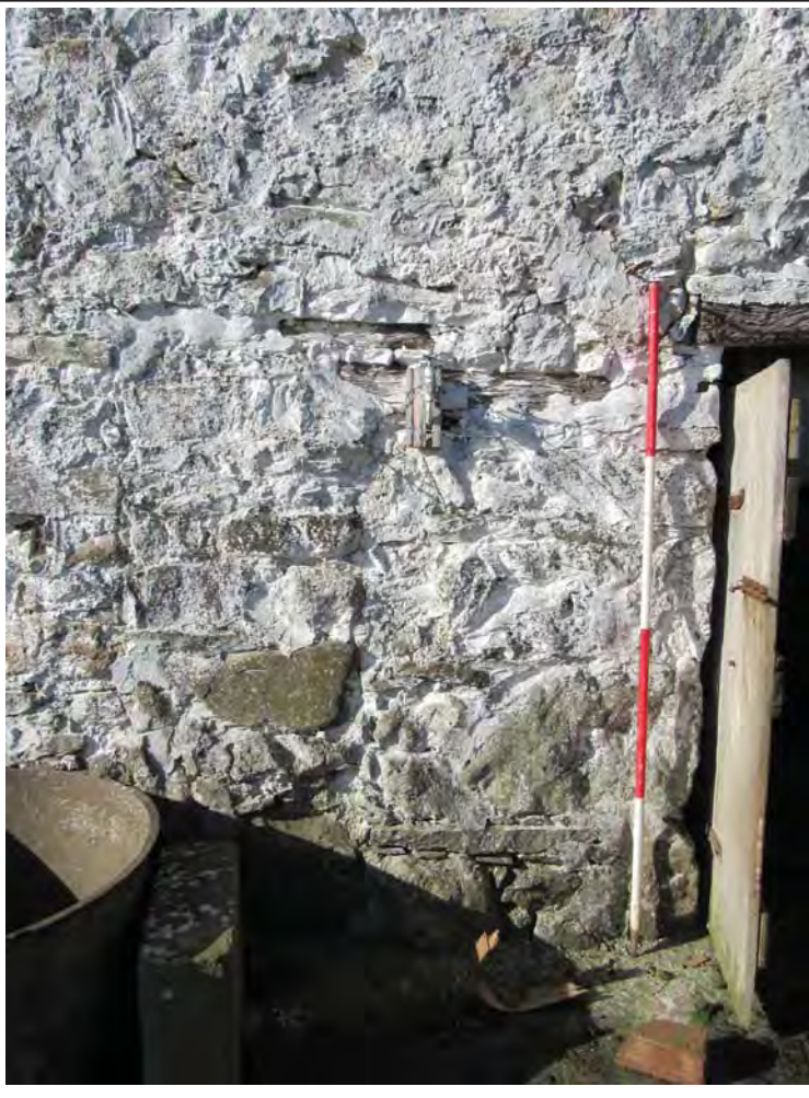
Plate 17. Main Range, central blocked windows, view SW. 2m scale
