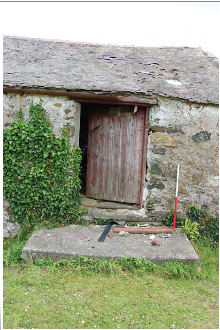
Plate 55. Main Range SE end door. View NE. 1m scale
