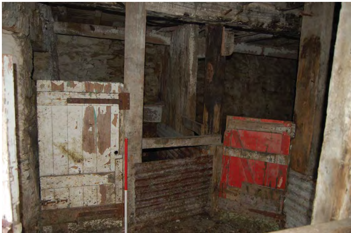
Plate 32. Interior of Room 2 of main range, view SE. 1m scale
