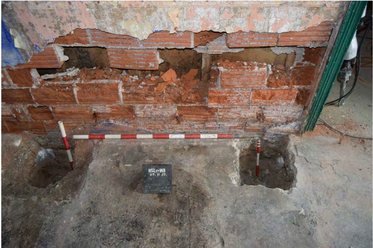
Plate 13: Phase 1 interior, test pits 7 and 8. View east, 1m, 0.5m & 0.3m scales.
