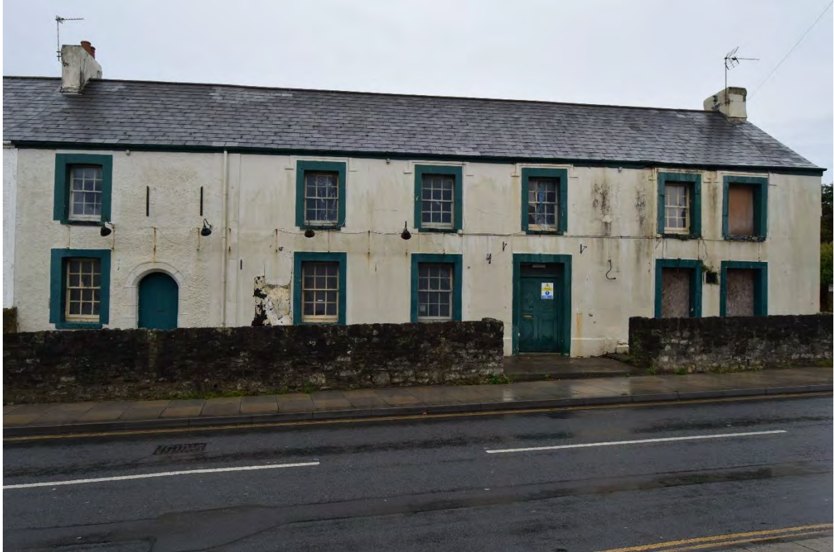
Plate 1: The former Oystercatcher Public House, as viewed from the High Street to the south.
