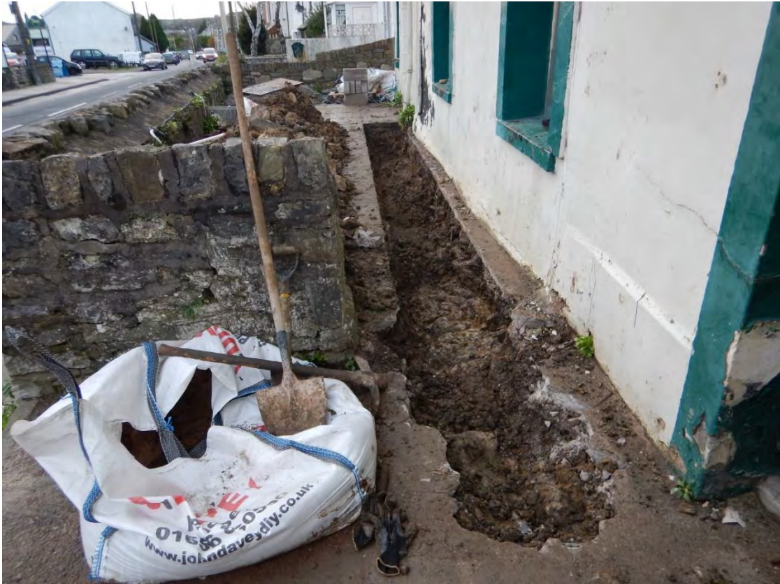
Plate 15: Phase 2 exterior (front), showing the excavated services trench, view west.
