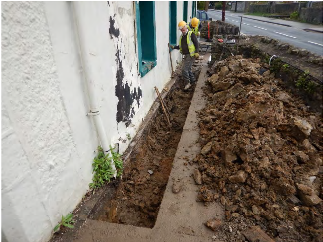
Plate 16: As above, under excavation, view east.
