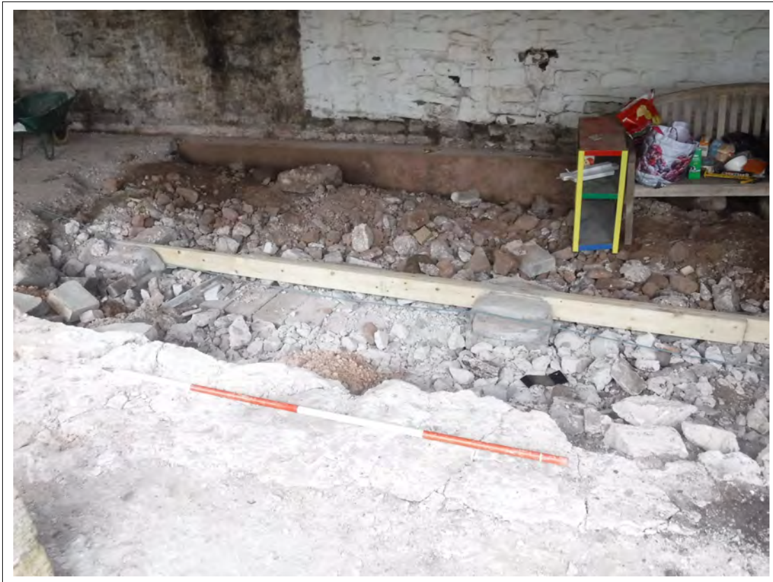
Plate 35. Remains of swimming pool, looking south-west. Scale 2m
