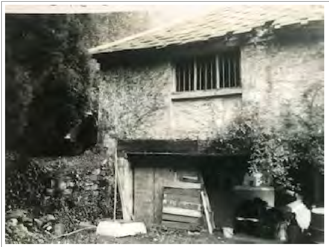
Plate 4. Photographs received from the current owner prior to and during renovations in the 1980s
