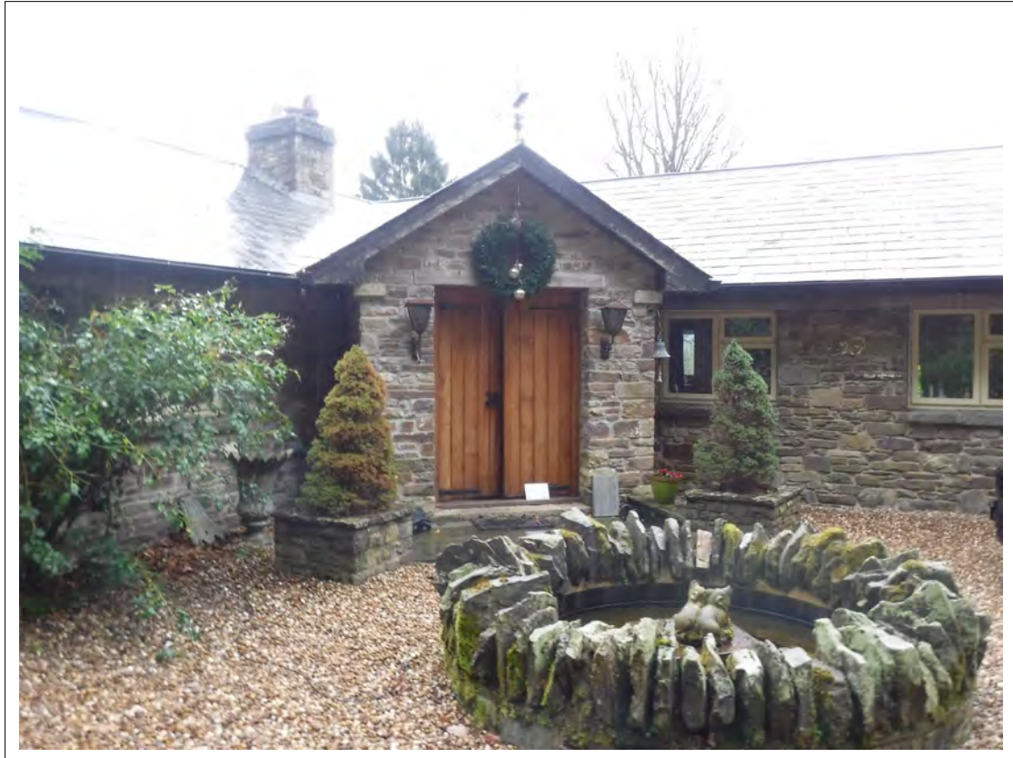
Plate 25. Entrance porch, looking north-east
