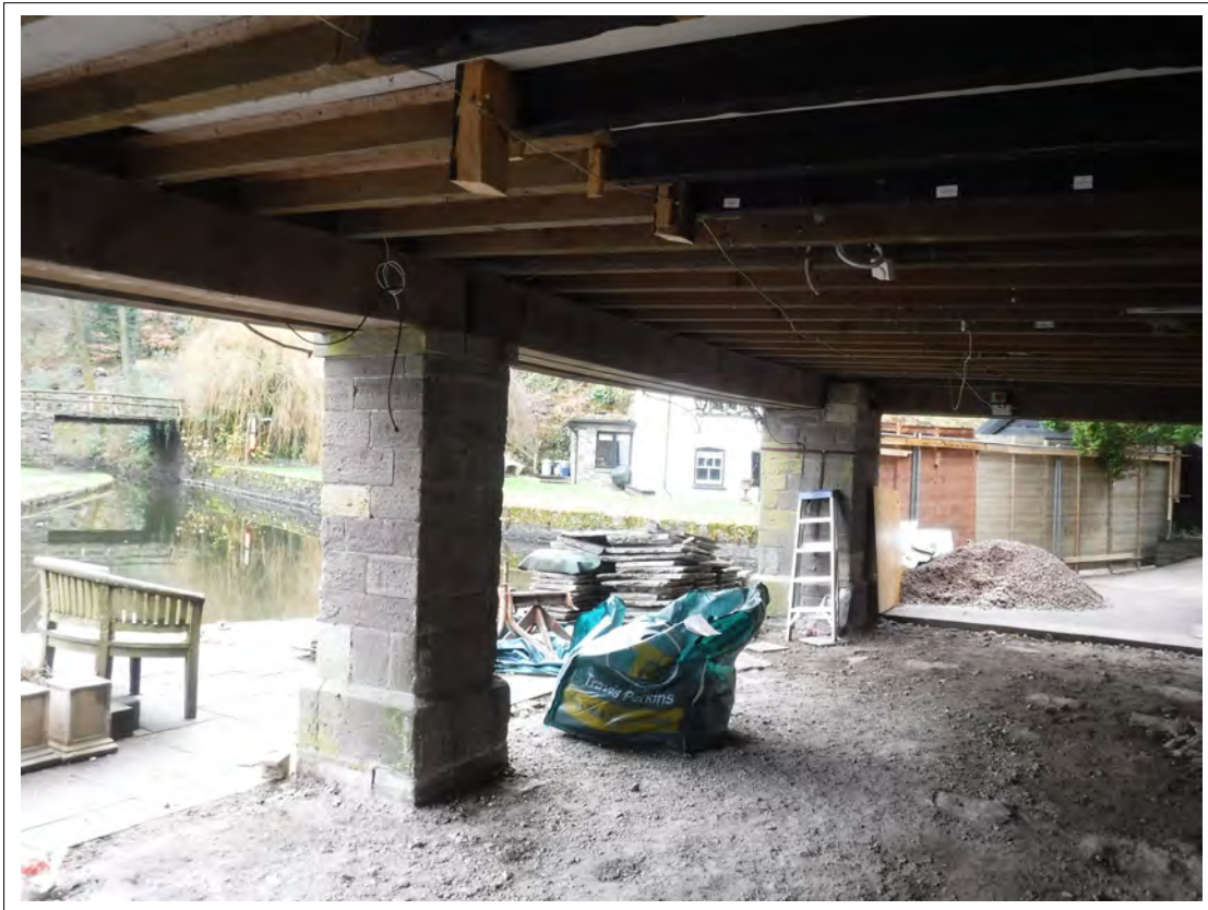
Plate 39. Ceiling of Open Sided Room, looking south-east
