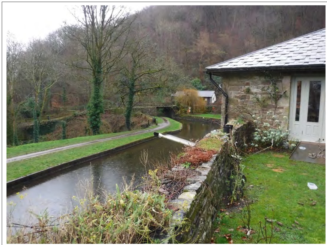
Plate 18. Retaining wall to the north of The Boathouse, looking south-east from The Boathouse garden
