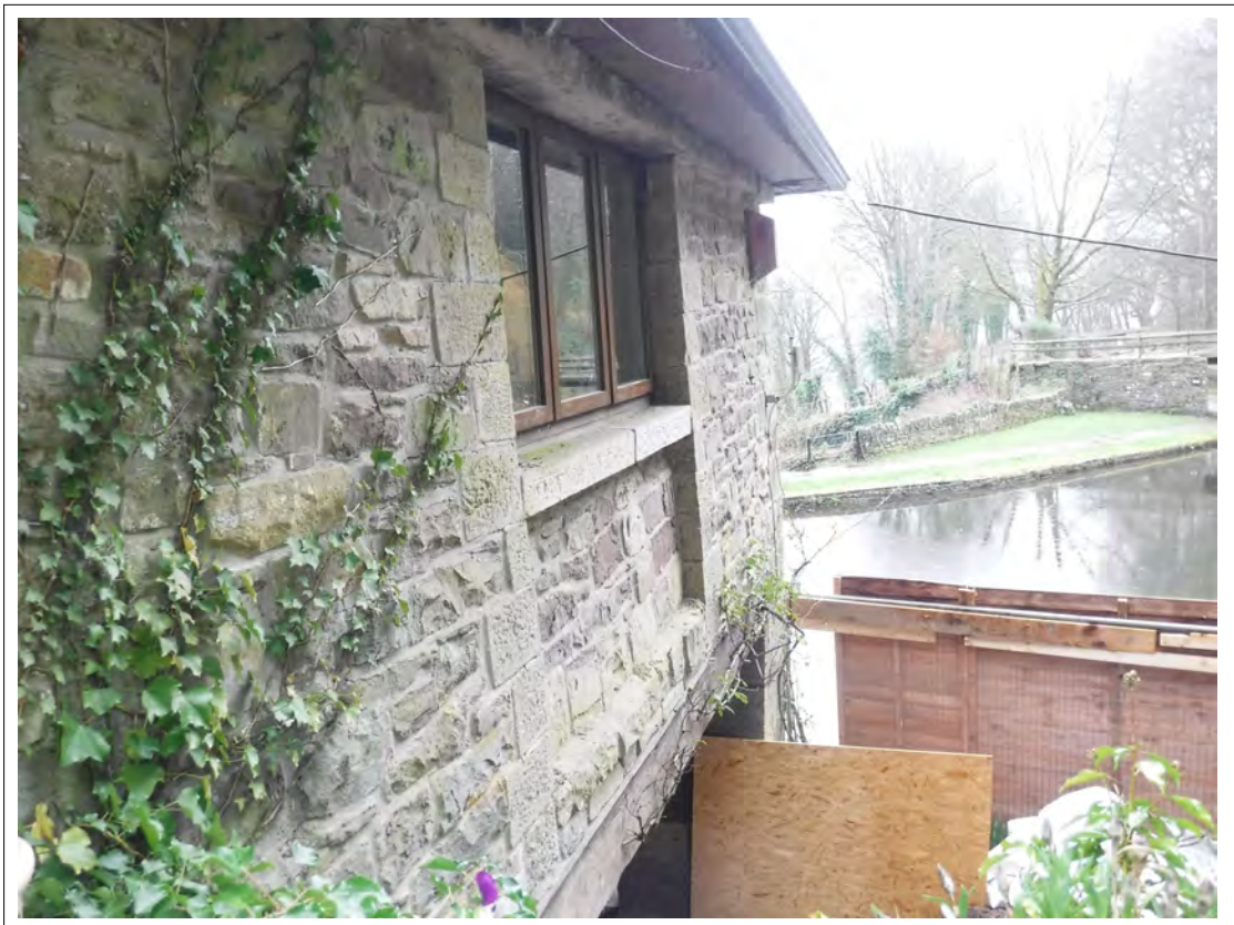
Plate 20. Detail of the window of the south-facing elevation, looking north-east
