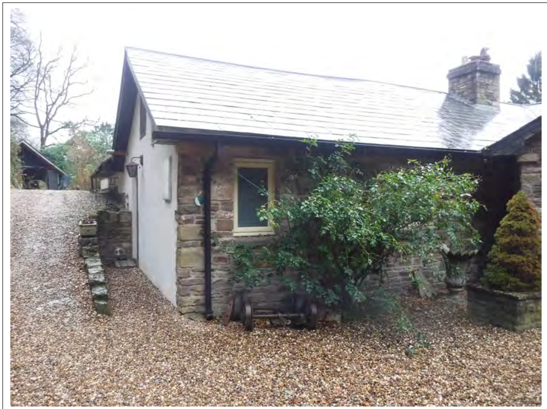
Plate 26. The gable end extension, looking north
