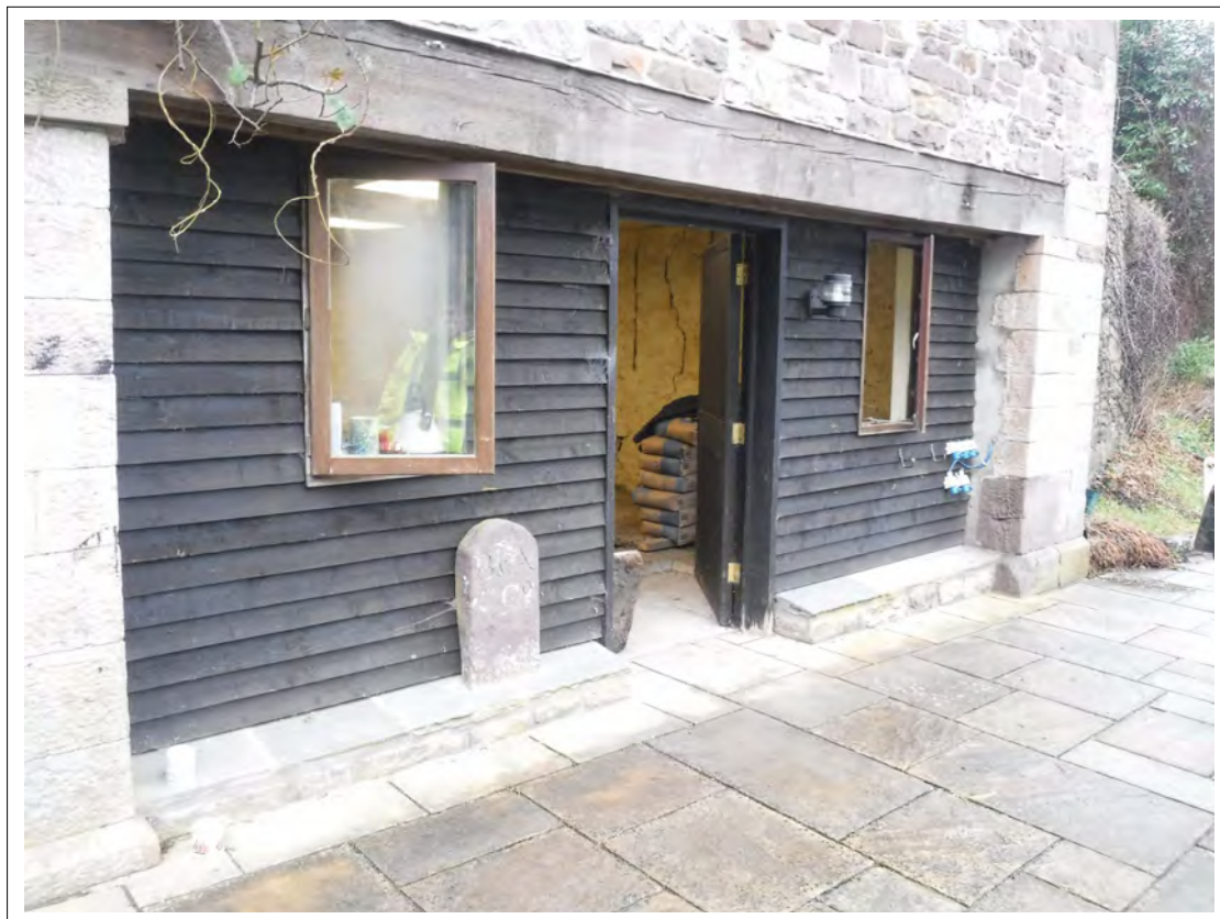
Plate 16. Exterior of Storage Room, east-facing elevation, looking north-west
