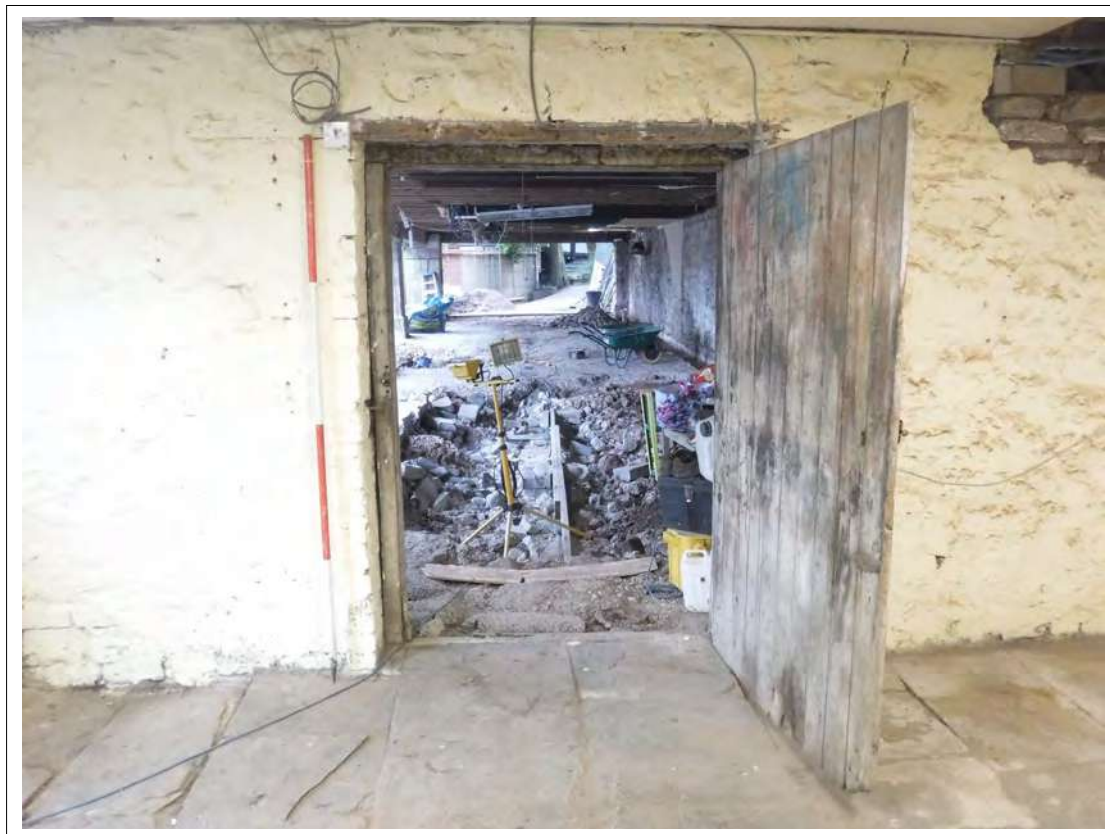
Plate 32. Doorway in southern wall of Storage Room, looking south. Scale 2m
