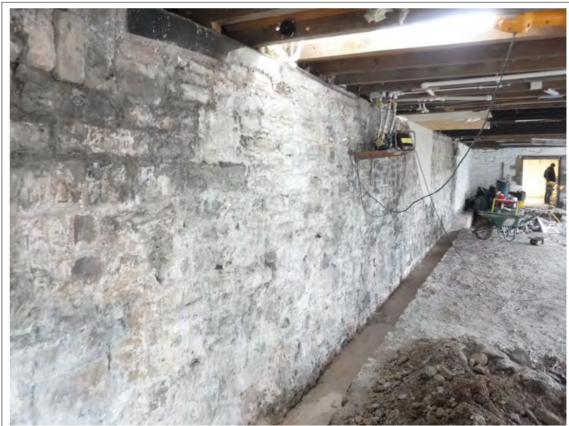
Plate 36. Western wall of Open Sided Room, looking north-west
