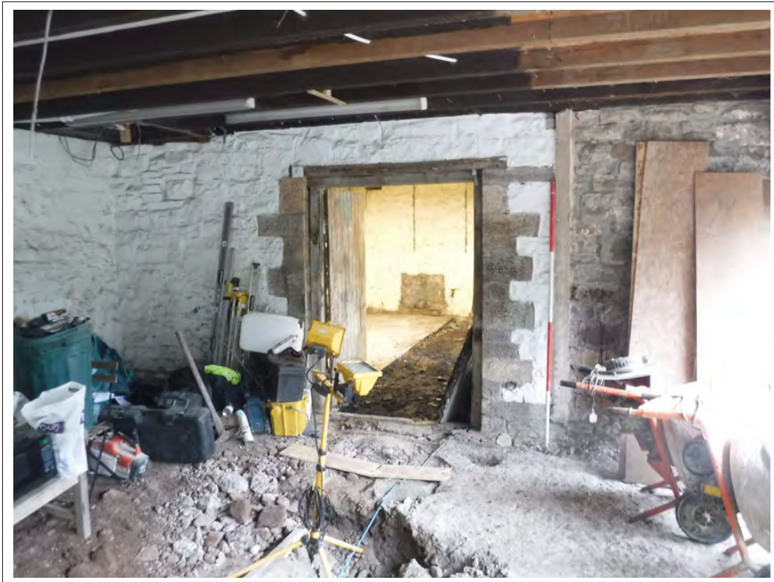
Plate 38. Northern wall and doorway, looking north. Scale 2m
