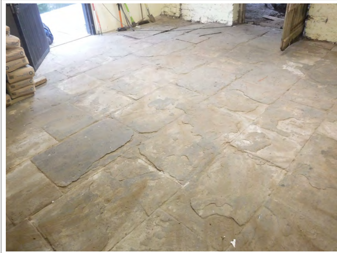
Plate 29. Flagstone floor of Storage Room, looking south-east
