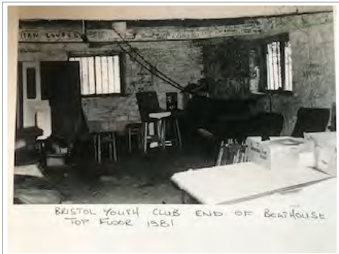
Plate 2. Photographs received from the current owner prior to and during renovations in the 1980s
