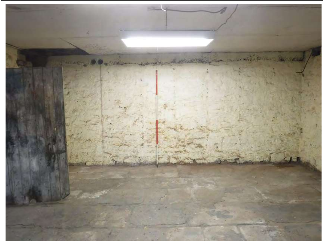
Plate 31. Western wall of Storage Room, looking west. Scale 2m
