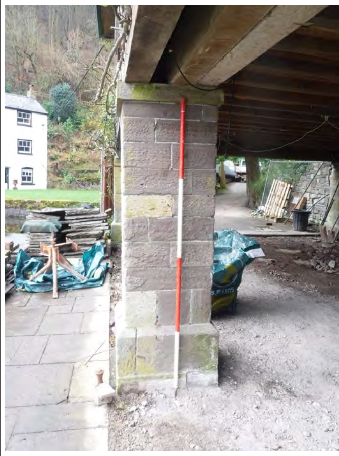
Plate 13. Pillar to south of the east elevation, looking south. Scale 2m
