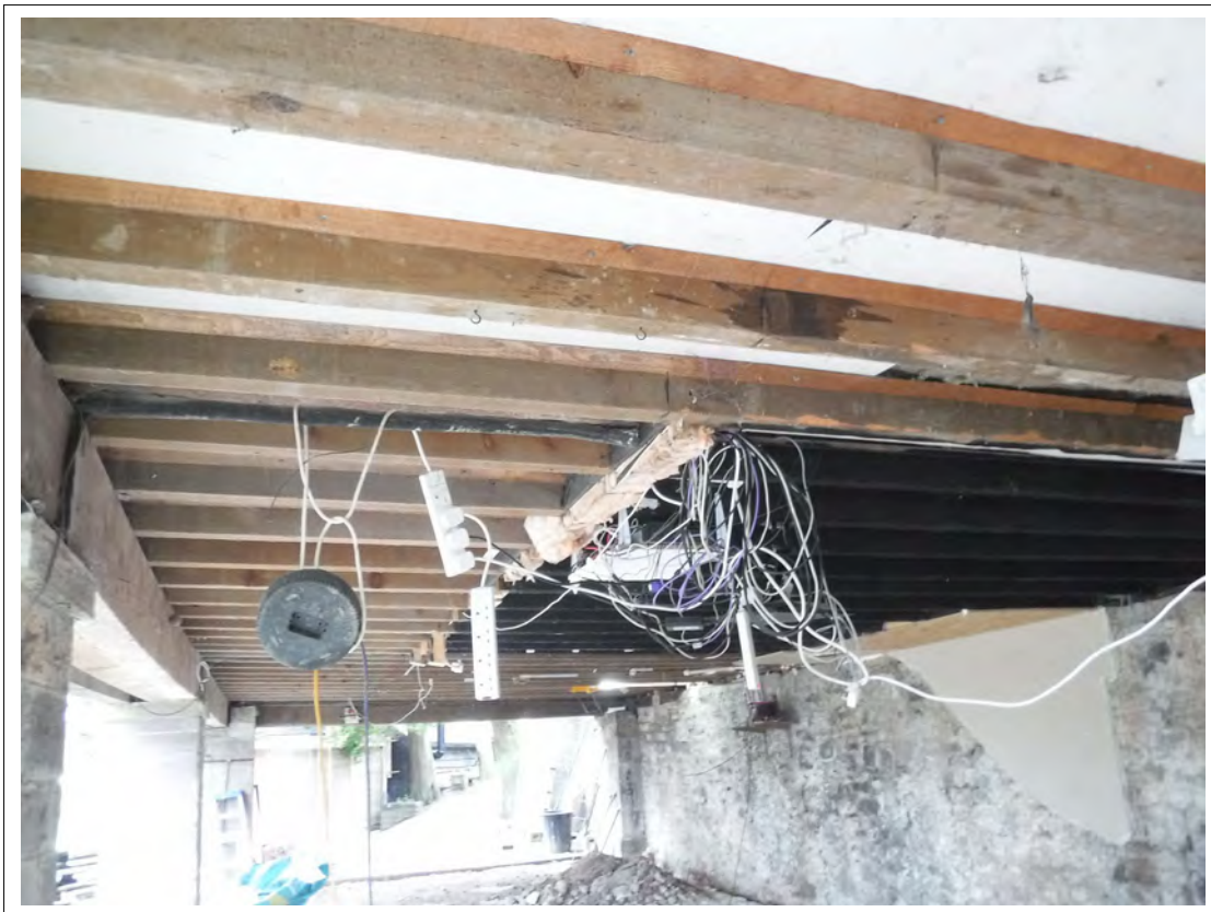
Plate 40. Ceiling of Open Sided Room, looking south
