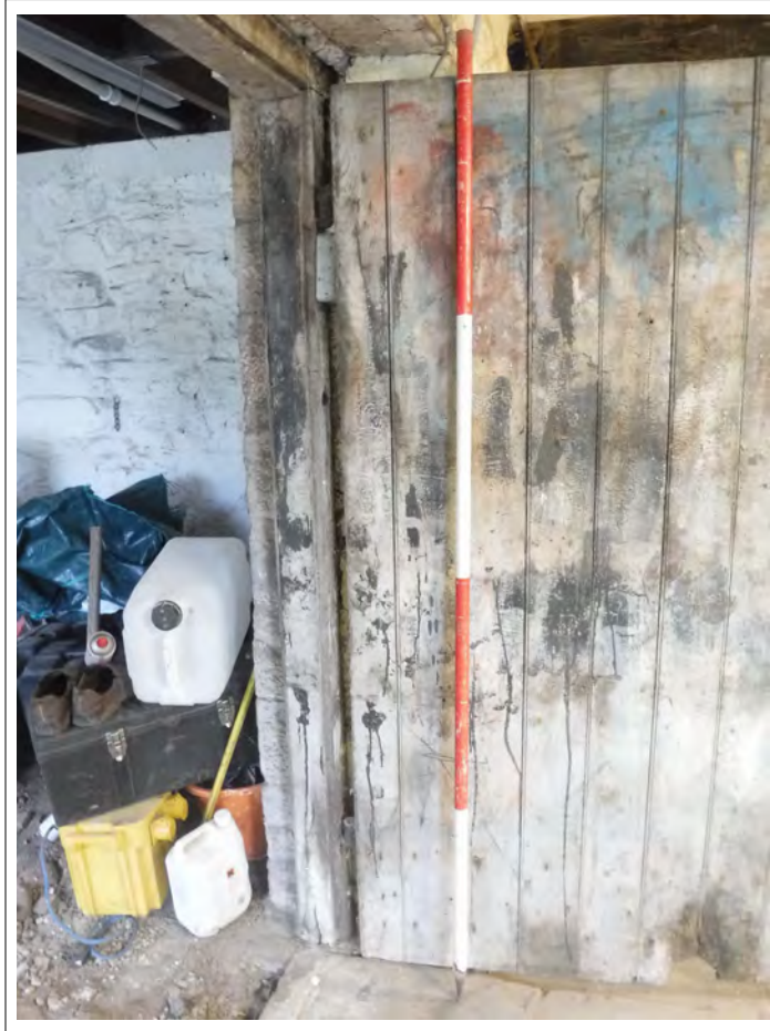
Plate 33. Detail of door in southern wall of Storage Room. Scale 2m
