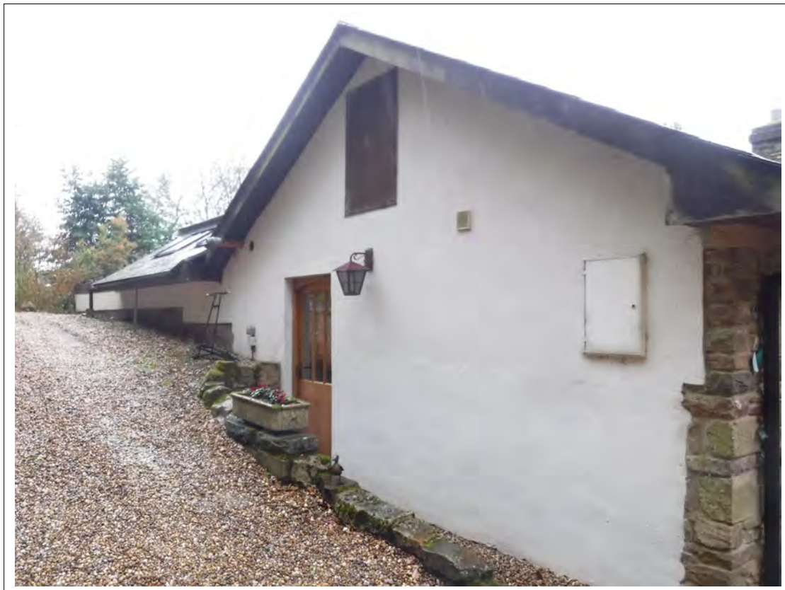
Plate 22. West-facing elevation, central extension, looking north-east
