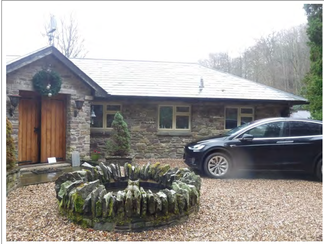
Plate 21. West-facing elevation, southern section, looking east
