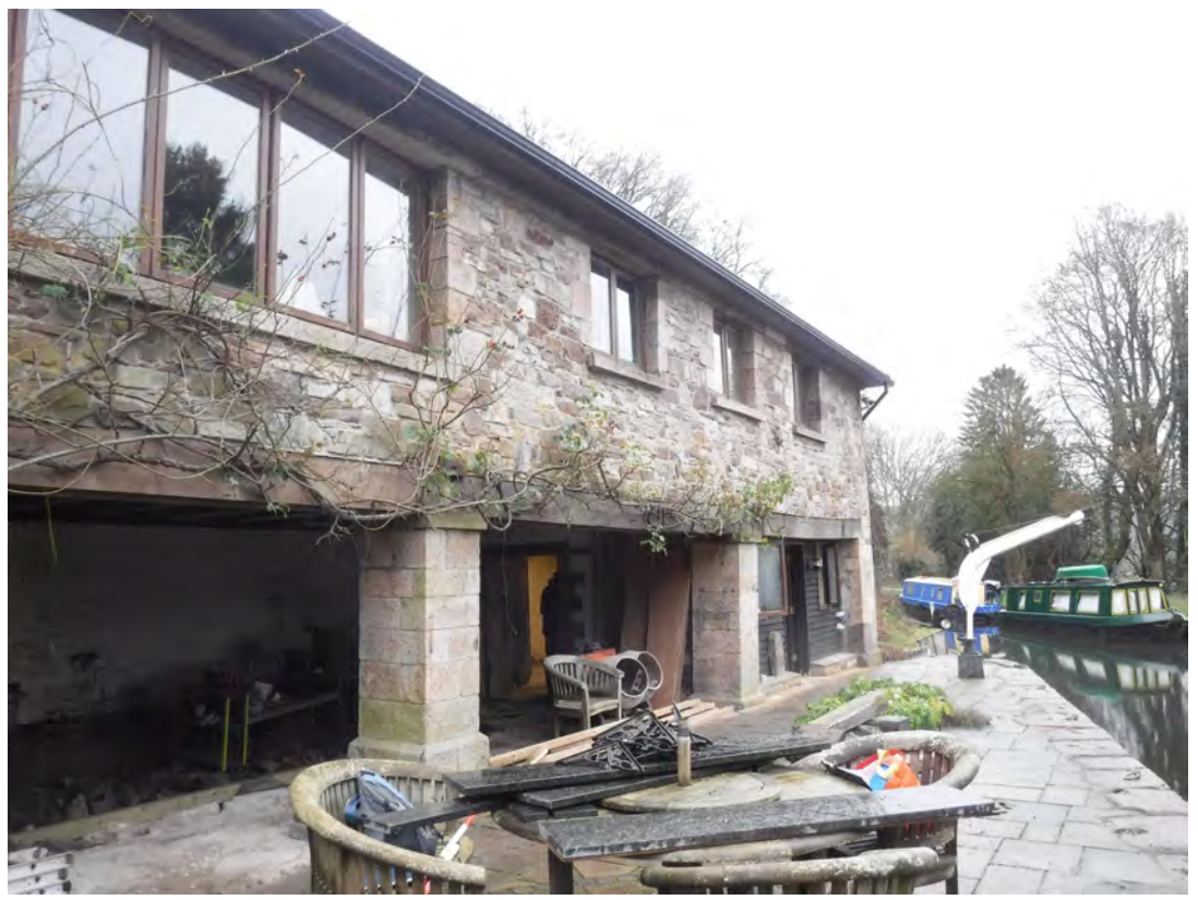
Plate 11. East-facing elevation, looking north-west
