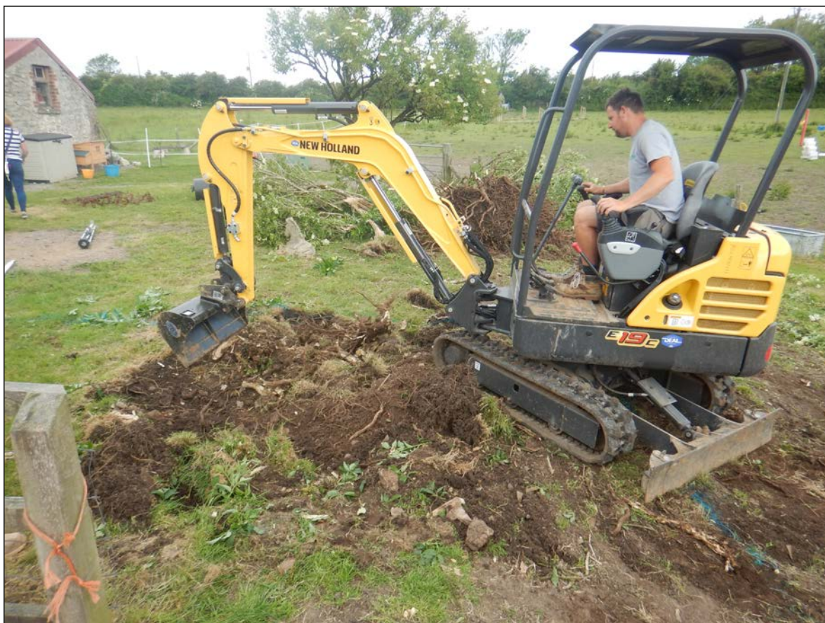
Plate 1. Removal of a small tree before strip looking W
