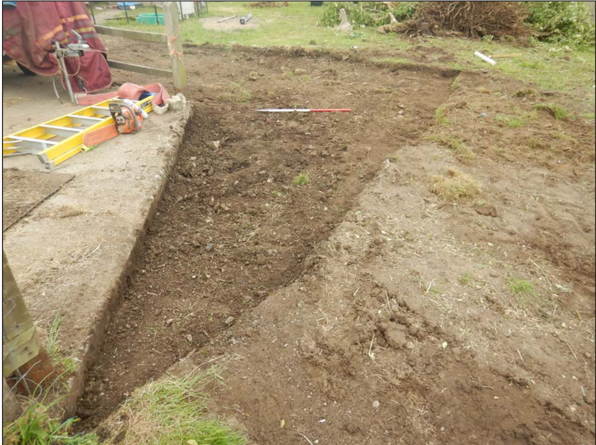
Plate 7. Shot of the NE end of the excavation, looking W
