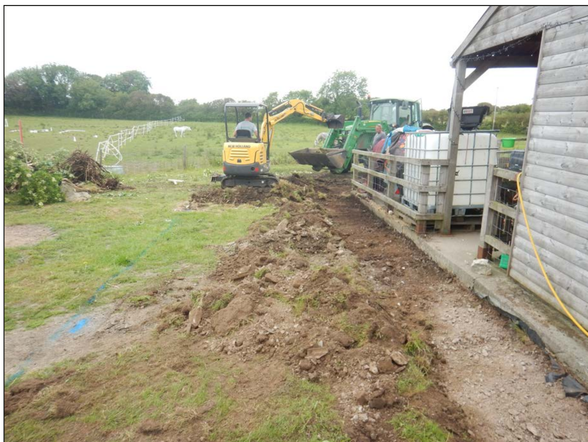
Plate 2. Working shot of strip looking NE
