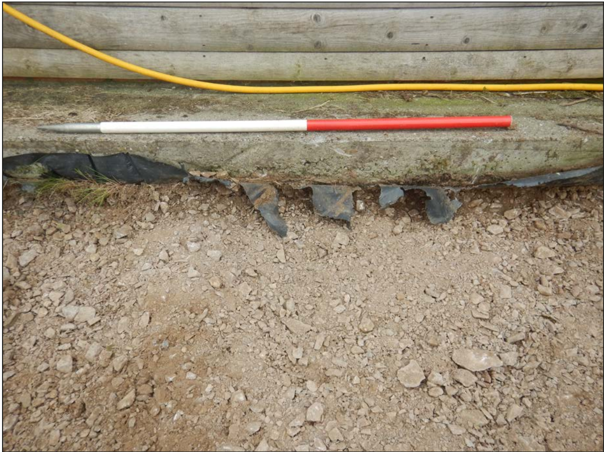
Plate 3. Shot of the NW facing section of hardstanding, looking SE
