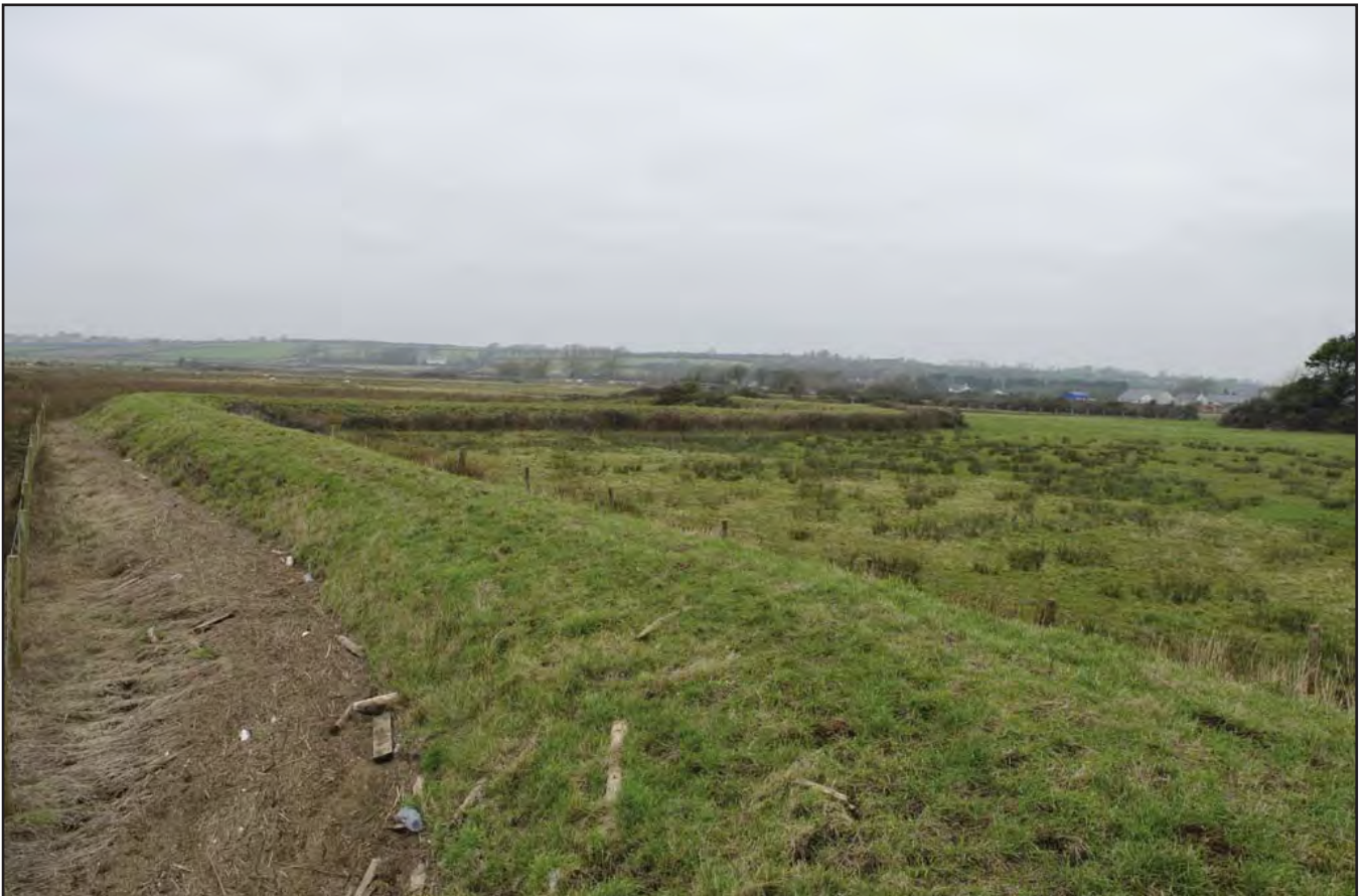
Plate 12: Flood embankment looking toward A4080 (archive reference: G2706_036).
