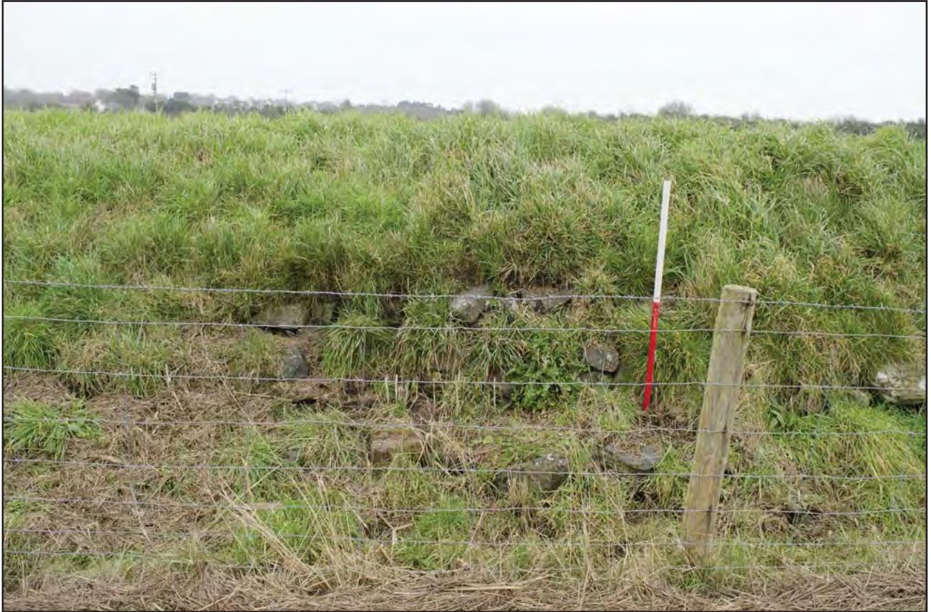
Plate 15: Example of stone façade of flood embankment beside tidal outflow ; scale: 1x1m (archive reference: G2706_038).
