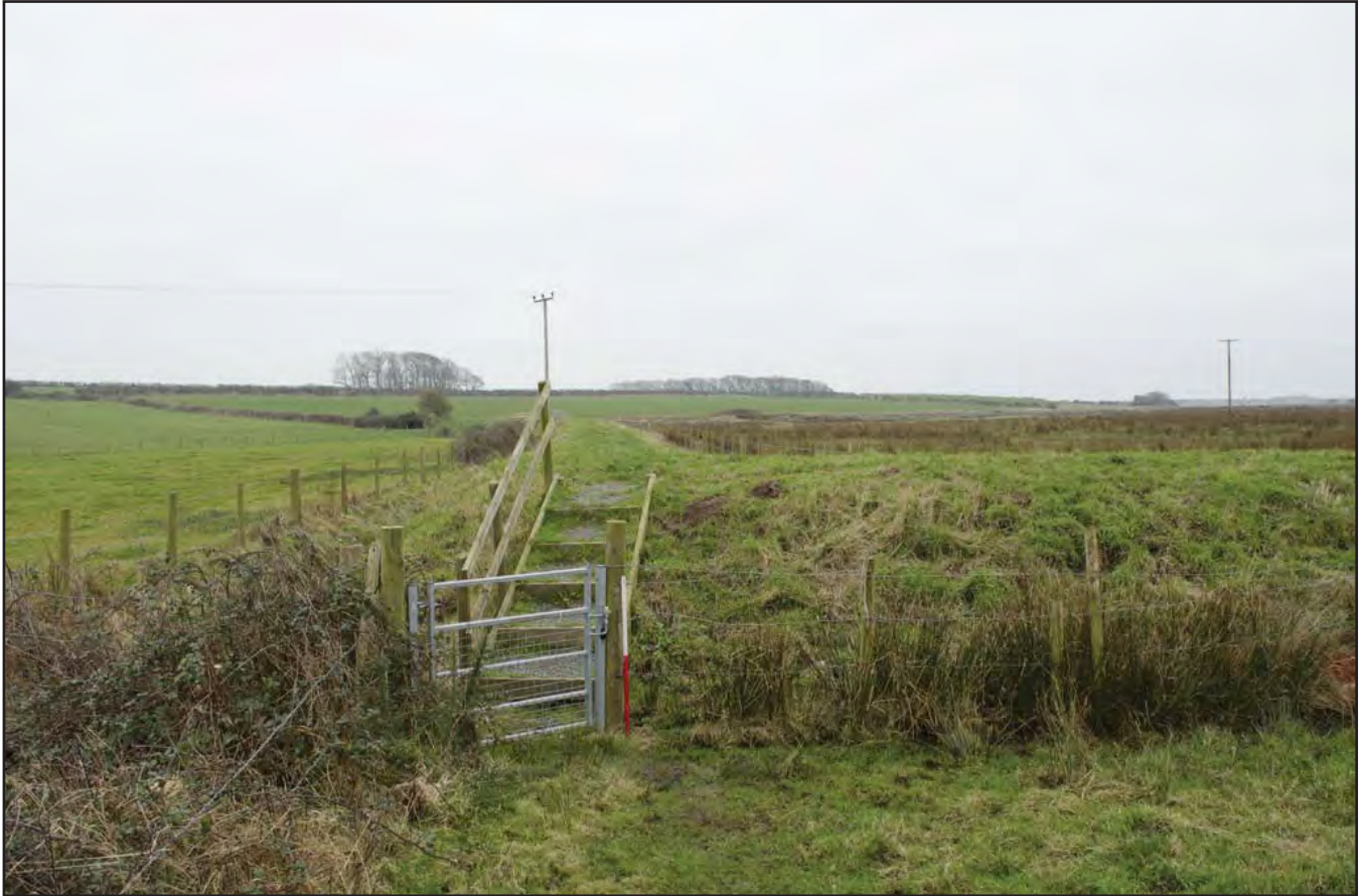
Plate 13: Flood embankment along public right of way; scale: 1x1m (archive reference: G2706_035).
