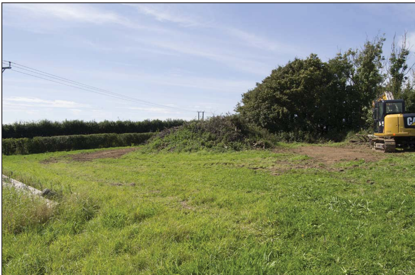
Plate 16: Field condition post-backfilling of trenches; scale not used; view from NE (archive reference: G2799_37).
