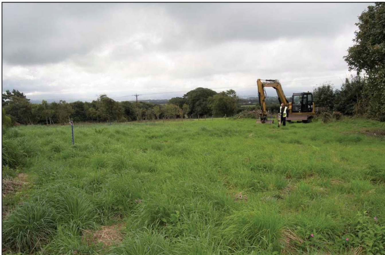
Plate 1: Pre-condition survey prior to trenching; scale not used; view from N (archive reference: G2799_02).
