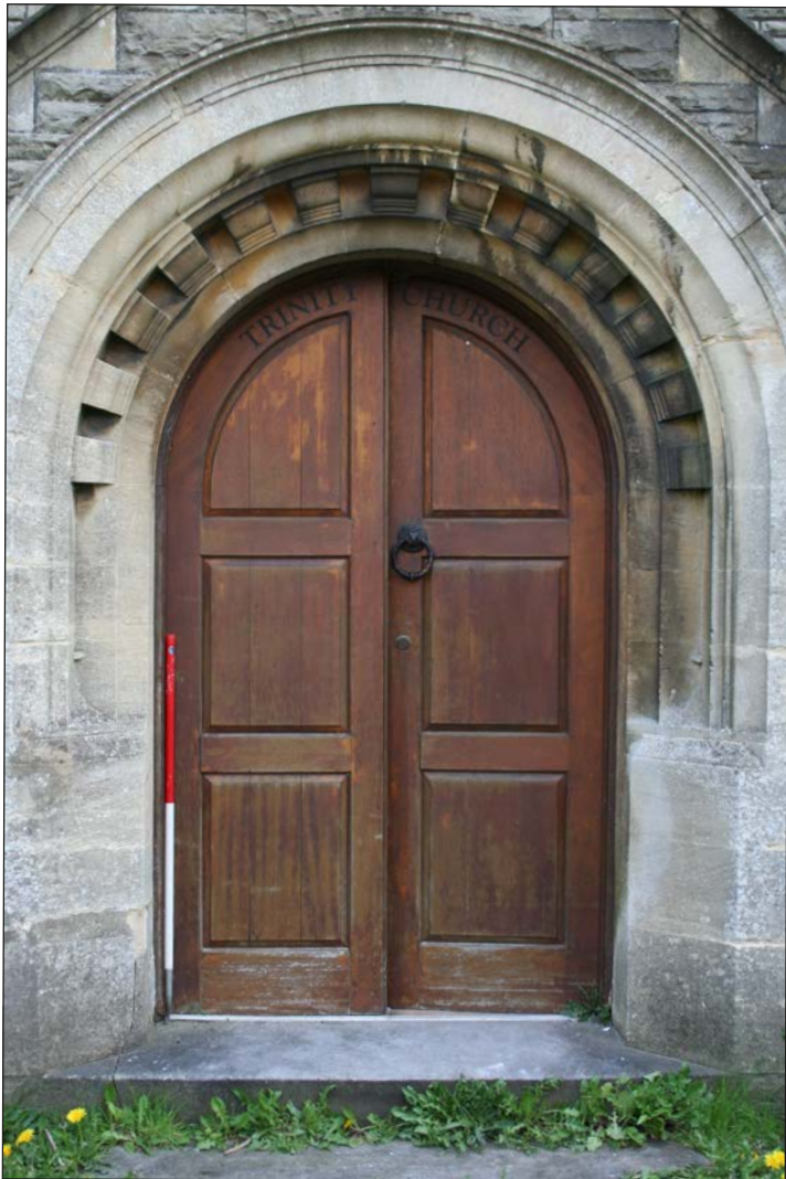
Plate 37. Main entrance and NW wall of vestibule, looking NW
