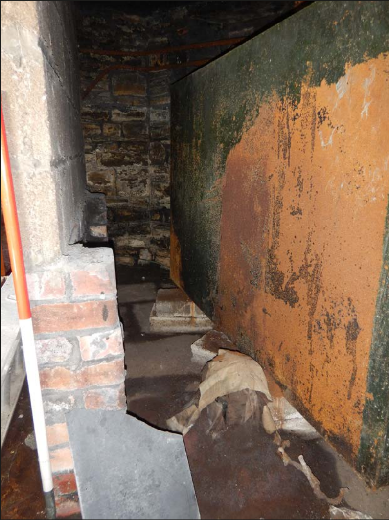
Plate 90. Chapel basement, looking NW
