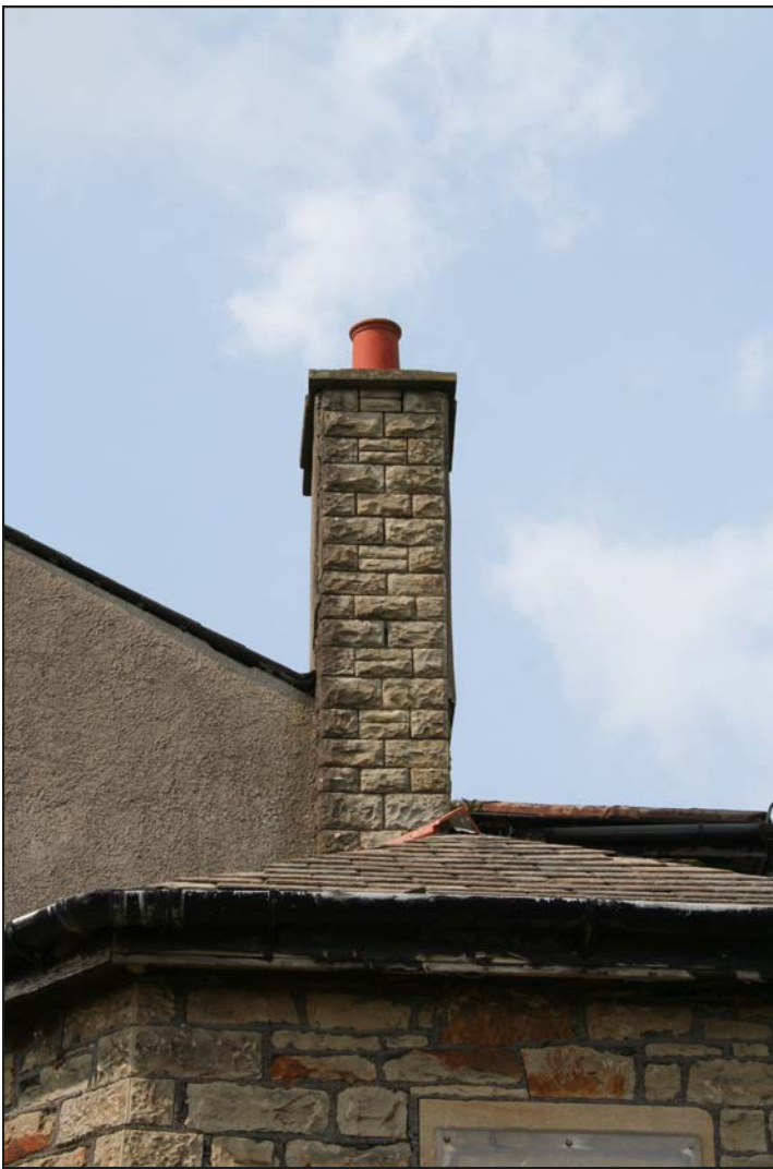
Plate 22. Chimney stack to rear elevation, looking NW
