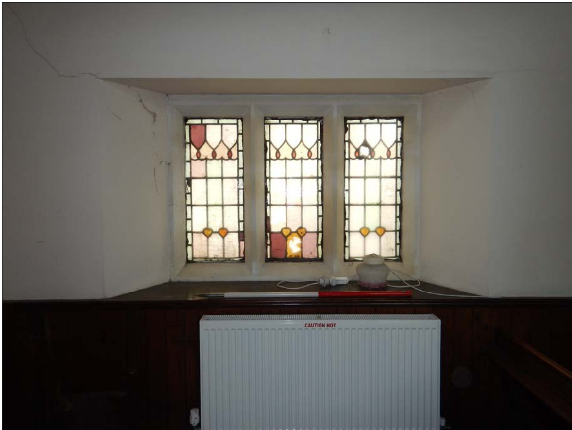
Plate 45. Detail of window to NE wall of nave, looking NE
