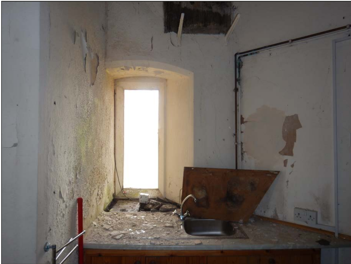
Plate 81. Window to NE wall of corridor/kitchen, looking NE
