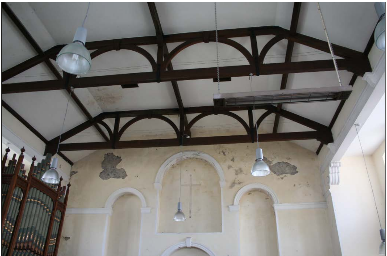
Plate 71. Nave ceiling, looking SE
