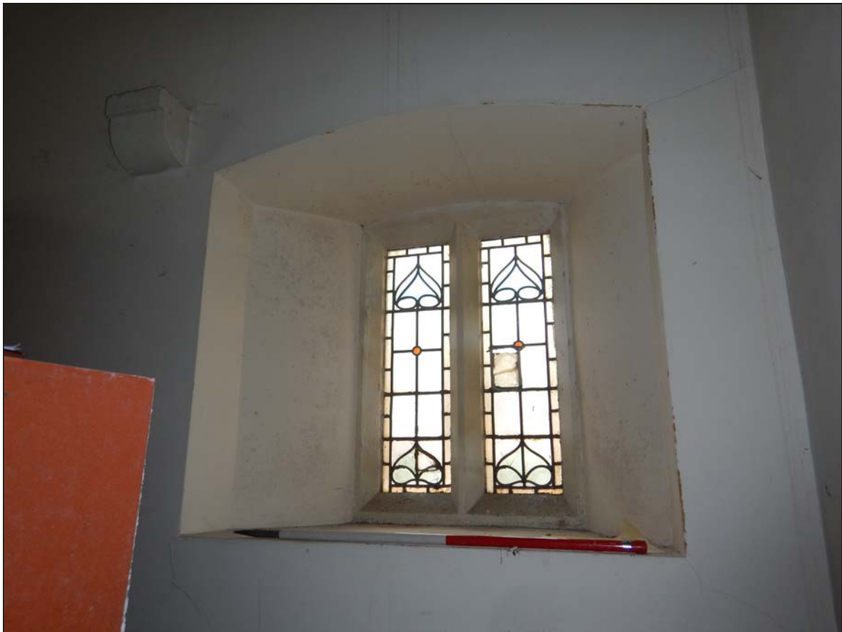
Plate 41. Detail of ground floor window to NW wall, looking NW
