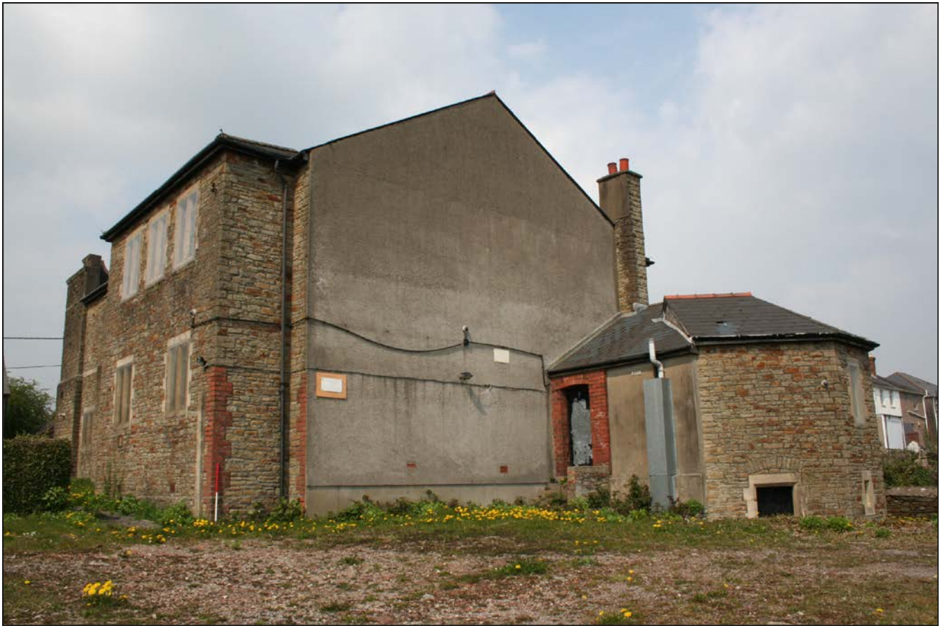
Plate 20. Rear elevation of Trinity Chapel, looking N
