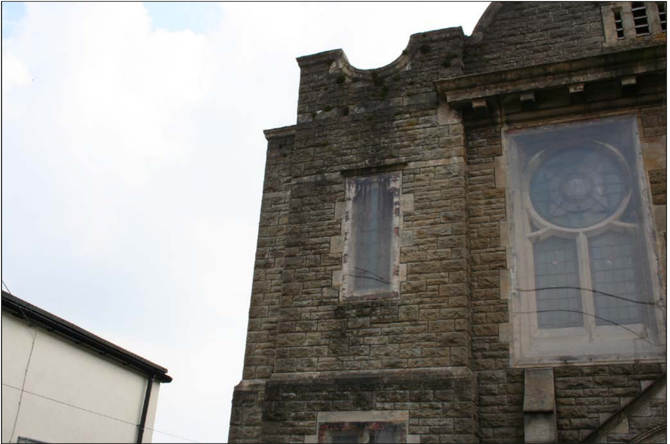
Plate 10. Upper window to first bay of front elevation, looking SE
