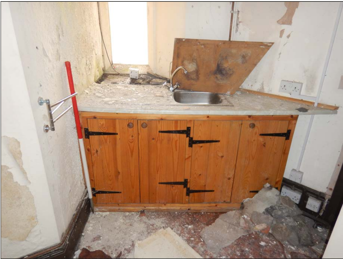
Plate 82. Kitchen fixtures in corridor/kitchen area, looking NE
