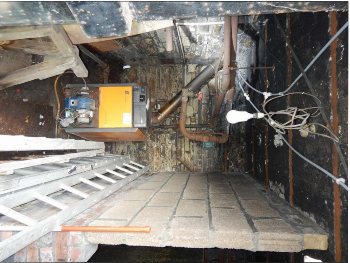
Plate 89. Chapel basement, looking NW
