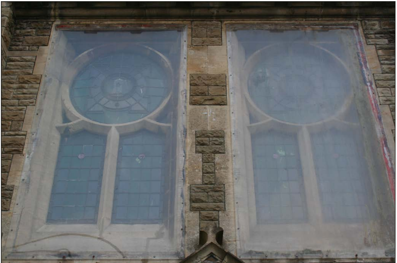
Plate 9. Upper central windows to front elevation, looking SE
