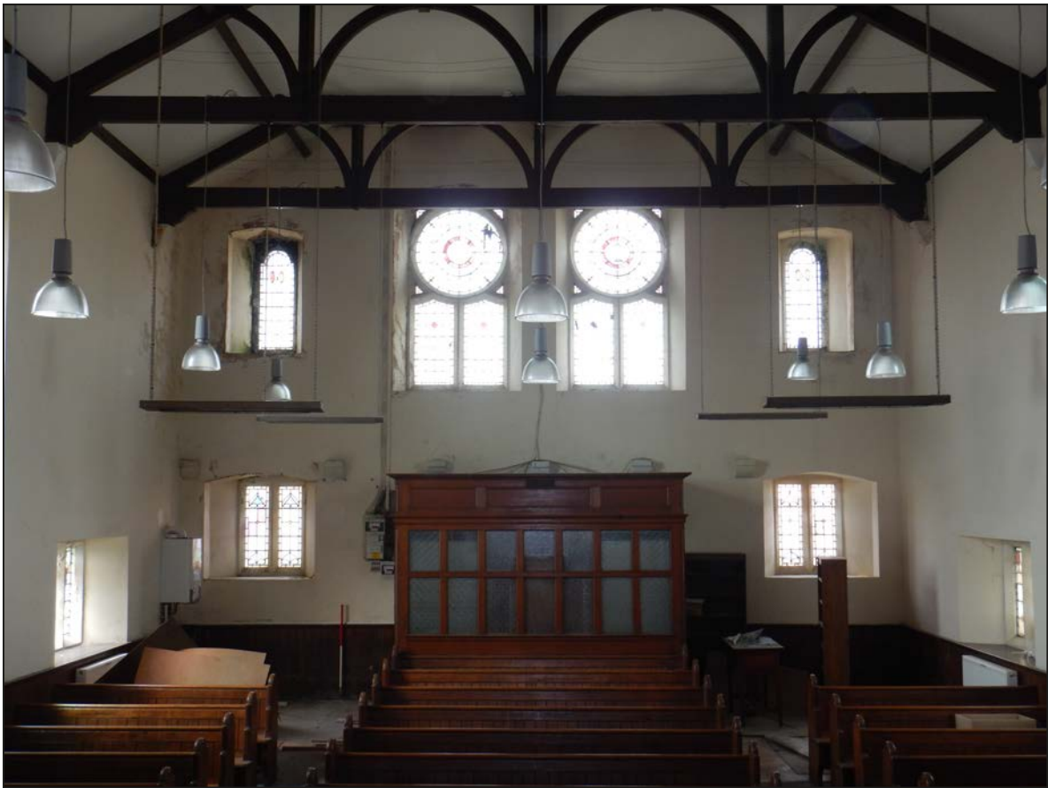
Plate 40. NW gable end of nave, looking NW
