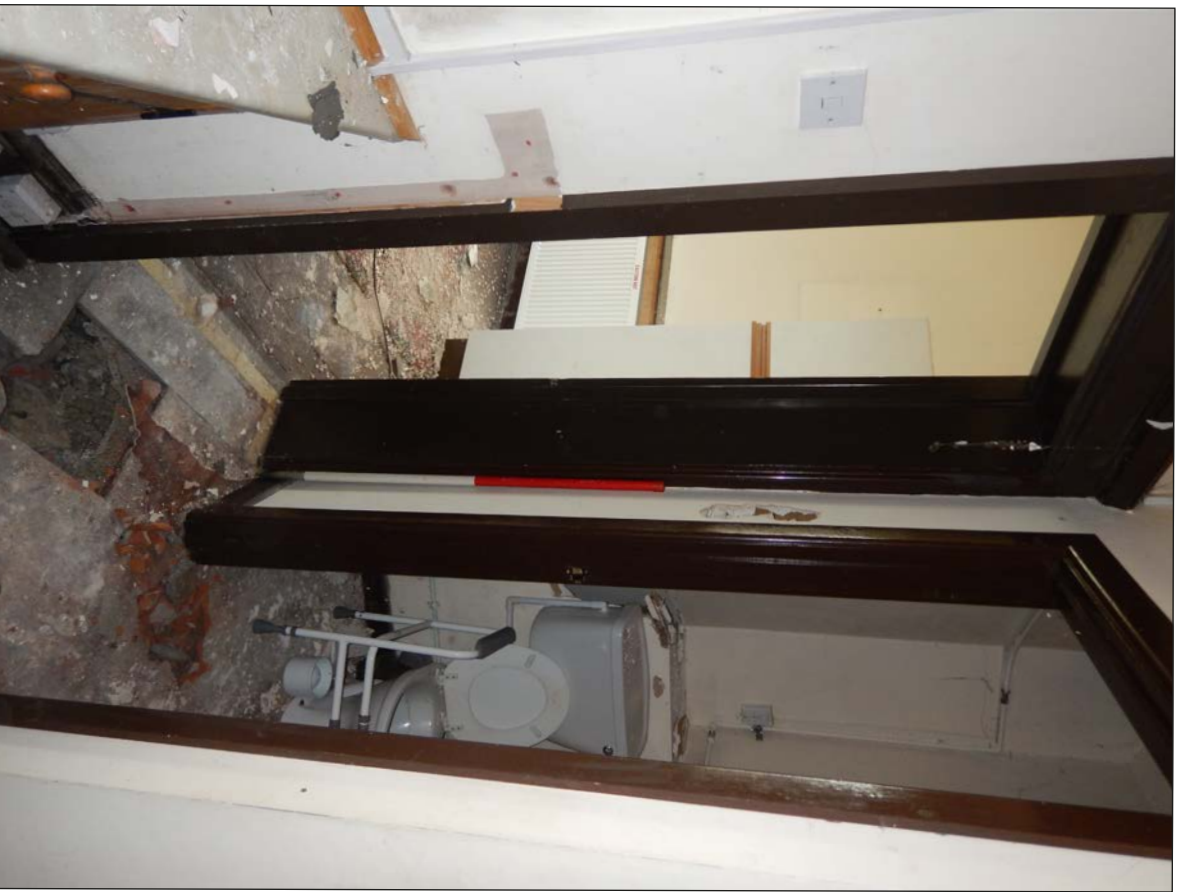
Plate 77. Doors to Minister's Room (left) and toilet (right), looking S
