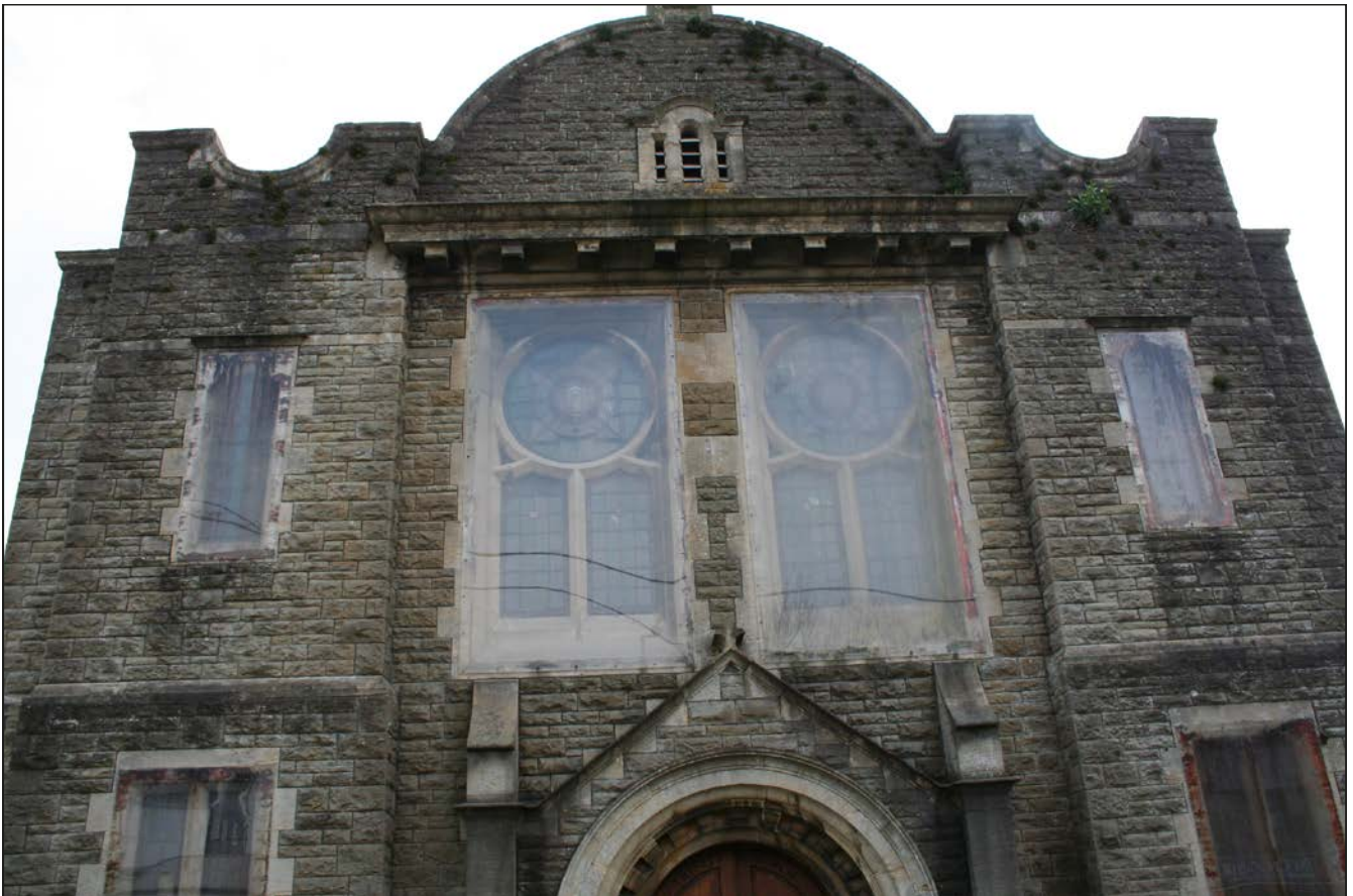
Plate 11. Front elevation, first floor level, looking SE
