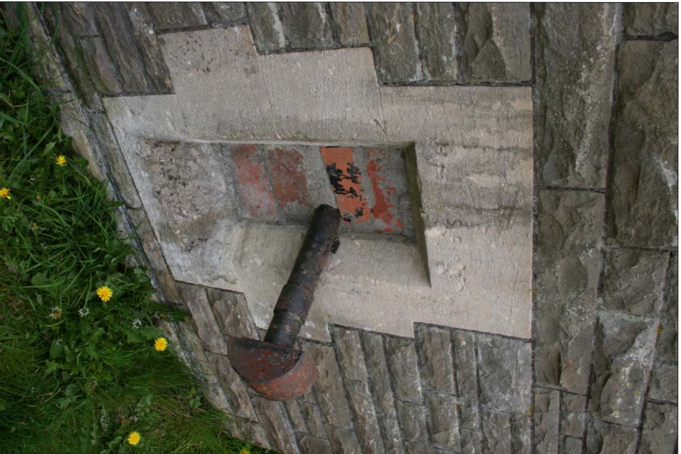
Plate 34. Detail of basement window, looking W
