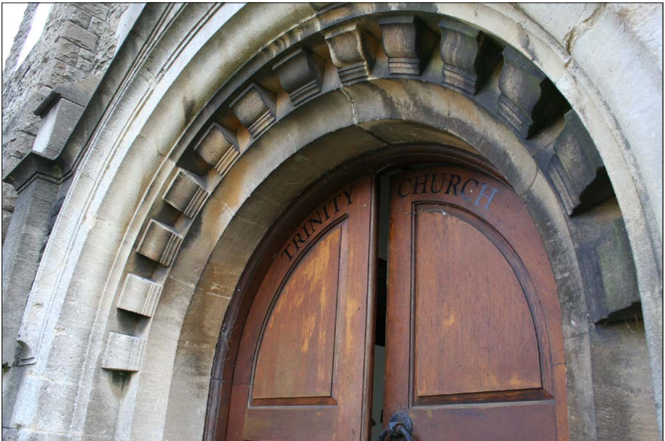
Plate 5. Detail of main entrance door surround
