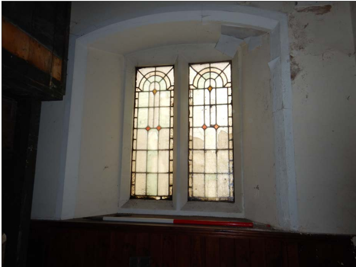
Plate 48. Ground floor window to NE wall of SE transept, looking NE
