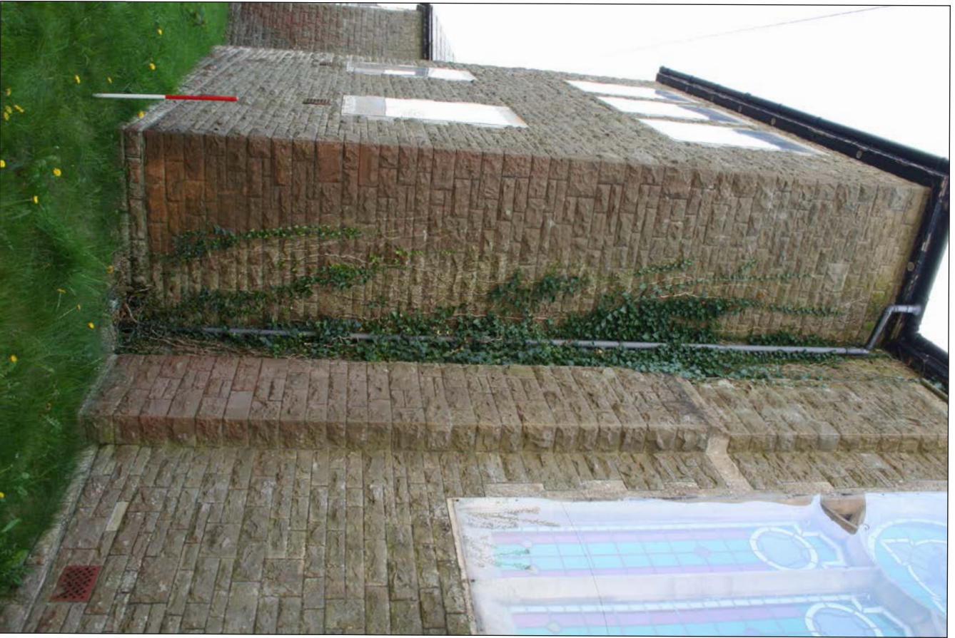
Plate 30. Oblique view of NE-facing elevation of SE hip end, looking SE
