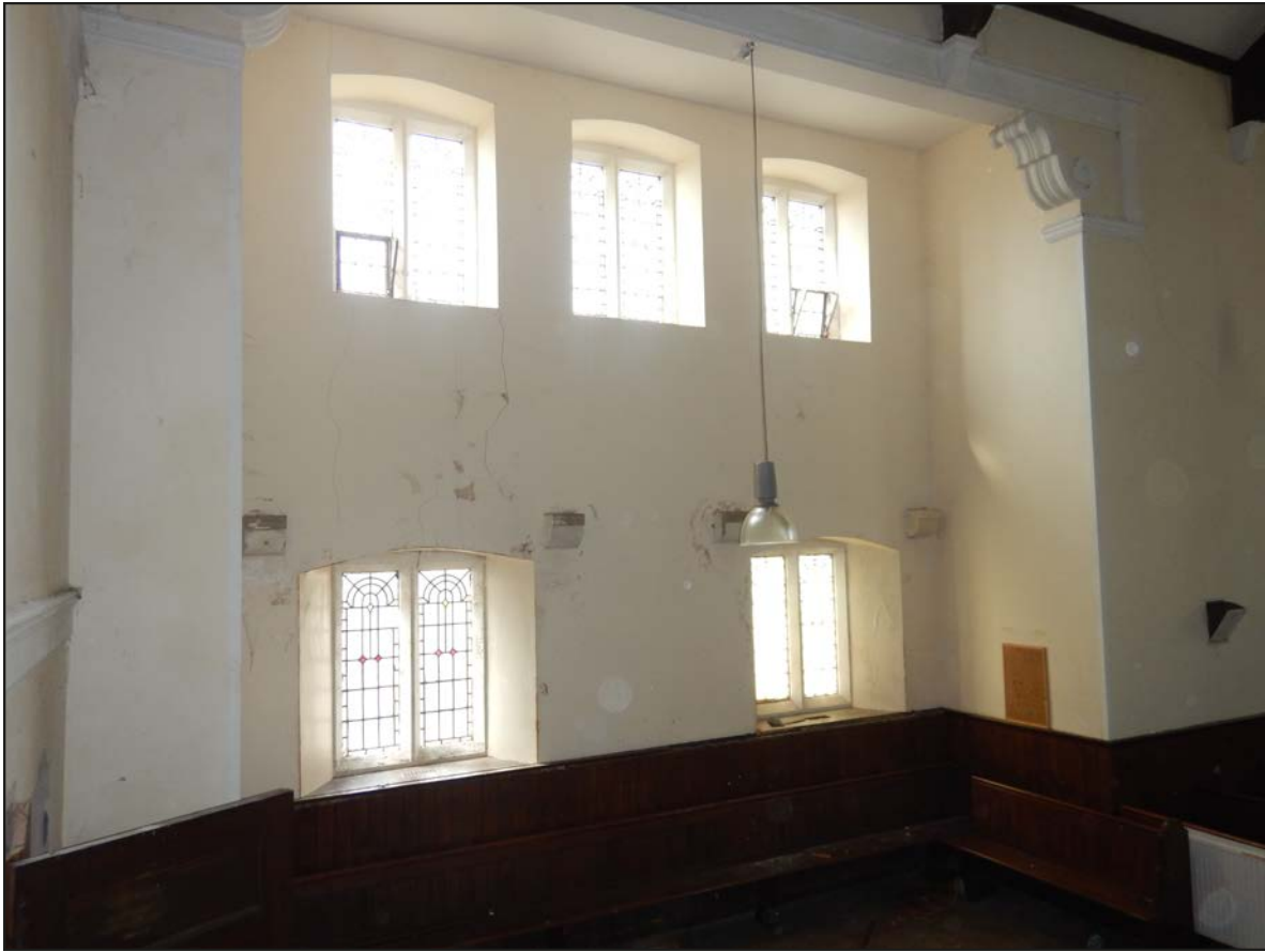
Plate 50. SW wall of SW transept, looking W
