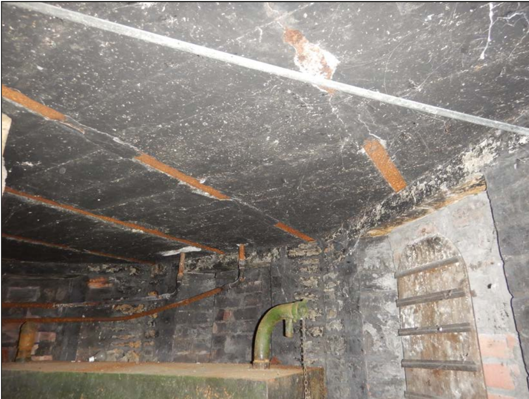
Plate 91. Chapel basement ceiling, looking N
