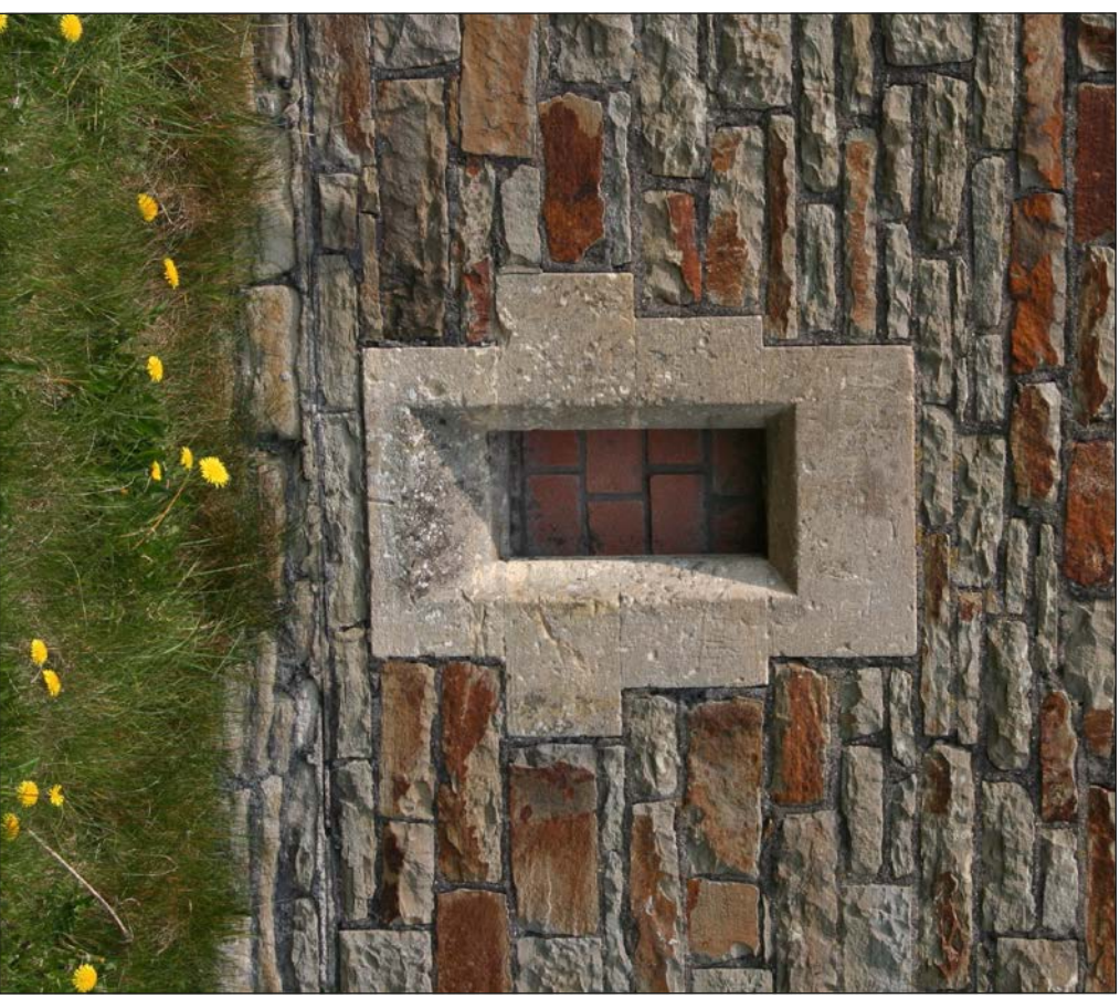
Plate 27. Detail of blocked window to basement of rear projecting element, looking NW
