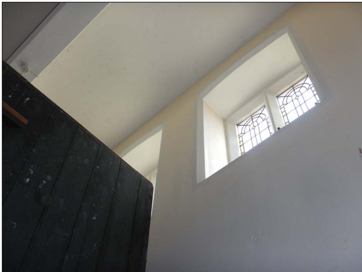
Plate 49. Upper window to NE wall of SE transept, looking NE
