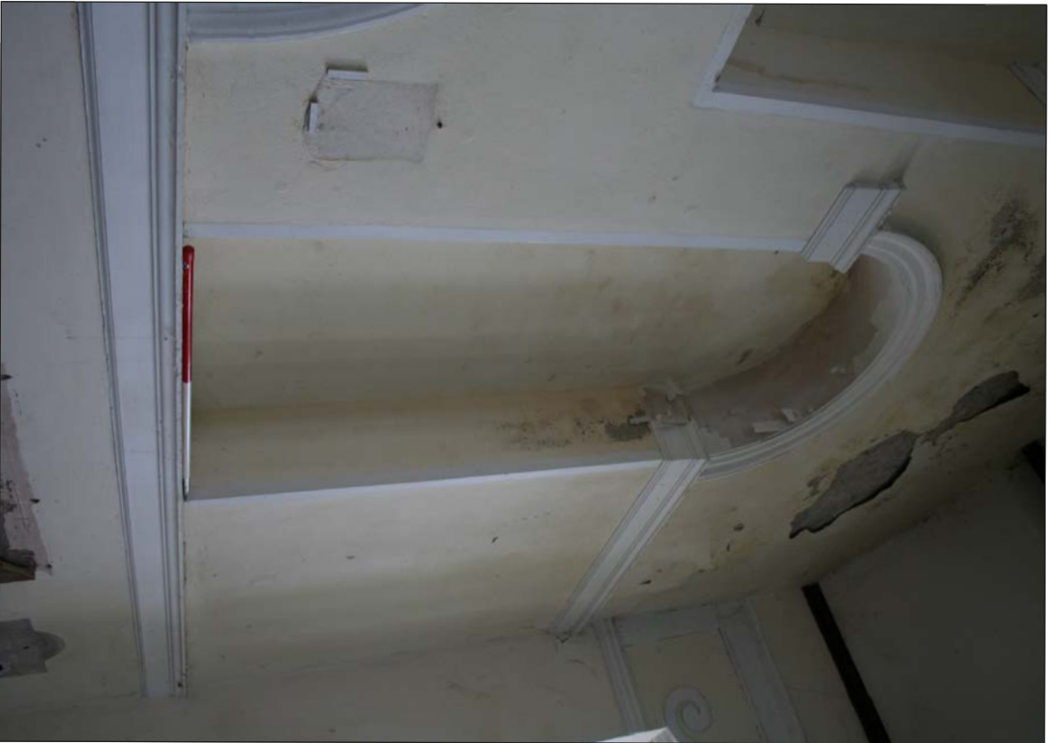
Plate 54. Detail of rear wall, flanking arched recess, looking S
