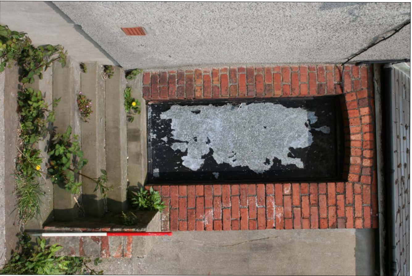
Plate 18. Door to SW-facing elevation of rear projecting element, looking NE
