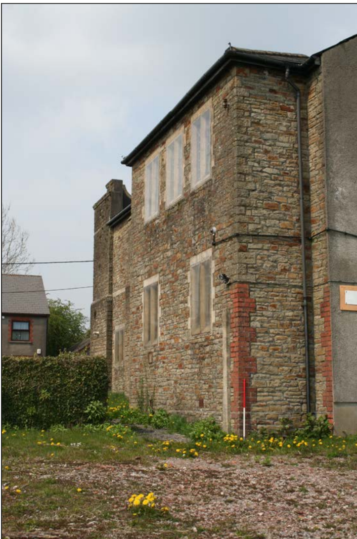
Plate 15. Window to NW end of SW-facing elevation, looking NE
