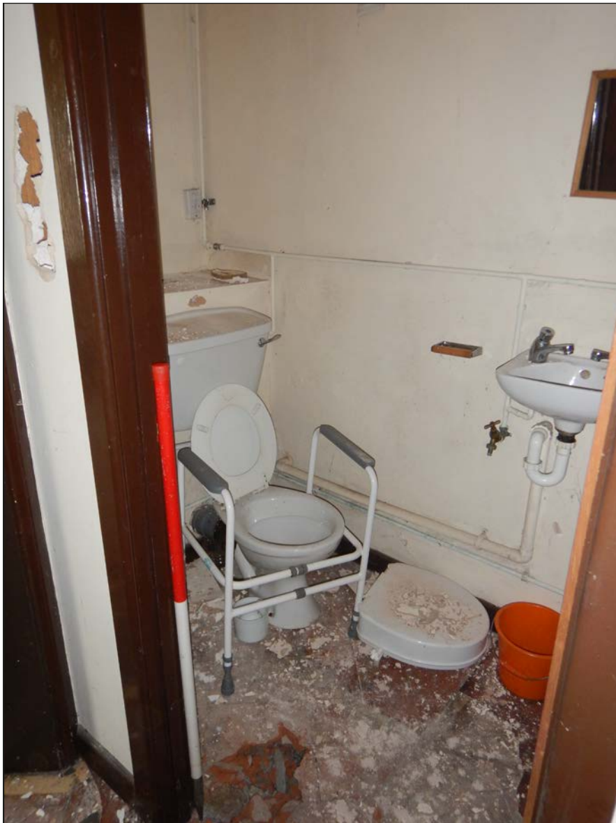
Plate 83. Toilet, looking S
