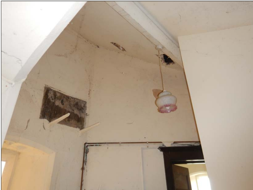
Plate 75. Corridor/kitchen ceiling, looking SE
