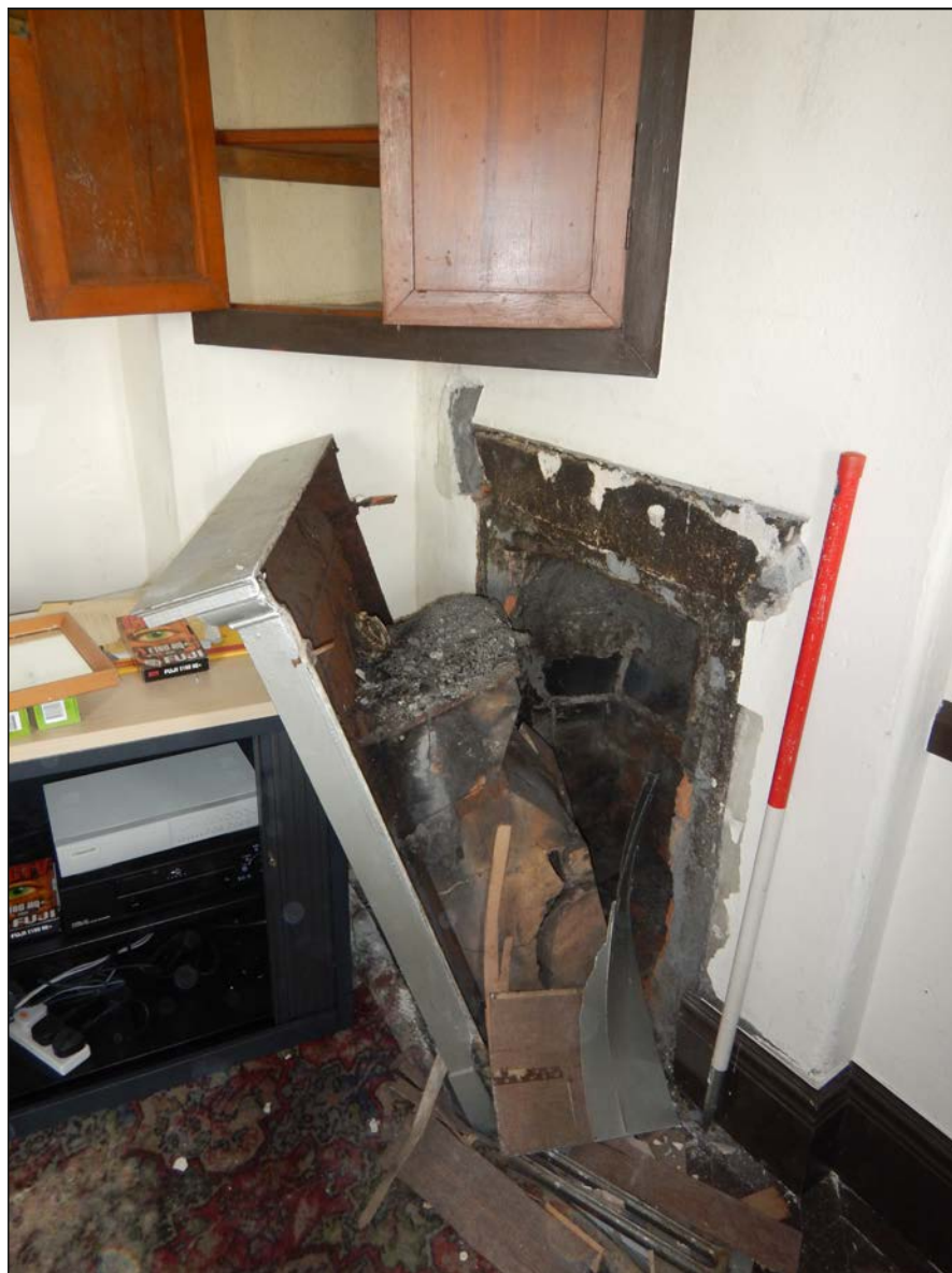
Plate 87. Fireplace on N wall of Minister's Room, looking NW
