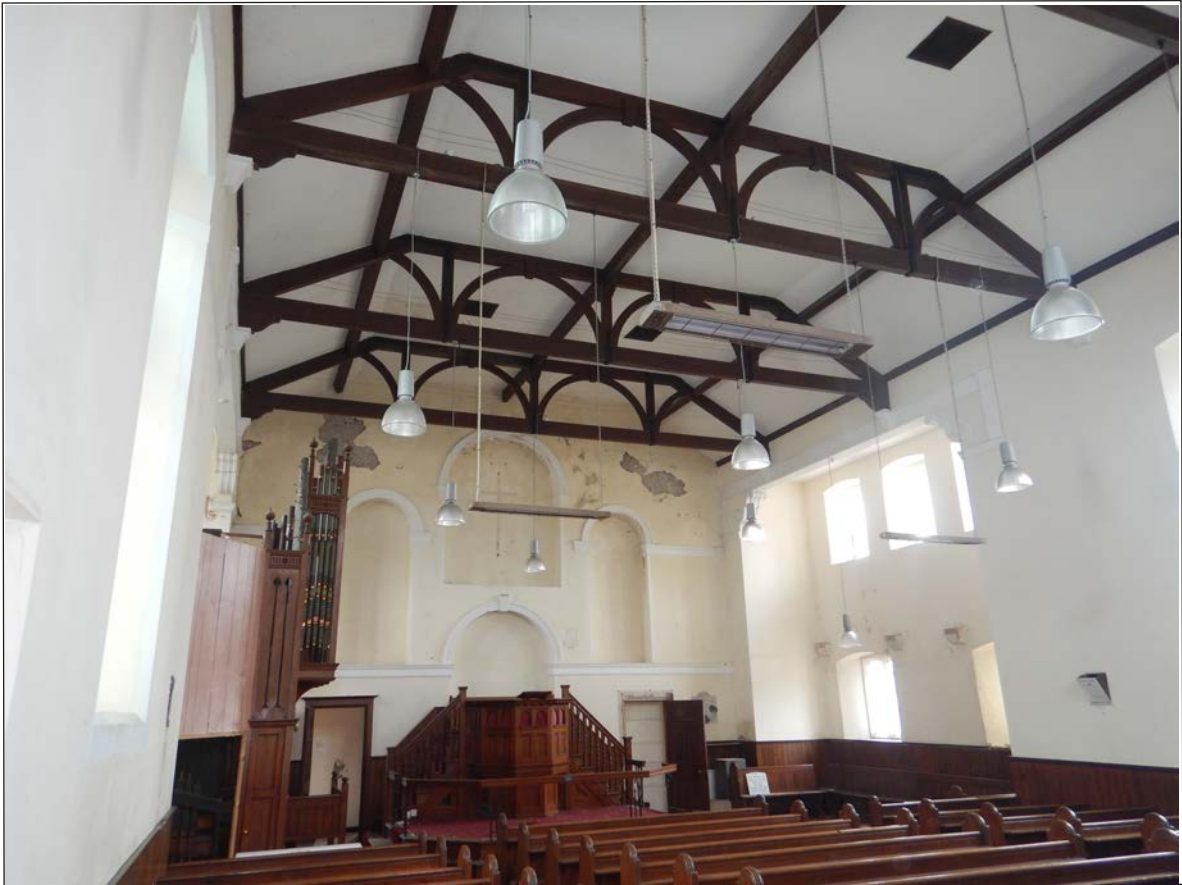
Plate 72. Nave ceiling, looking S
