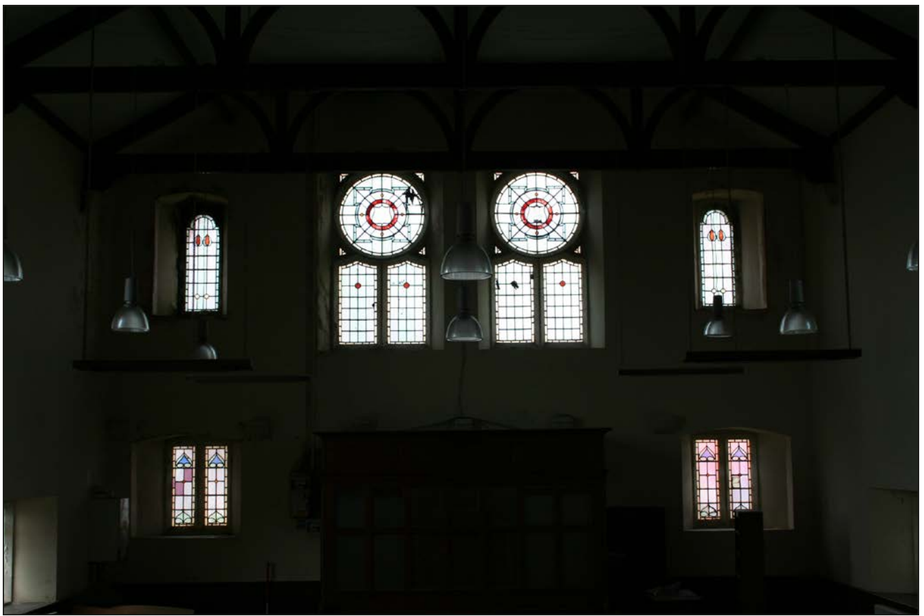
Plate 42. Upper windows to NW wall of nave, looking NW
