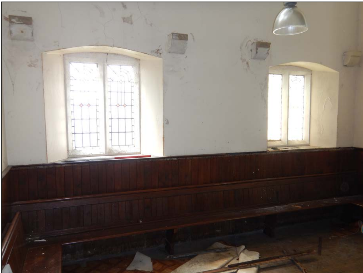
Plate 51. Ground floor windows to SW wall of SW transept, looking W
