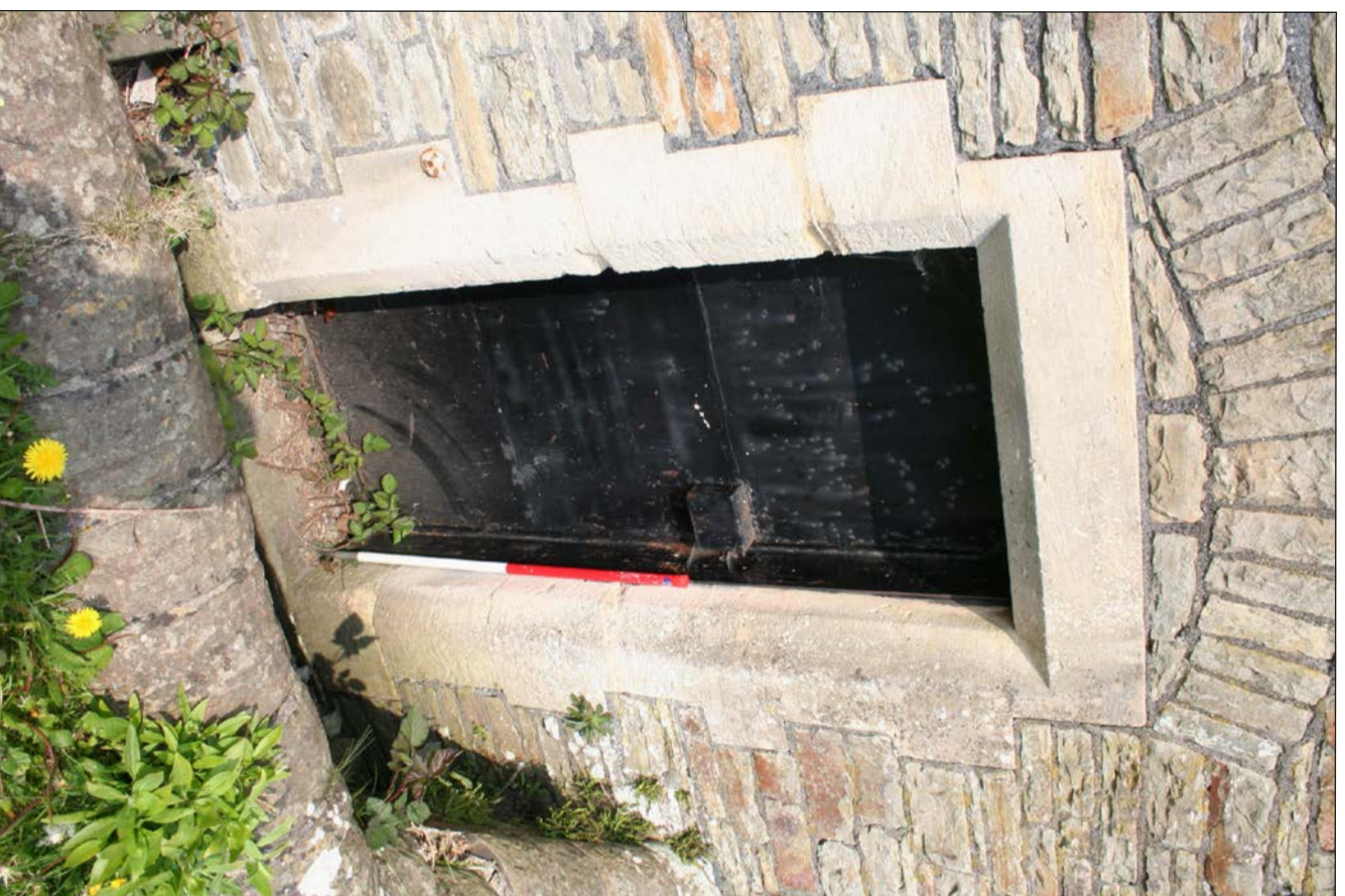
Plate 25. Door to basement of rear projecting element, looking N
