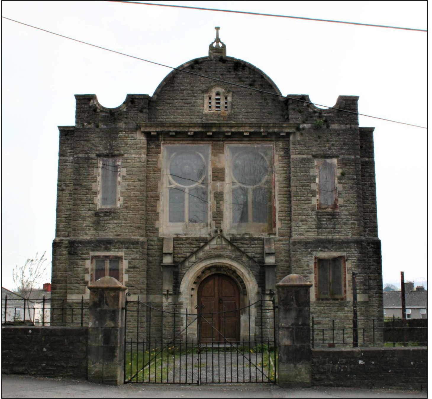
Plate 1. Trinity Chapel facade.
