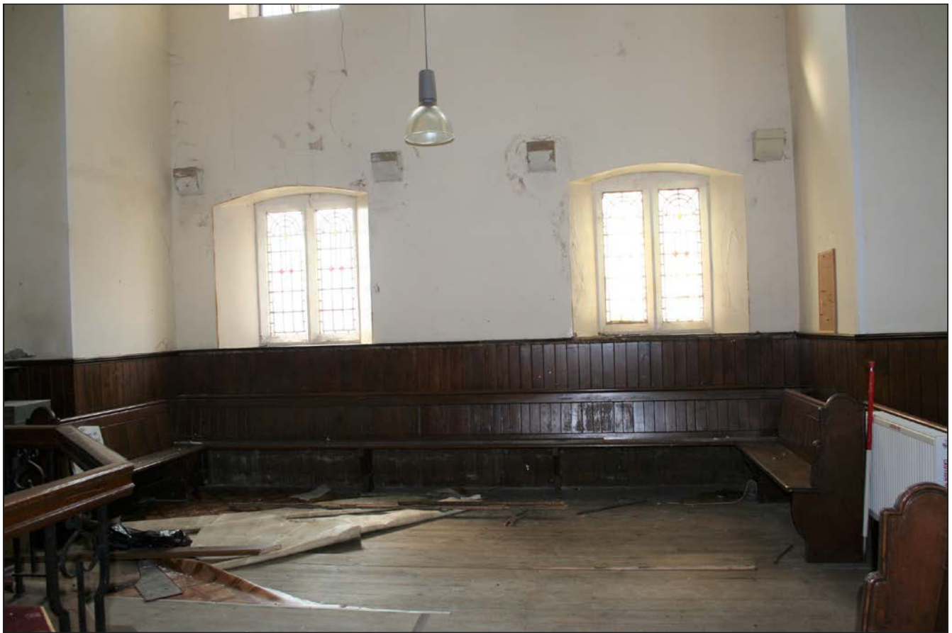
Plate 70. SW transept, looking SW
