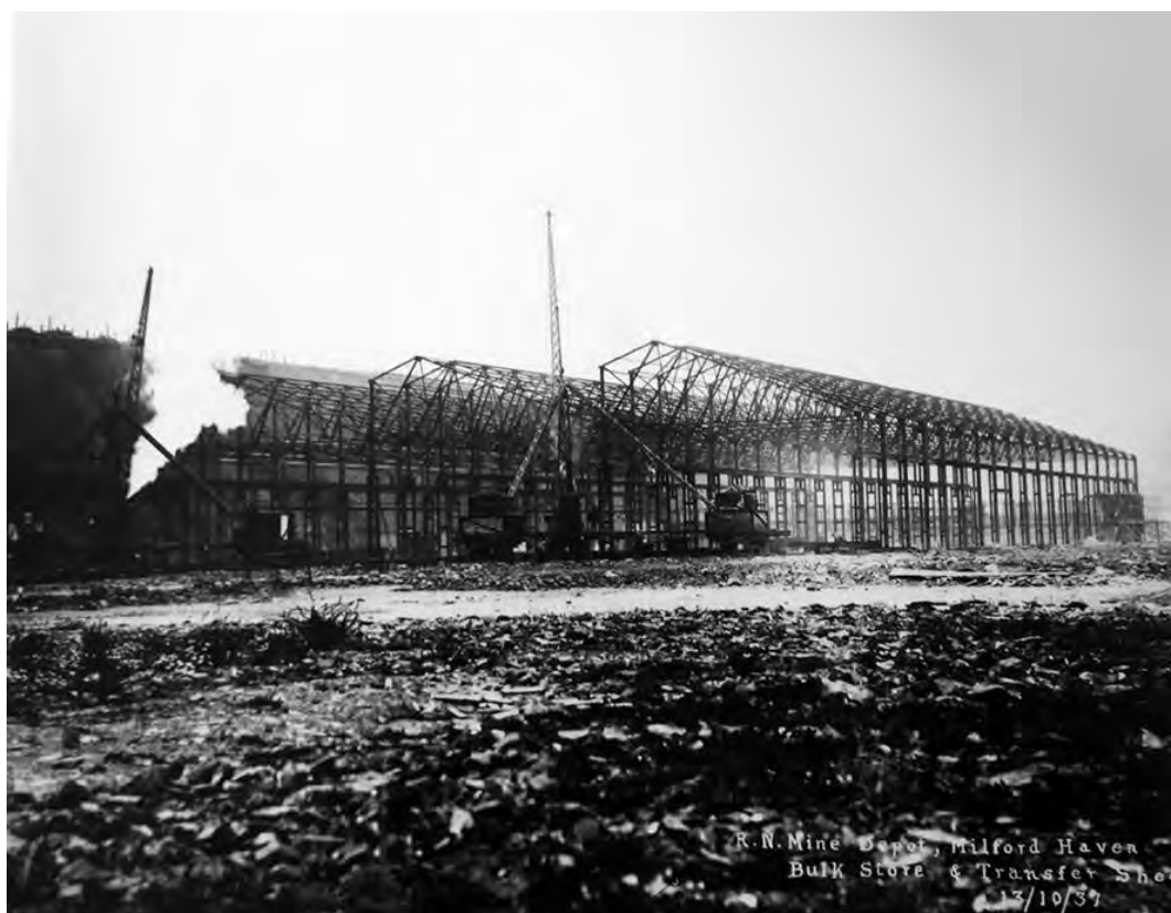
Photo 8: The Bulk Store (PRN 26001) under construction, 1937. Image courtesy of Scolton Manor Museum.
