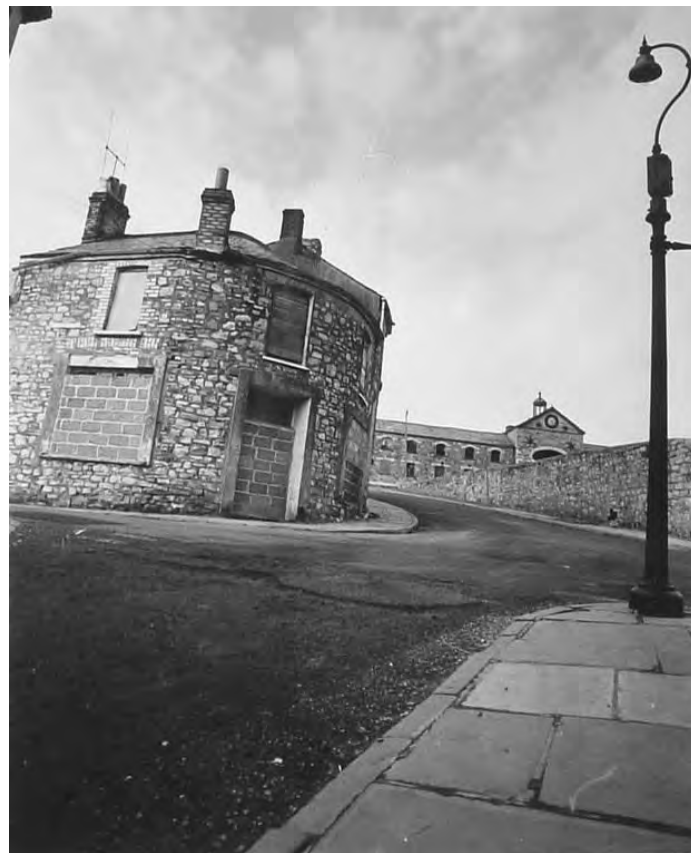
Photo 10. View taken from the corner of East Street and Commercial Street, looking north towards the Dowlais Stables. The property in the foreground lies within the proposed development area. Photo taken in the 1970s, prior to demolition. Image available on www.alangeorge.co.uk .
