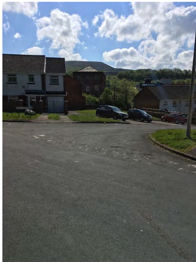
Photo 20: View southeast from the southeast corner of the site, looking towards Listed Building Dowlais Works Blast Engine House (LB 11491), with modern housing in the foreground.
