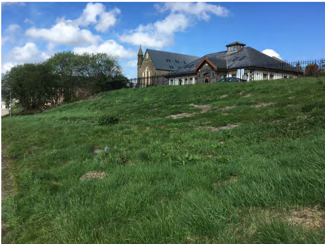
Photo 12: View west-northwest across the proposed development area. Cancer Aid building and St John's Church (PRN 4310m, LB 17931) visible in the centre. The Library (LB 27083) lies behind the trees to the left.
