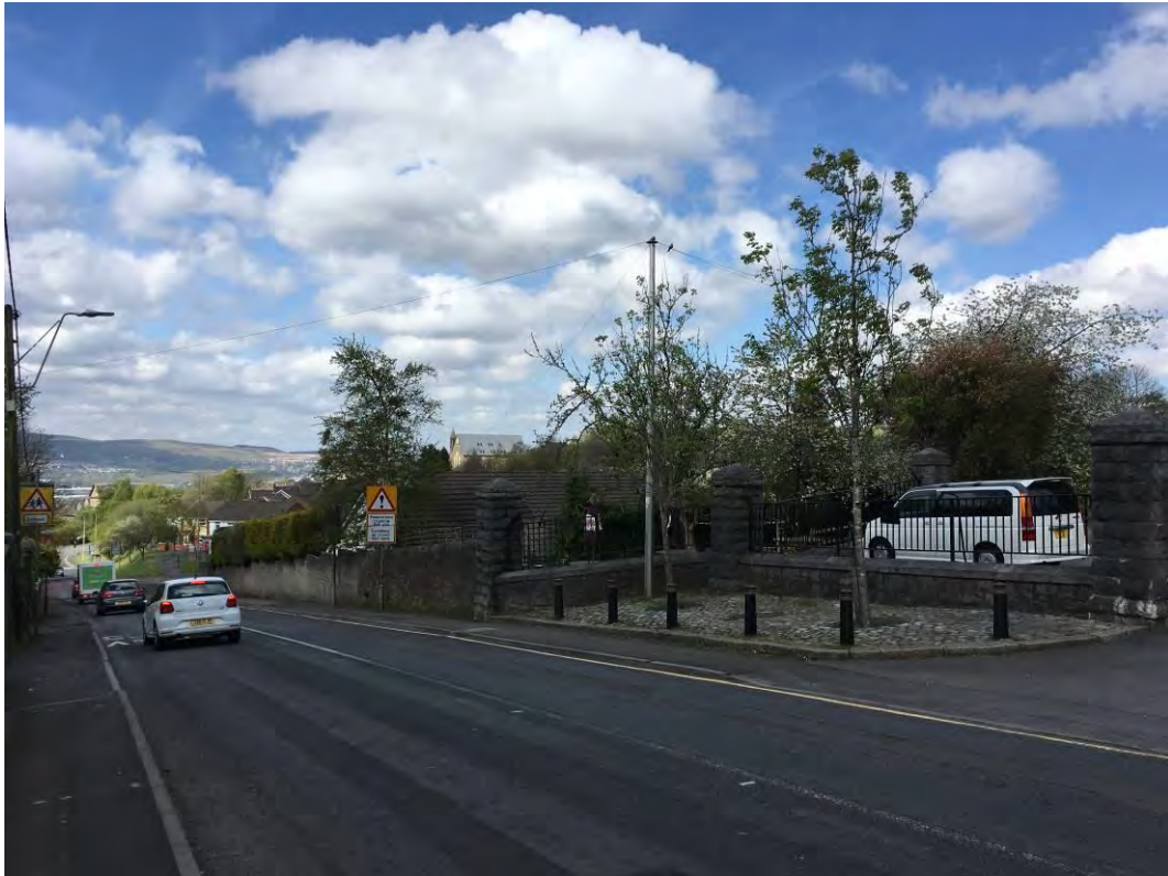
Photo 23: View west towards the site from in front of Listed Building Former Guest Memorial Library (LB 11490). The roof of St John's Church (LB 17931) visible in the centre.
