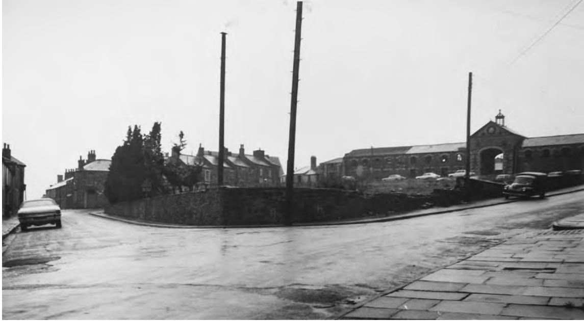
Photo 9: View west, from the corner of East Street and Market. The former site of the Market House is visible in the foreground, with the Dowlais Stables to the right, and the terraced housing fronting Commercial Street (within the proposed development area) in the centre. Photo taken in the 1970s prior to demolition works within the proposed development area. Image available on www.alangeorge.co.uk .
