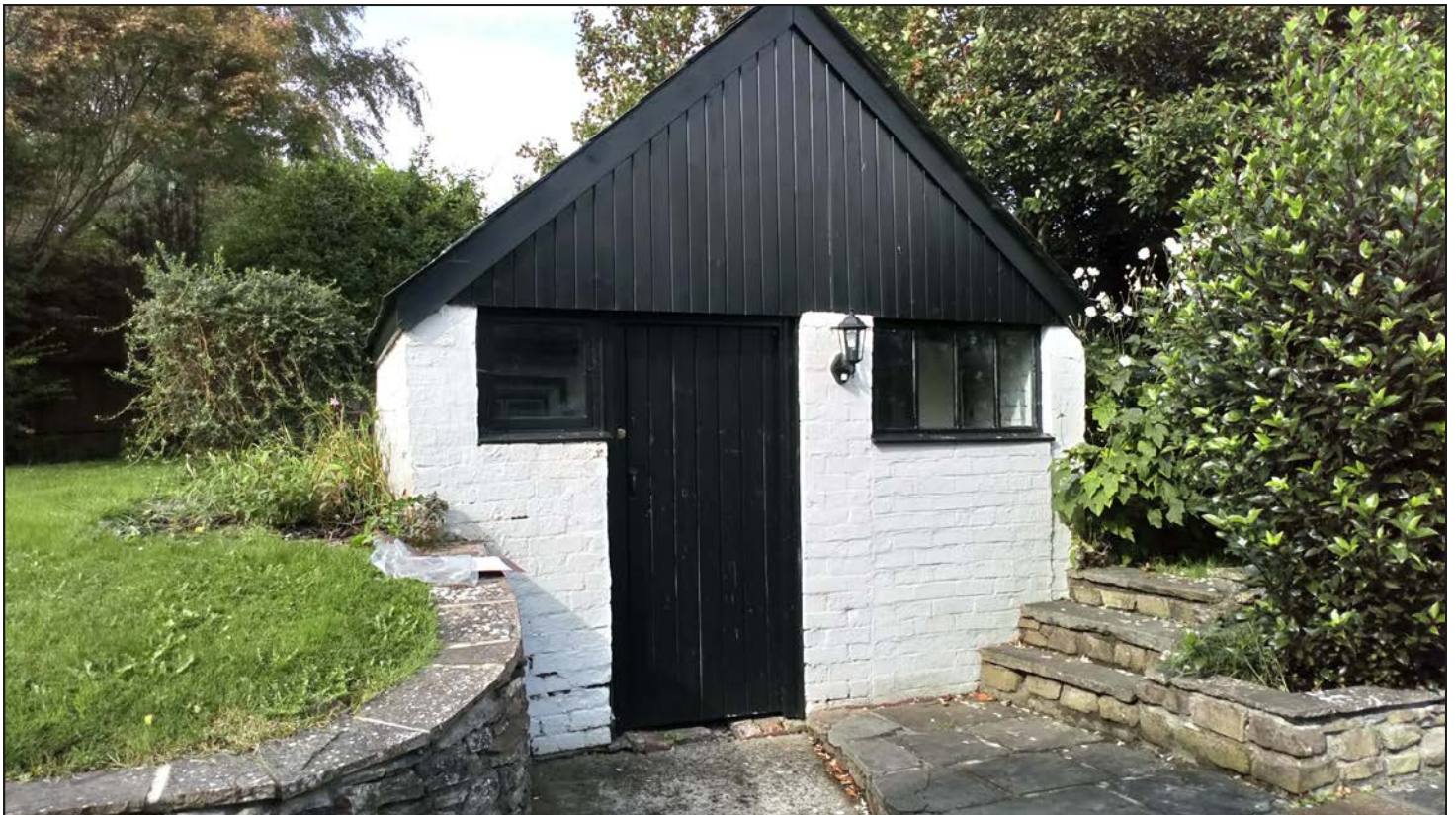
Plate 12. View of outbuilding.
