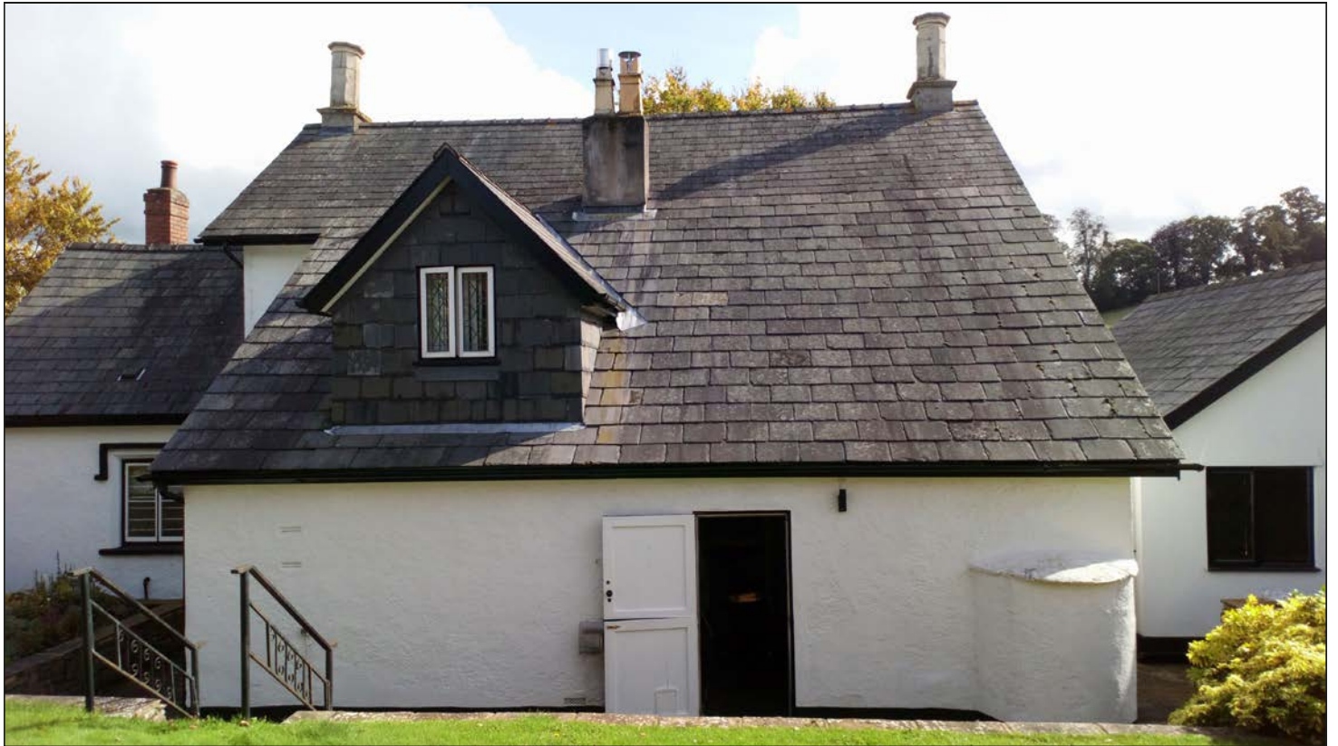
Plate 8. NW elevation looking SE.
