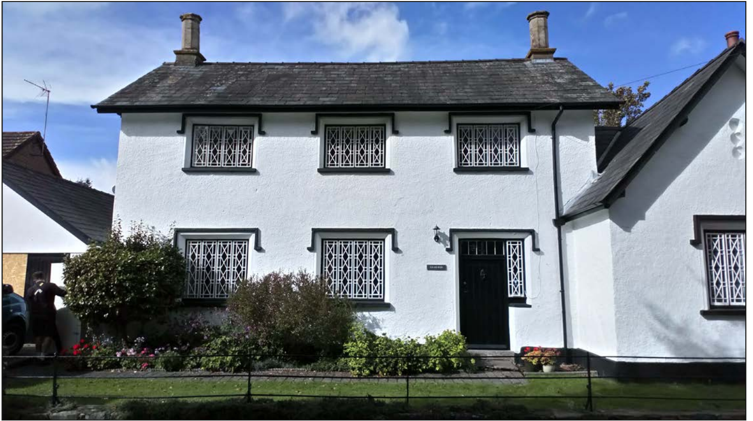
Plate 1. Front elevation looking NW.
