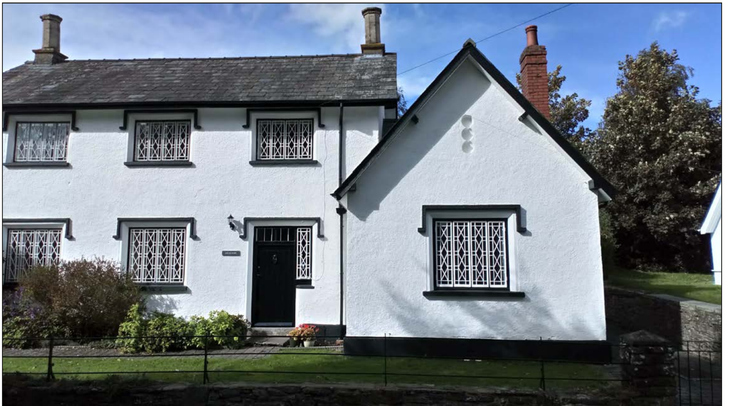
Plate 2. Front elevation looking NW.
