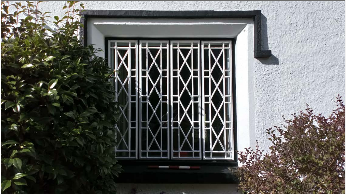
Plate 3. Detail of cast iron window.
