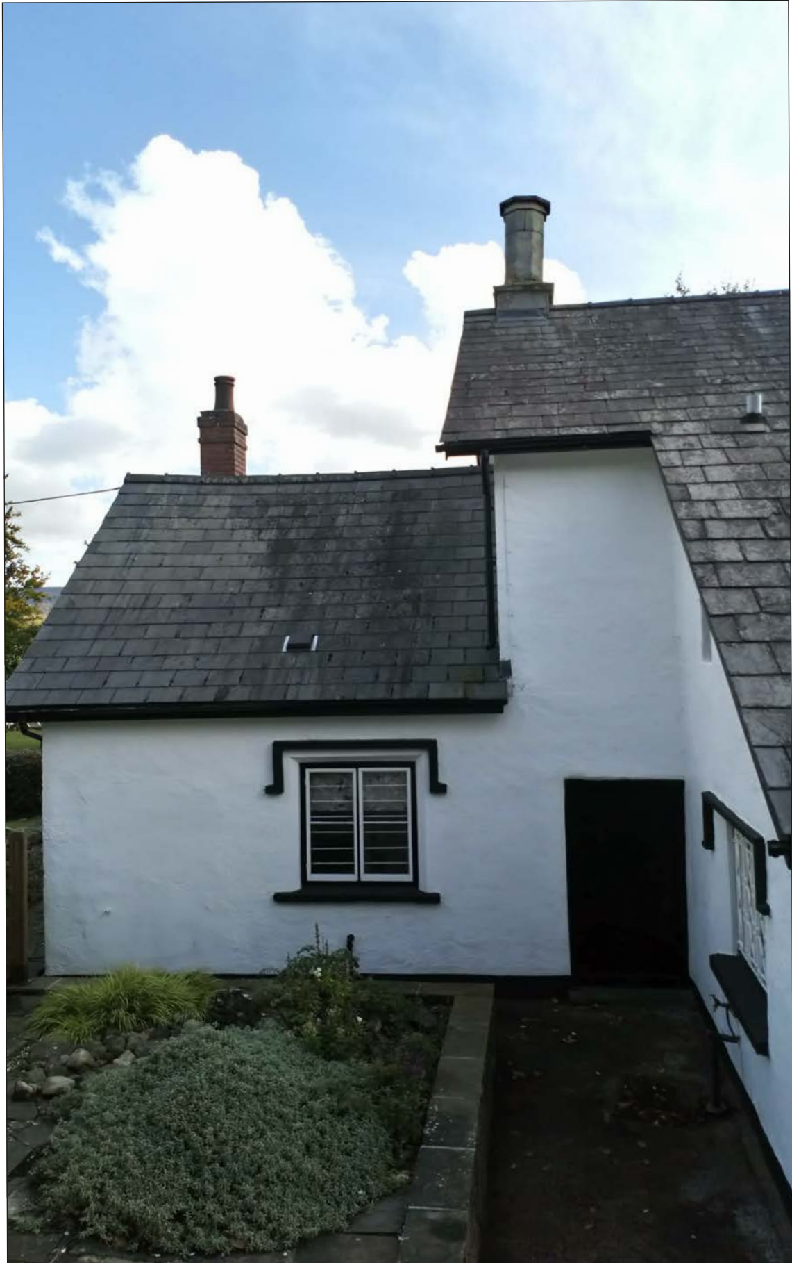
Plate 10. Extension looking SE.
