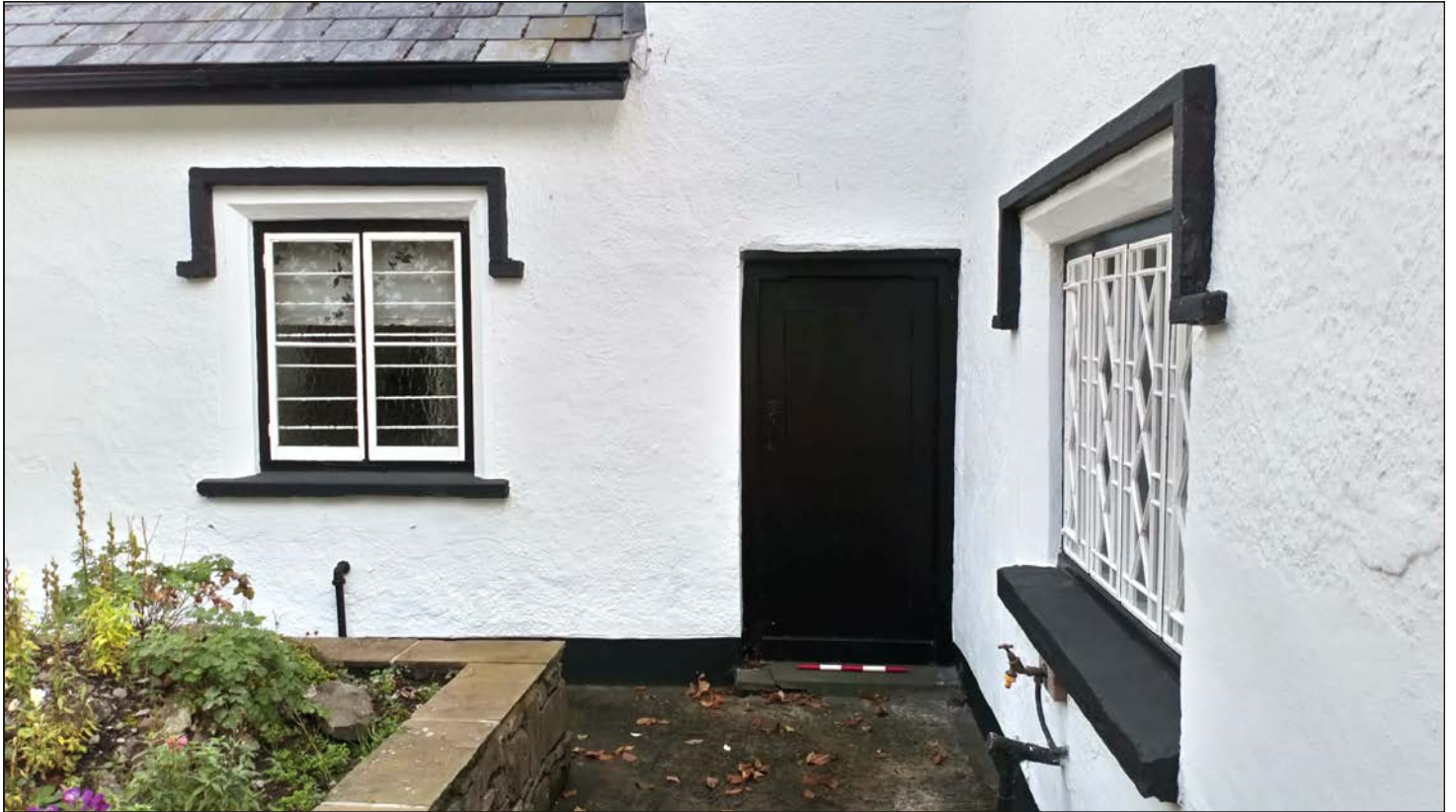
Plate 11. Extension looking SE.
