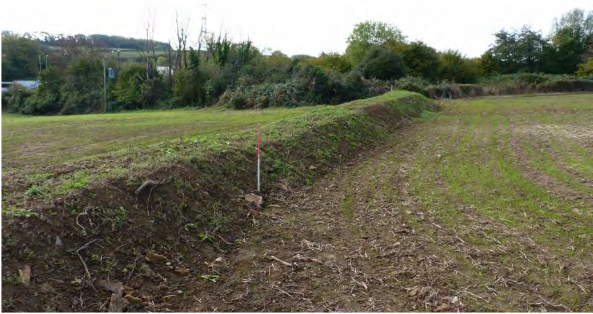
Photo 26: Newly created boundary SE corner of D1, between D1 and C4. 1m scale. Looking SW.
