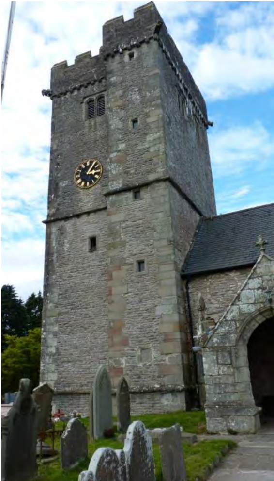
Photo 41: Church tower (LB 11246). Looking NNW.
