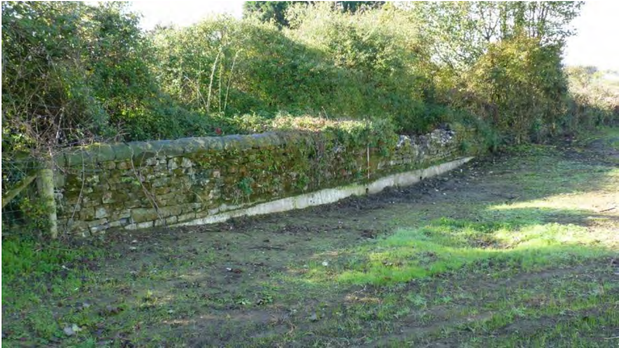
Photo 20: Mortared stone walling along the southern boundary where A3 meets C3, adjacent to roundabout on the A48. 1m scale. Looking SW.
