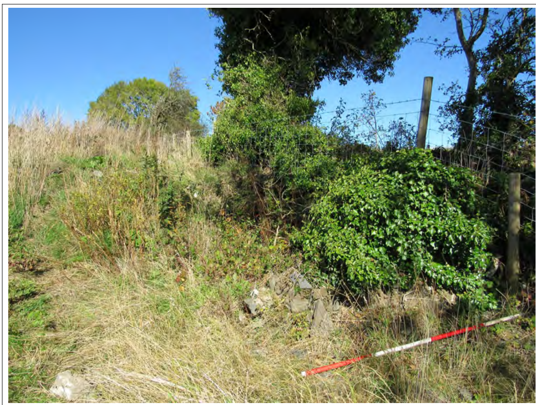
Plate 23. Northern wall protruding westwards from eastern boundary dry stone wall. View N. 2m scale.
