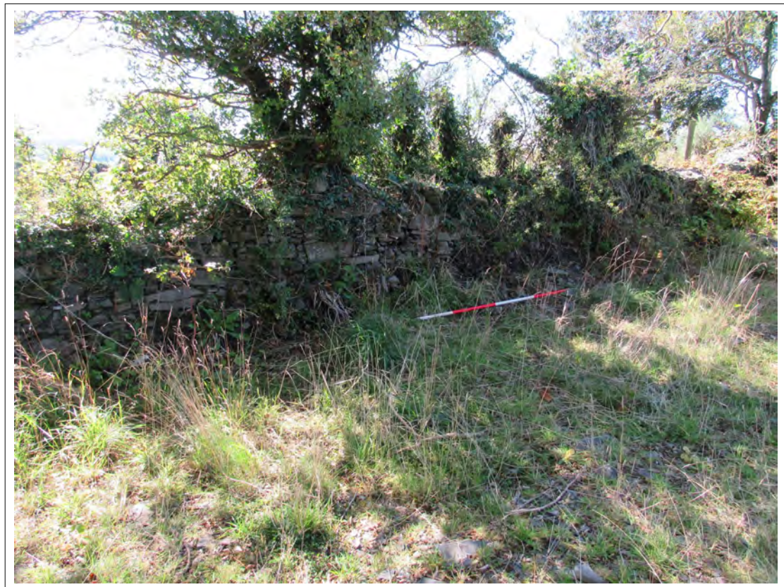
Plate 20. Southern dry stone boundary wall. View SW. 2m scale
