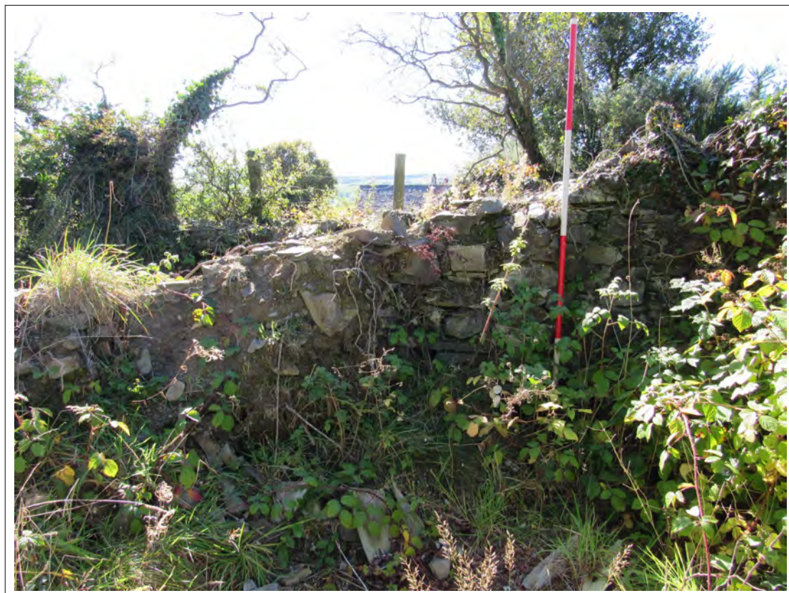
Plate 18. House ruins, southern wall interior. View S. 2m scale
