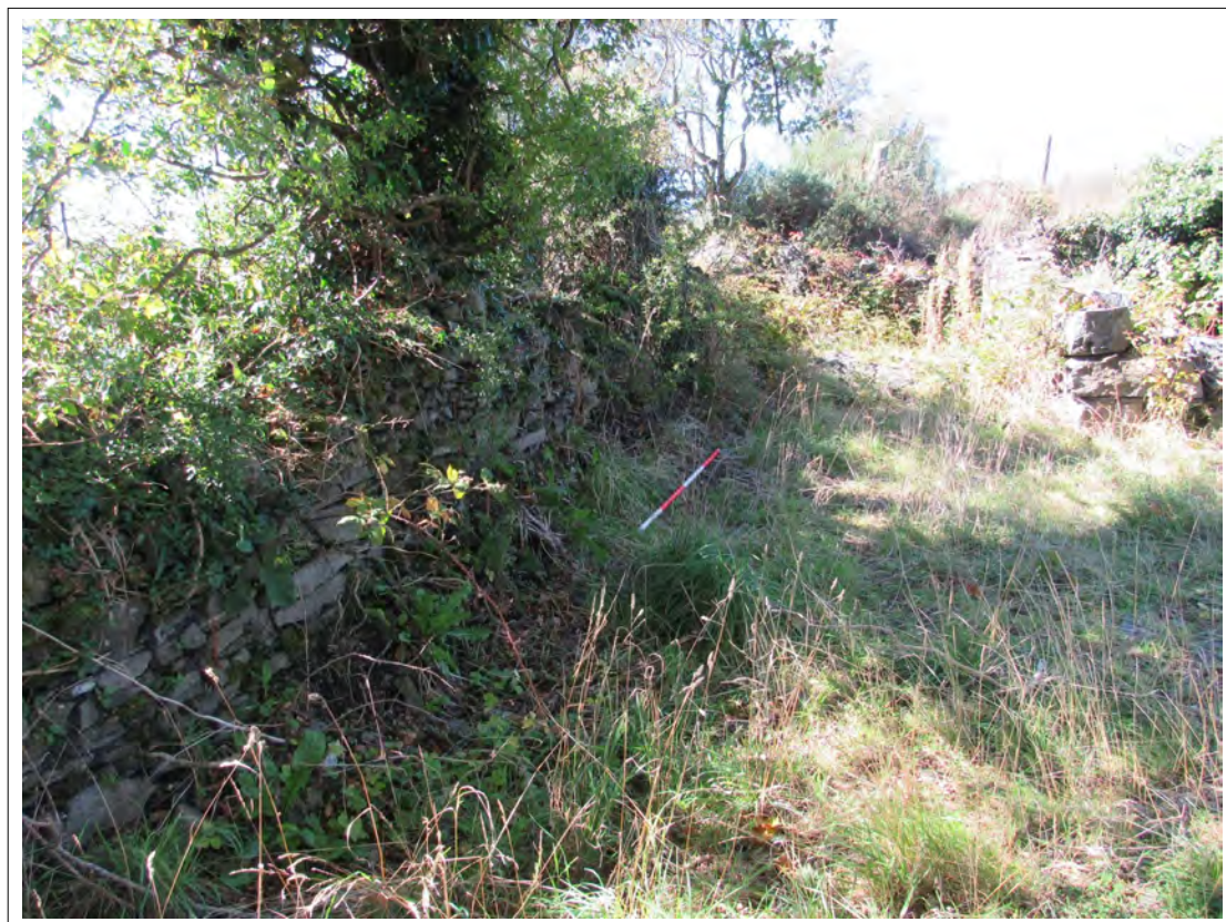
Plate 22. Southern and western dry stone boundary wall. View W. 2m scale
