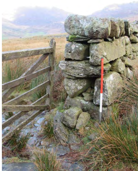
Photo 3: Stone field boundary wall at the southern end of the proposed development area, which will be crossed by the pipeline route. View northeast. 1m scale.
