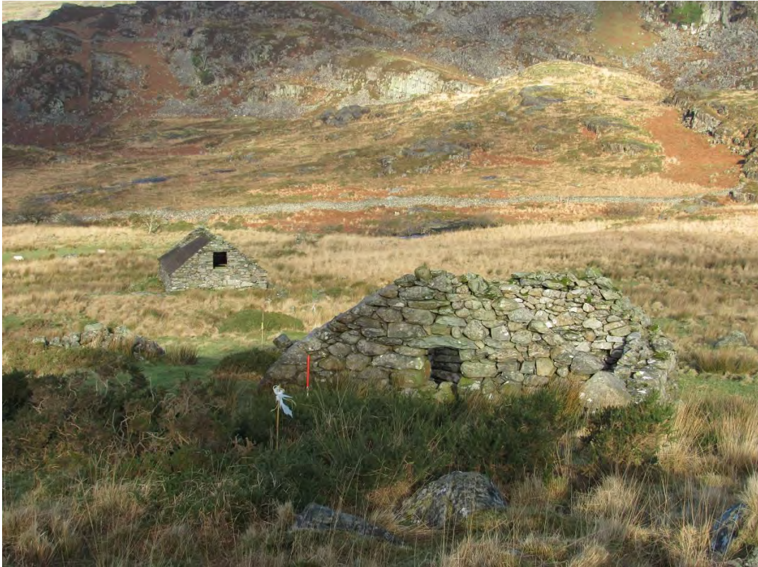
Photo 19: General view encompassing both barns HW02 and HW03, looking down the pipeline route which would pass to the left of the foreground barn, to a new turbine house in front of the rear barn. View north. 1m scale.
