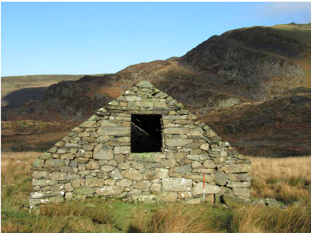
Photo 20: Northern gable wall of barn HW03. View NNW. 1m scale.
