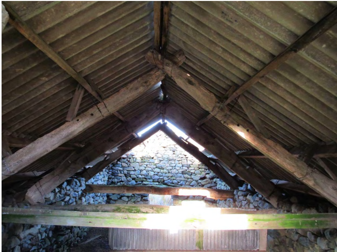
Photo 23: Internal roof structure of barn HW03. View NNW.
