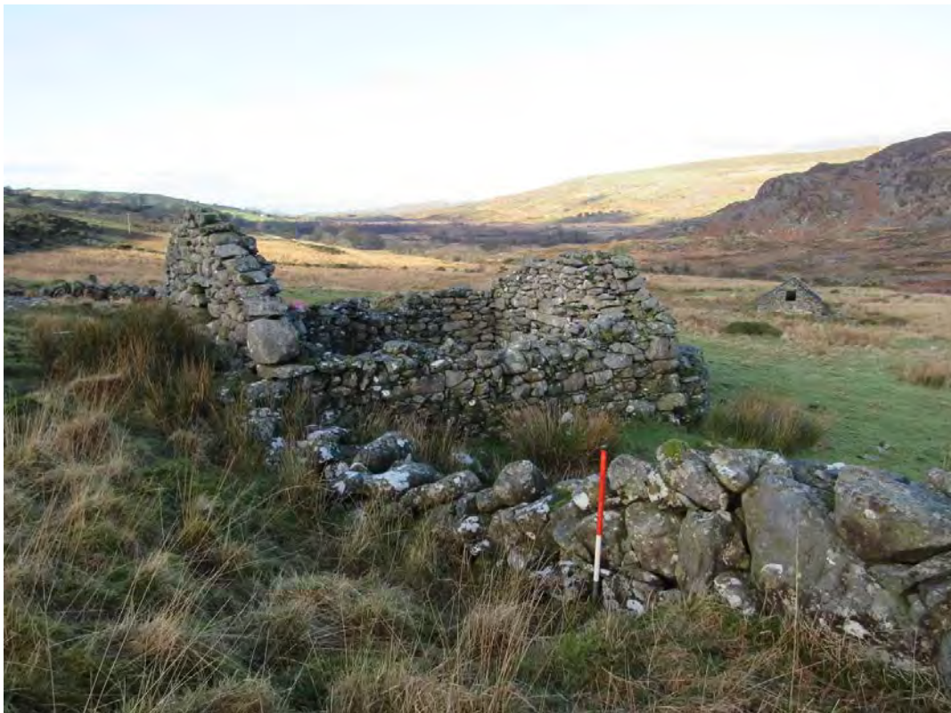
Photo 18: Dry-stone walling attached to the east side of the Cow Barn HW02. View WNW. 1m scale.
