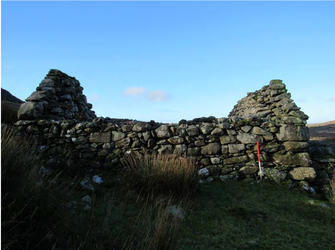
Photo 15: Eastern side wall of Cow Barn HW02. View west. 1m scale.
