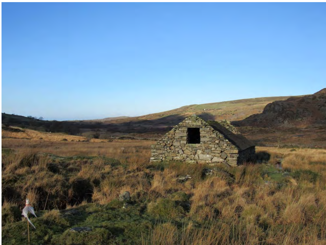
Photo 24: View of proposed turbine house location (marked by cane) in front of barn HW03. View northwest.
