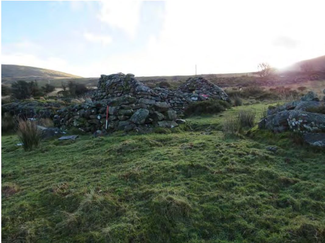
Photo 17: General view of Cow Barn HW02 showing attached dry-stone walling running off to the west. The pipeline route should pass through the visible opening in the wall. View southeast. 1m scale.
