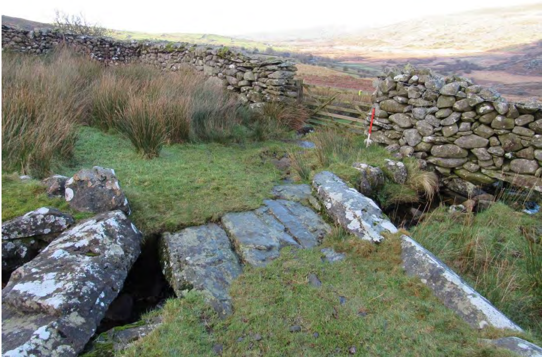
Photo 12: The footpath access through the wall illustrated in Photo 11, with the stone crossing the Hendre Waelod stream. View northwest. 1m scale.
