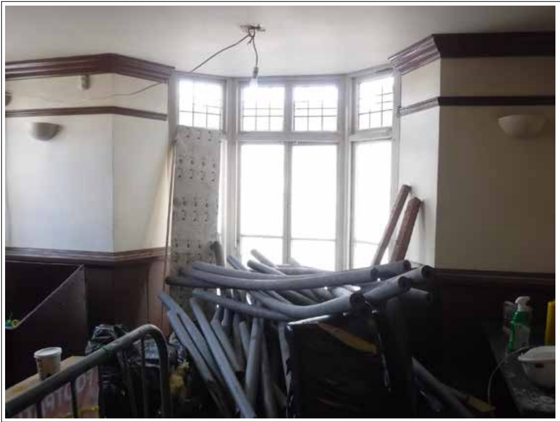
Plate 9. Internal room 12. Looking NE
