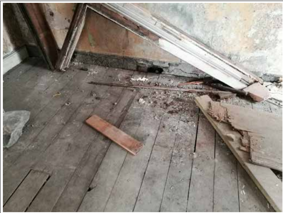
Plate 104. Floor room 11. Looking S.
