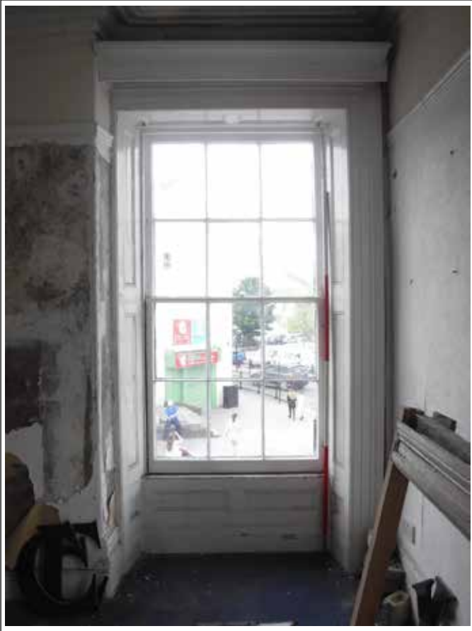
Plate 37. Room 25. Looking NW. Scale 2m
