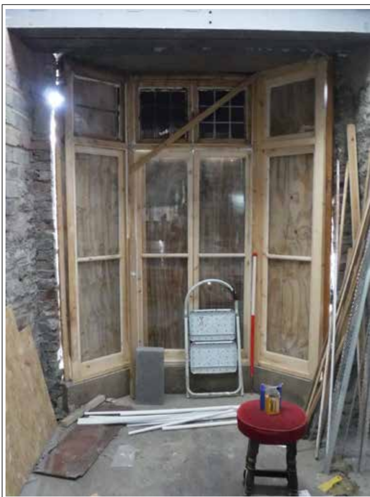
Plate 18. Bay window room 17. Looking N. Scale 1m
