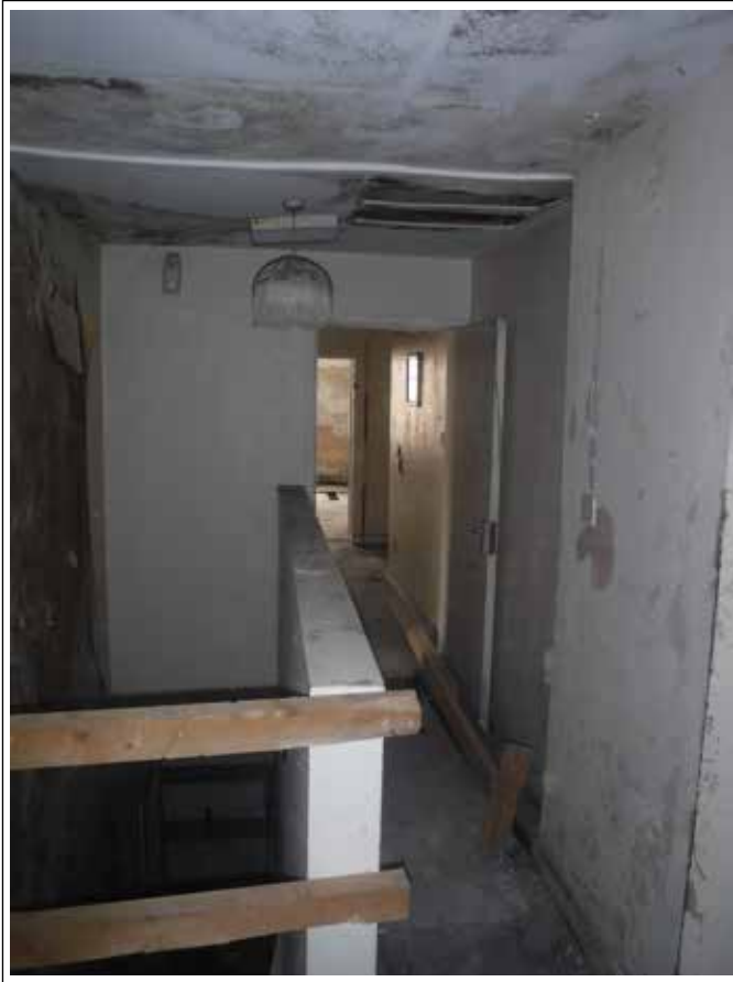
Plate 59. Corridor. Looking NW. Scale 2m
