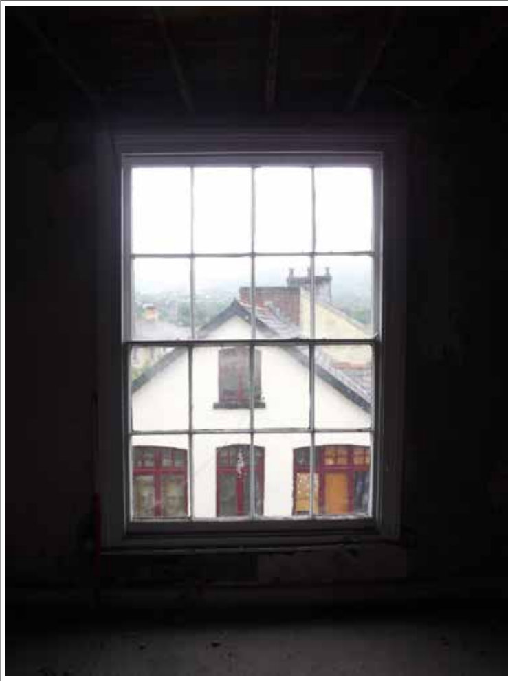
Plate 69. Window room 4. Looking NE. Scale 1m
