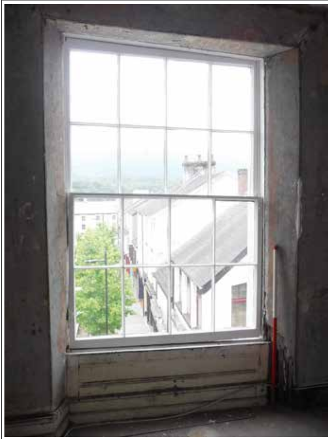
Plate 89. Window room 8. Looking NE. Scale 1m
