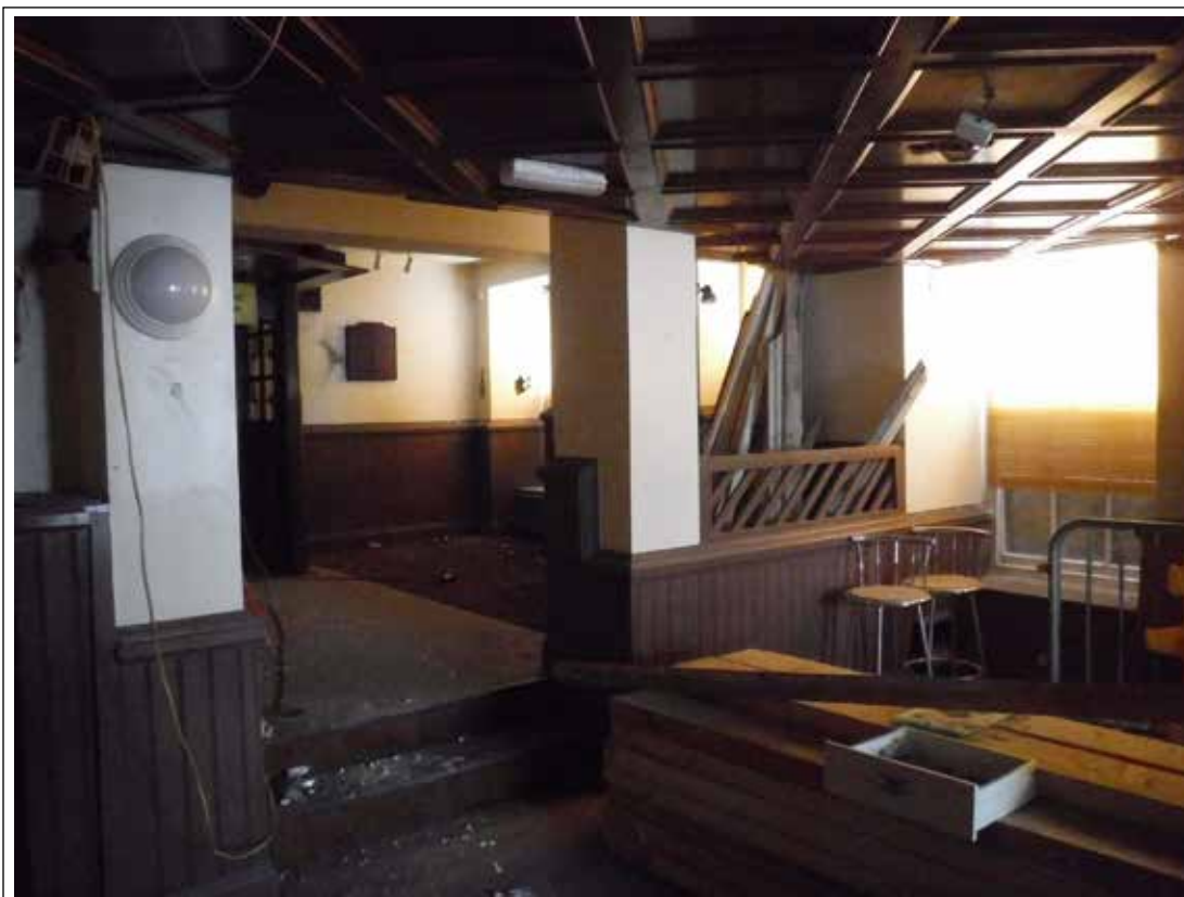
Plate 13. Internal room 12 towards 13. Looking W.
