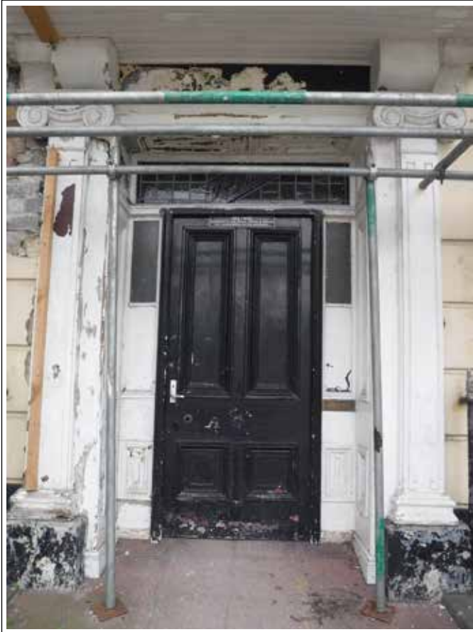
Plate 7. Hotel main entrance. Looking SW.
