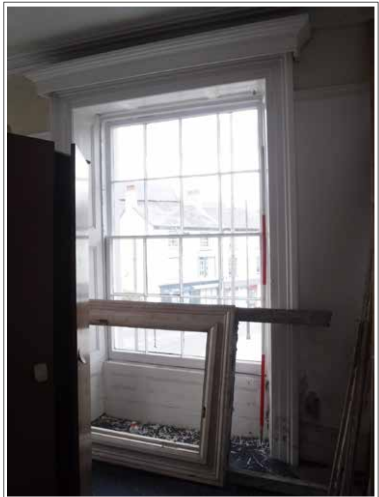
Plate 36. Room 25. Looking NE. Scale 2m
