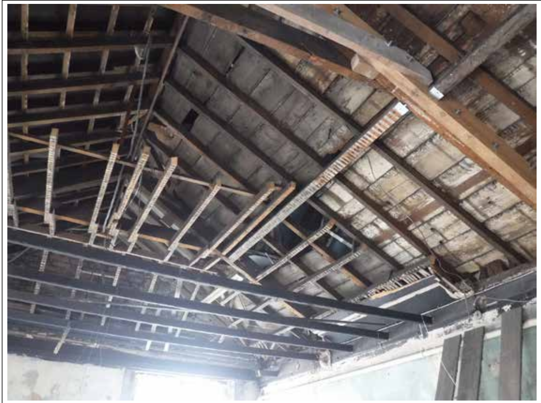
Plate 47. Ceiling room 29. Looking NW.
