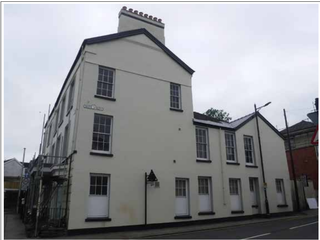
Plate 2. Monk Street elevation. Looking S.
