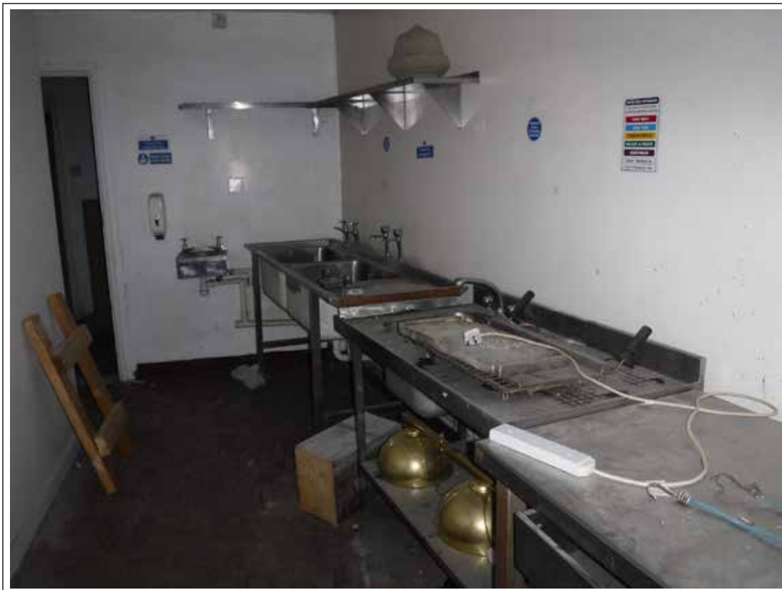
Plate 15. Kitchen room 14. Looking SW.
