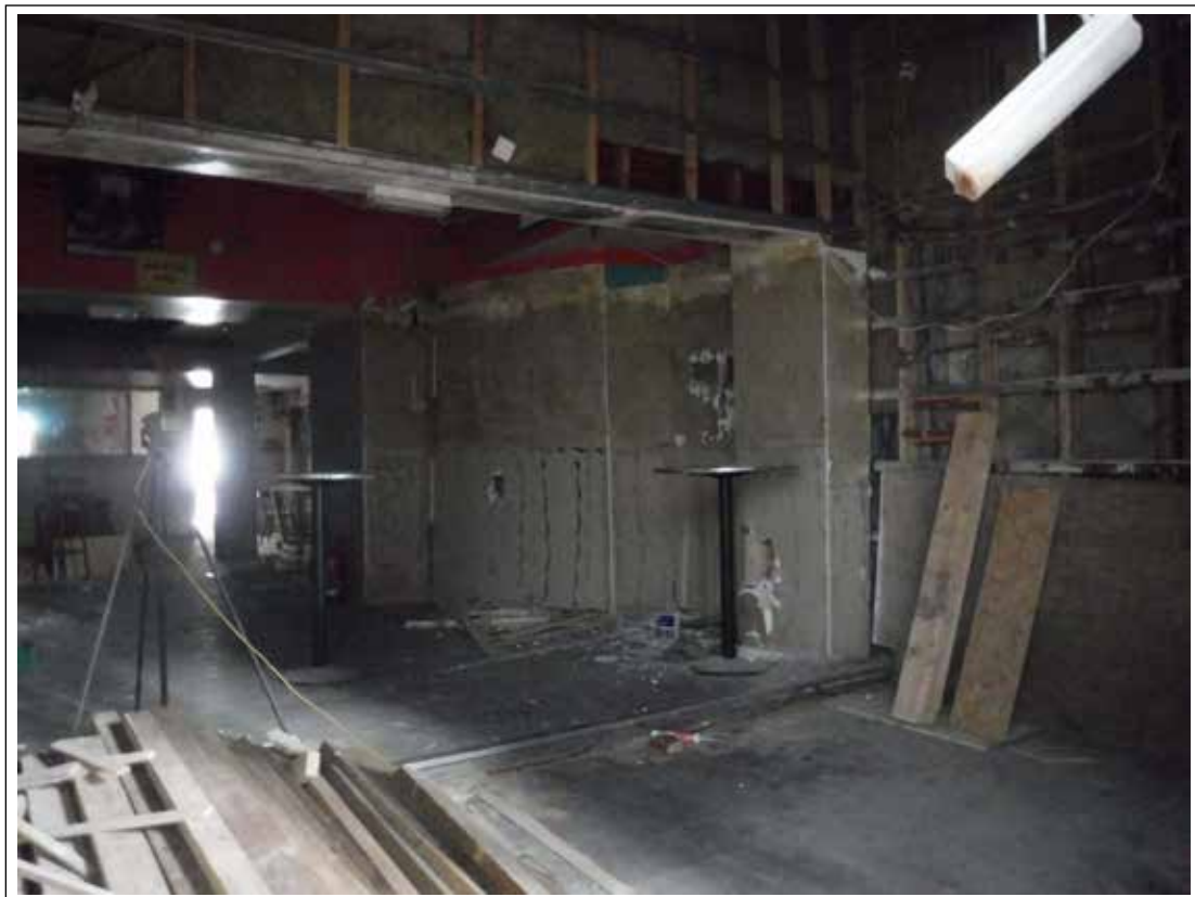
Plate 20. Room 20. Looking W. Scale 2m
