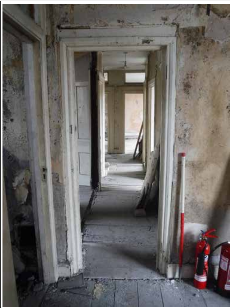
Plate 80. Corridor 2nd floor. Looking NW. Scale 1m
