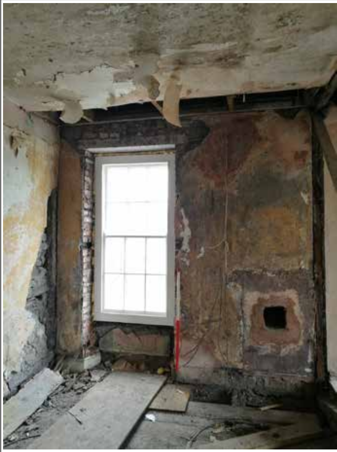
Plate 101. Room 11. Looking NW. Scale 1m
