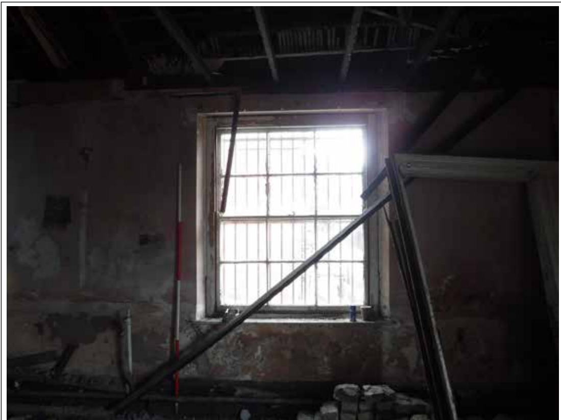
Plate 50. Room 29. Looking SW.
