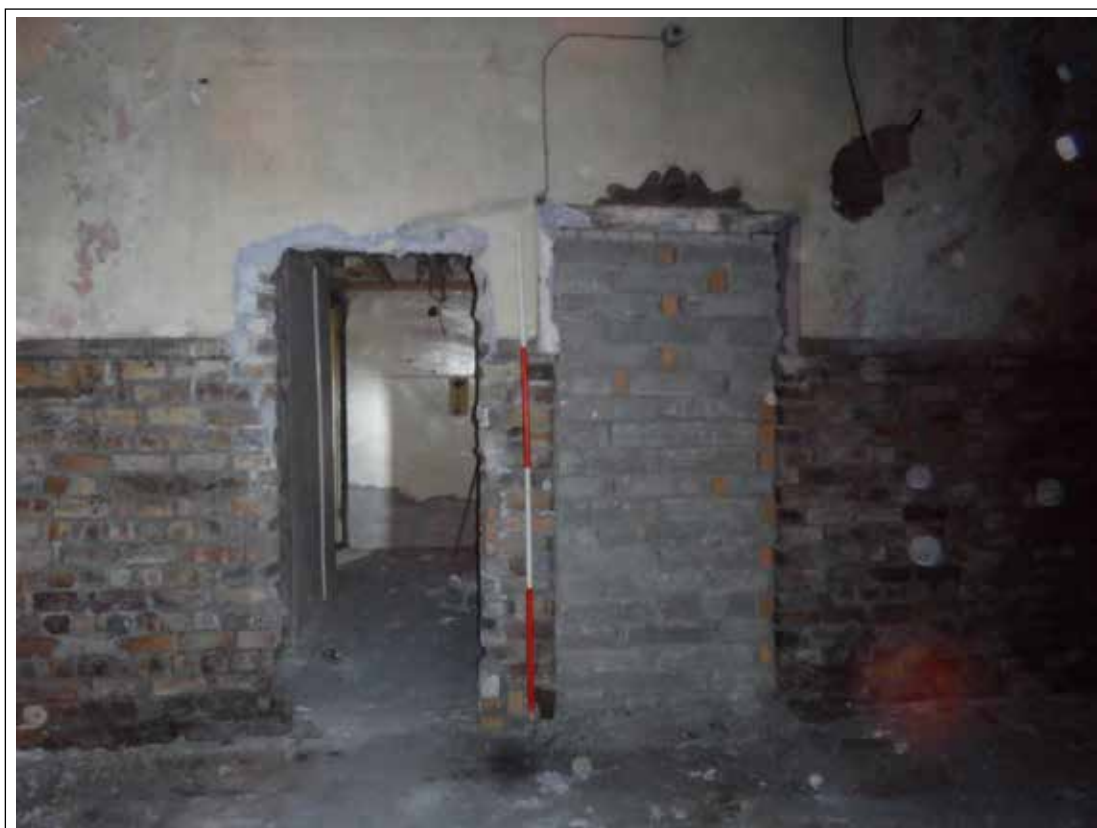
Plate 54. Corridor from room 29. Looking NE. Scale 2m
