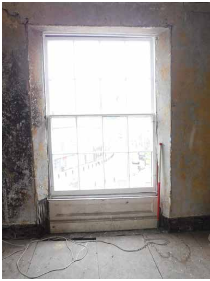
Plate 97. Window room 10. Looking NE. Scale 1m
