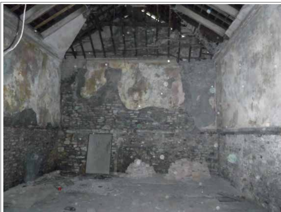
Plate 55. Room 30. Looking SW.
