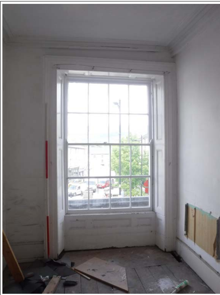
Plate 34. Window room 24. Looking NE. Scale 2m
