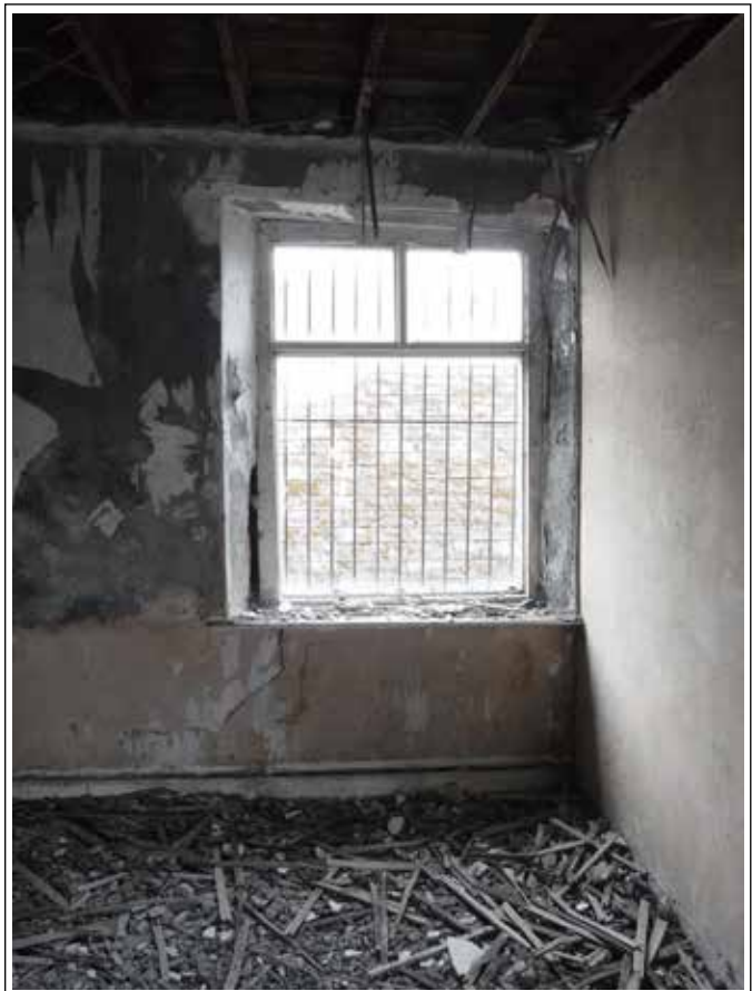
Plate 66. Room 3. Looking SW.
