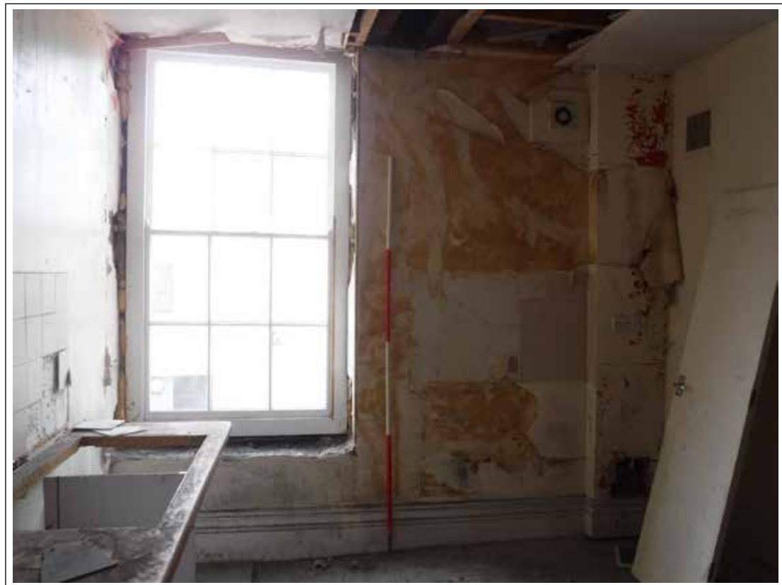
Plate 40. Room 26. Looking NW. Scale 2m
