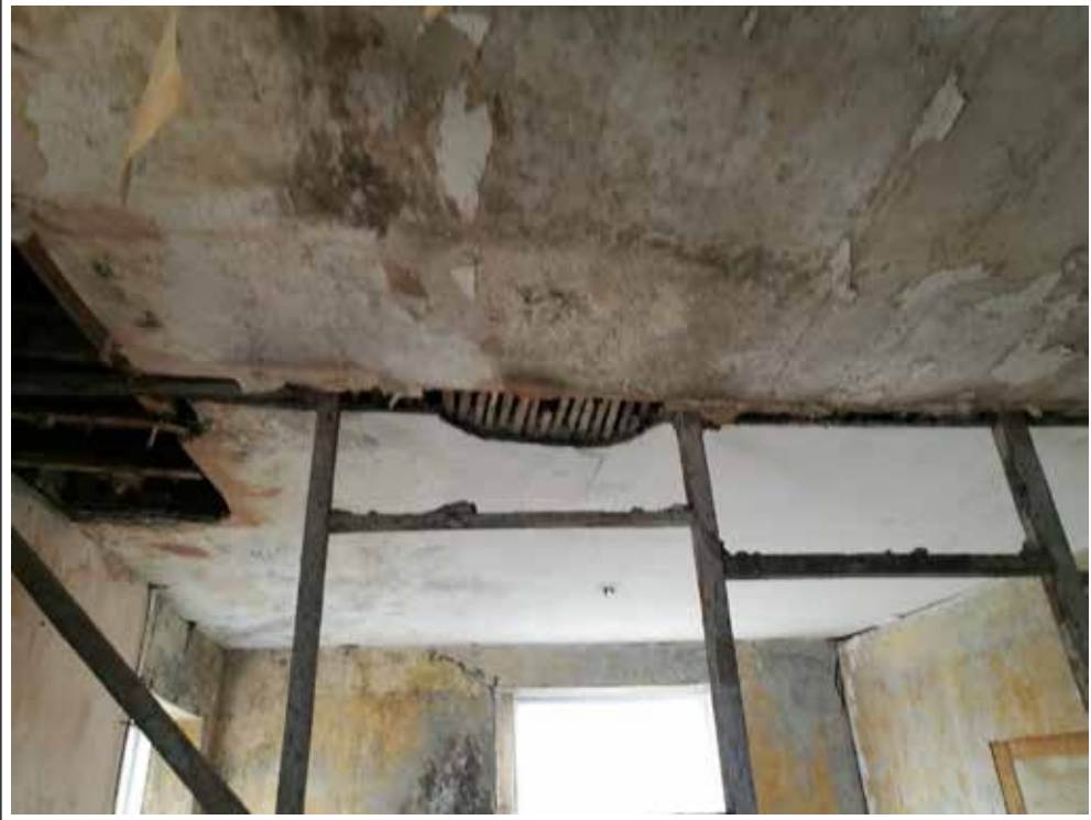
Plate 103. Ceiling room 10 into room 11. Looking NE.
