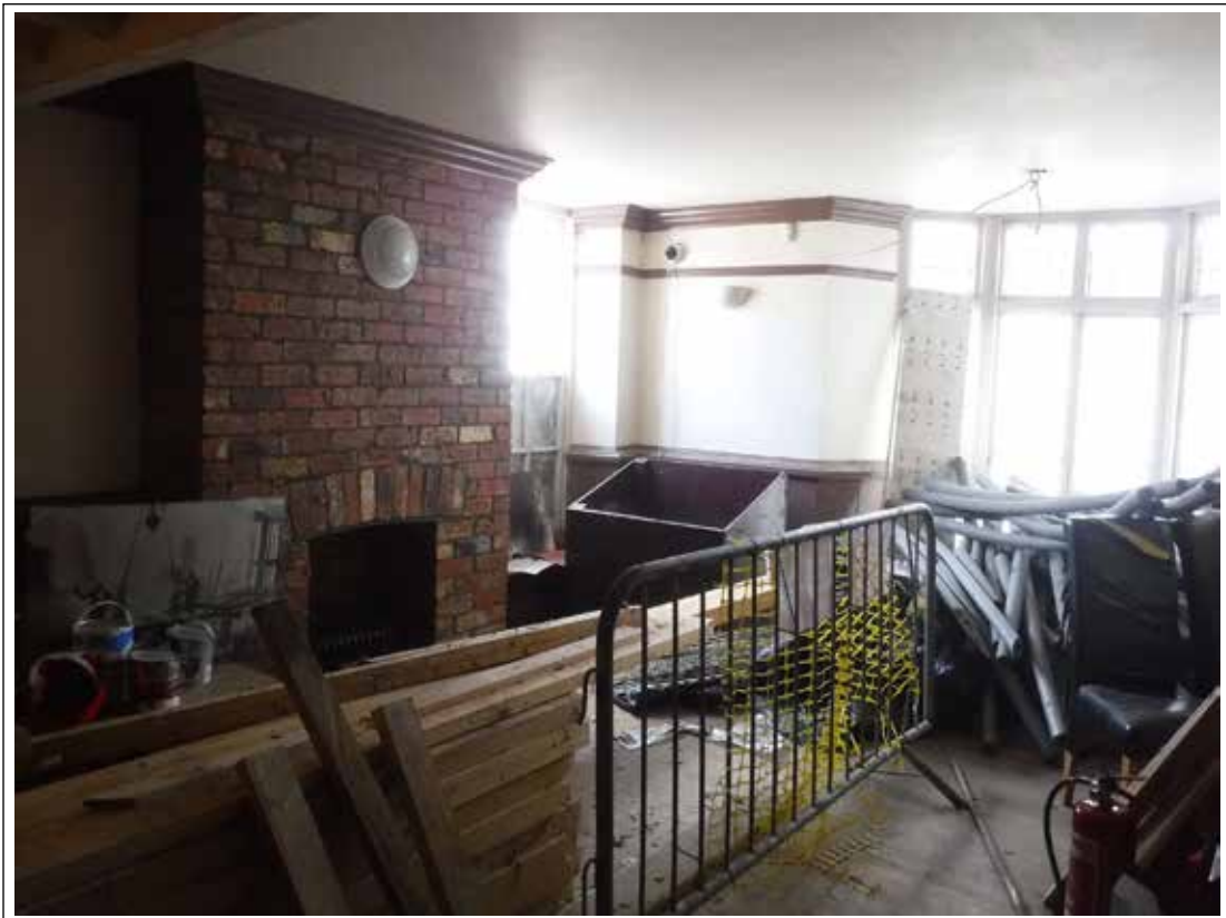
Plate 10. Internal room 12. Looking N.
