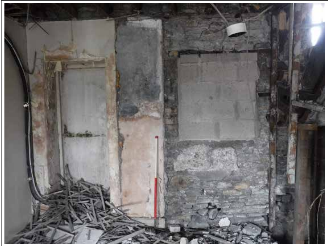
Plate 73. Room 5. Looking SW. Scale 1m
