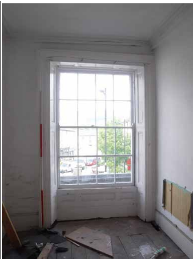
Plate 34. Window room 24. Looking NE. Scale 2m
