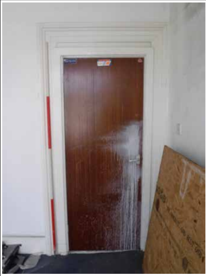
Plate 35. Room 24. Looking SW. Scale 2m
