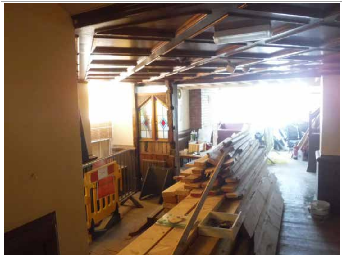
Plate 12. Internal room 12. Looking N.
