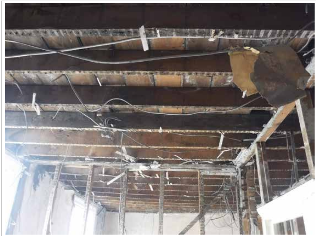
Plate 78. Ceiling room 6 into room 4 . Looking SE.
