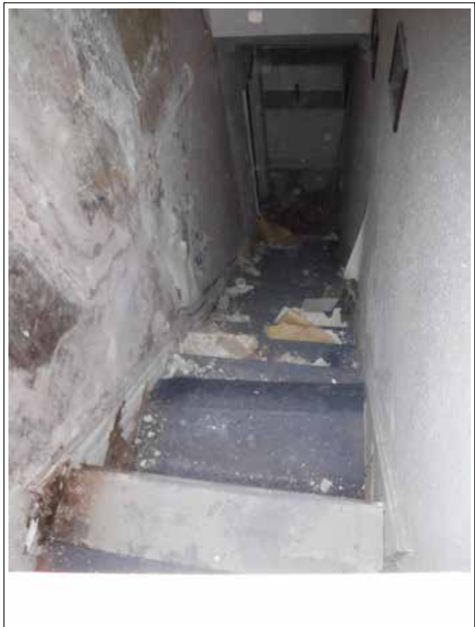
Plate 60. Staircase. Looking NW.
