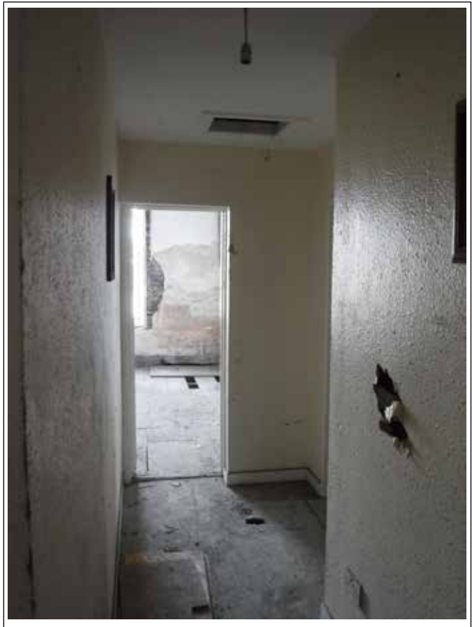
Plate 46. Corridor. Looking NE
