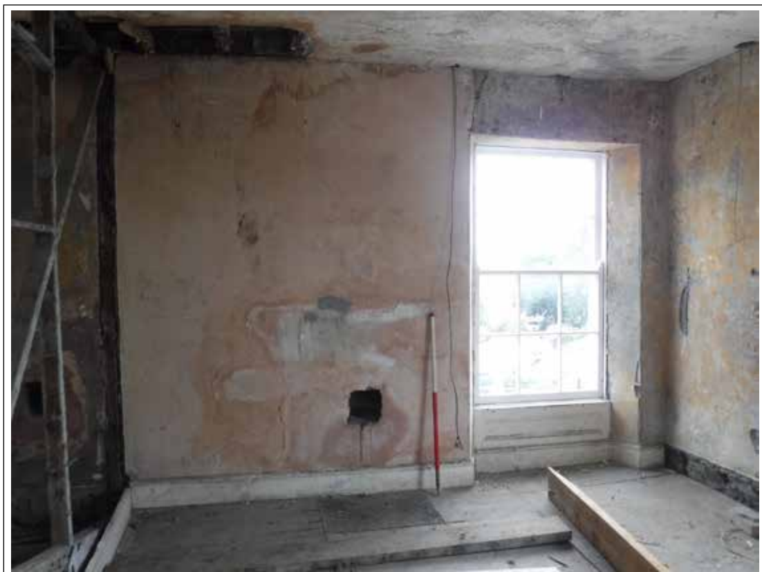
Plate 96. Room 10. Looking N. Scale 1m
