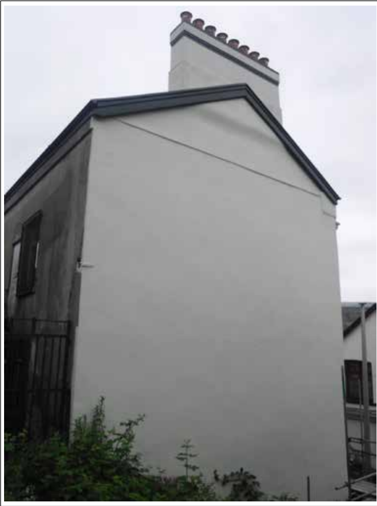
Plate 3. Side elevation. Looking N.
