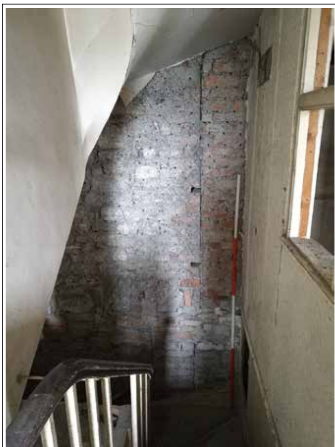
Plate 105. Staircase to first floor. Looking SW. Scale 2m
