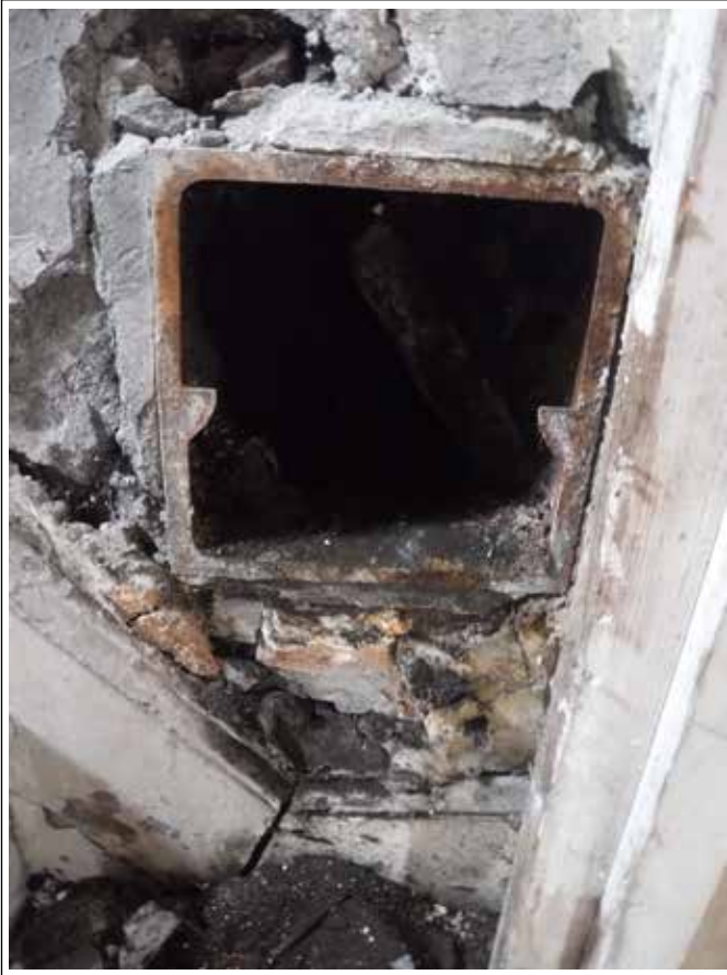
Plate 81. Near staircase room 5.
