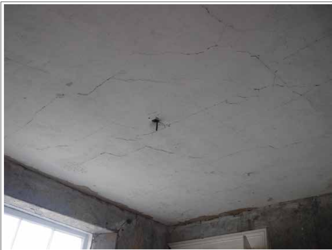
Plate 92. Ceiling room 8 similar in room 9.
