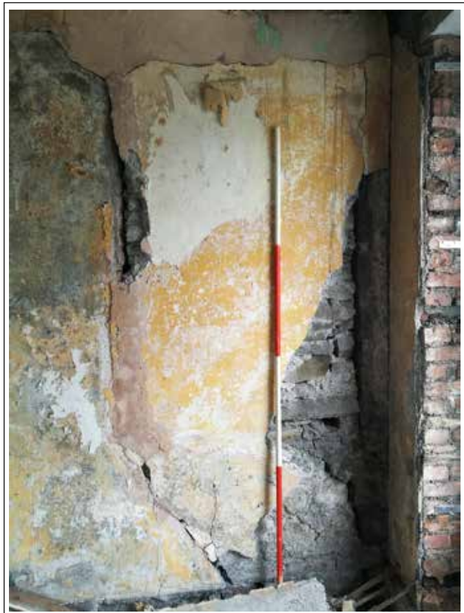
Plate 102. Room 11. Looking SW. Scale 2m
