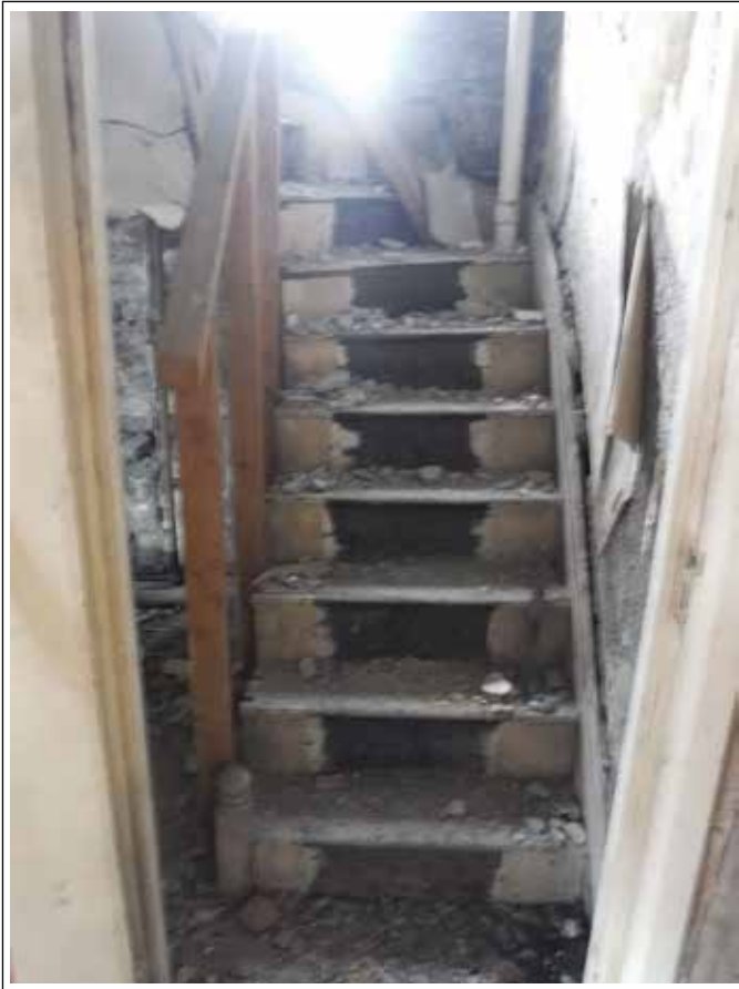
Plate 65. Staircase. Looking SW.
