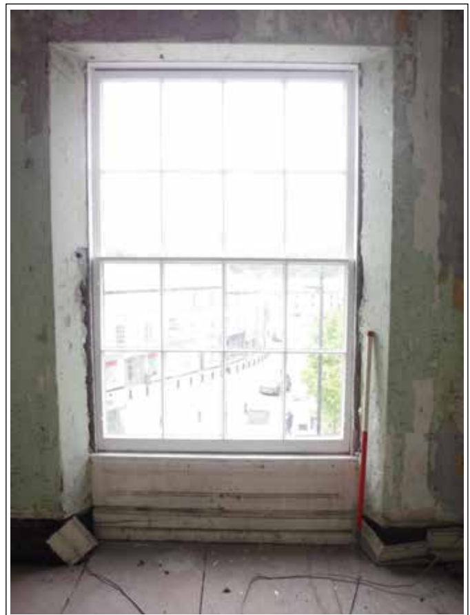
Plate 94. Window room 9. Looking NE. Scale 1m
