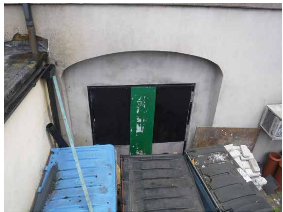
Plate 30. External back BL. Looking SE.
