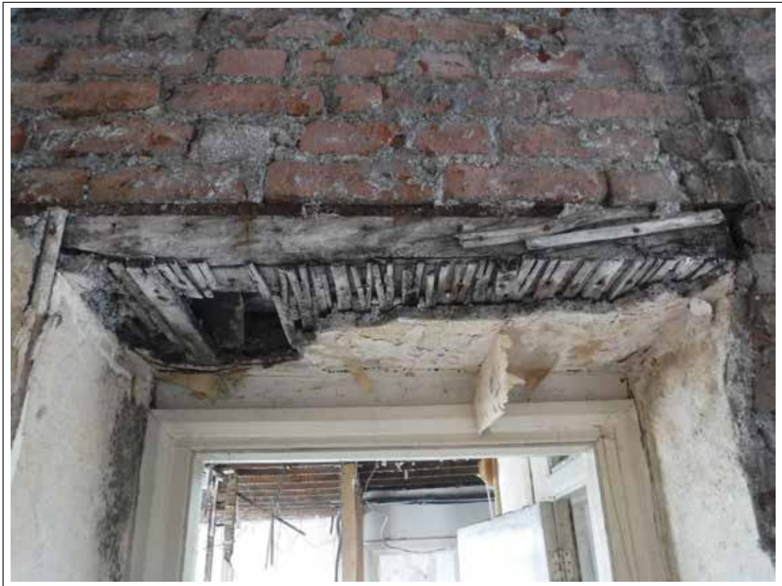
Plate 84. Above doorway room 7. Looking SE.
