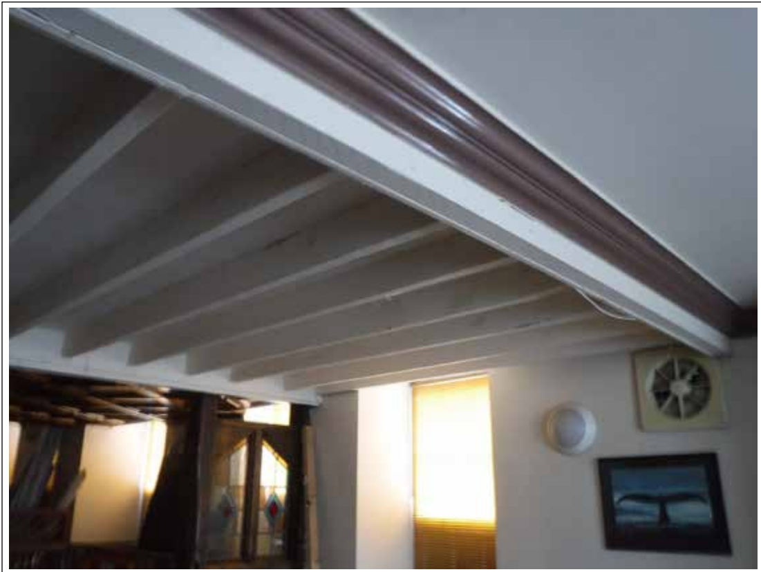
Plate 11. Internal room 12. Looking W.
