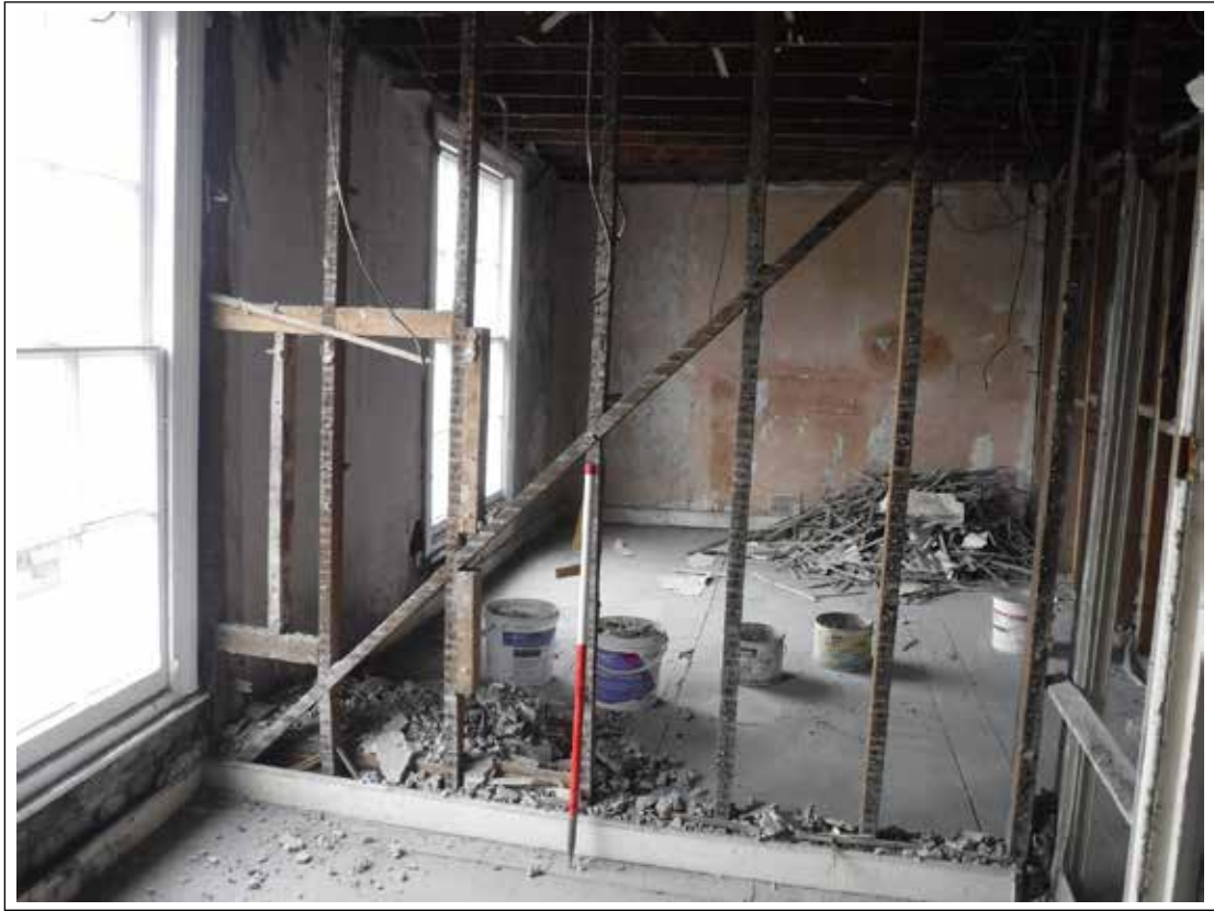
Plate 77. Room 6 into room 4. Looking SE. Scale 1m
