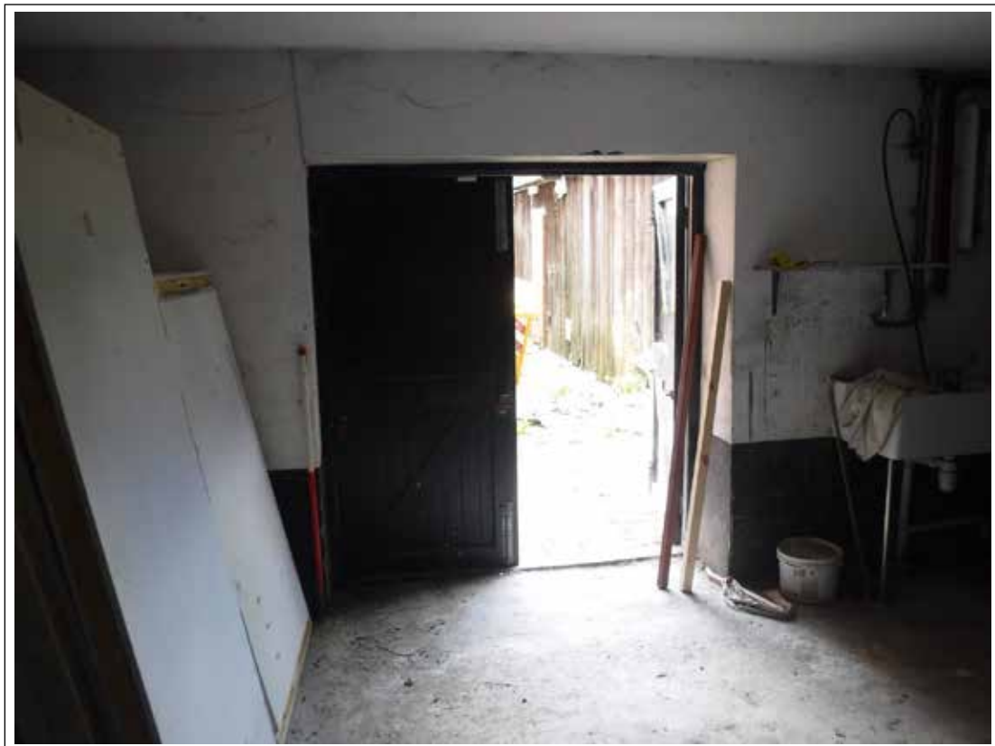
Plate 22. Room 21. Looking N. Scale 1m
