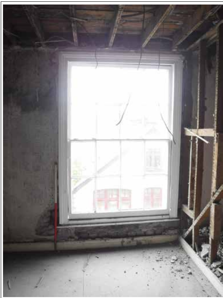
Plate 76. Window room 6. Looking NE. Scale 1m
