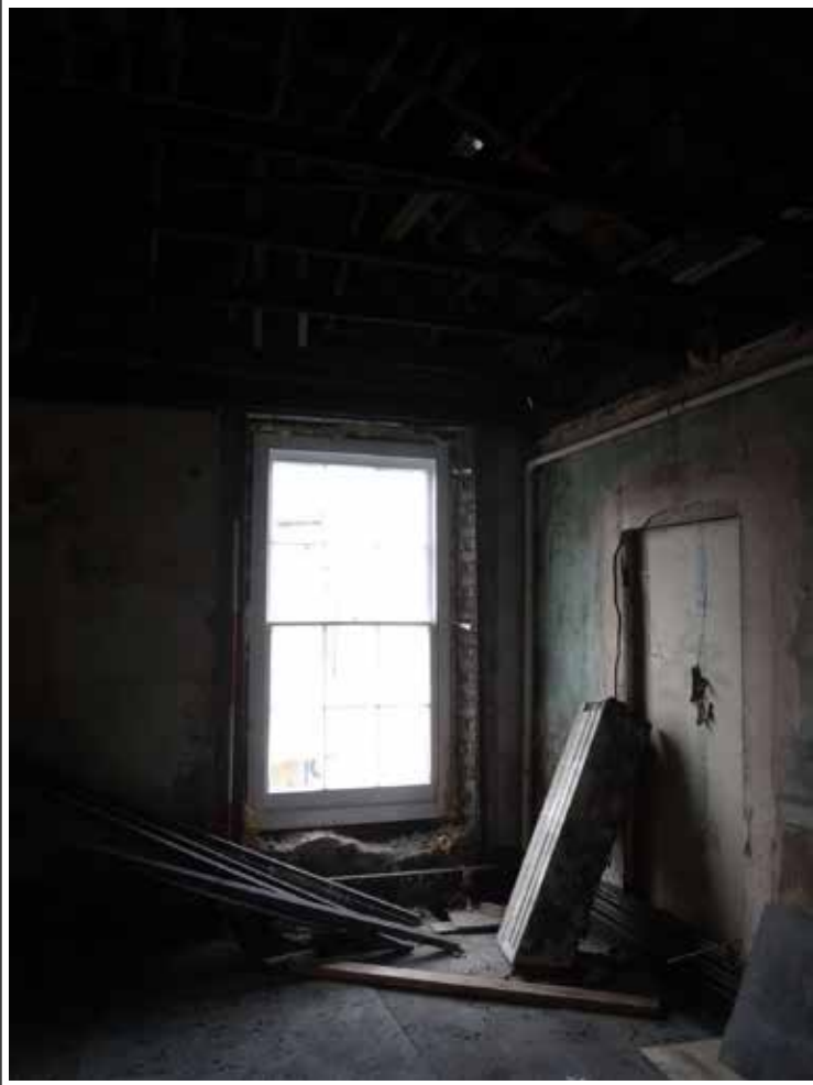
Plate 49. Room 29. Looking NW.
