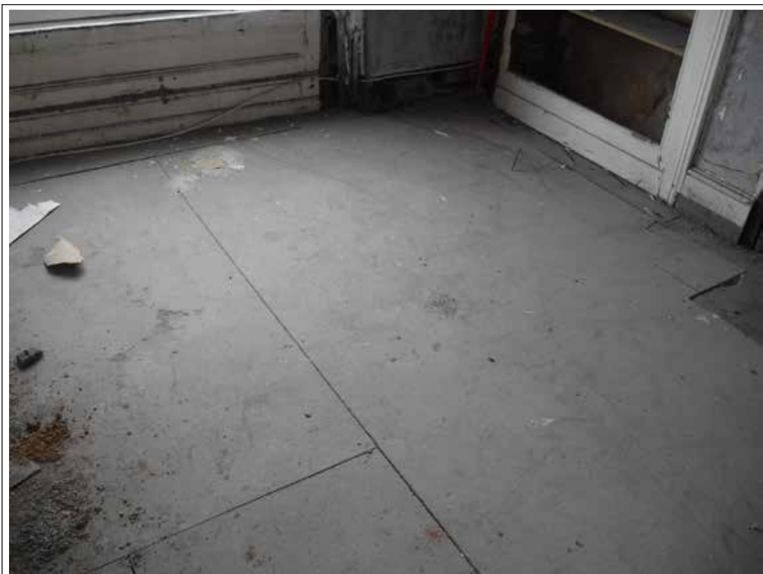
Plate 91. Floor room 8, similar in room 9.
