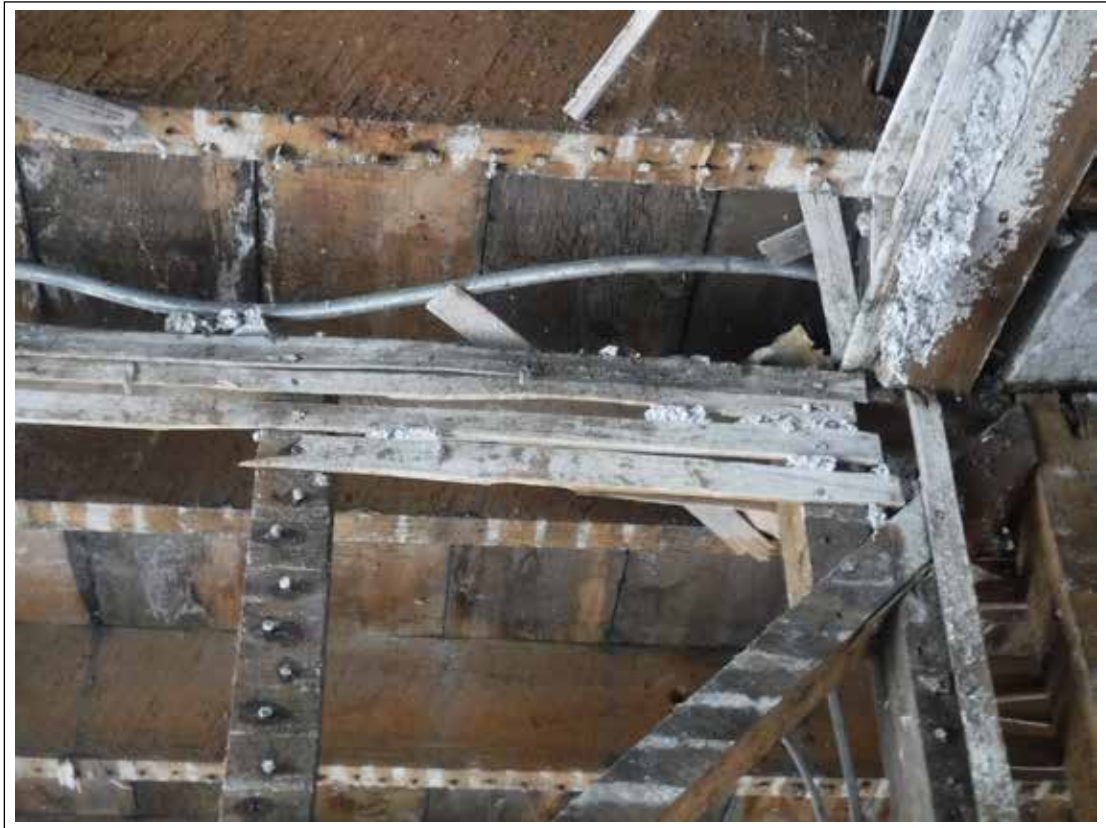
Plate 79. Room 6 into room 4. Looking SE. Scale 1m
