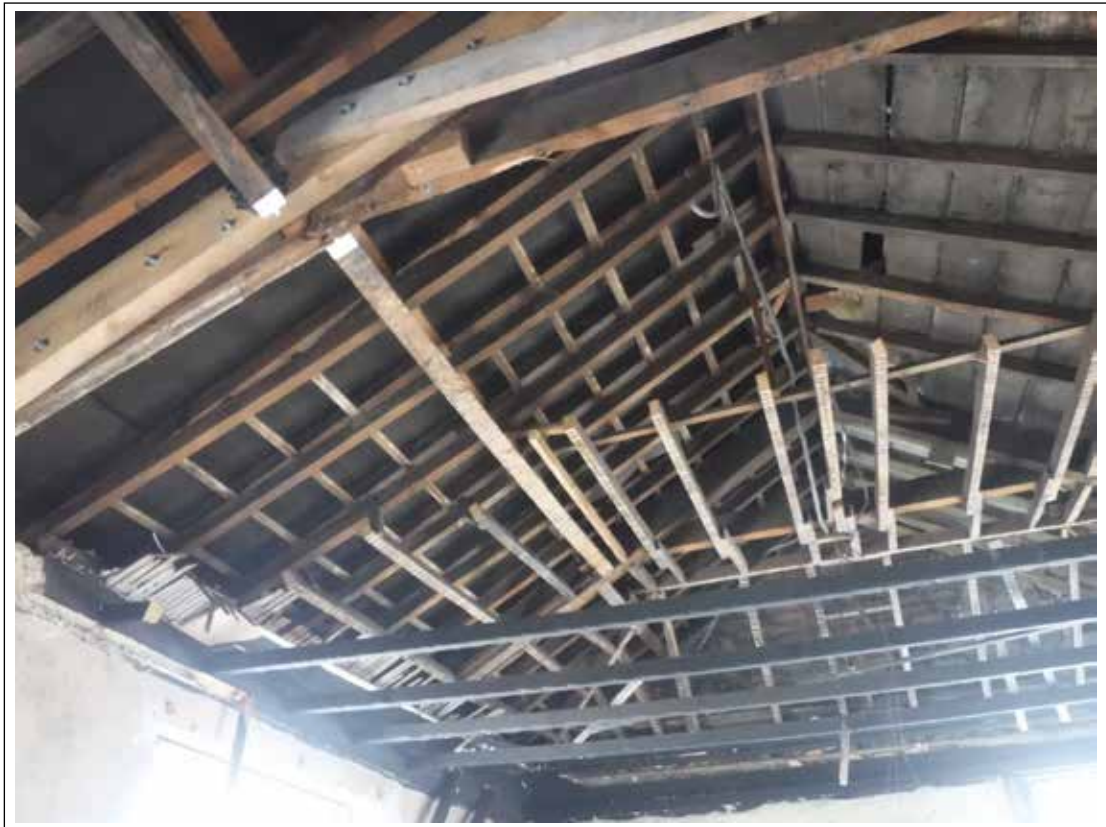
Plate 48. Ceiling room 29. Looking NW.
