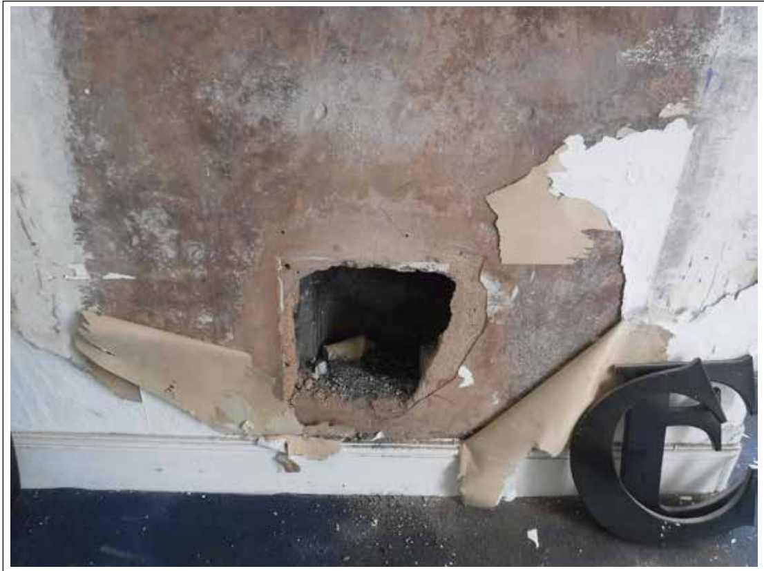
Plate 39. Room 25. Looking NW.
