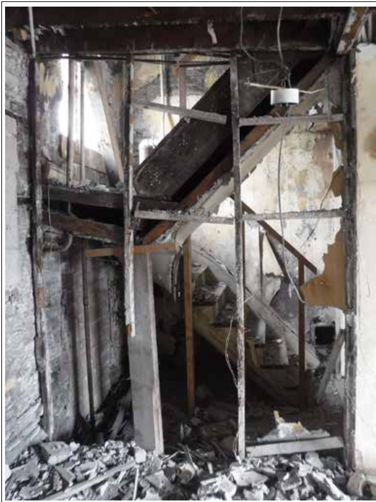
Plate 74. Room 5. Looking NW.
