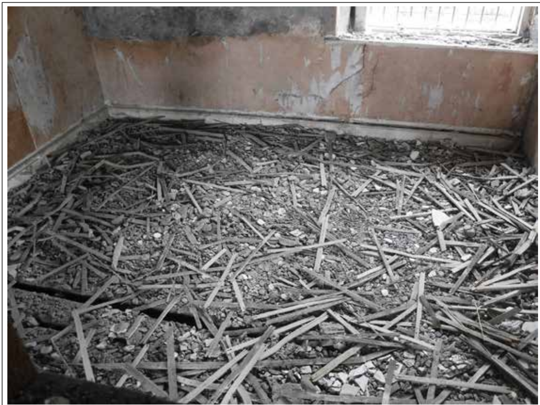
Plate 68. Floor room 3. Looking S.
