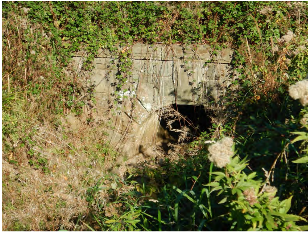
Plate 37. By-wash channel outlet culvert, looking north-west.
