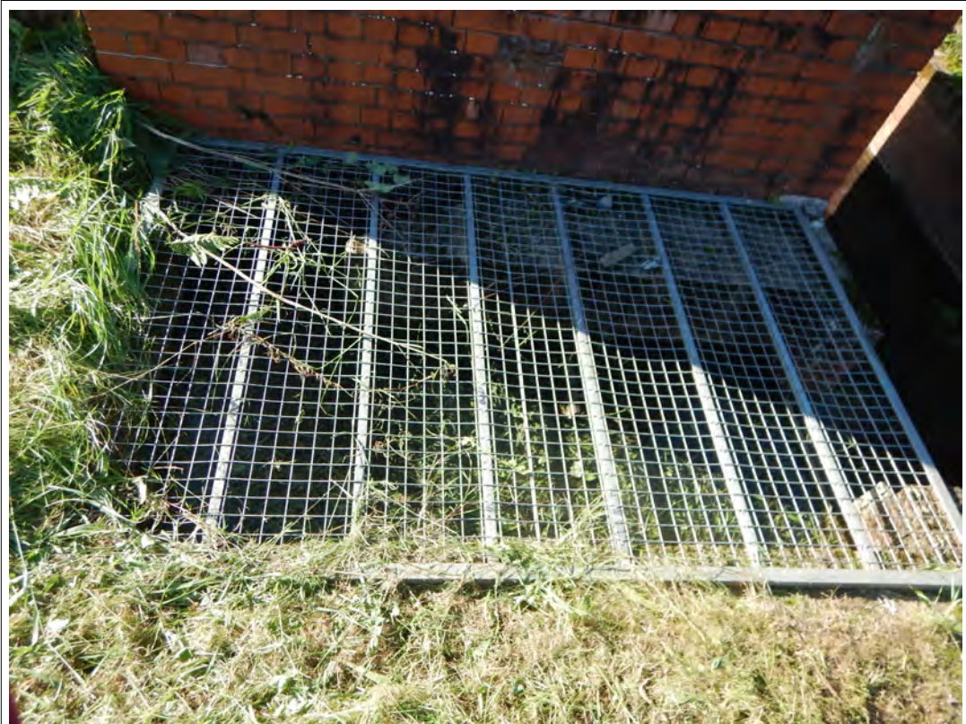
Plate 62. Tank to the north-east of the Gauging Station building.
