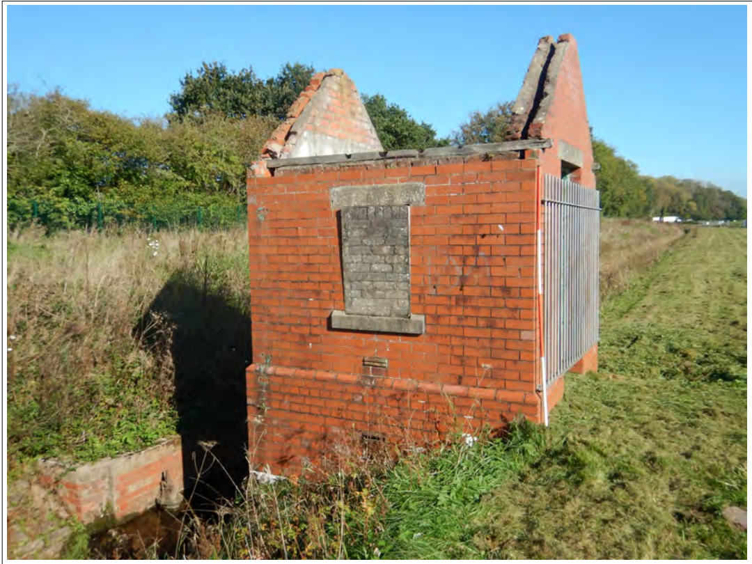
Plate 55. The Gauging Station building, looking north. Scale 2m
