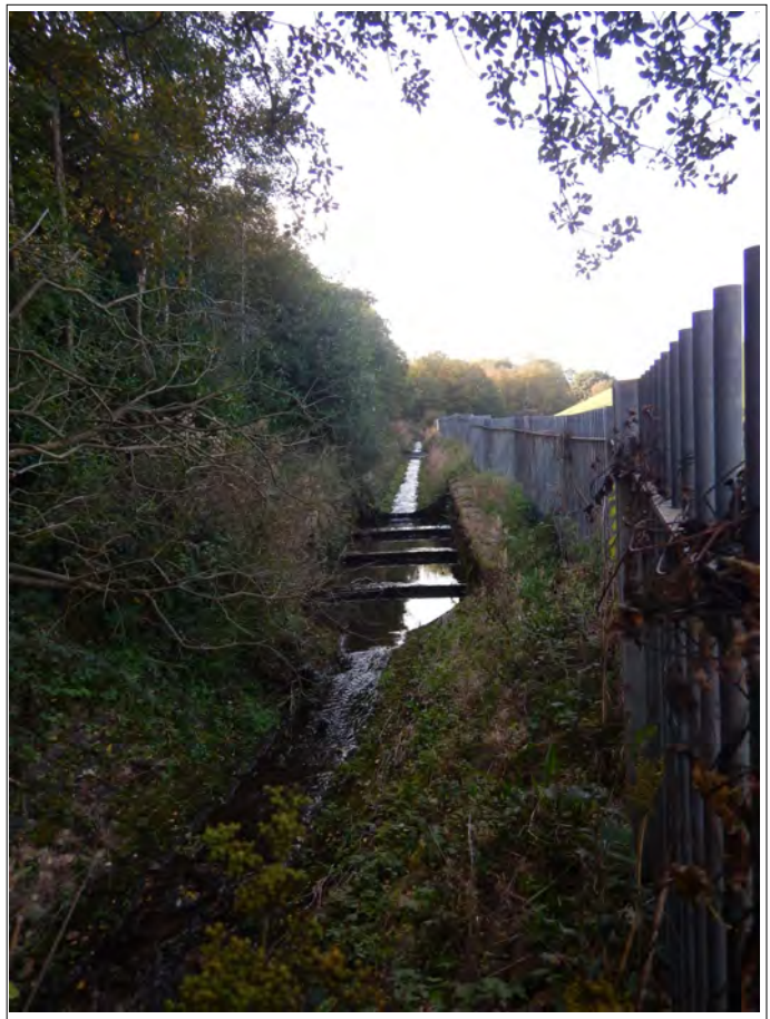
Plate 30. View looking west along the stepped weir.
