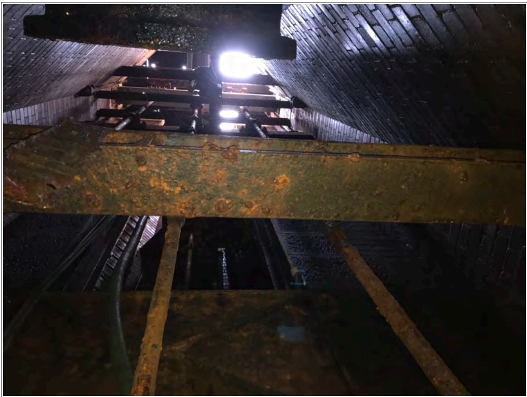
Plate 18. Interior of the valve shaft, looking upwards.
