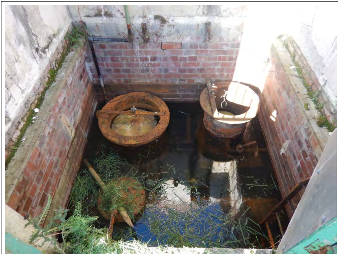
Plate 60. Interior of the Gauging Station building.
