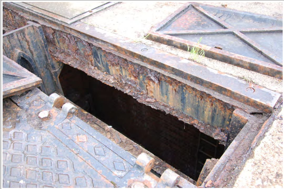
Plate 49. Wrought iron access hatches to the screening chamber.
