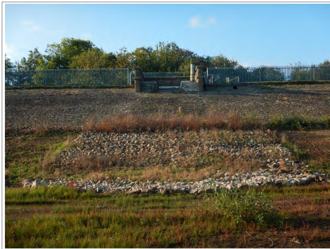
Plate 40. Cipoletti Weir, taken from the interior of the reservoir, looking west.
