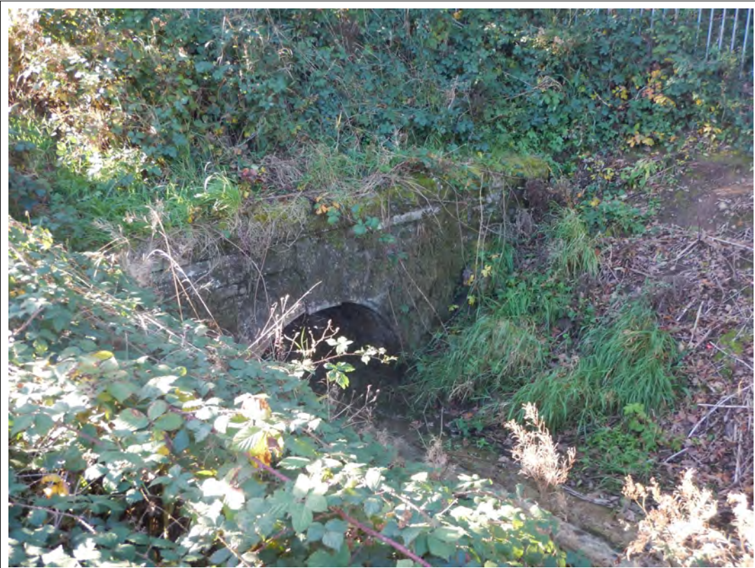
Plate 38. By-wash channel inlet culvert, looking south-west.
