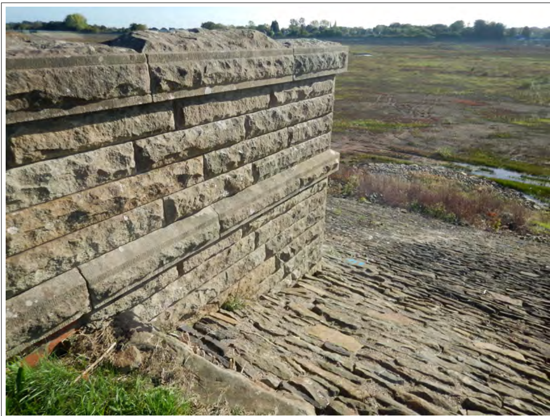
Plate 41. Southern exterior wall of the Cipoletti Weir, looking east.
