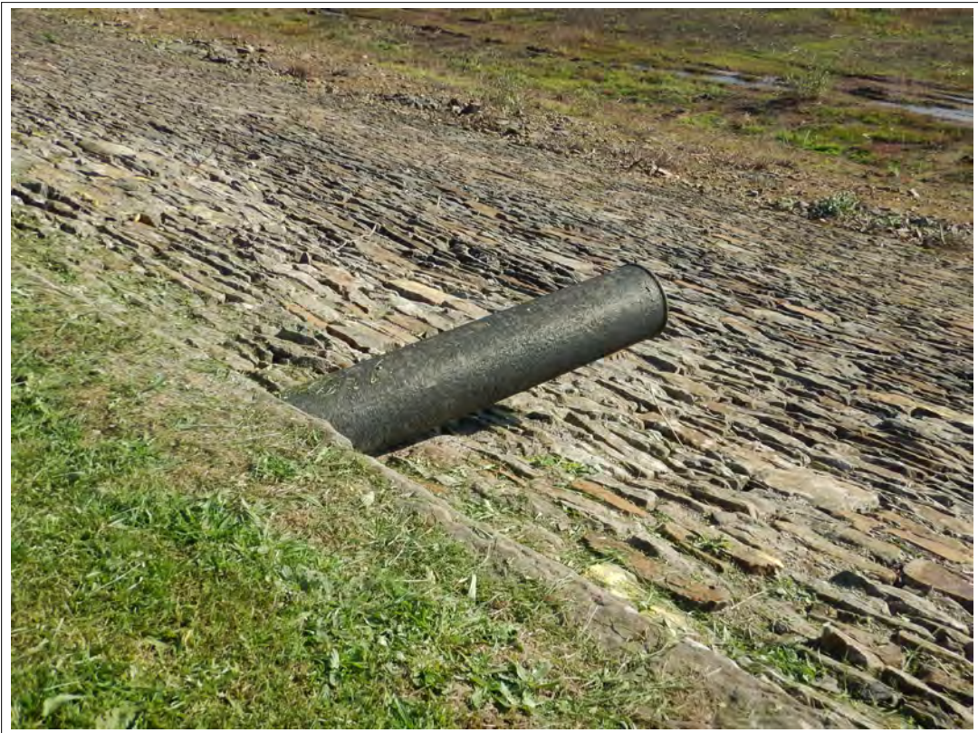
Plate 11. Outlet pipe on the western bank of the reservoir, looking north-east.
