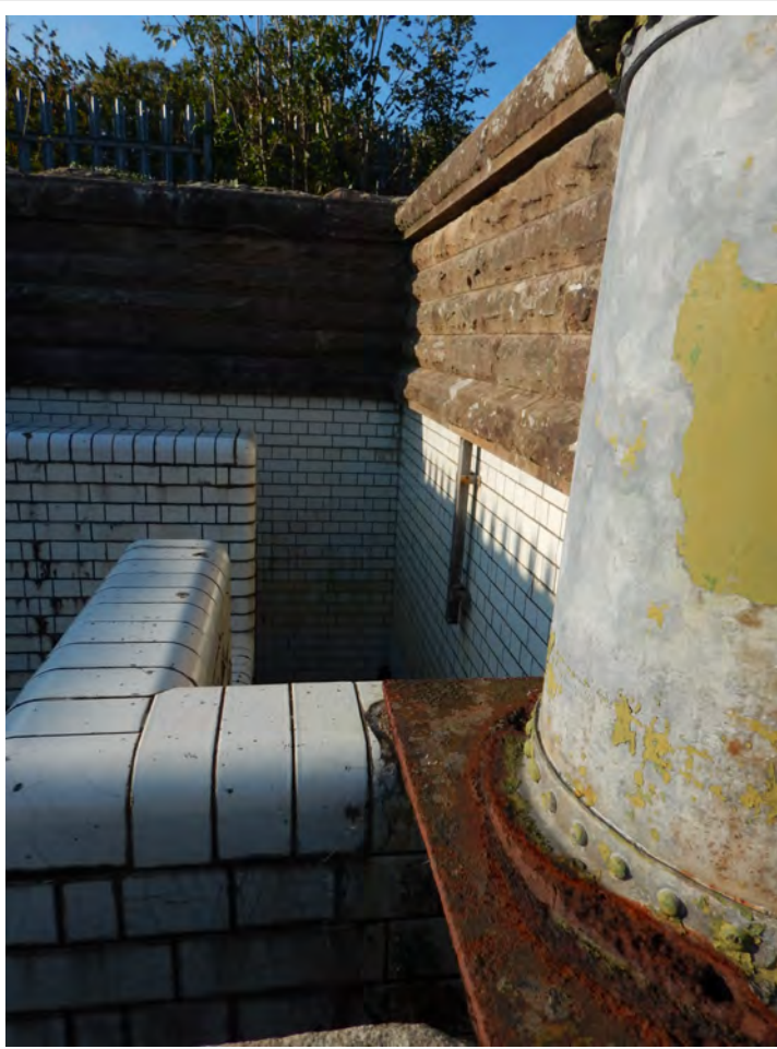
Plate 45. Interior of the Cipoletti Weir showing the side chamber, looking west.
