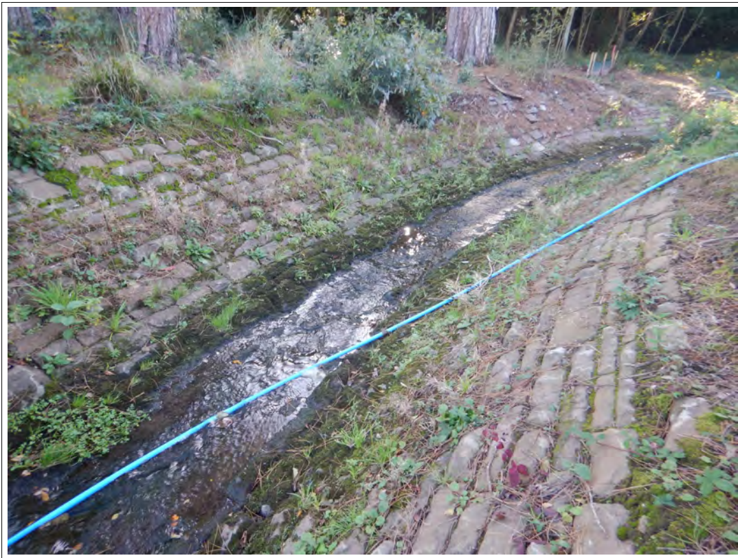
Plate 36. Southern part of the by-wash channel, looking south.
