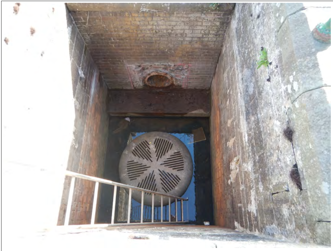
Plate 69. Interior chamber of the Inlet Gauge Chamber.
