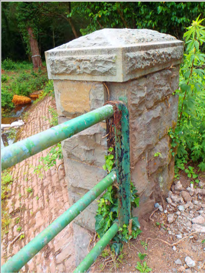
Plate 29. The south-eastern pillar of the 'SEMD' bridge, looking south-east.
