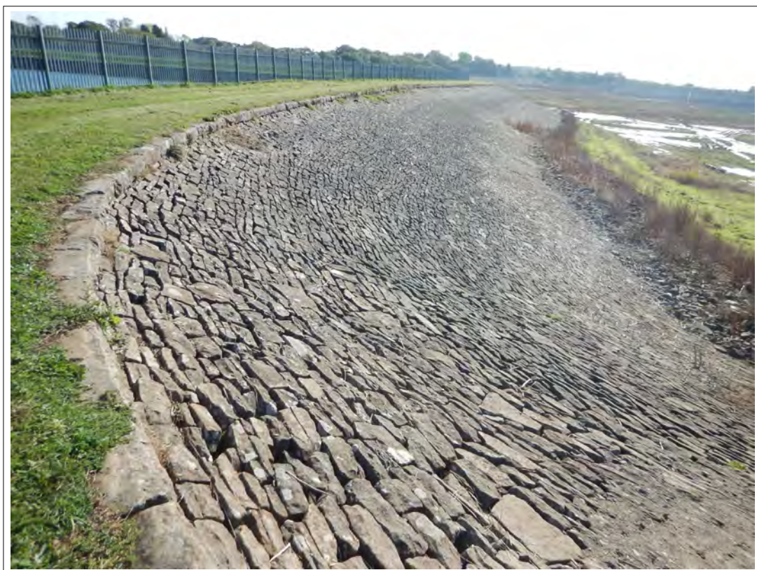
Plate 4. Interior of the northern bank of the reservoir, looking south-east.
