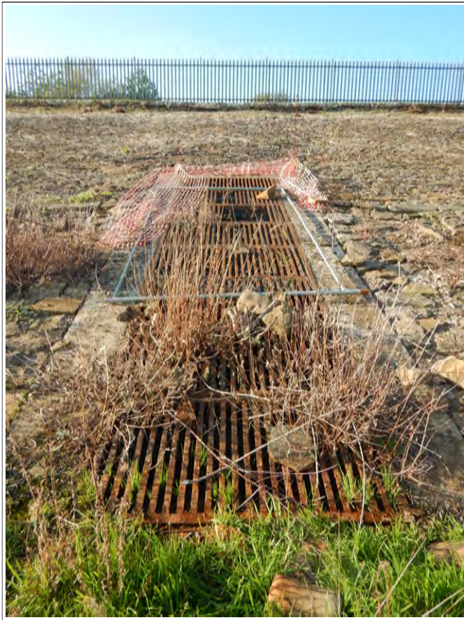
Plate 65. Outlet situated on west bank of the reservoir, looking west.
