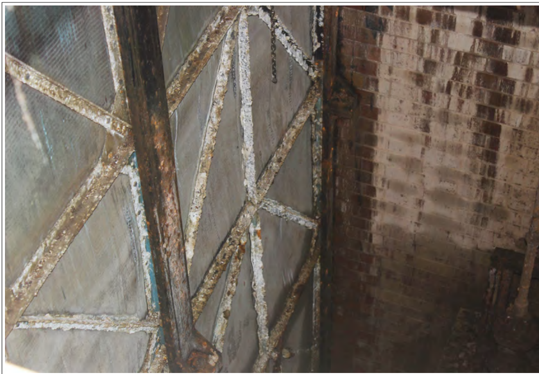
Plate 52. Interior of the screening chamber, showing the screen.
