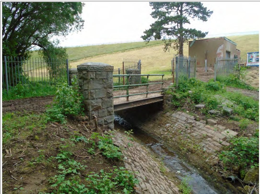
Plate 26. The 'SEMD' bridge, looking north-west.
