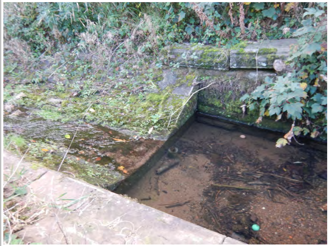
Plate 33. Detail of the stepped weir showing outflow into the by-wash channel.
