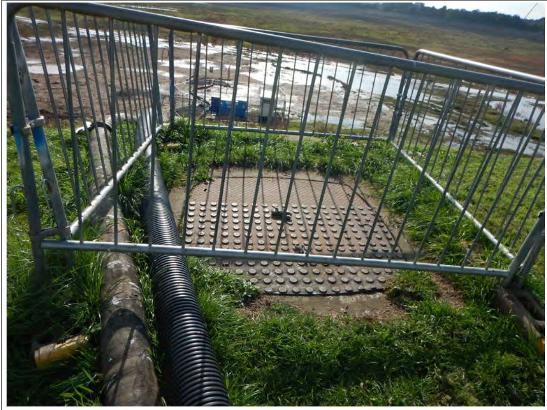
Plate 75. Isolated Valve Chamber on the northern bank of the reservoir.
