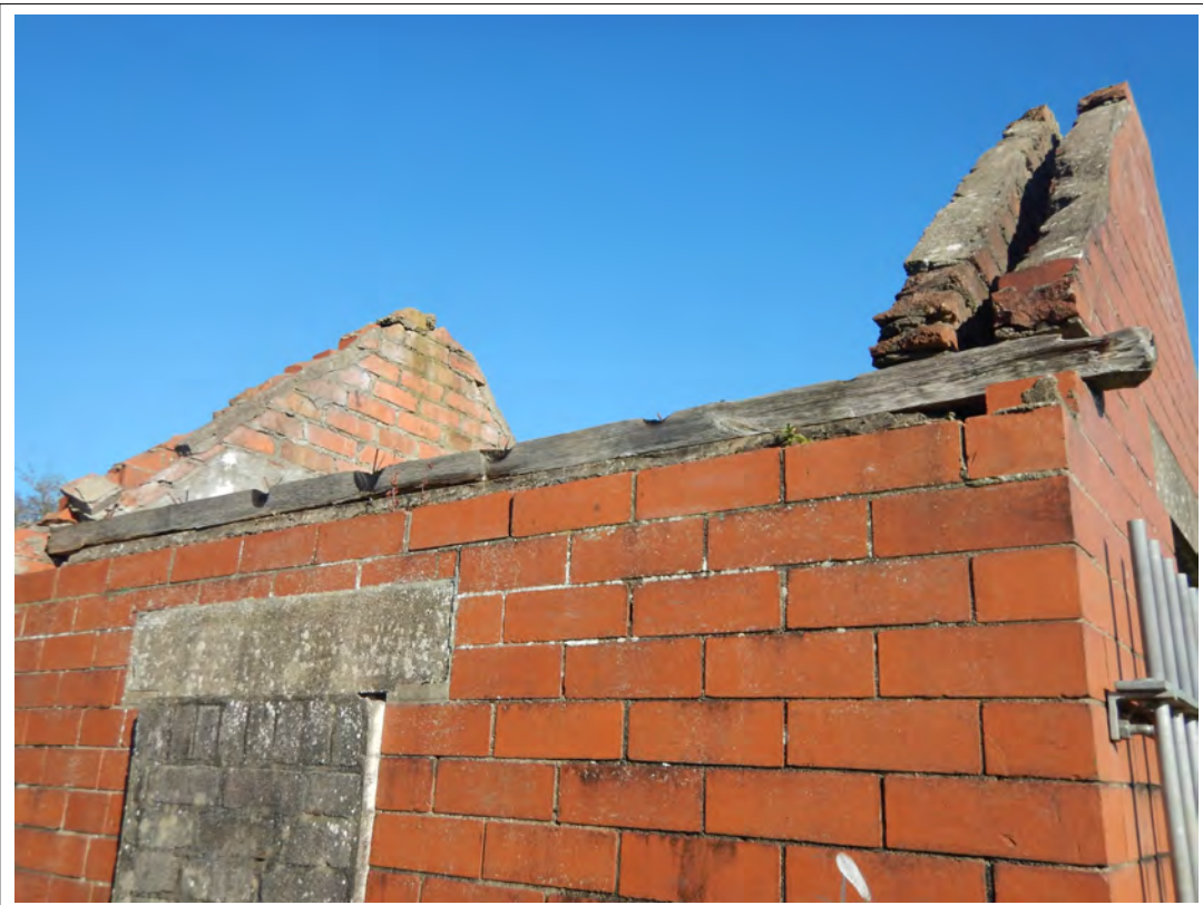
Plate 56. Detail of the Gauging Station walls.
