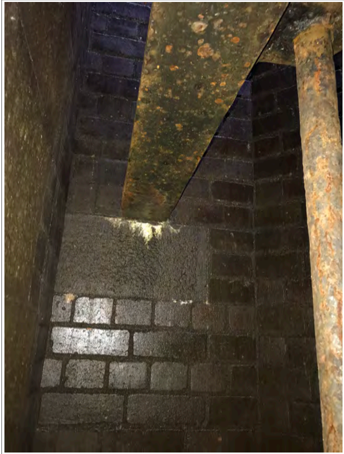
Plate 19. Original girder within the valve shaft, showing the supporting stone block.
