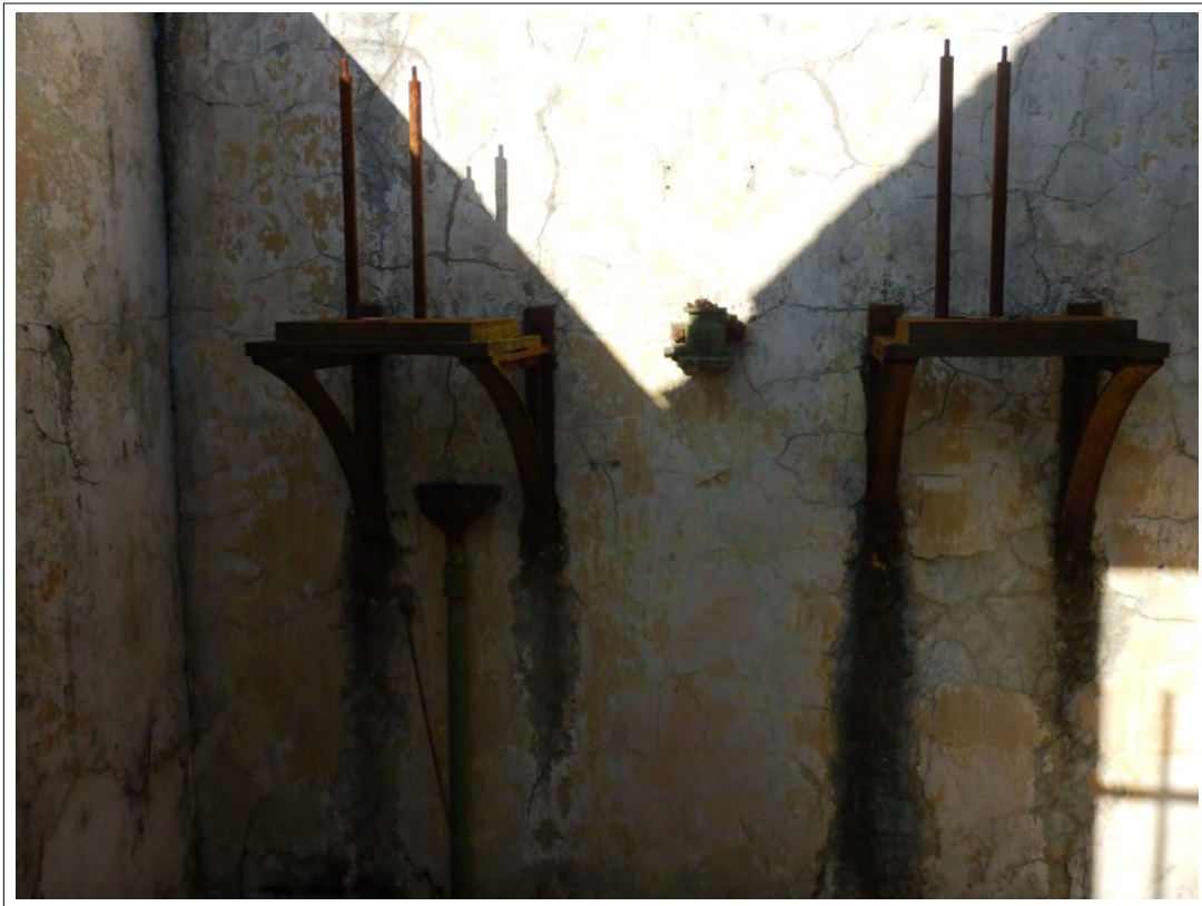
Plate 61. Gauging Station building showing brackets for the water meter.
