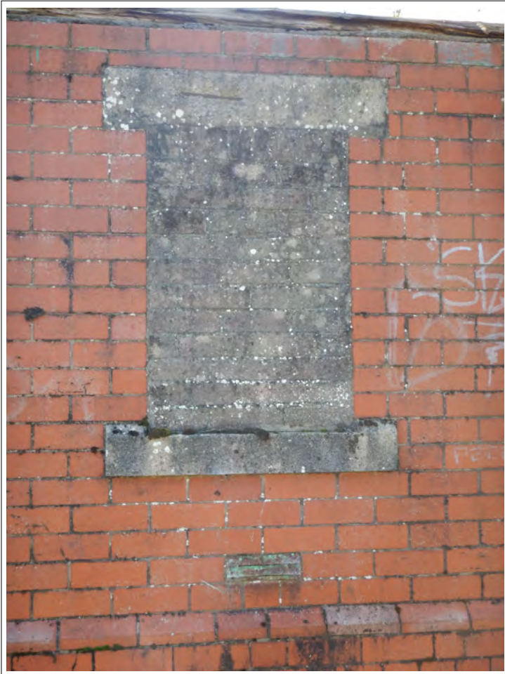
Plate 59. Blocked-up window on the north-east elevation of the Gauging Station building.
