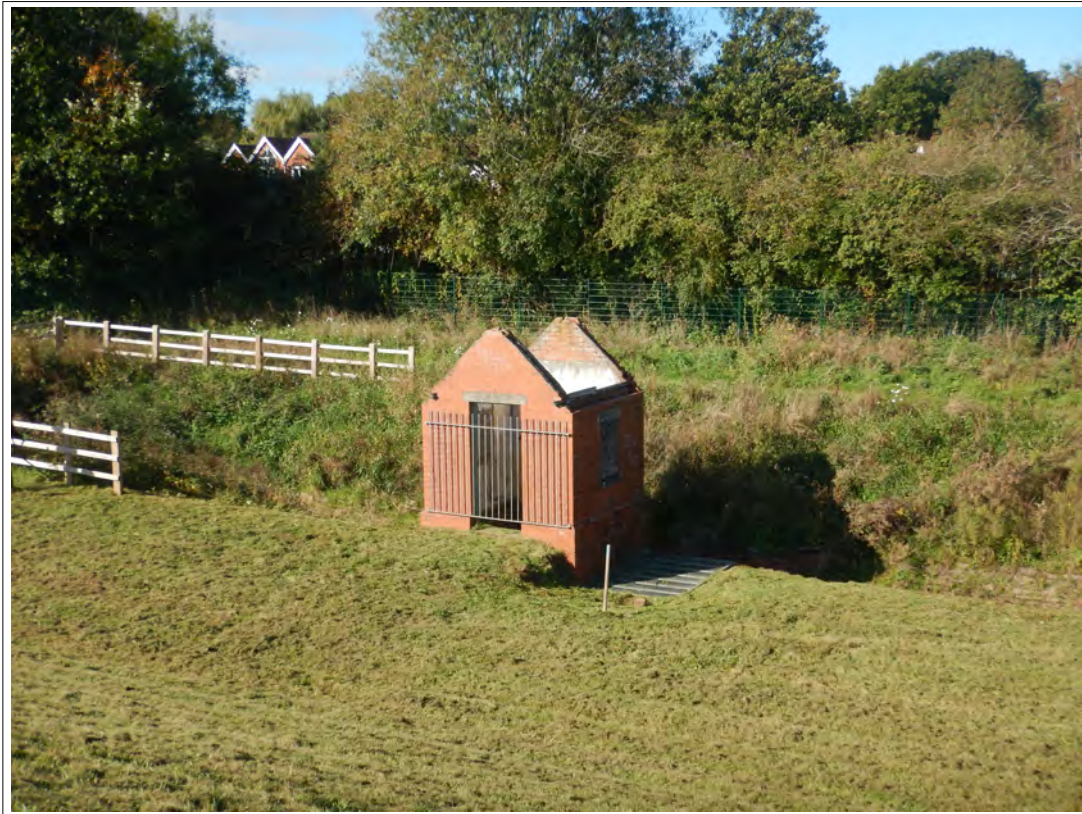
Plate 57. The Gauging Station building, looking south-west.
