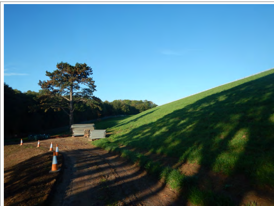
Plate 2. Exterior of the southern reservoir bank, looking west.
