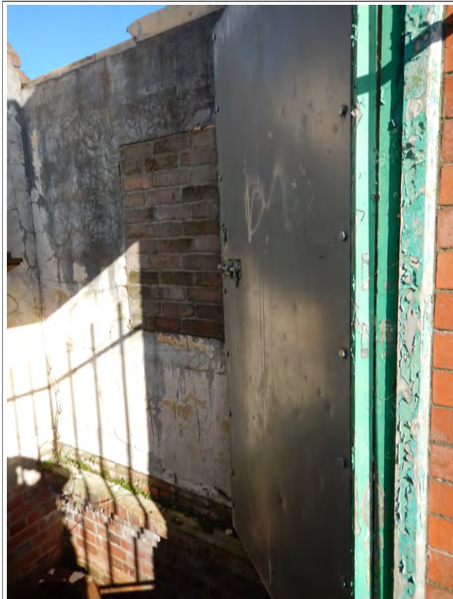
Plate 58. Door and interior wall of Gauging Station building.
