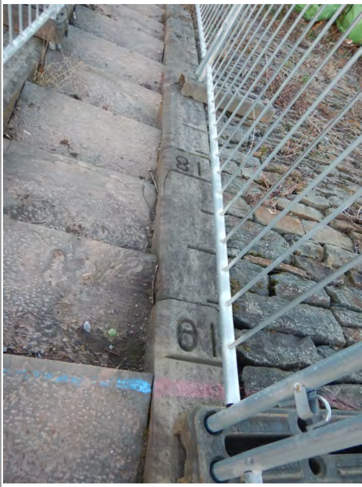
Plate 13. Depth markings on the side of the access steps.
