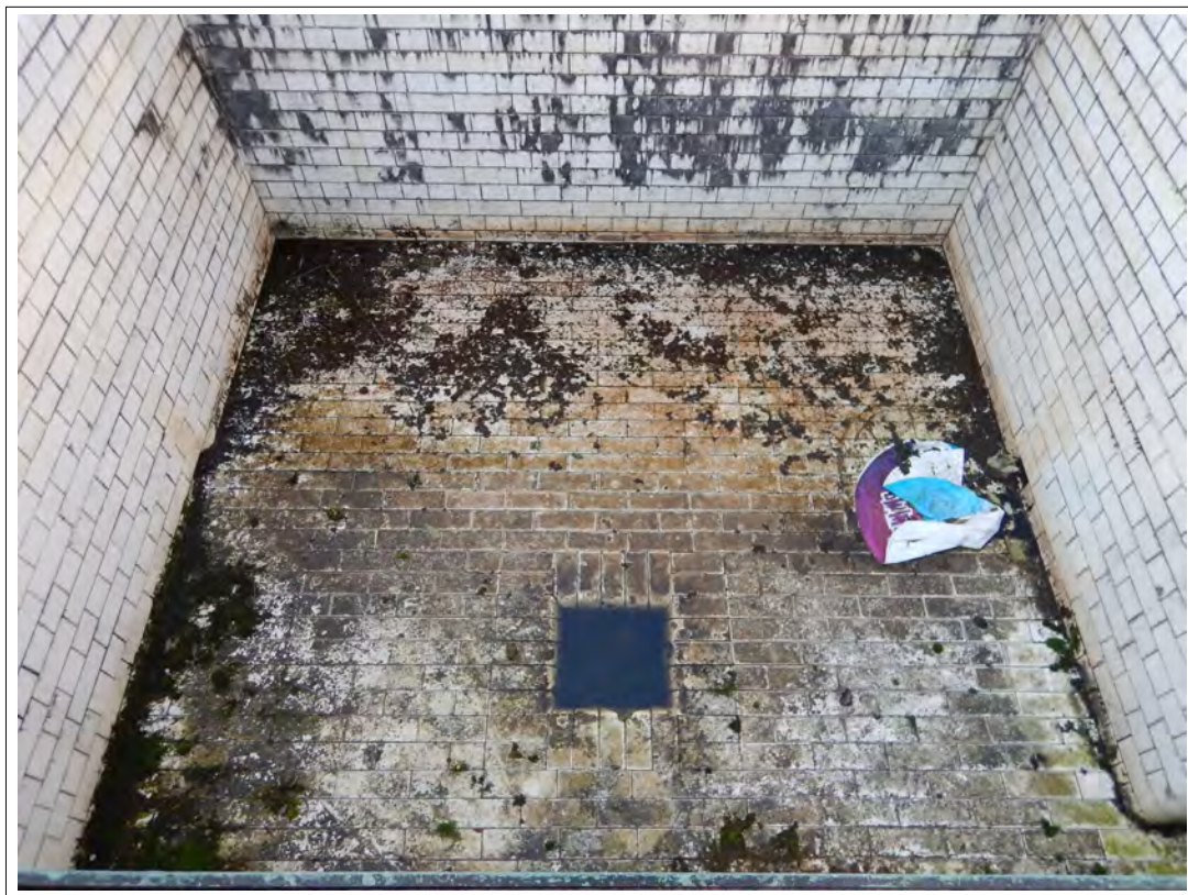
Plate 46. Interior of the Cipoletti Weir showing the central outlet.
