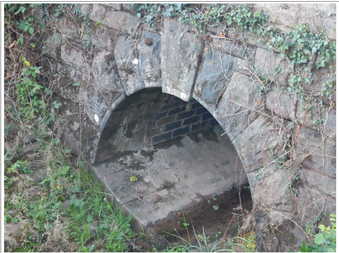
Plate 24. Detail of the scour channel culvert outlet.
