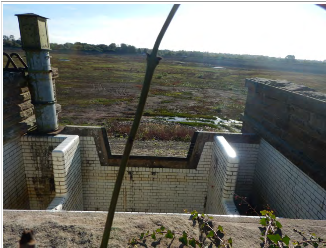
Plate 43. Interior of the Cipoletti Weir, looking east.
