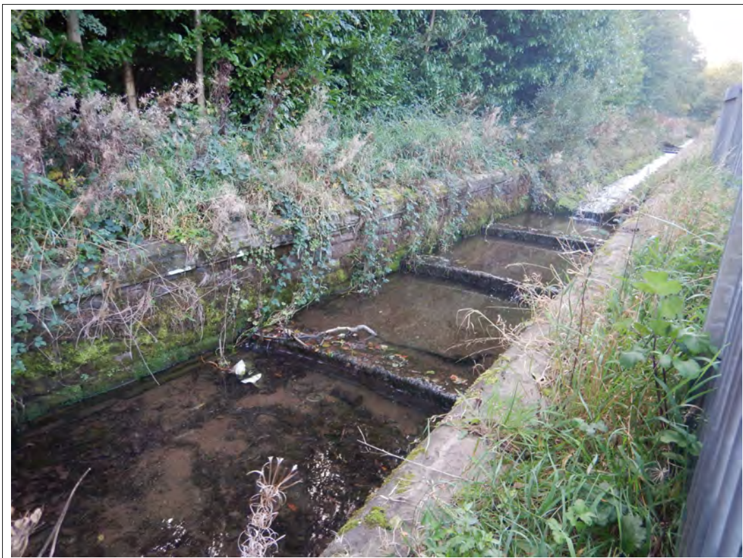
Plate 31. Lower part of the stepped weir, looking south-west.
