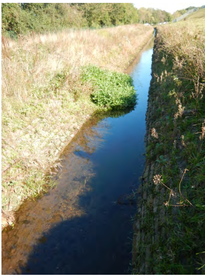
Plate 35. By-wash channel on the western side of the reservoir, looking north.
