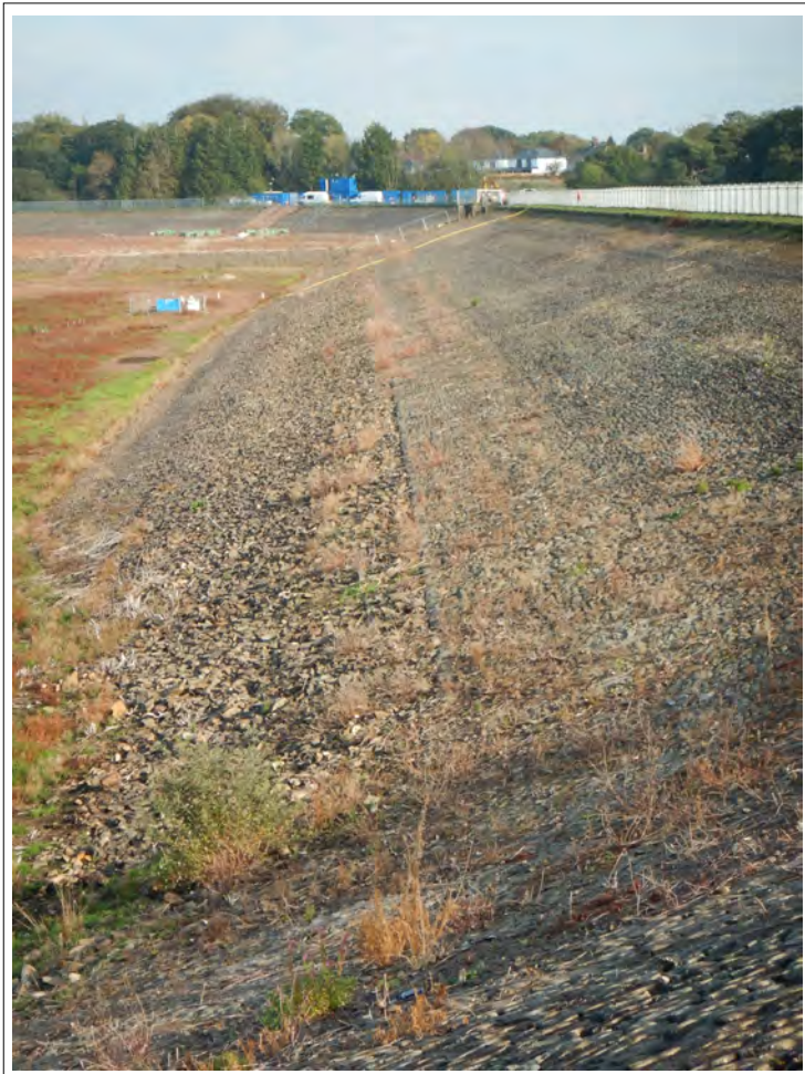
Plate 5. Interior of the southern bank of the reservoir, looking east.
