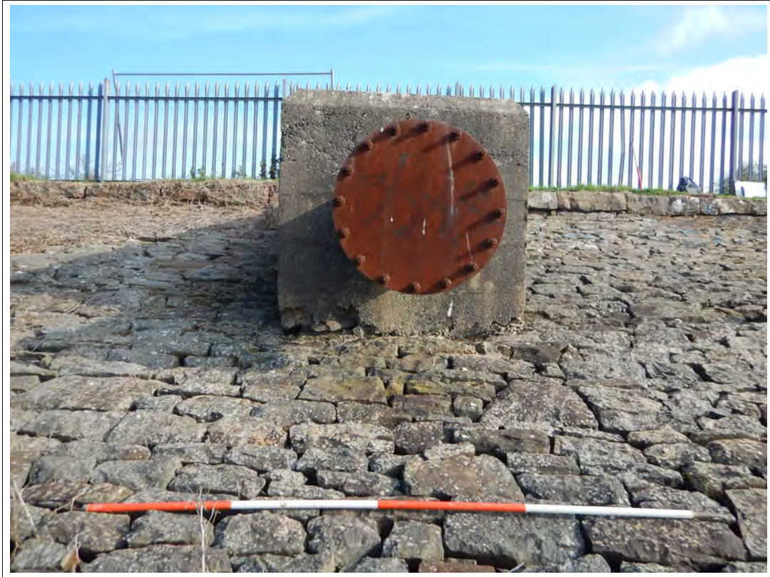
Plate 77. Pipe penetration, looking east. Scale 2m.
