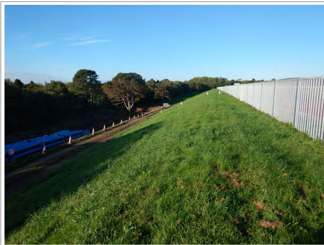
Plate 1. Exterior of the southern reservoir bank, looking west from the top of the embankment.
