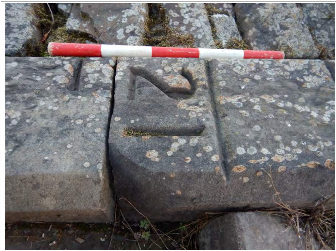
Plate 14. Detail of the depth markings on the side of the access steps. Scale 0.5m.
