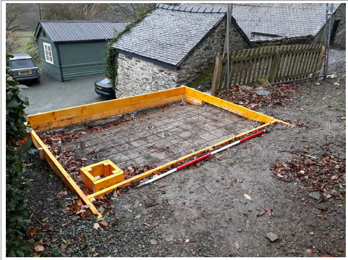
Plate 15. Base constructed at top of the retaining wall. View SW. 2m scale
