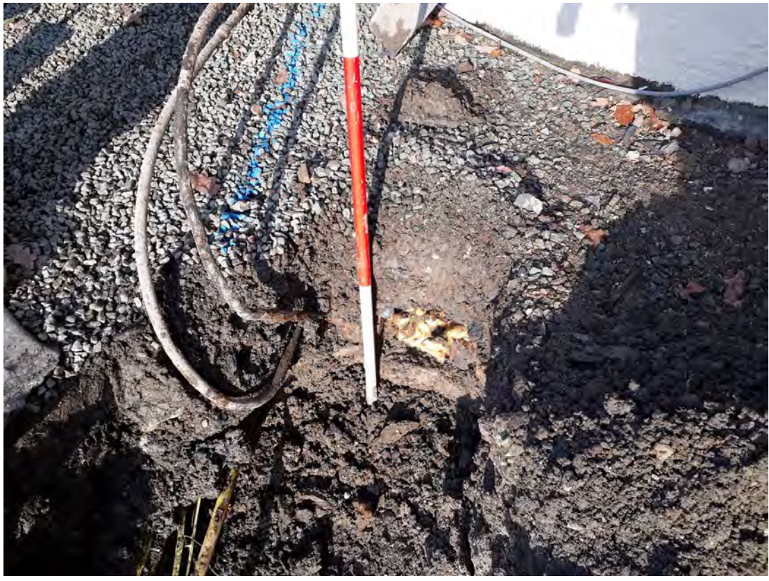
Plate 19. Drainage run to the NW of the house, showing rockwool insulation within pipe to boiler house. View SE. 2m scale
