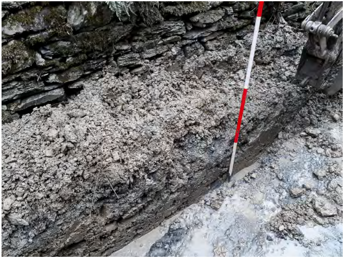
Plate 29. Drainage run to the NE (rear) of the house, clay in section. View NE. 2m scale
