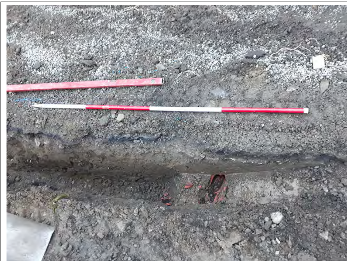
Plate 10. Drainage run at the SW (front) of the house with land drain. View NE.
