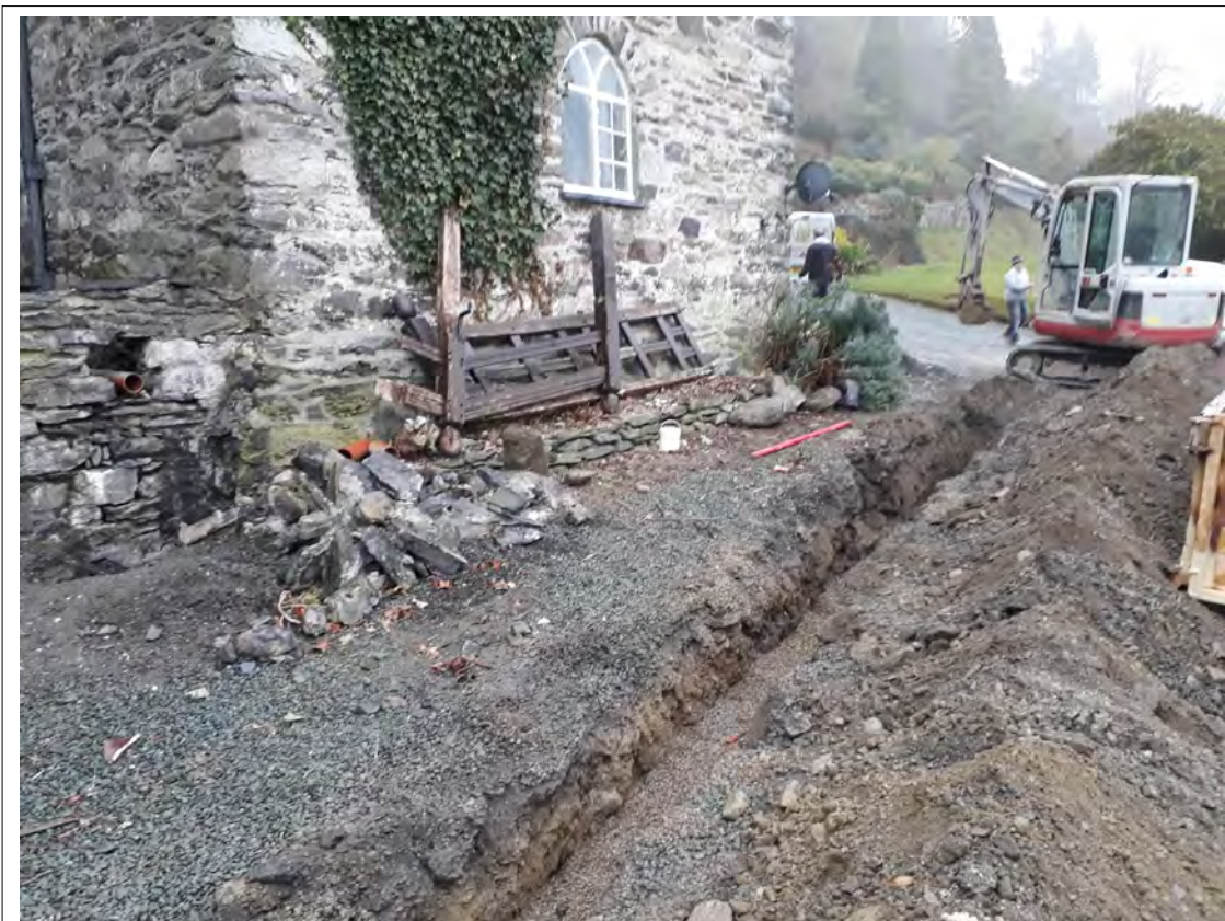
Plate 8. Drainage run at the SW (front) of the house. View SE.
