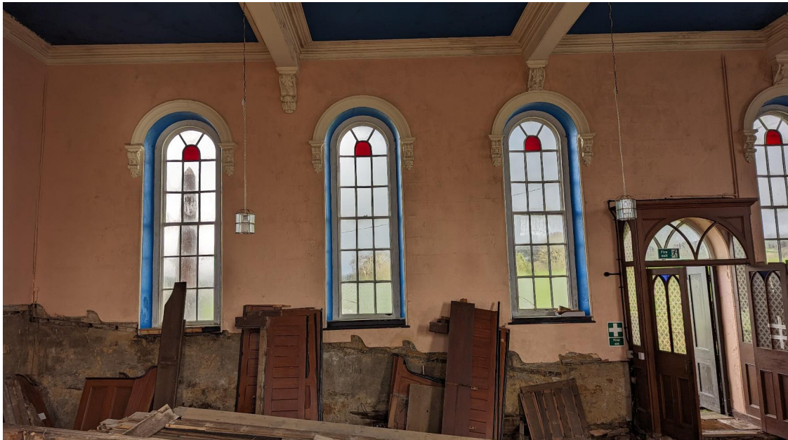
Plate 32: Removed pews and panelling
