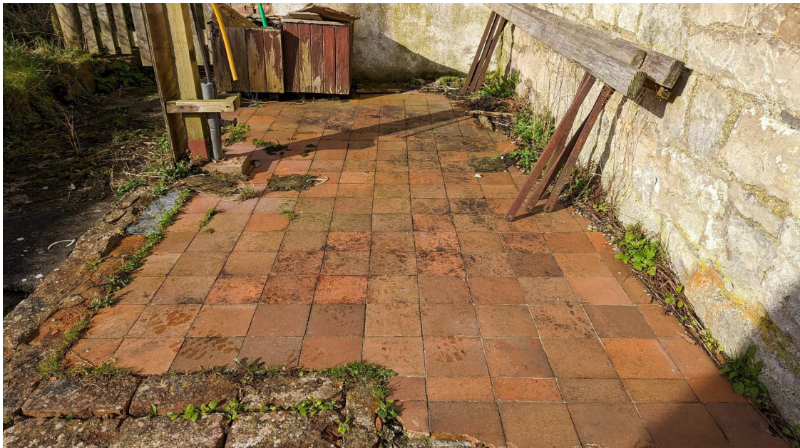
Plate 15: Demolished toilet block floor
