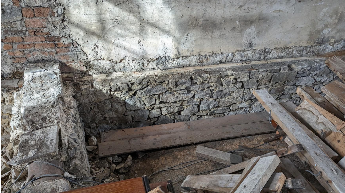
Plate 31: Foundation wall on western wall of chapel, with heating pipework in amalgam
