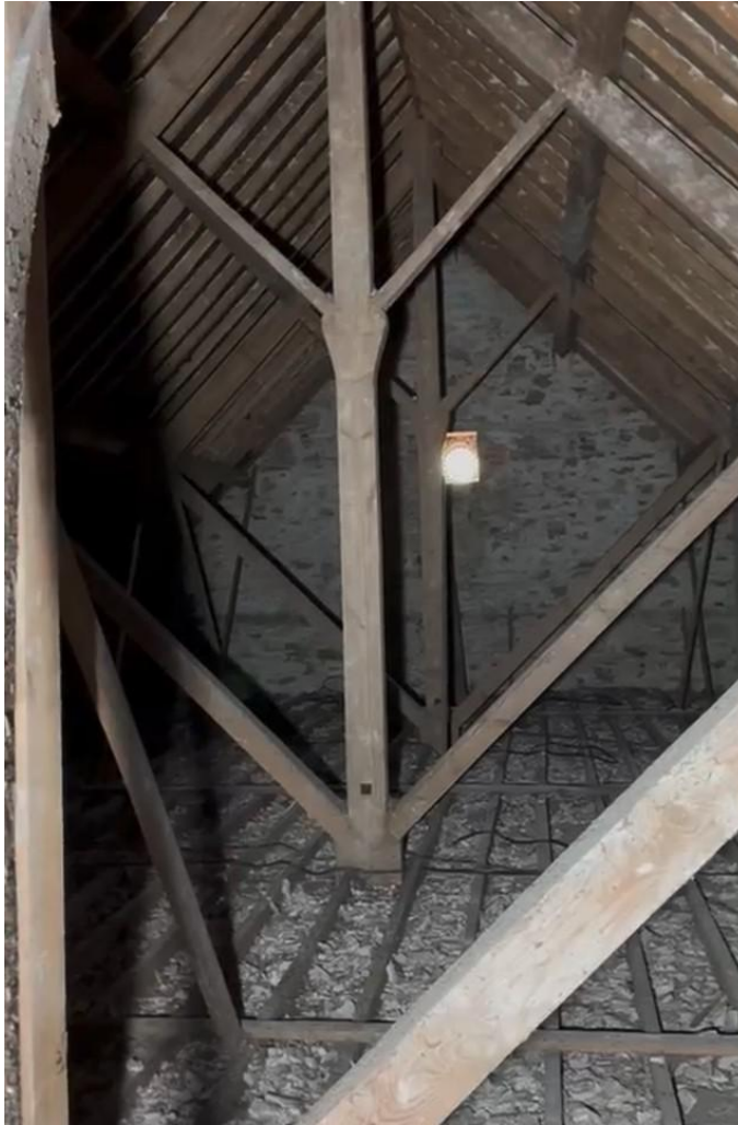
Plate 30: Roof posts and trusses
