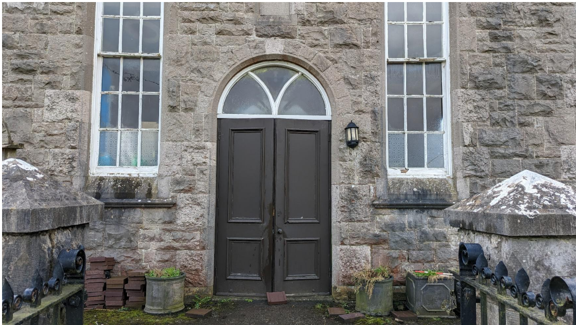
Plate 24: Northern elevation main entrance
