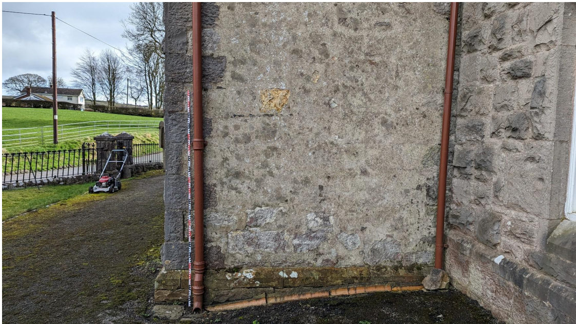
Plate 9: The west elevation showing render and plinth
