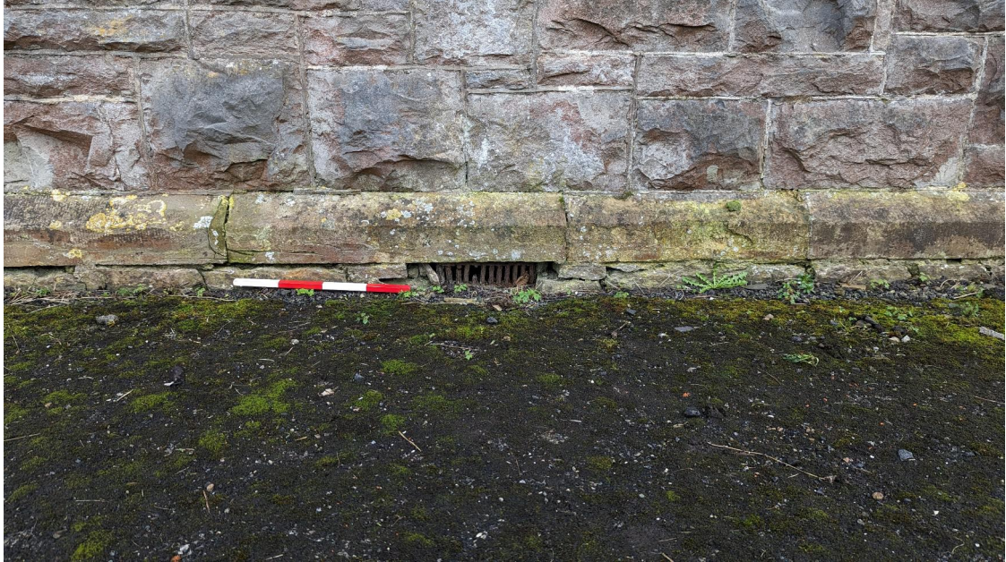
Plate 22: Northern elevation vents and plinth
