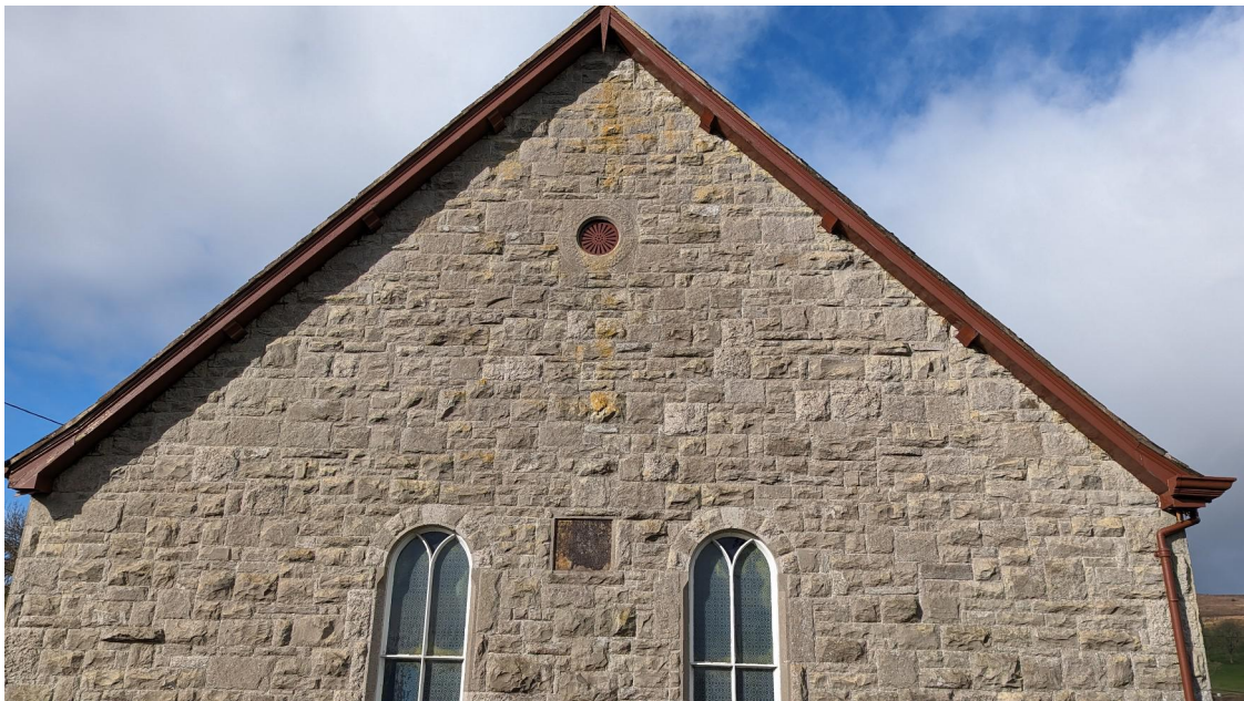
Plate 17: Eastern elevation detail
