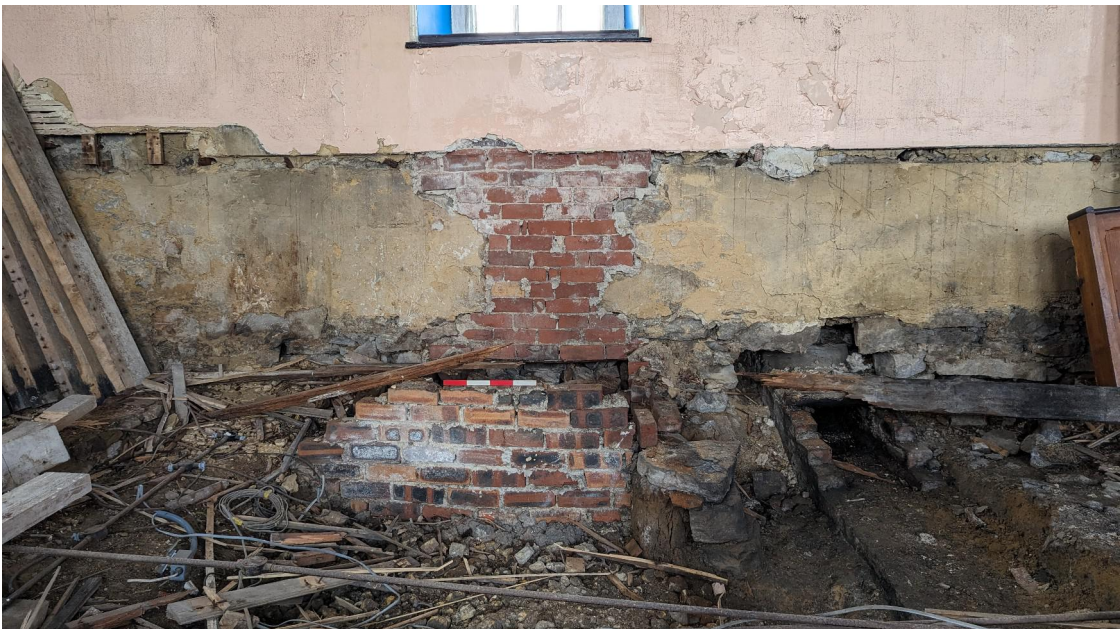
Plate 34: 20 th century repair and 19 th century heating culvert
