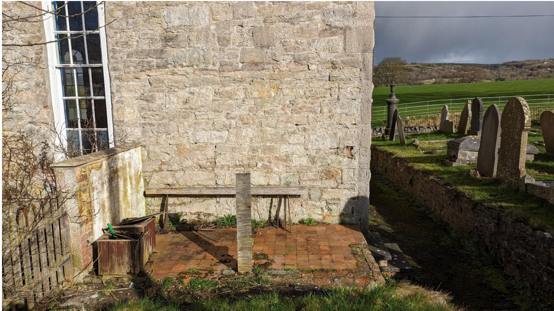
Plate 14: Demolished toilet block
