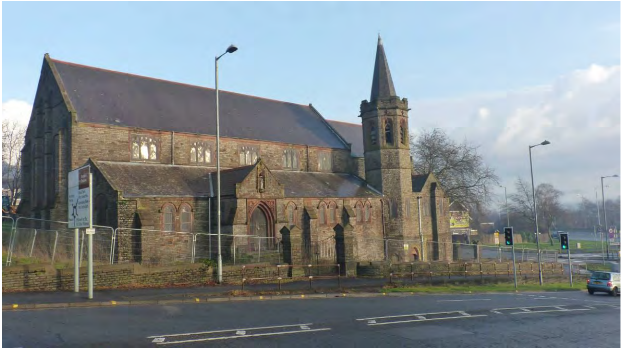
Photo 9: View of the south face of St Paul's Church, Cwm Level Road in the foreground.
