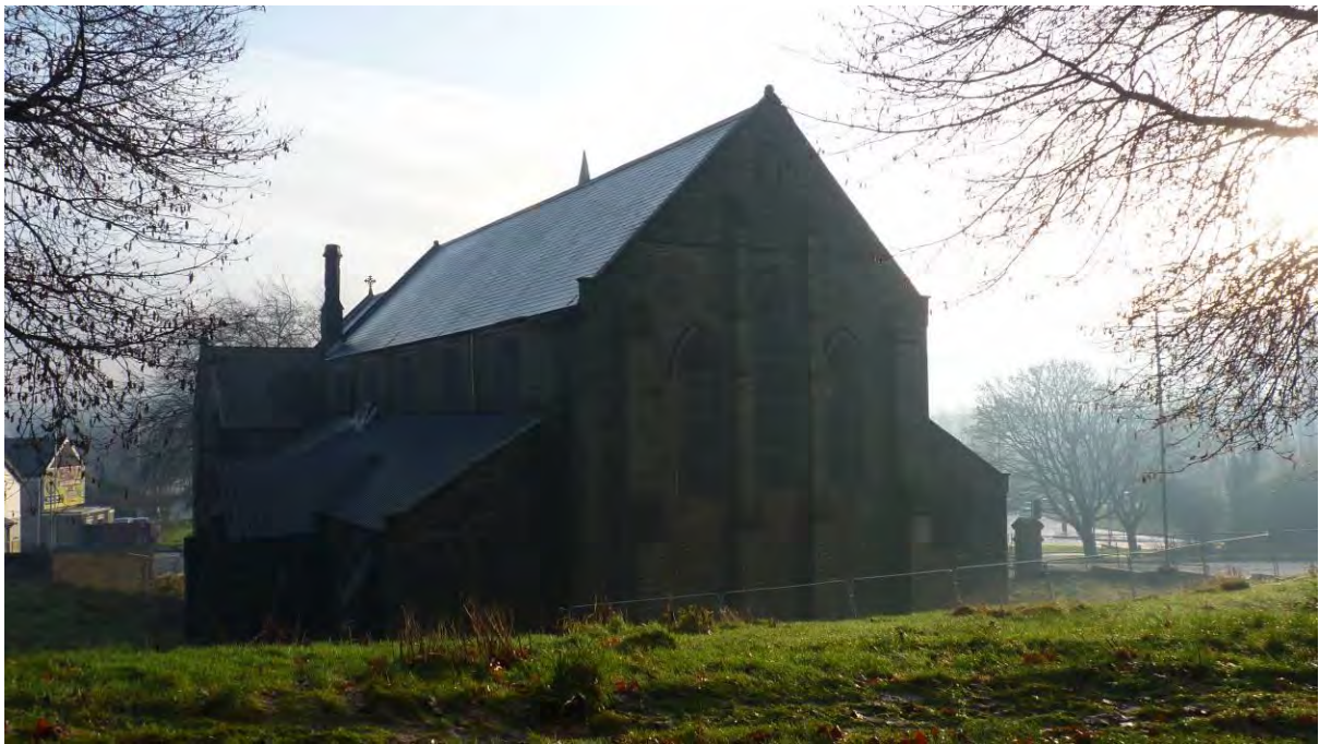
Photo 10: View of the west face of St Paul's church from within the proposed development area.
