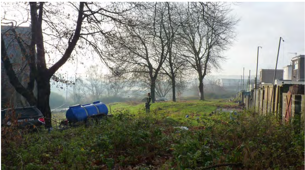
Photo 18: View south across the proposed development area, proposed dwellings will occupy the higher ground. Landeg Street property boundaries visible on the right, St Paul's Church on the left.
