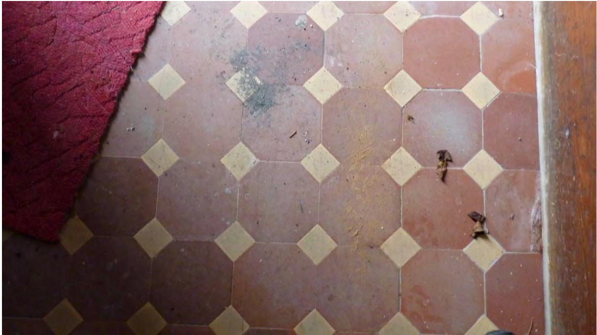
Photo 15: Floor of the vestibule.
