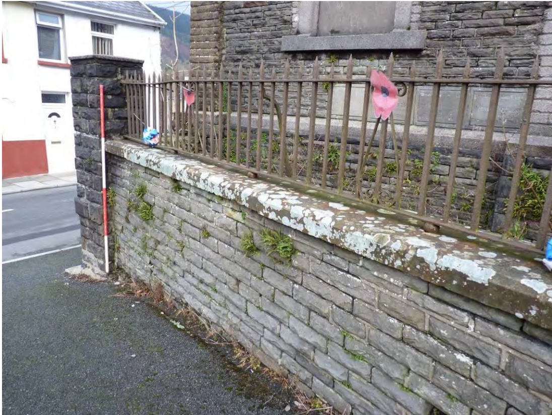
Photo 7: Enclosure wall around front of the chapel. View north, 2m scale.
