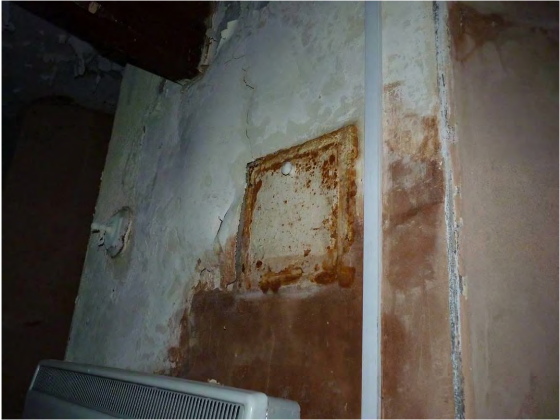
Photo 35: Original fittings on the wall of the main chapel.
