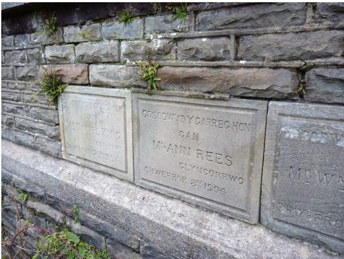
Photo 6: Foundation plaques on front wall. View north.
