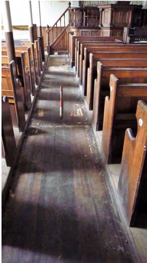
Photo 21: Flooring (wooden floorboards) within the chapel area. View northeast, 2m scale.
