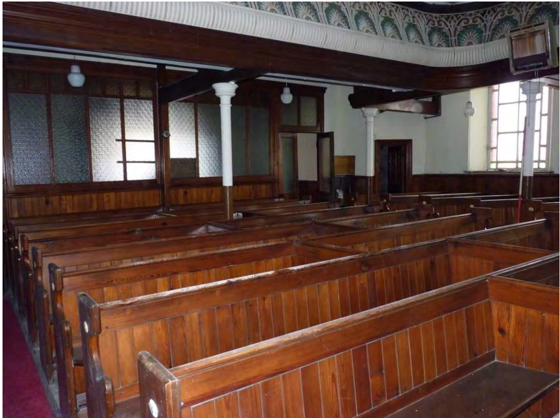
Photo 41: Buttresses and columns holding the gallery above, at the southwest end of the chapel. View west, 2m scale.
