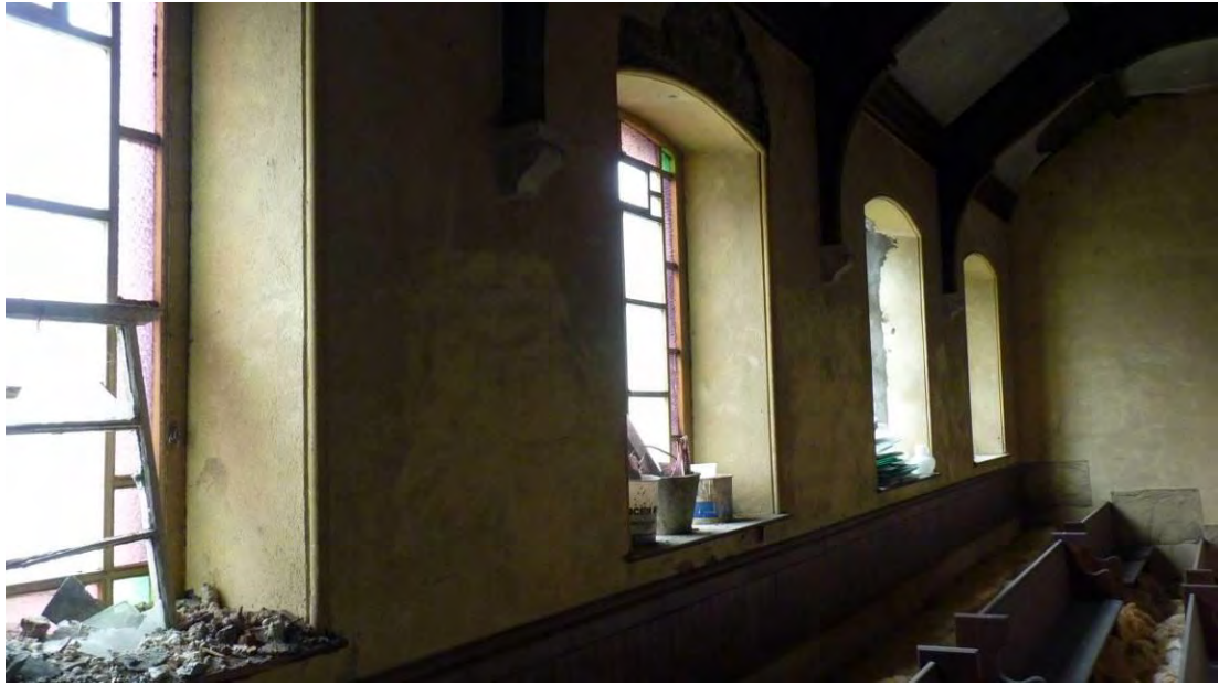
Photo 51: 1 st floor windows along the northwest wall. View north.
