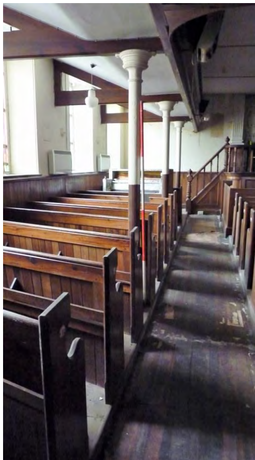
Photo 40: Buttresses and columns holding the gallery above. View northeast, 2m scale.
