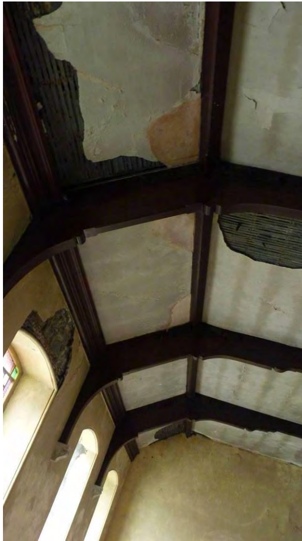
Photo 52: Ceiling detail, showing the ceiling joists against the northwest wall.
