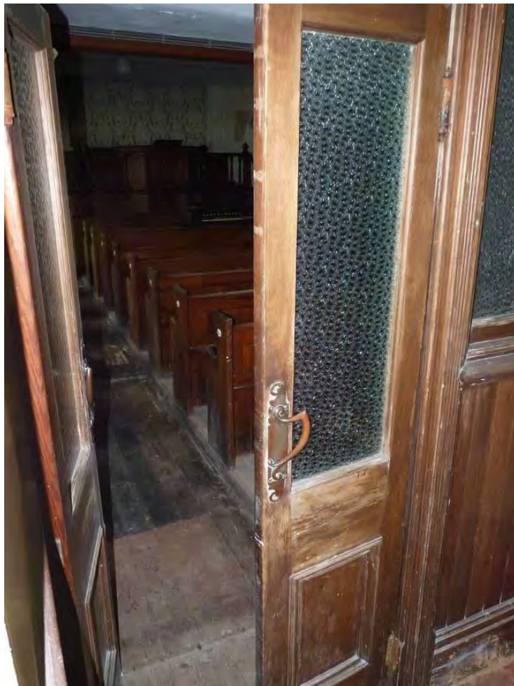
Photo 16: Doorway (one of two) giving access from the vestibule to the main chapel. View northeast.
