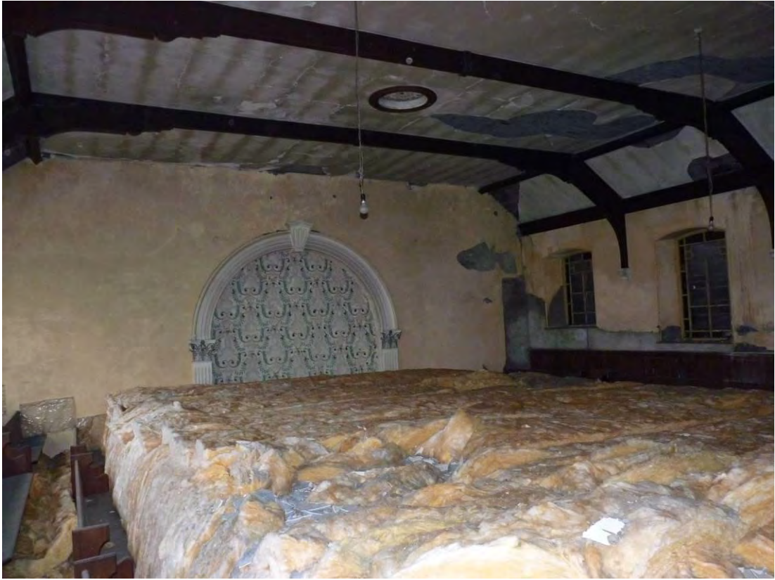
Photo 45: View from the top of the 1 st floor access stairs, showing the insulation-covered inserted ceiling. View east.
