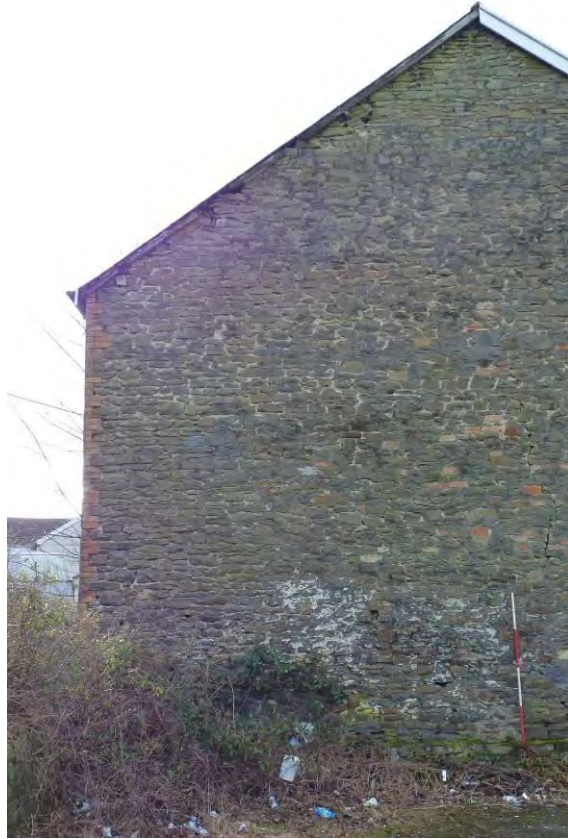
Photo 11: North-east gable elevation. View southwest, 2m scale.
