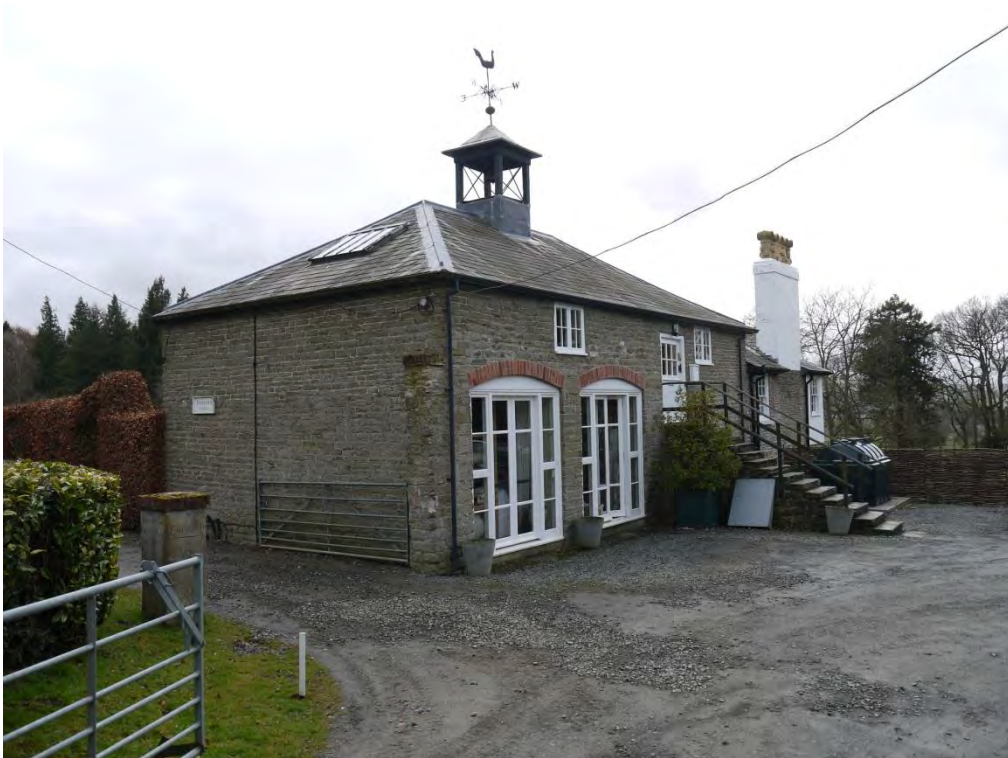
Photo 8: View of Coach House (LB 9150) from within courtyard looking south.
