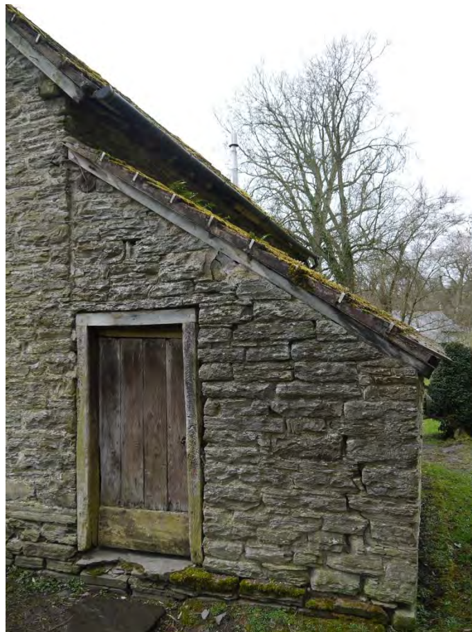
Photo 6: Lean to outbuilding, looking west.
