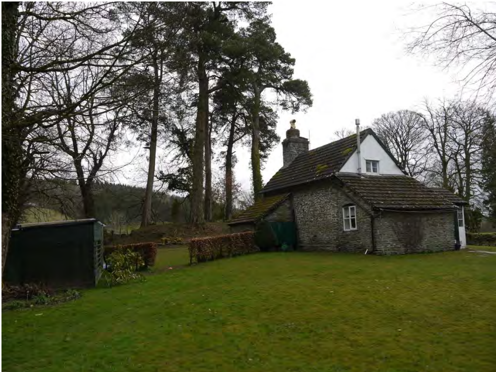
Photo 2: Rear of cottage, mound in background and hills behind, looking southeast.
