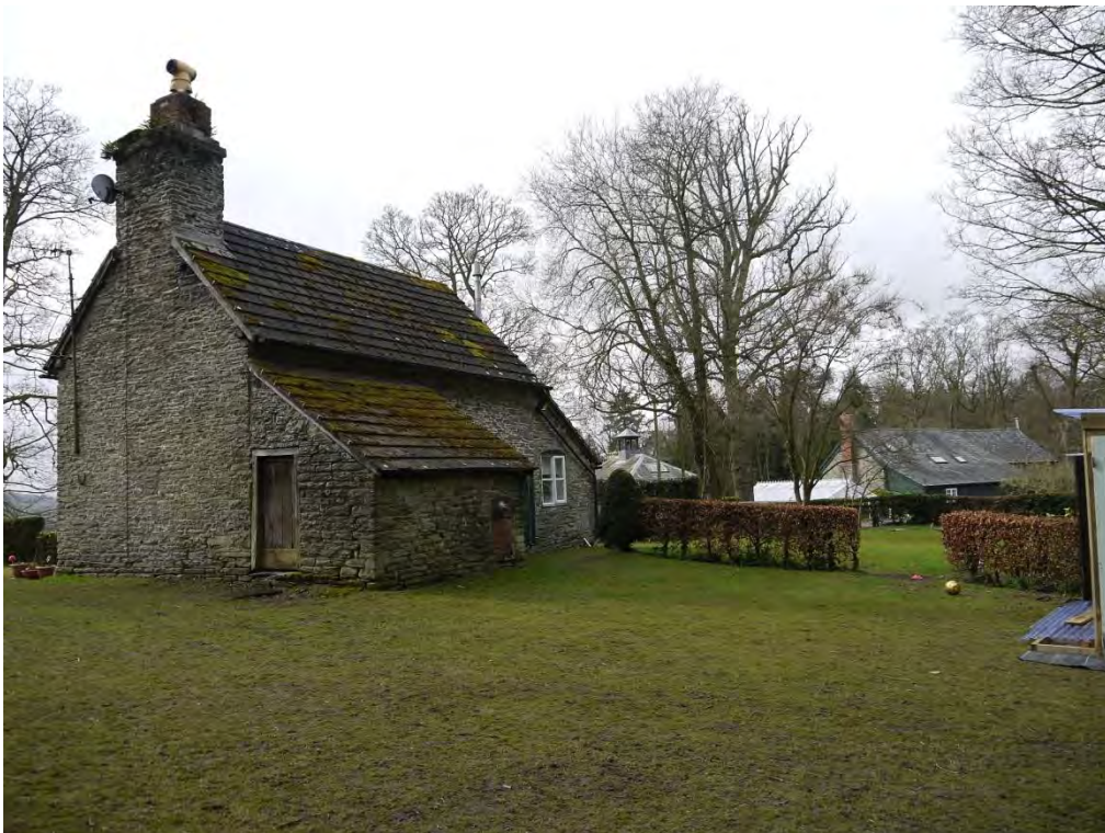
Photo 4: Rear of cottage with view towards stable block (LB 9151) and coach house (LB 9150), looking southwest.
