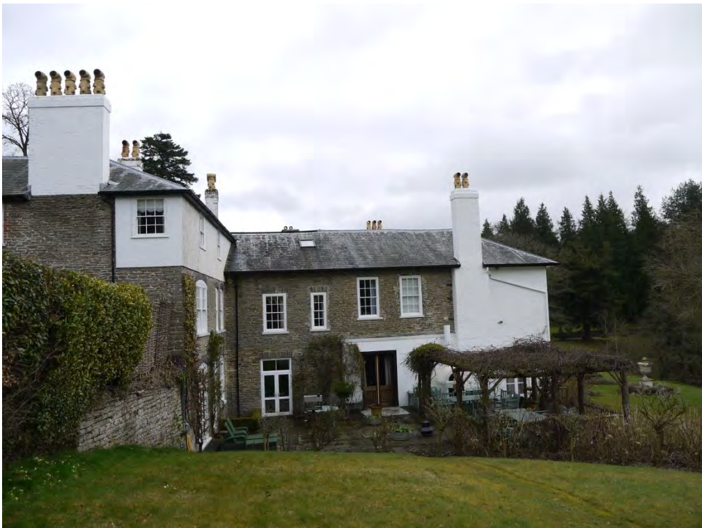
Photo 10: Rear of Evancoyd House (LB 9149) looking east.
