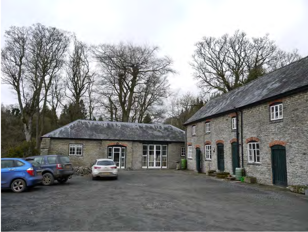
Photo 9: View of outbuildings (LB 9152 & 9151) looking northwest.
