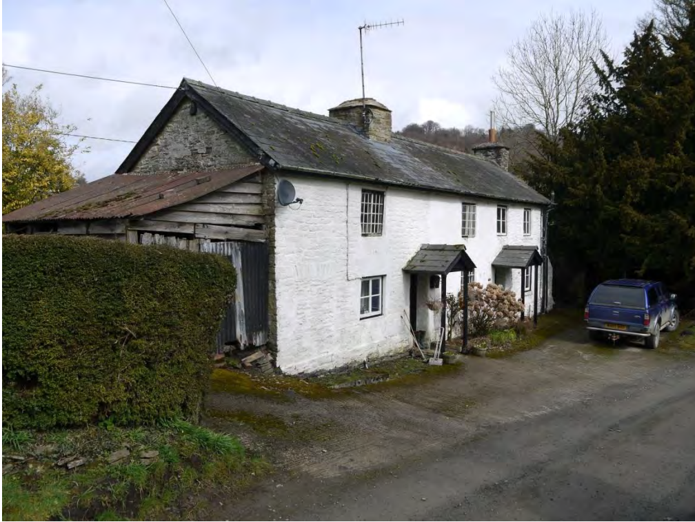
Photo 17: Gardener's Cottage (LB 9153) looking northeast.
