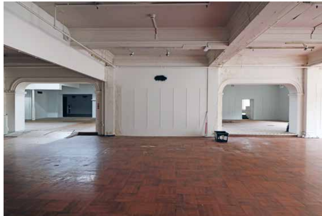
View of room 2/01. IMG_7525.
