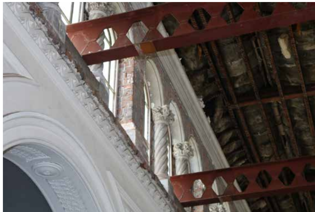
Detail of the clerestory with moulded masonry columns. IMG_7282.
