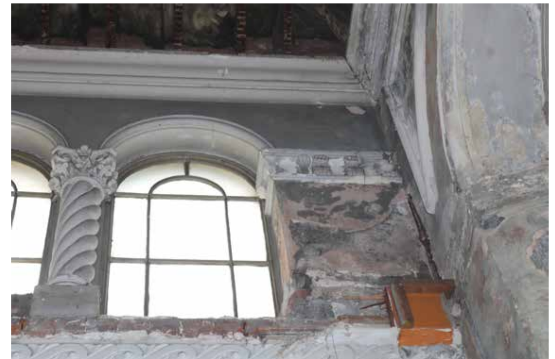
Detail of the clerestory with moulded masonry columns. IMG_7684.
