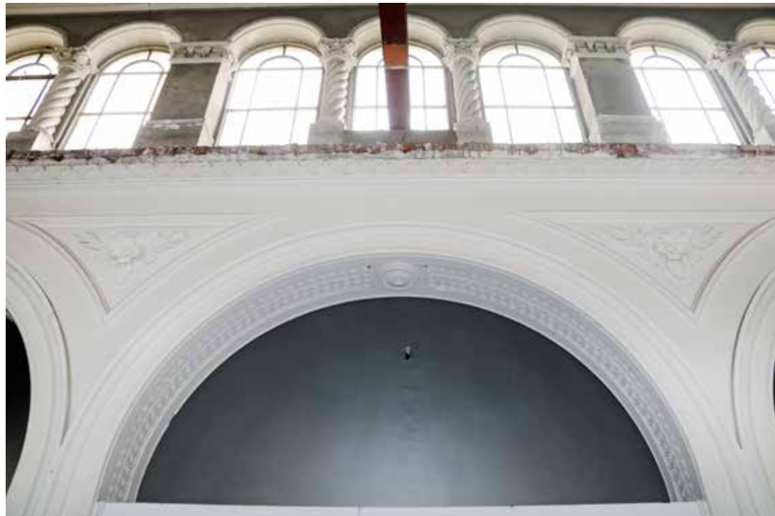
Detail of the original plasterwork side aisle arches. IMG_7664.
