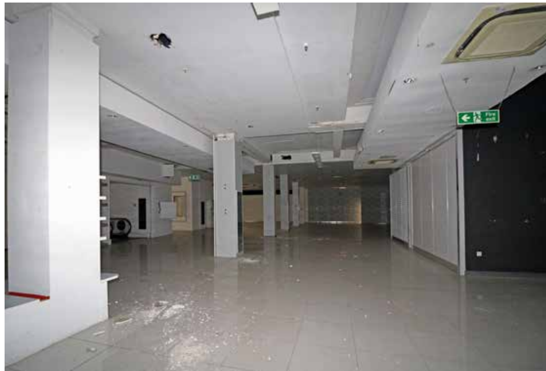
View of room 1/04, in character area IA. IMG_7702.
