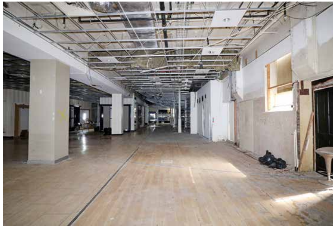
View of room 0/05, in character area IA. IMG_8075.
