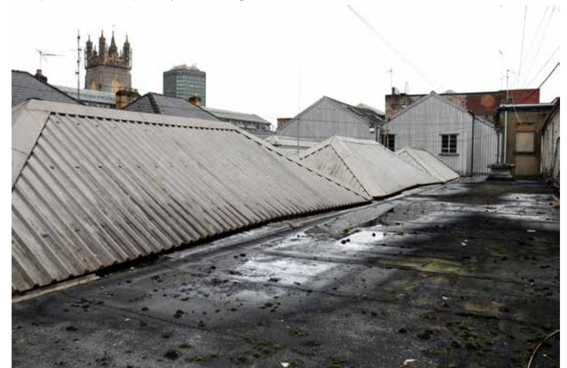
View of St Mary building roof, 2/10. IMG_7641.
