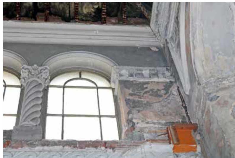
Detail of windows and steel support at clerestory level, 1/02. IMG_7684
