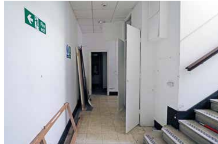
0/25 staircase and landing at ground floor level. IMG_8280
