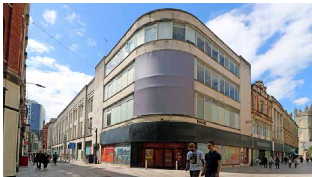
View of Howells and elevations B and C, looking west. IMG_8317.
