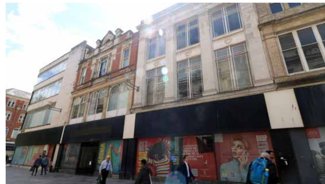
View of external elevation C, Trinity Street, IMG_8313.
