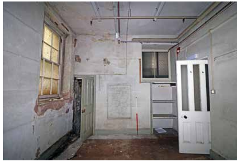
Southeast view of room 0/16. IMG_8172.
