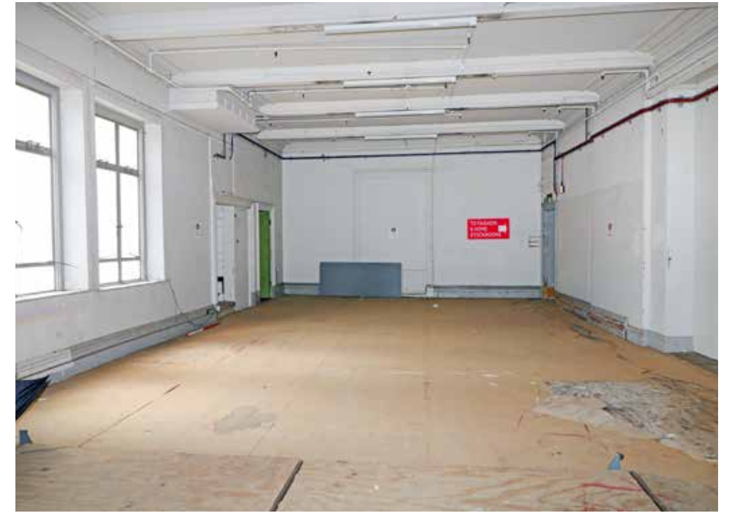
Room 2/15 on the second floor looking south west. IMG_7617
