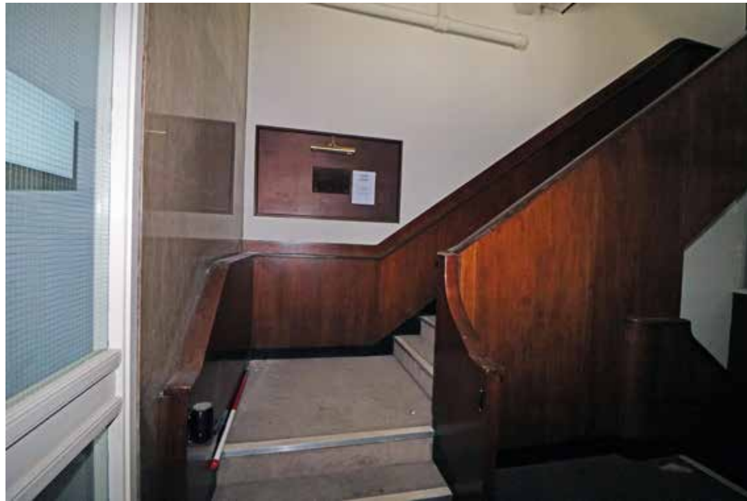
2/13 staircase at second floor. IMG_7602
