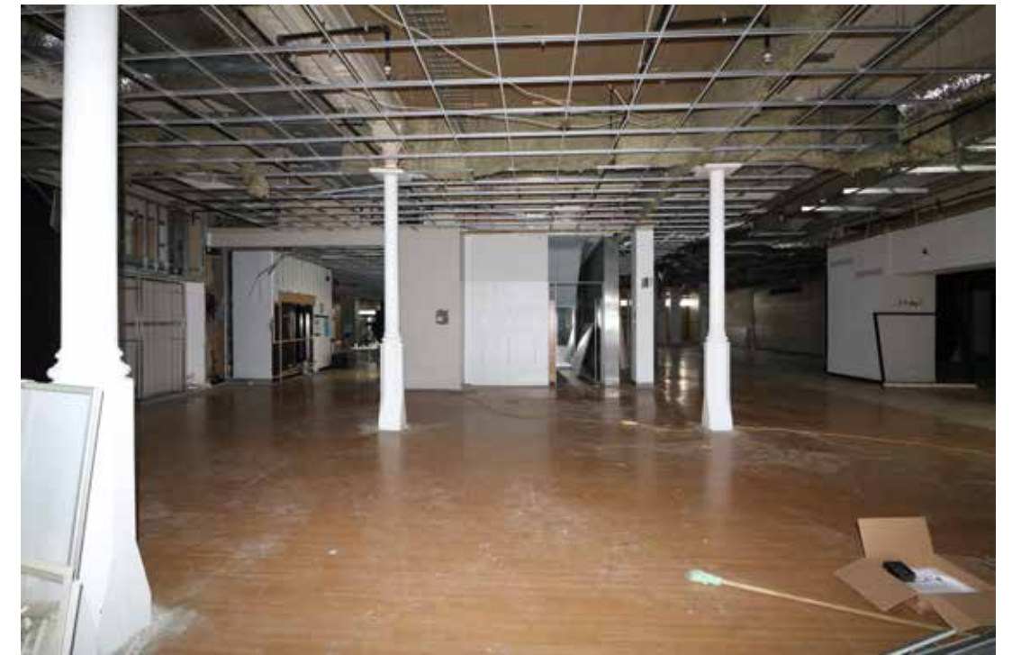
View of room 0/04, in character area IA. IMG_8062.
