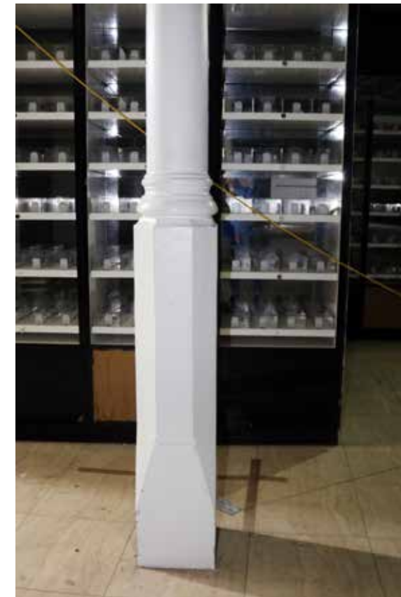
Detail of the column base on the ground floor. (IMG_8084, 1878 column)
