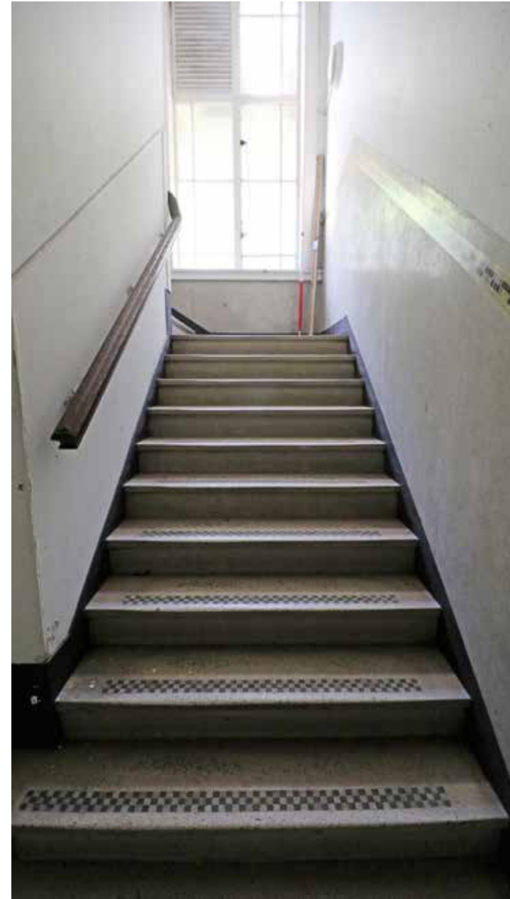
0/25 staircase and landing at ground floor level. IMG_8282
