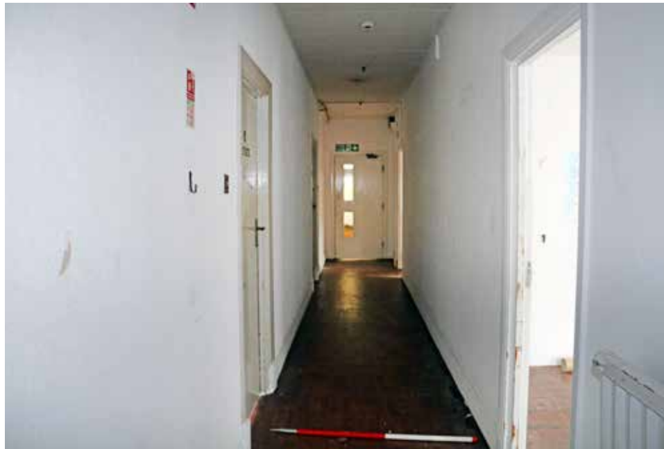
View of corridor, room 3/22, from type 7D. IMG_7467.
