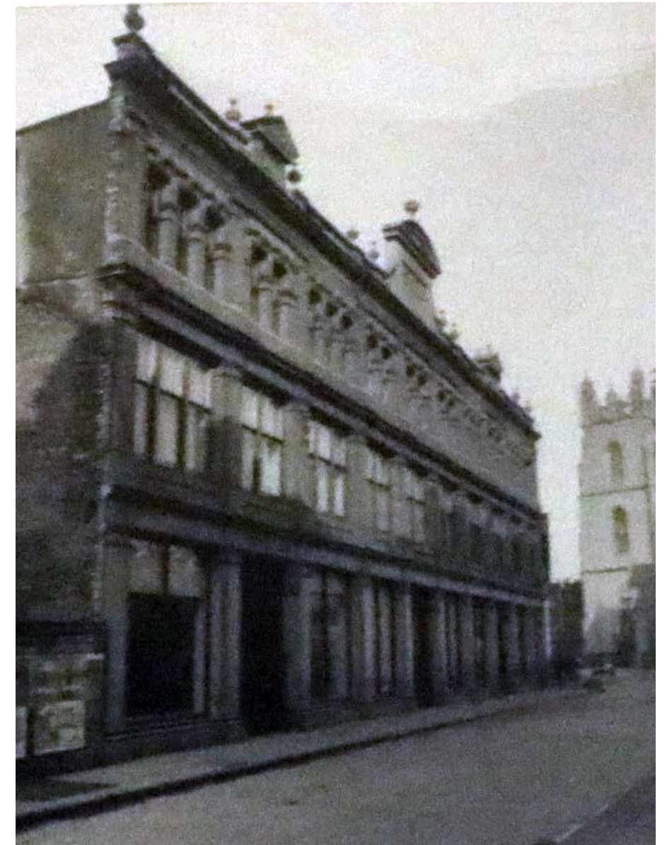
Trinity Street buildings pictured in the late 19th century or early 20th century - note the now missing urns to the parapet and the taller ground floor windows (House of Fraser Archive) (**permission pending**)
