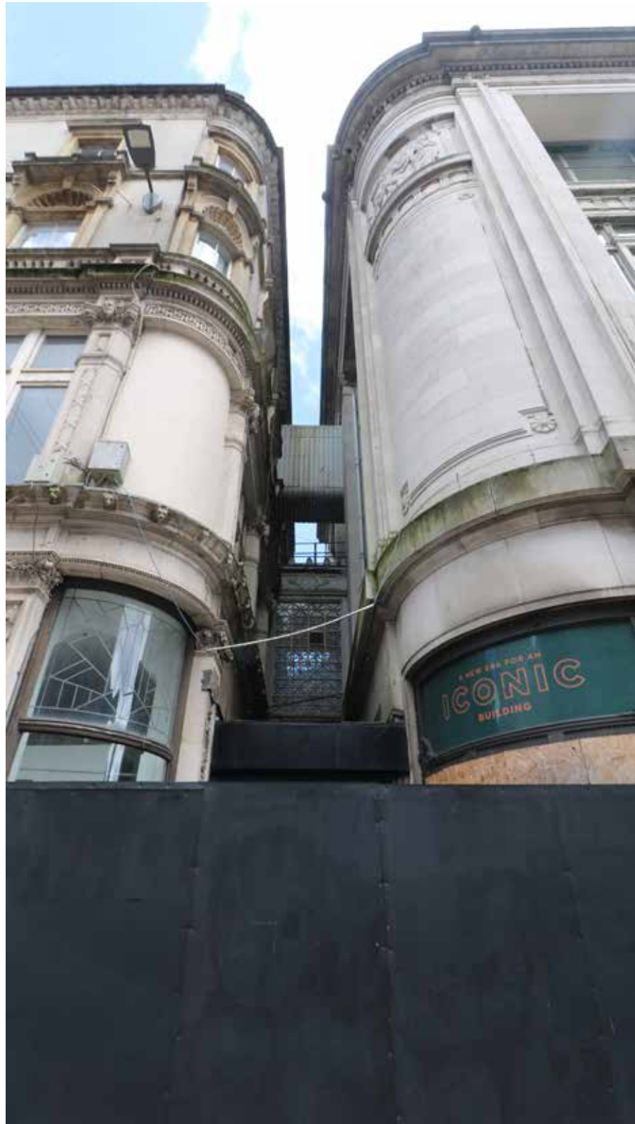
View of external elevation A, St Mary's Street. IMG_8332.
