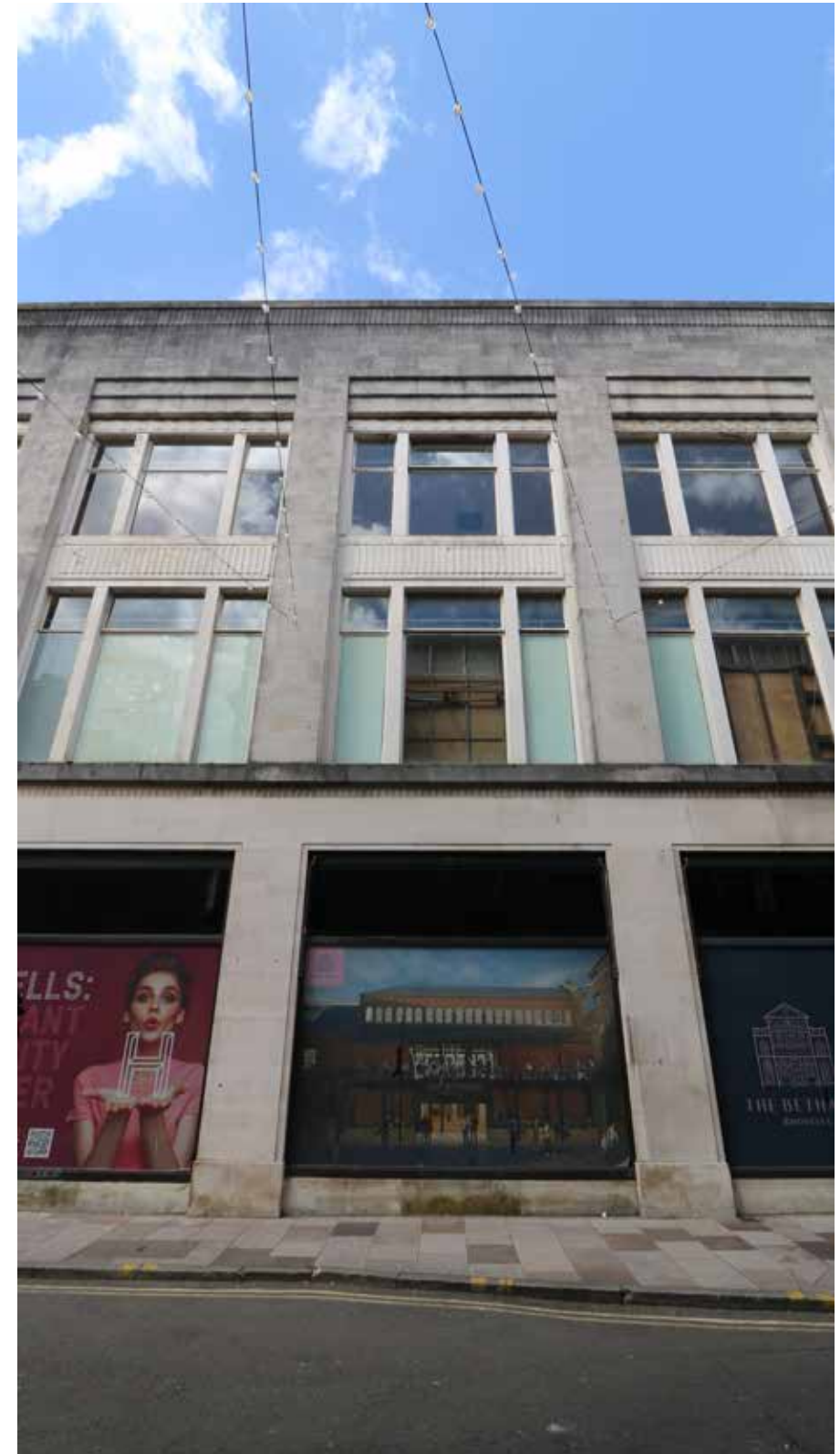
View of external elevation B, Wharton Street. IMG_8324.
