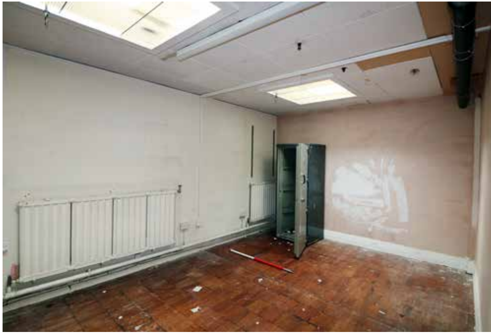
View of room 3/2, from type 7A. IMG_7462.
