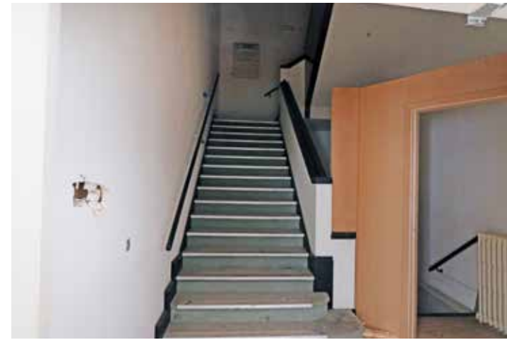
0/22 staircase at ground floor level. IMG_8238
