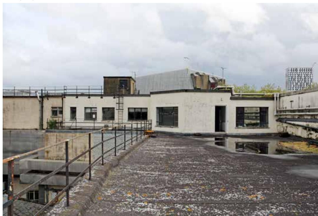
View of roof, 3/26. IMG_7479
