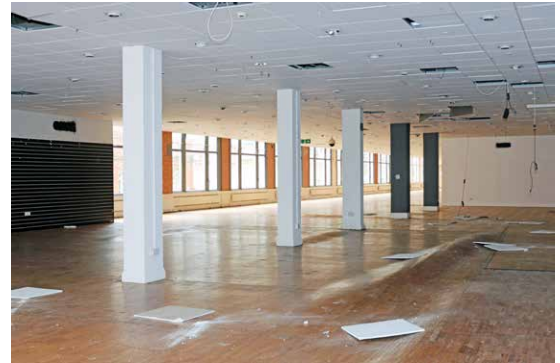
View of room 2/04, in character area IB. IMG_7547.
