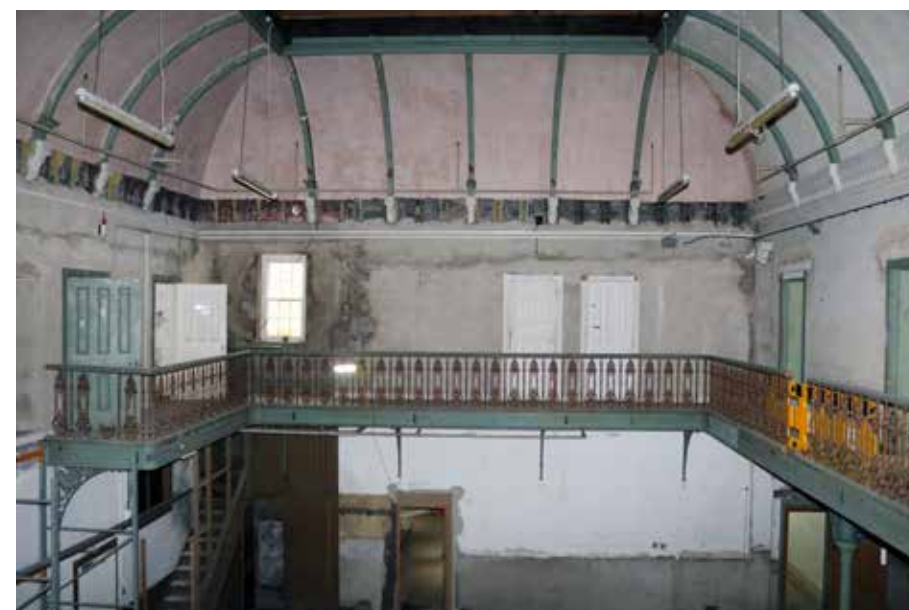
View of the hall, 0/06, from 1F balcony. IMG_7815.
