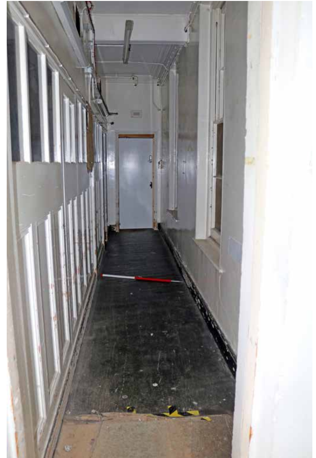
The timber partition within the corridor space, looking south east. IMG_7640.
