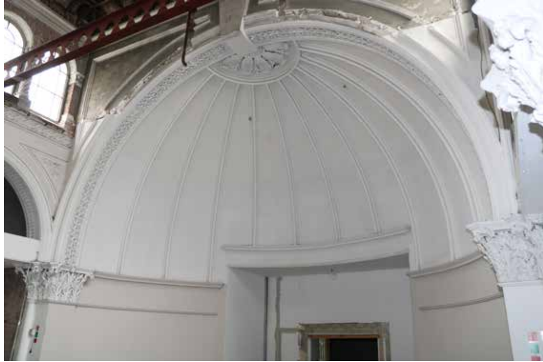
Decorative plasterwork of the domed ceiling on the north east end of the Chapel. IMG_7668.
