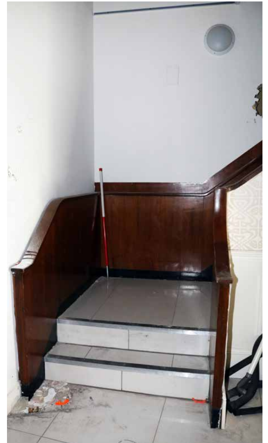
1/01 staircase at first floor level. IMG_7651
