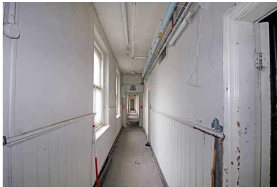
View of corridor, 3/32, from type 7E. IMG_7503.
