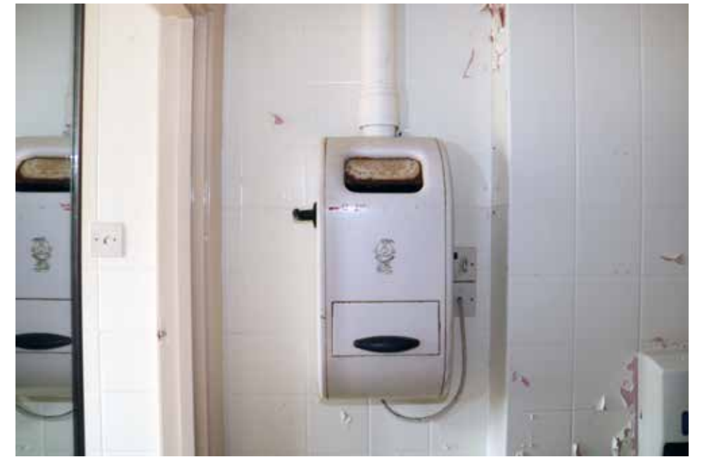
Detail of incinerator in room 3/16, from type 7C. IMG_7440.
