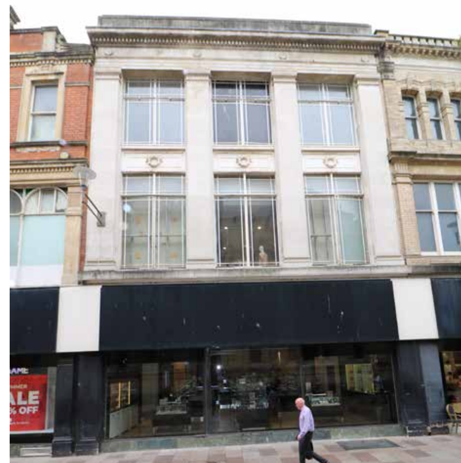
Photo of the Gas and Plumbing building facade, taken in 2022, IMG_0493
