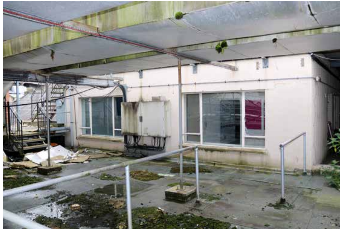
View of roof, 3/18. IMG_7445
