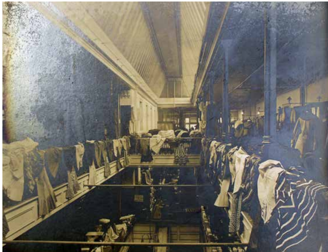
Interior of the St Mary Street shop floor in 1912, showing the long glazed lantern where the 1870s and 1880s phases met. (Glamorgan Archives) (**permission pending**)
