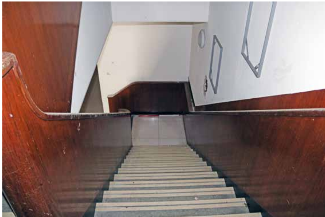
1/01 staircase at first floor level. IMG_7649
