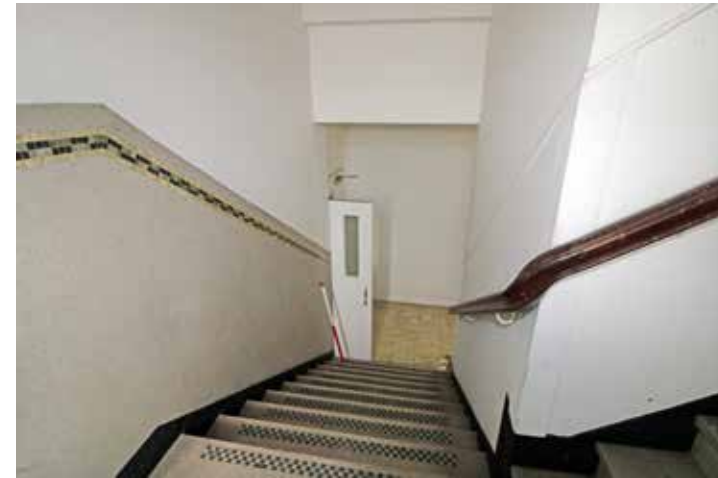
1/27 staircase between first and second floors. IMG_7847
