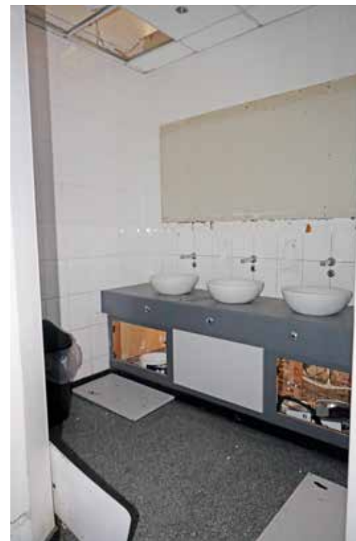
Modern toilet fit out, 1/07. IMG_7742.
