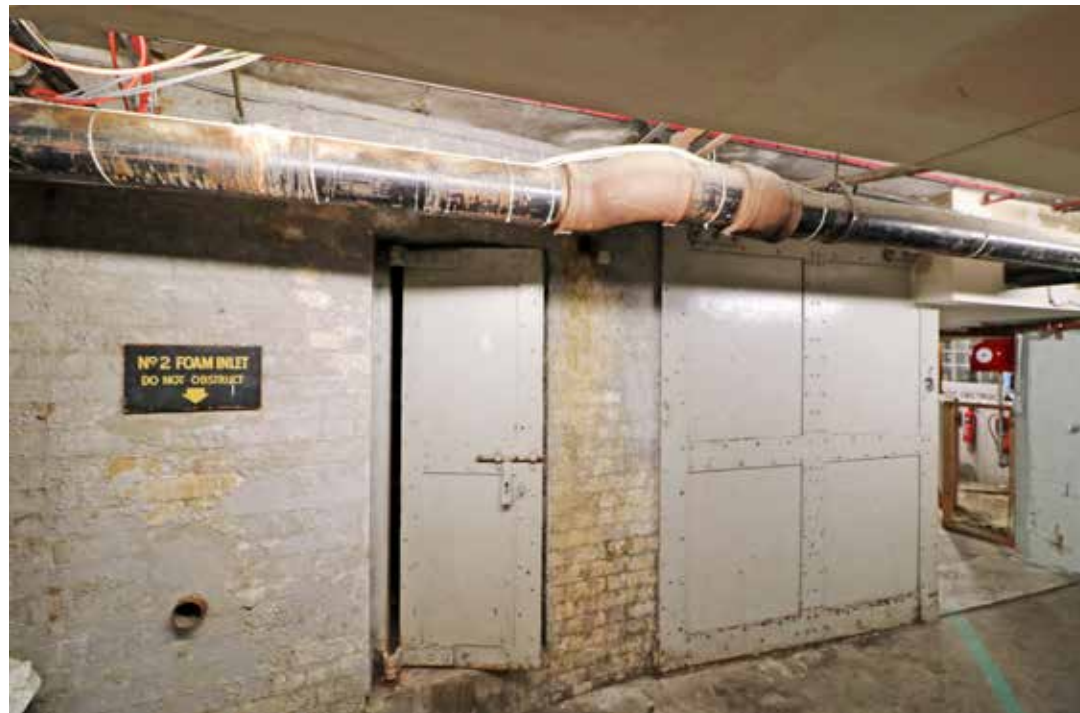
View of the two fire doors looking south (b(5)).
