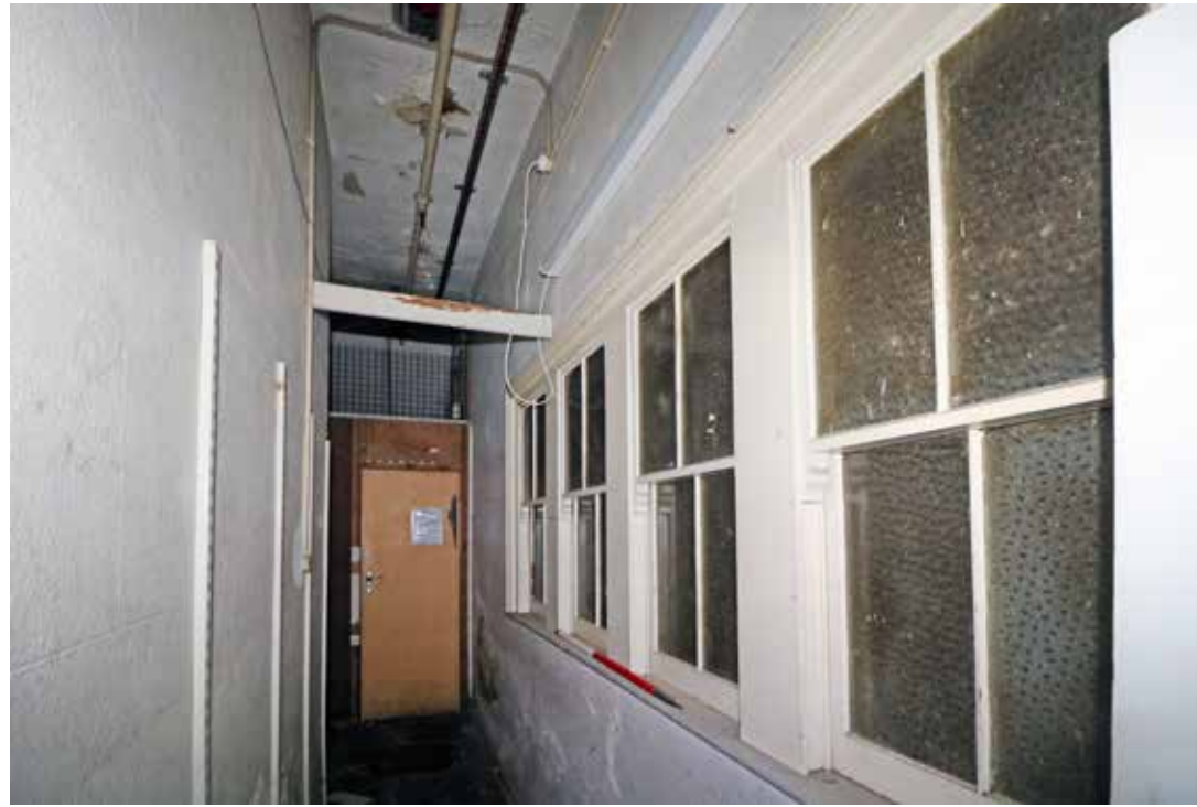
Timber sash windows as seen from 0/08 entrance hall corridor. IMG_8124.
