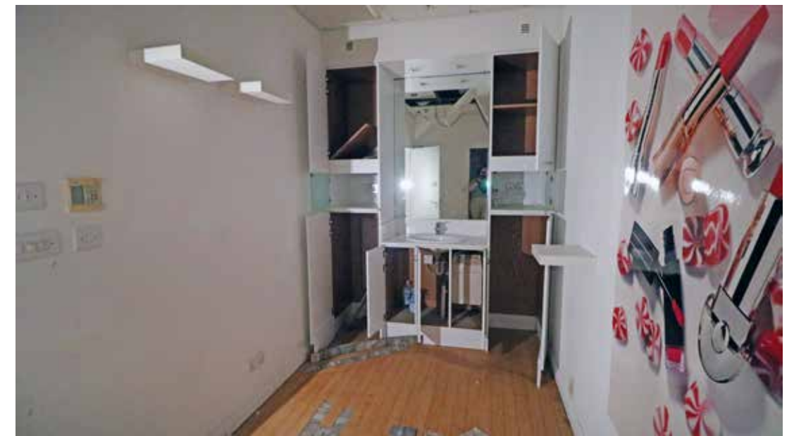
View of room 0/25a on the ground floor. IMG_8288.
