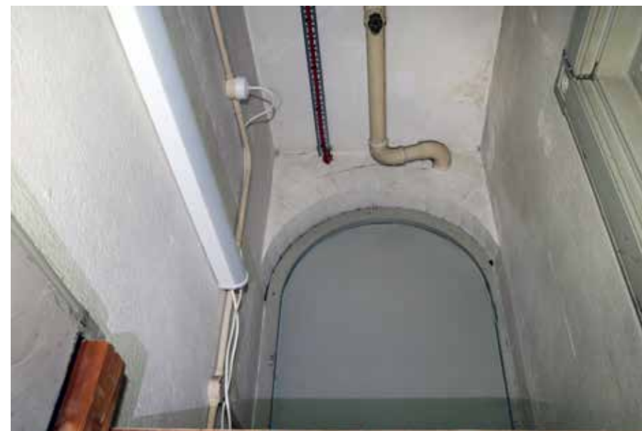
Detail of door arch in room 0/08. IMG_8127.
