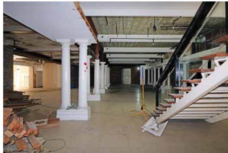
South-west view of the chapel, 0/20, including plywood columns, historic arcade plaster roof and modern steel and concrete roof. IMG_8208
