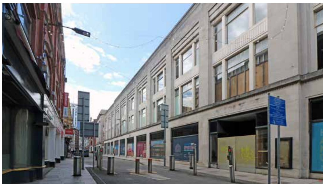
View along Wharton Street (Elevation B). IMG_8320
