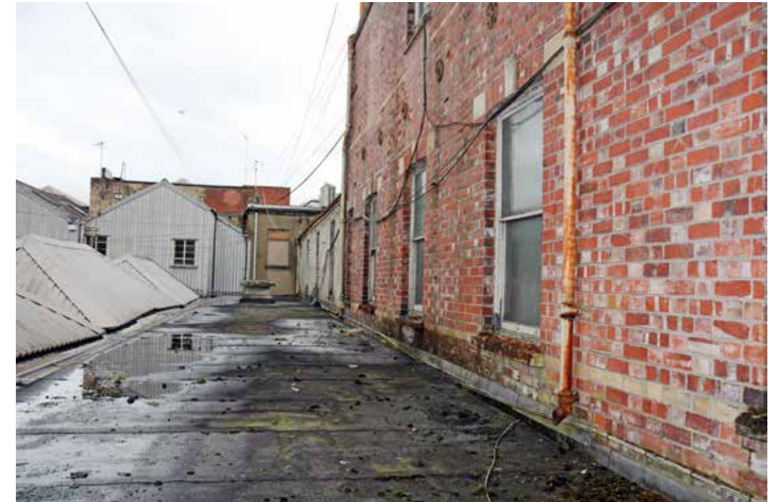
View of the northern wall of St Mary Street building, 2/10. IMG_7642.
