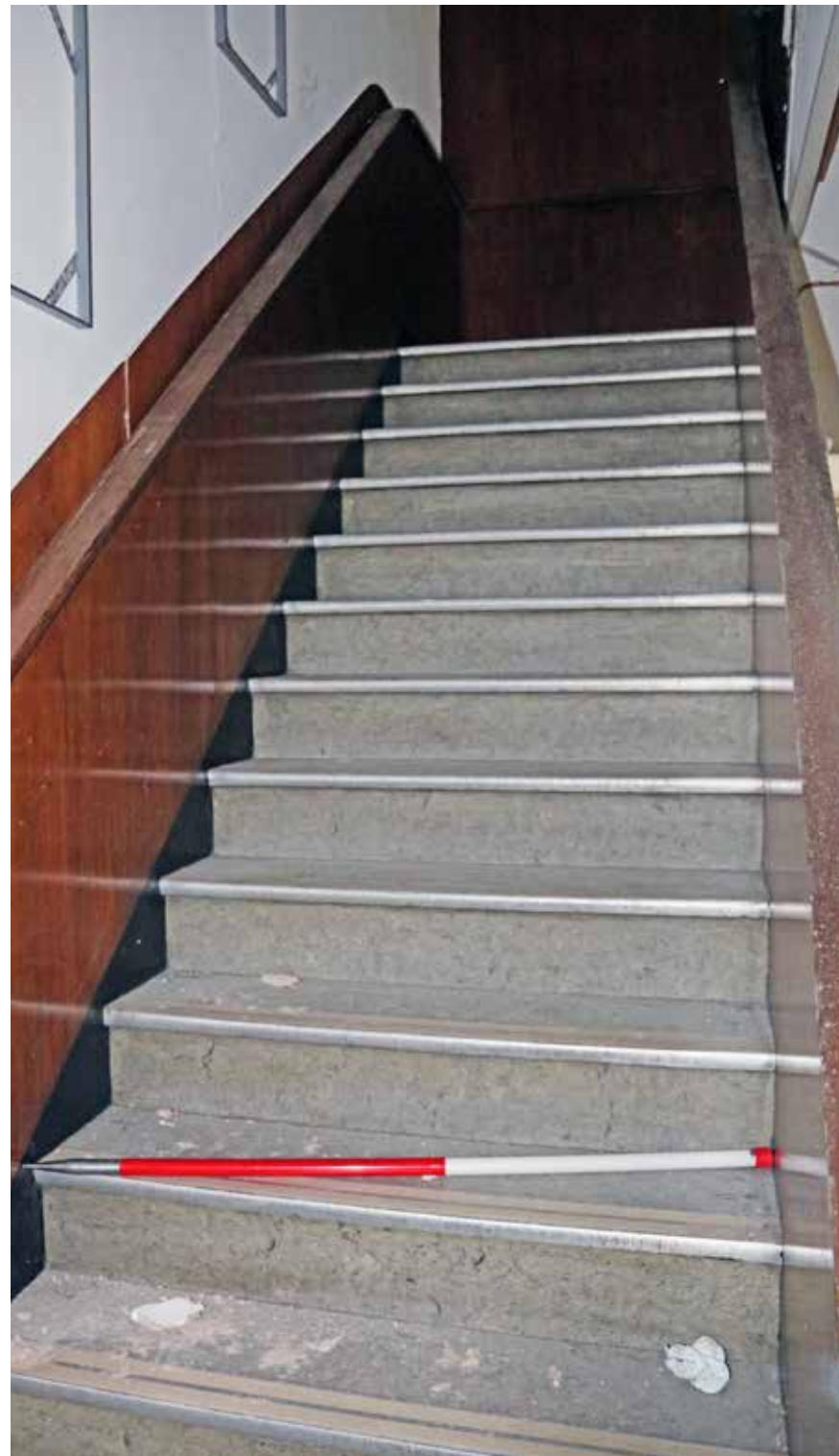
1/01 staircase at first floor level. IMG_7650
