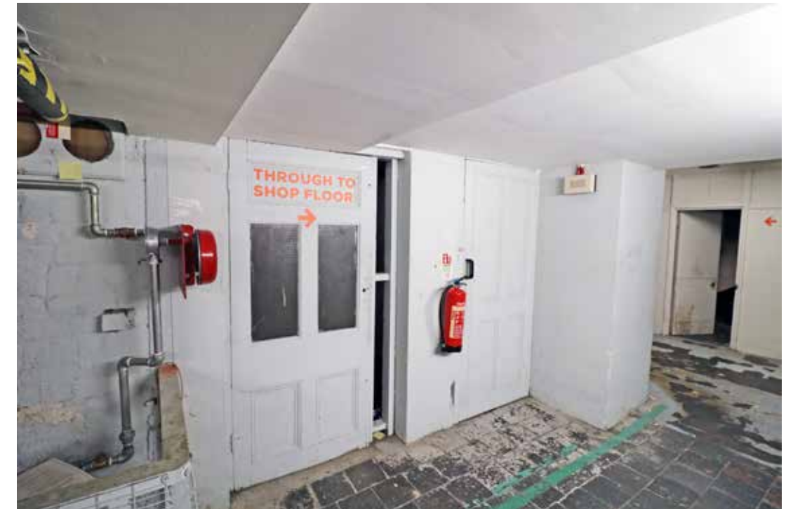
View of corridor, B/01
