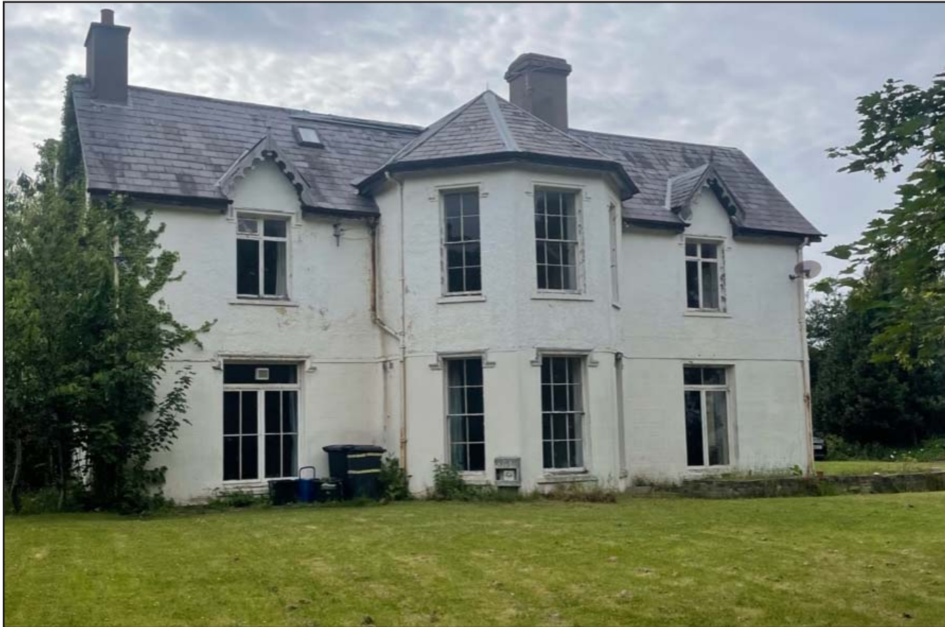
Plate A: View of Tan-yr-Allt Hall prior to renovation works, taken by the Client - from the southeast.
