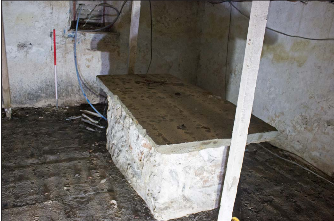
Plate 42: Store/preparation room, basement, Tanrallt Hall, Abergele Road, Llanddulas, Abergele - from the southwest - 1.00m scale
