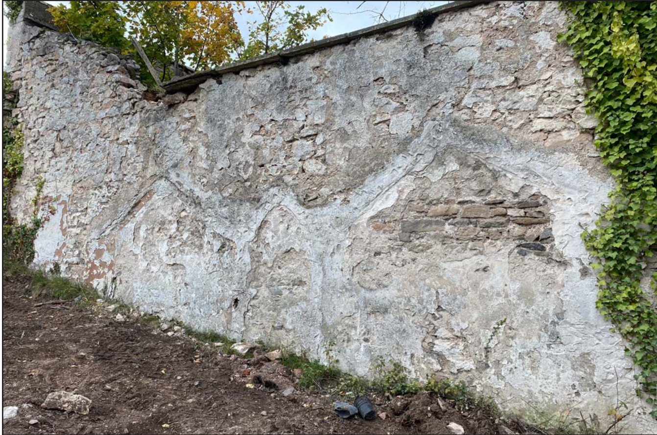
Plate 13: Outline of former buildings on the stable yard wall of Tanrallt Hall, Abergele Road, Llanddulas, Abergele - from the northeast - no scale
