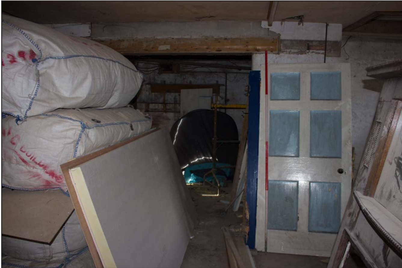
Plate 12: Internal shot of Store 2 and Store 3 within Dairy Outbuilding at Bryn Cwnin Farm, Pentre Lane, Rhuddlan, Rhyl, Denbighshire - from the northeast - 2.00m scale
