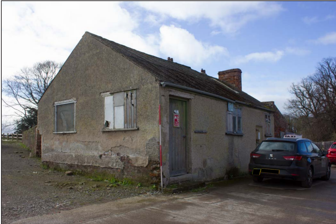
Plate 10: Oblique shot of northeast and northwest elevations of Dairy Outbuilding at Bryn Cwnin Farm, Pentre Lane, Rhuddlan, Rhyl, Denbighshire - from the north - 2.00m scale
