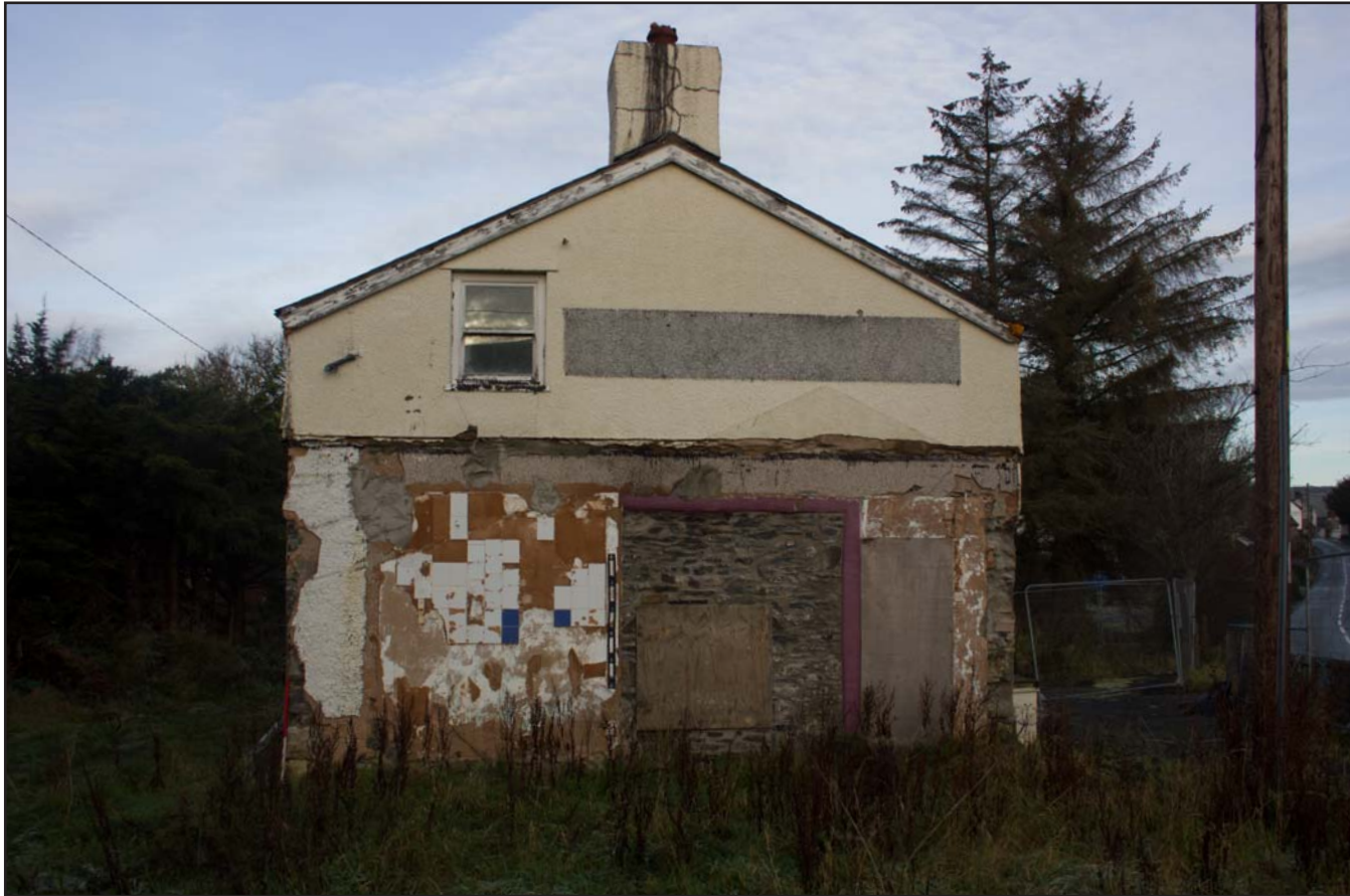
Plate 08: South facing external elevation, from the south. Scale 1.0m.
