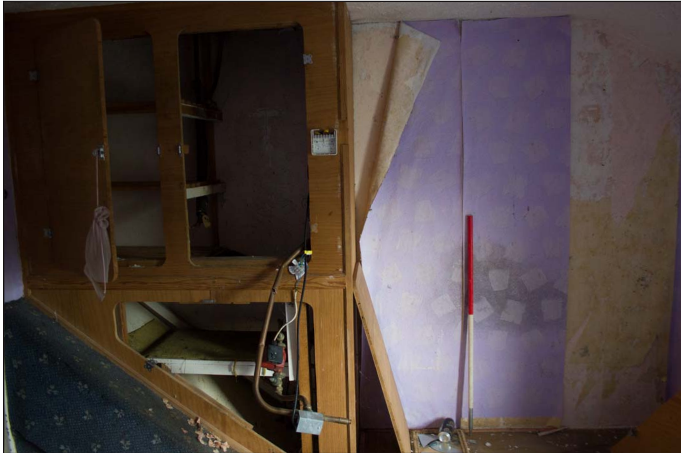
Plate 21: First Floor - Bedroom 2, from the south. Scale 1.0m.
