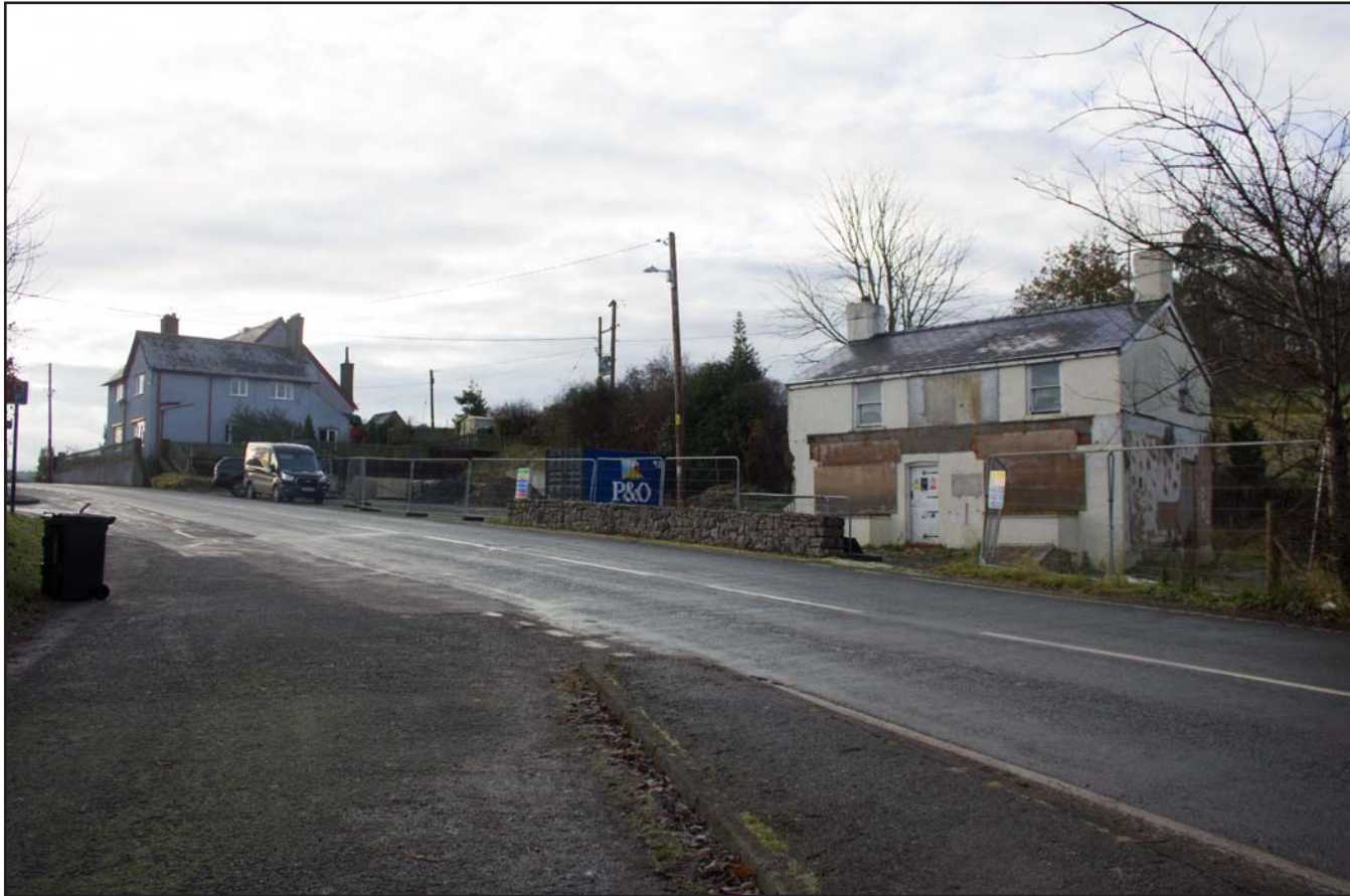
Plate 01: Context photograph of The Bridge Inn, from the northeast. Scale 1.0m.
