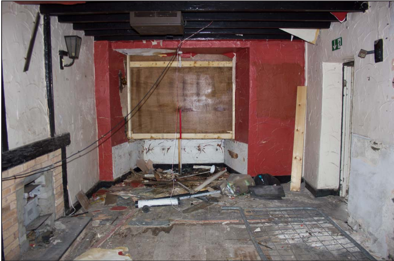
Plate 14: Ground Floor - Lounge, from the west. Scale 1.0m.
