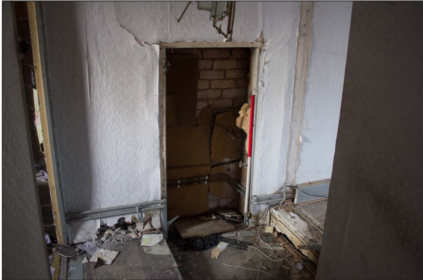
Plate 17: First Floor - Landing, from the southeast. Scale 1.0m.
