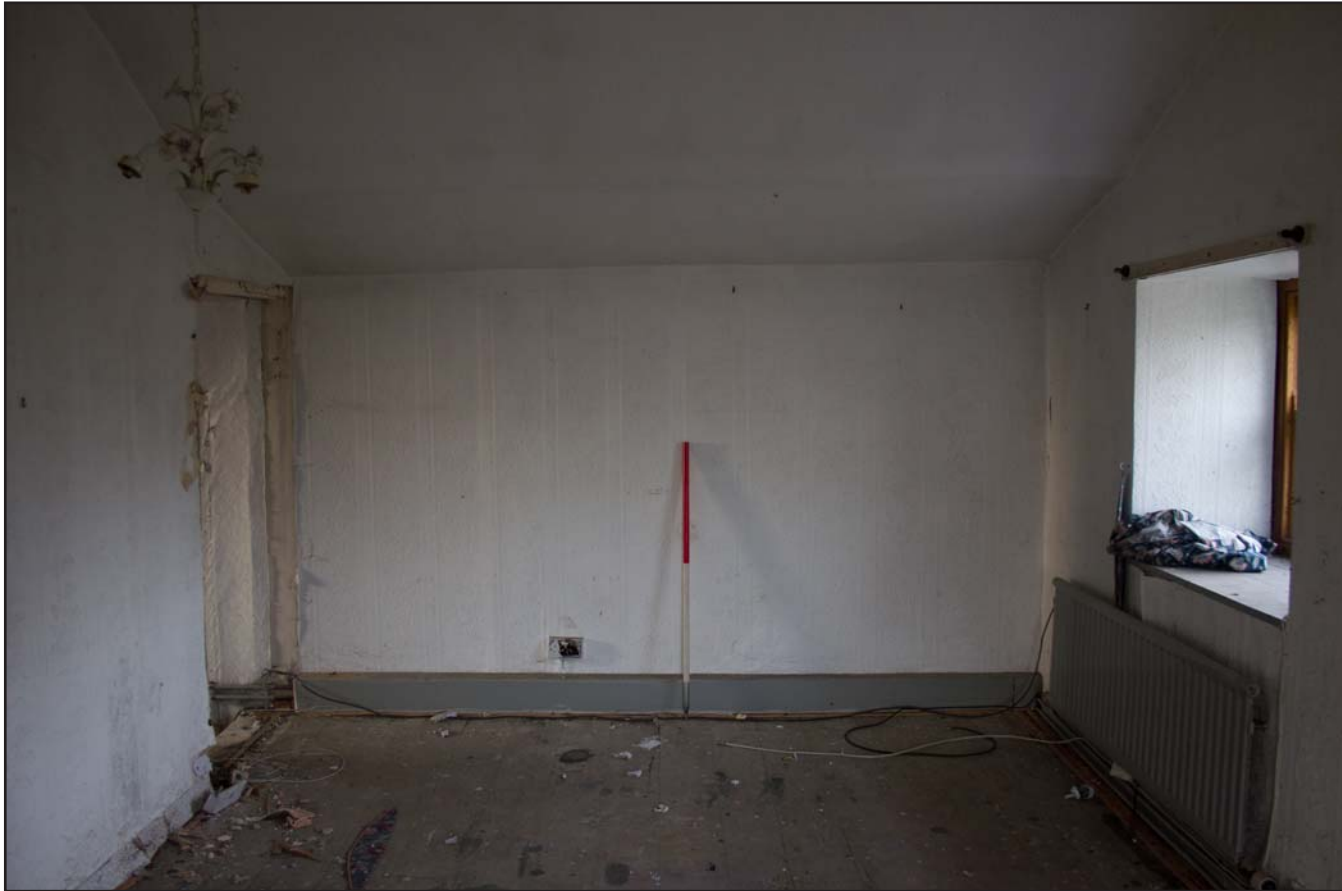
Plate 19: First Floor - Bedroom 1, from the east. Scale 1.0m.
