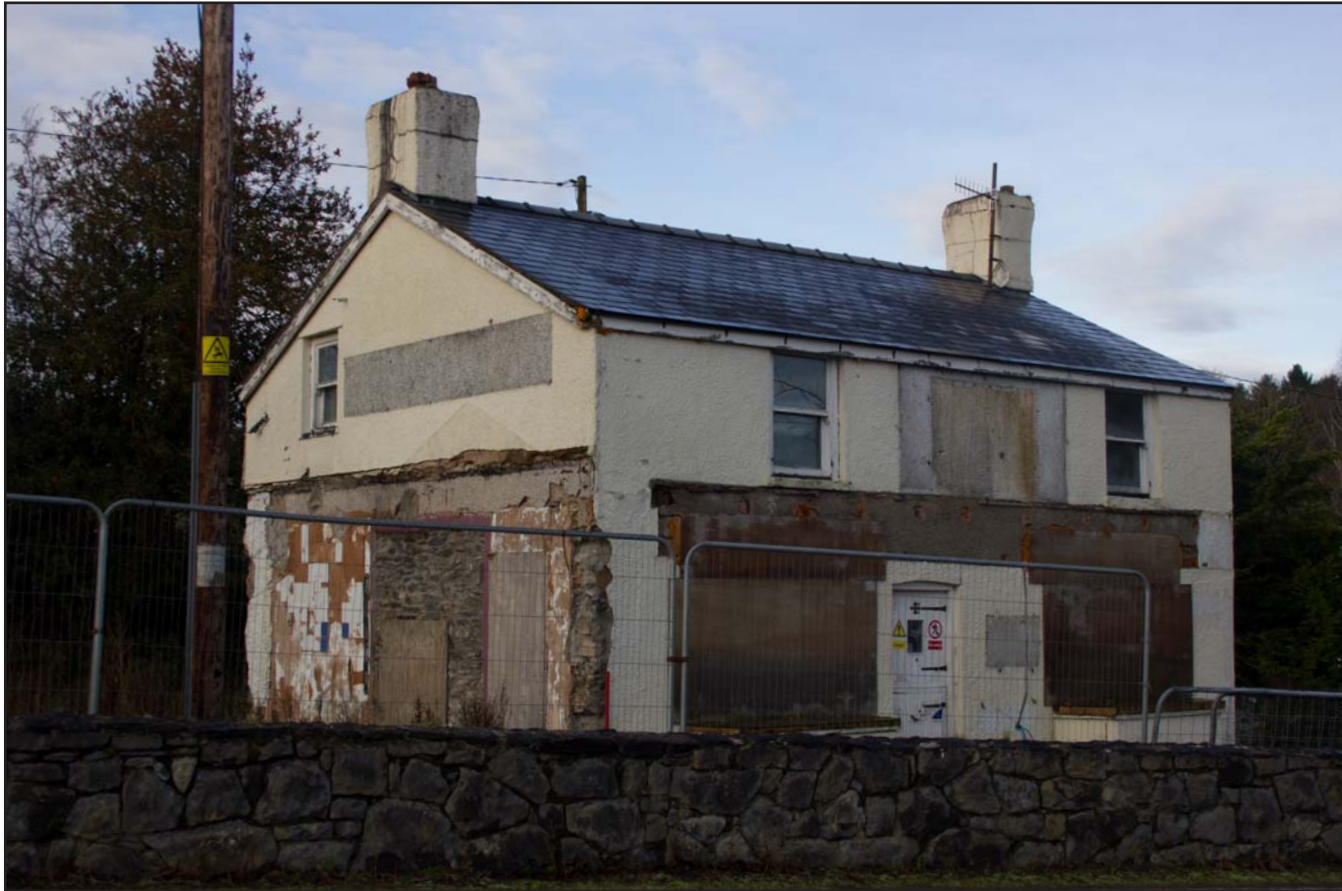
Plate 09: South and east facing external elevations, from the southeast. Scale 1.0m.
