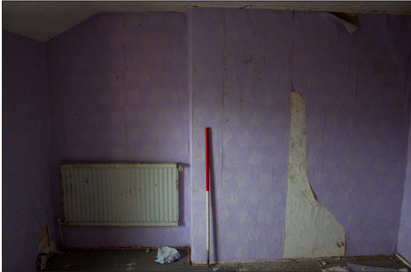
Plate 20: First Floor - Bedroom 2, from the north. Scale 1.0m.
