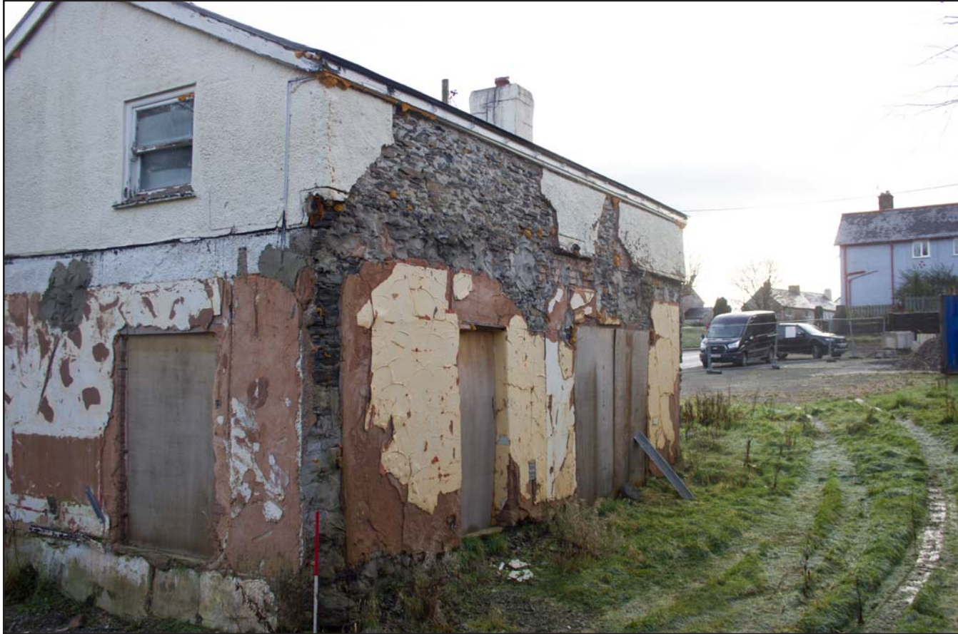
Plate 06: West facing external elevation, from the northwest. Scale 1.0m.
