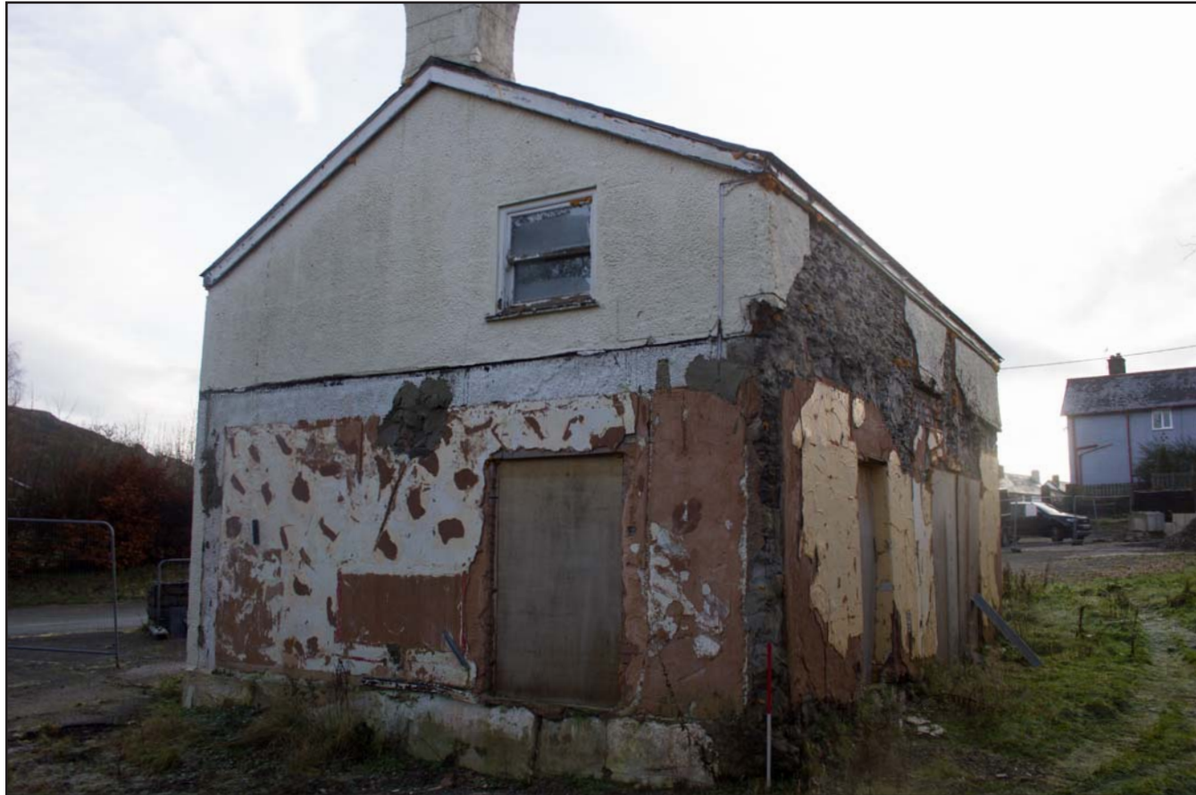
Plate 05: North and west facing external elevations, from the northwest. Scale 1.0m.
