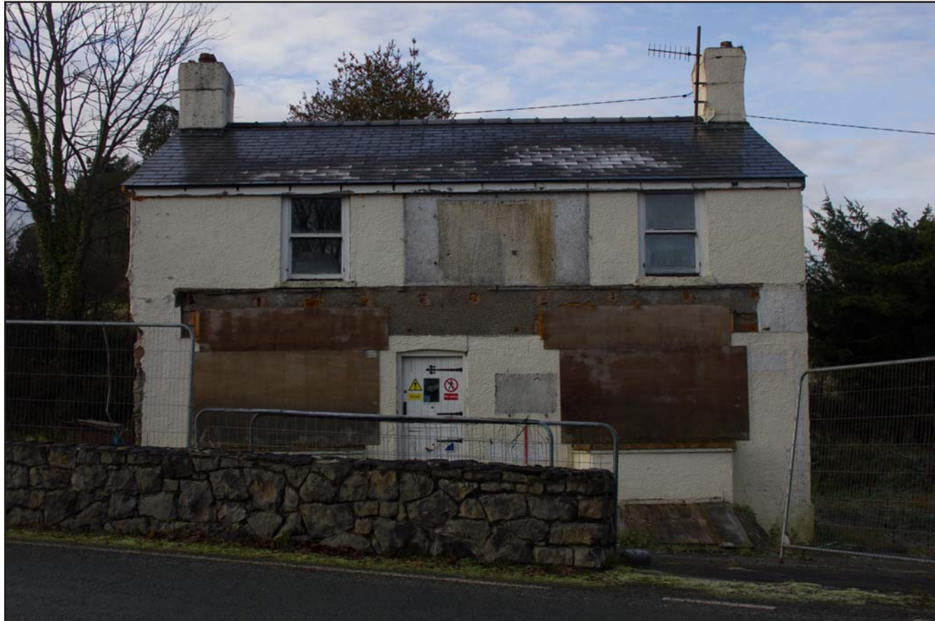
Plate 02: East facing external elevation, from the east. Scale 1.0m.
