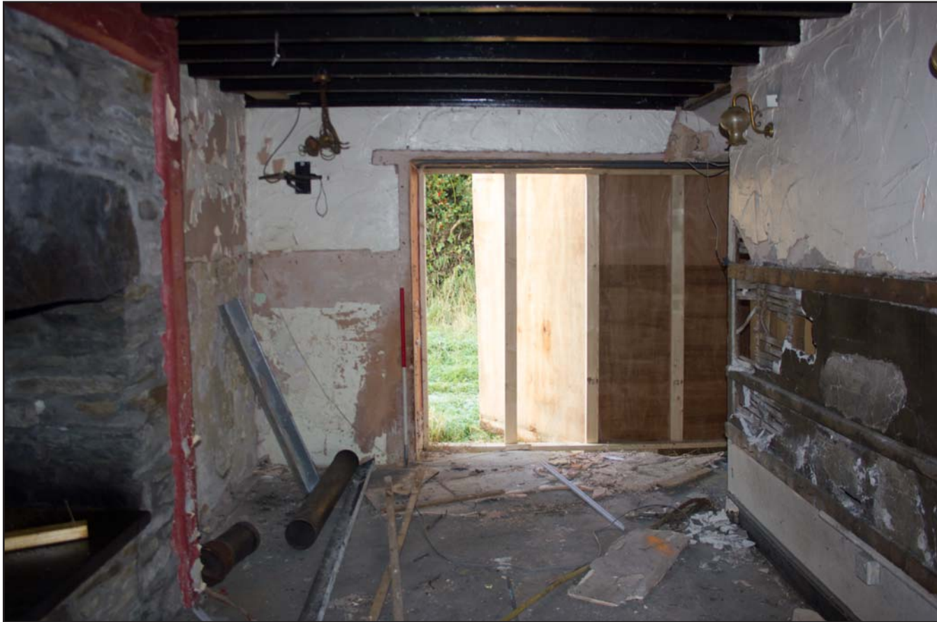
Plate 10: Ground Floor - Bar, from the east. Scale 1.0m.
