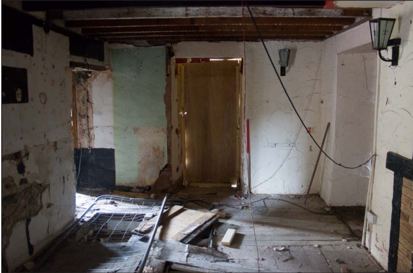
Plate 13: Ground Floor - Lounge, from the east. Scale 1.0m.
