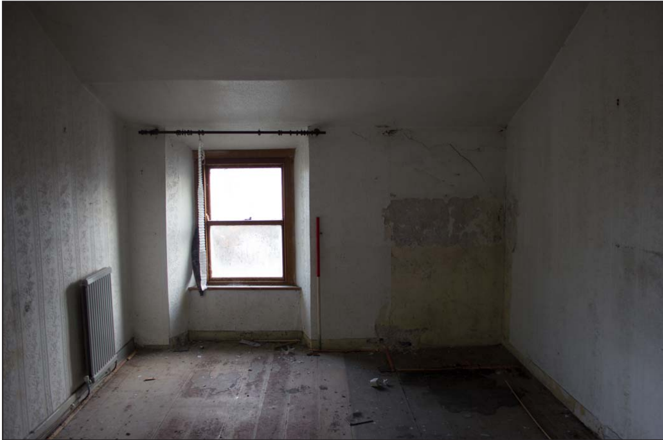
Plate 18: First Floor - Bedroom 1, from the west. Scale 1.0m.
