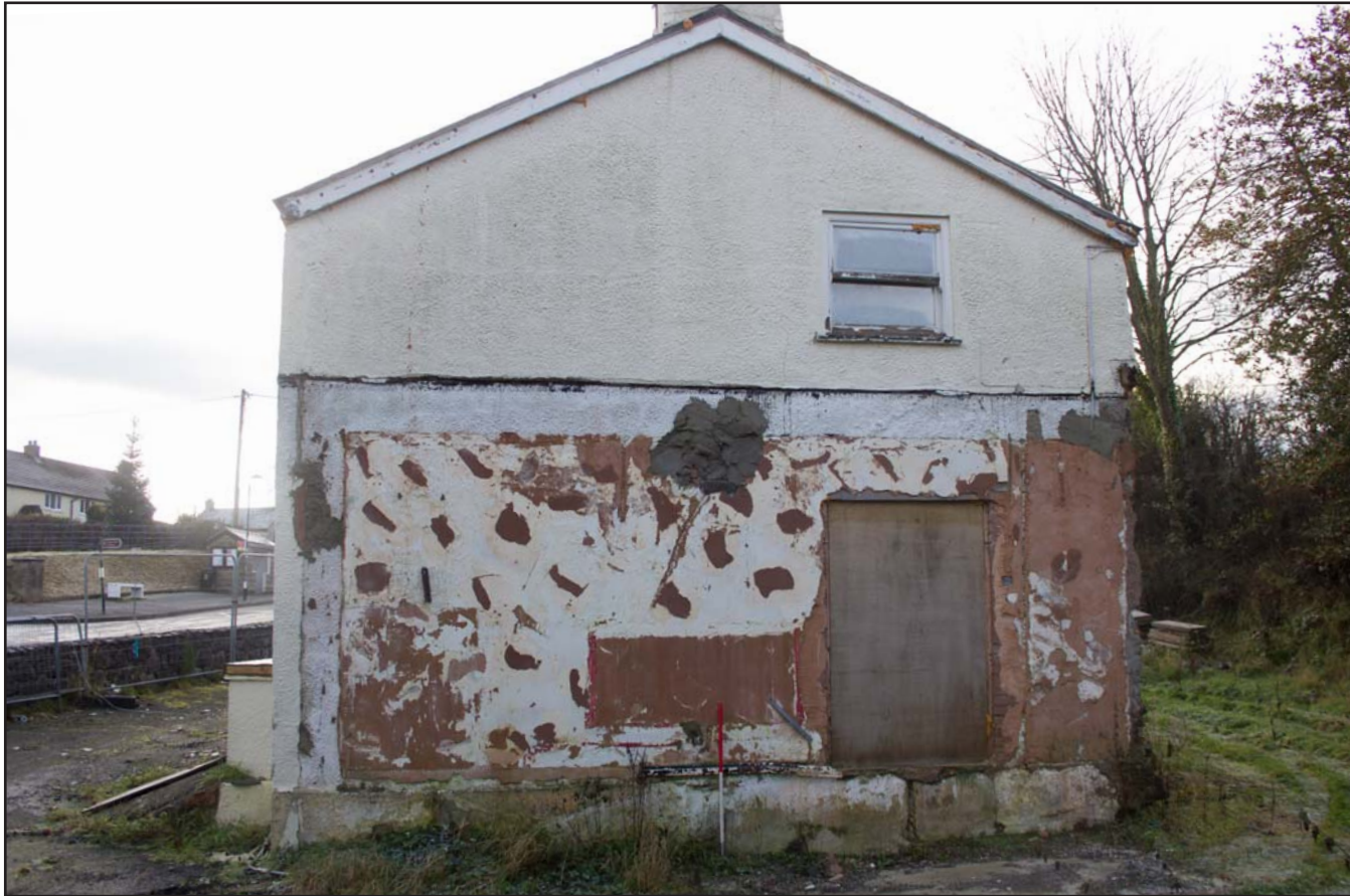
Plate 04: North facing external elevation, from the north. Scale 1.0m.
