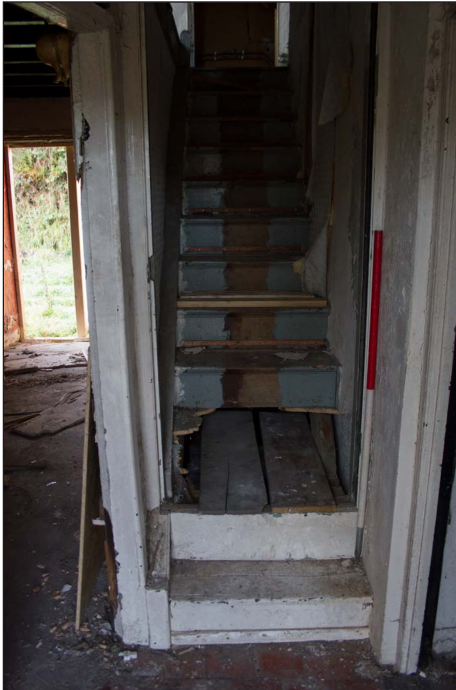
Plate 16: Ground floor - Staircase, from the east. Scale 1.0m.
