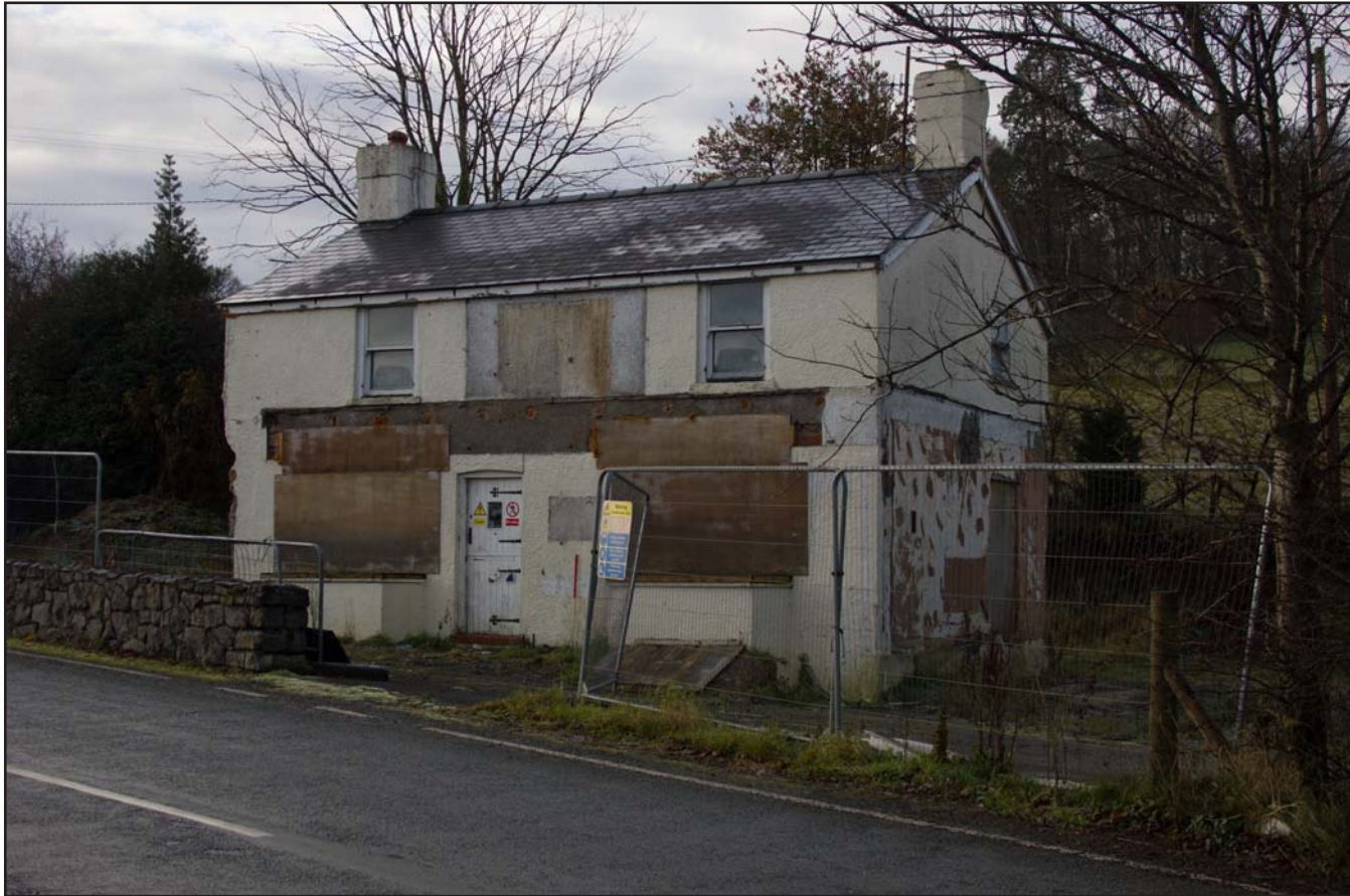
Plate 03: East and north facing external elevations, from the northeast. Scale 1.0m.
