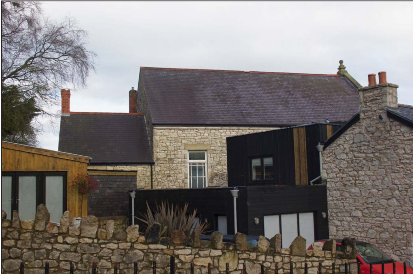
Plate 13: Shot showing eastern elevation (oblique) of Capel Carmel, Carmel Road, Carmel, Flintshire - from the southeast - 2.00m scale
