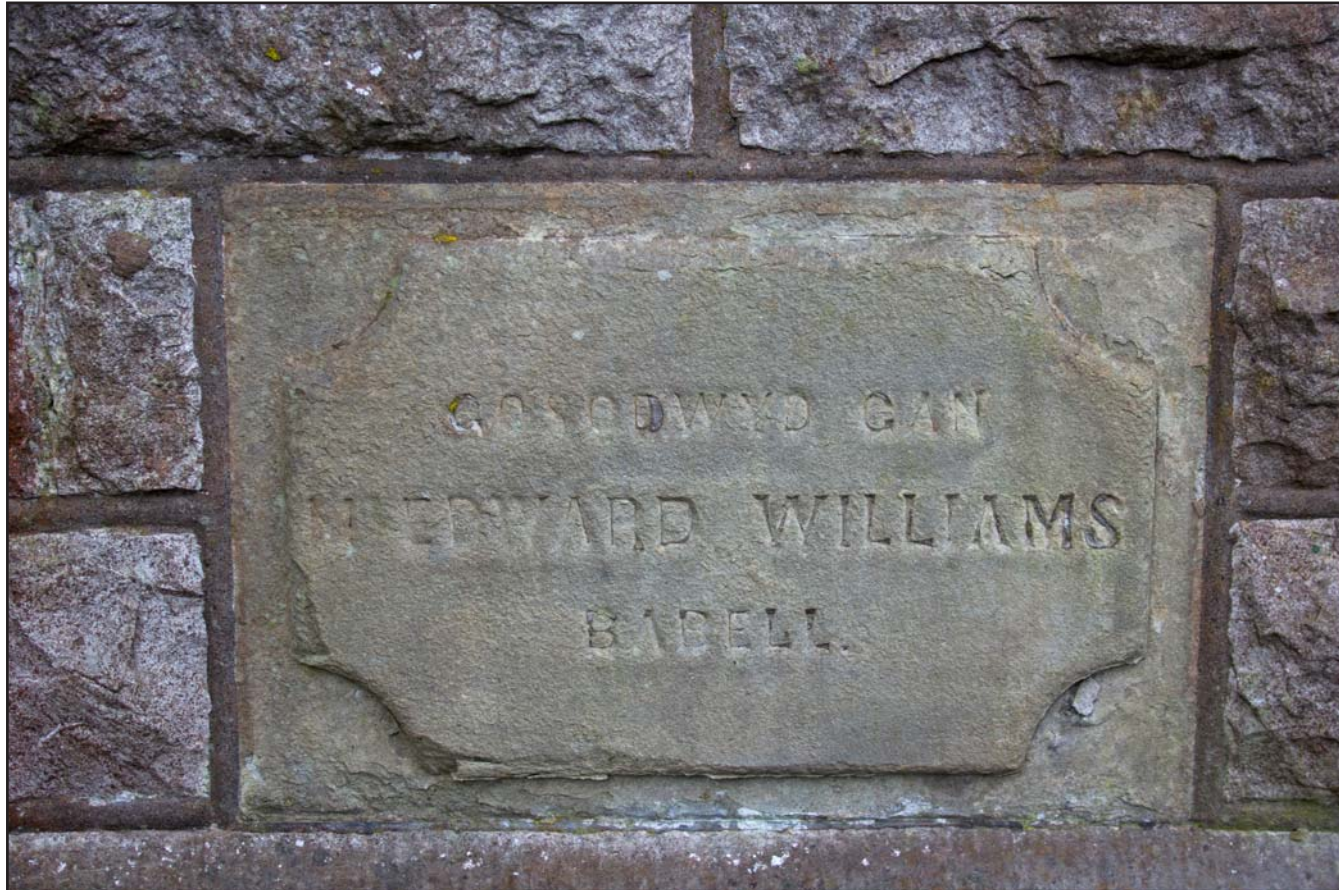
Plate 21: Commemorative stone reads "Gosodwyd Gan Richard Williams Babel" on lower portion (right side) of northern elevation of Capel Carmel, Carmel Road, Carmel, Flintshire - from the north - no scale
