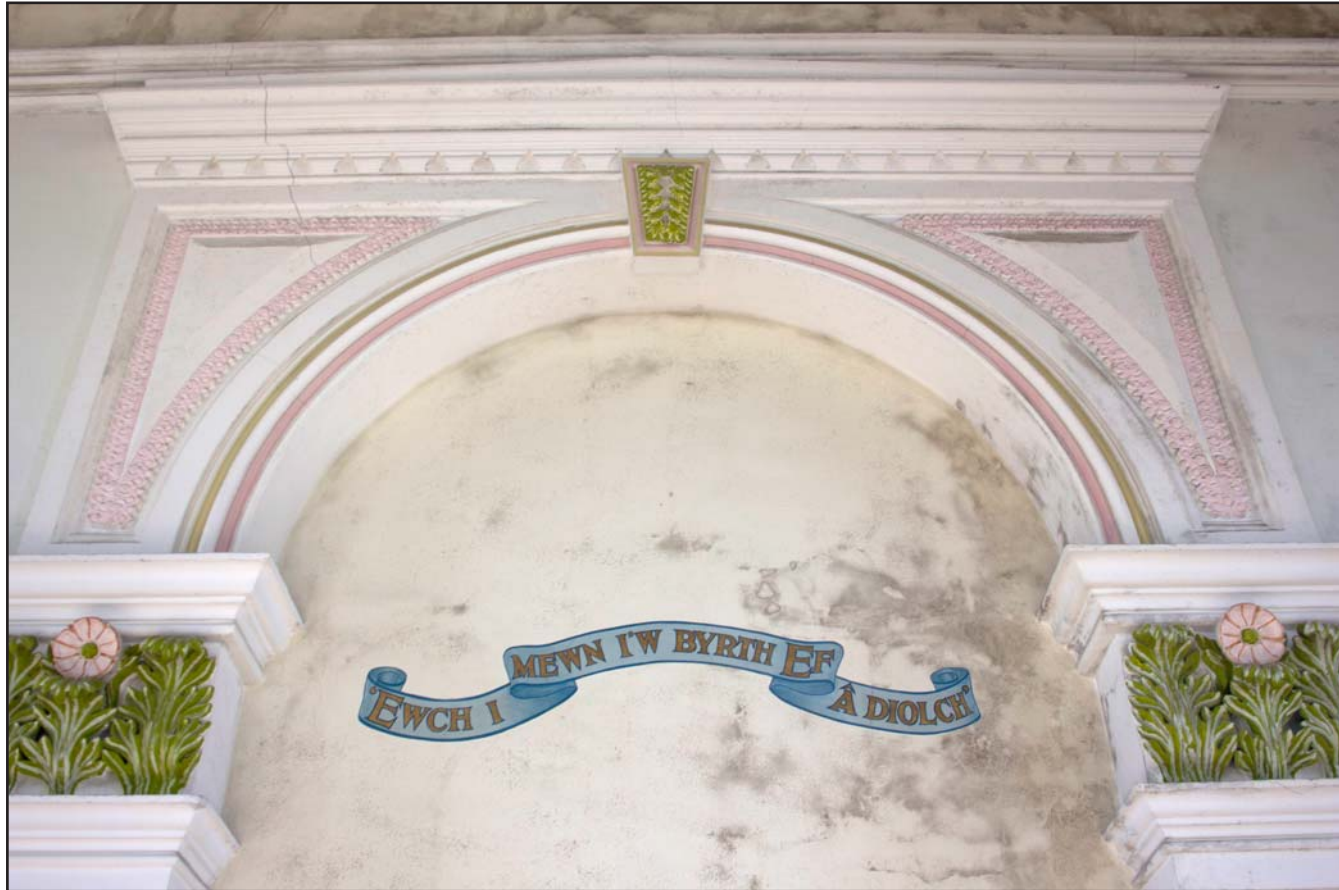
Plate 49: Central arch with extract from psalm 100 (BWM), internal shot, at Capel Carmel, Carmel Road, Carmel, Flintshire - from the north - 2.00m
