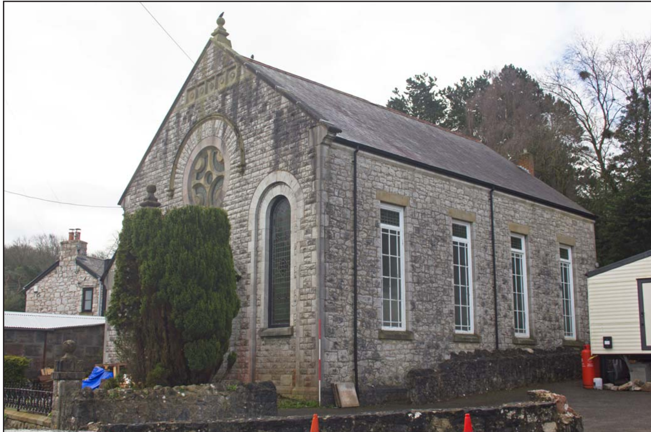
Plate 05: Oblique shot showing western and principal elevations of Capel Carmel, Carmel Road, Carmel, Flintshire - from the northwest - 2.00m scale
