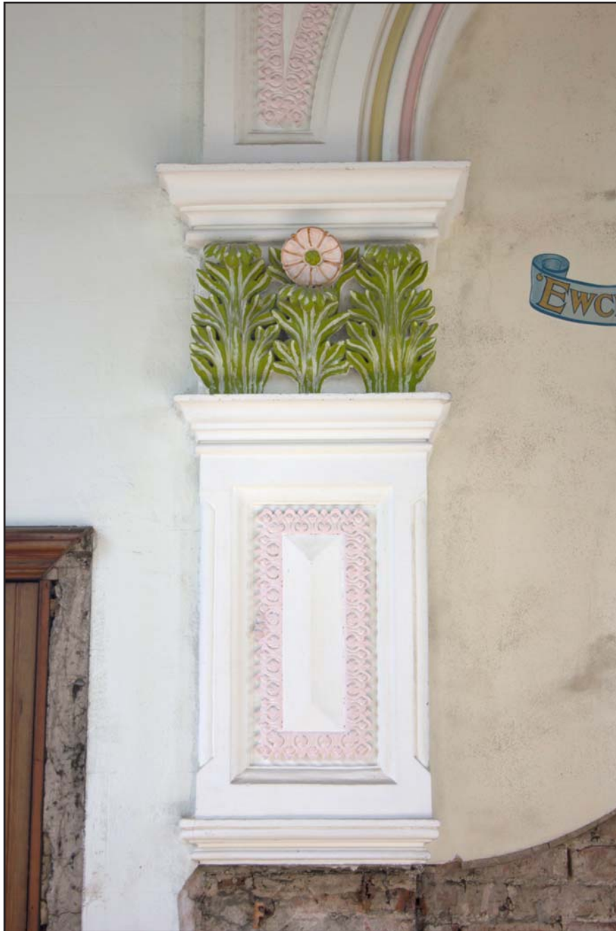
Plate 48: Decorative timber and plaster pillar (left), internal shot, at Capel Carmel, Carmel Road, Carmel, Flintshire - from the north - 2.00m
