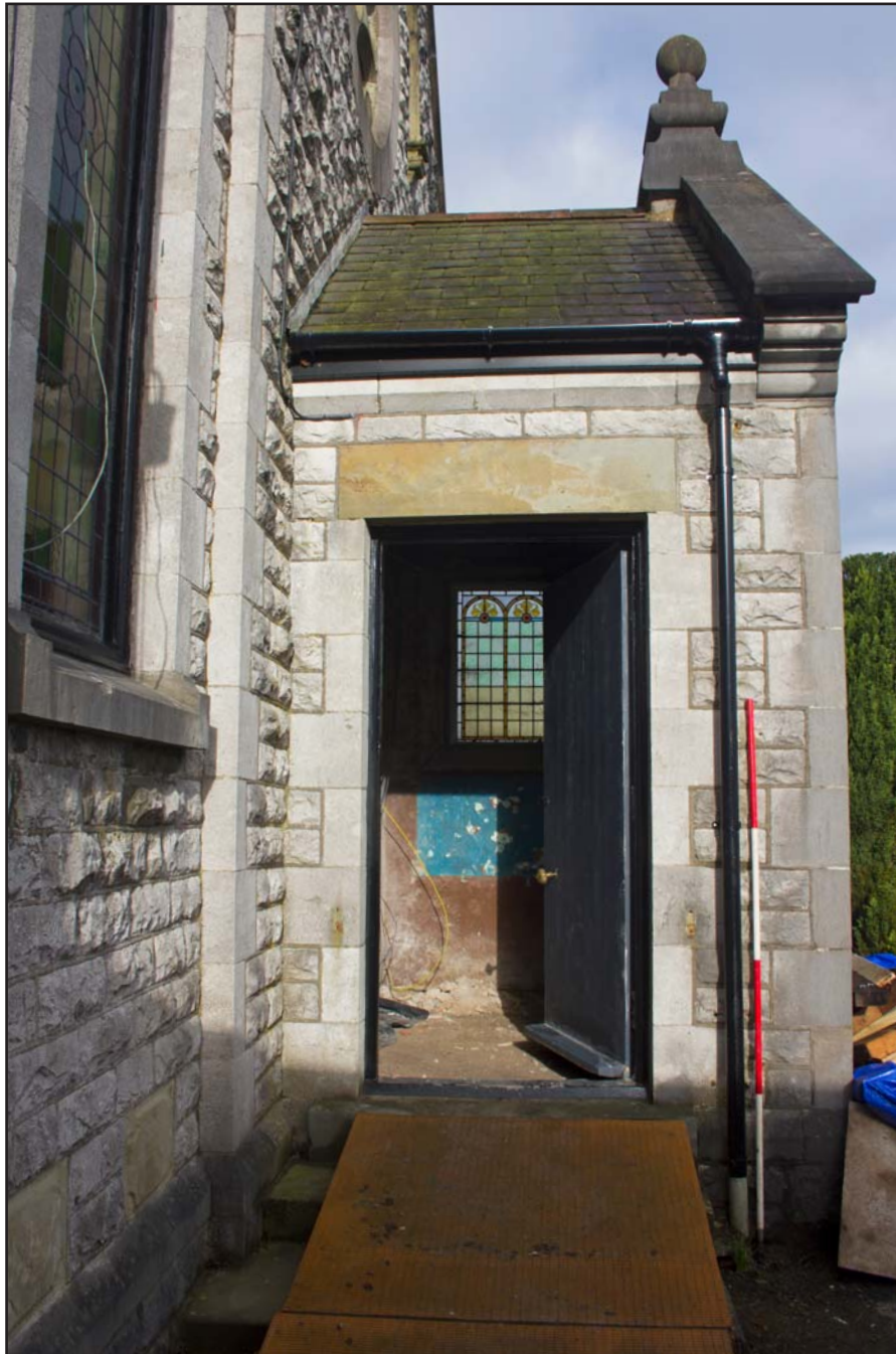
Plate 17: Shot of porch entry doorway of Capel Carmel, Carmel Road, Carmel, Flintshire - from the east - no scale
