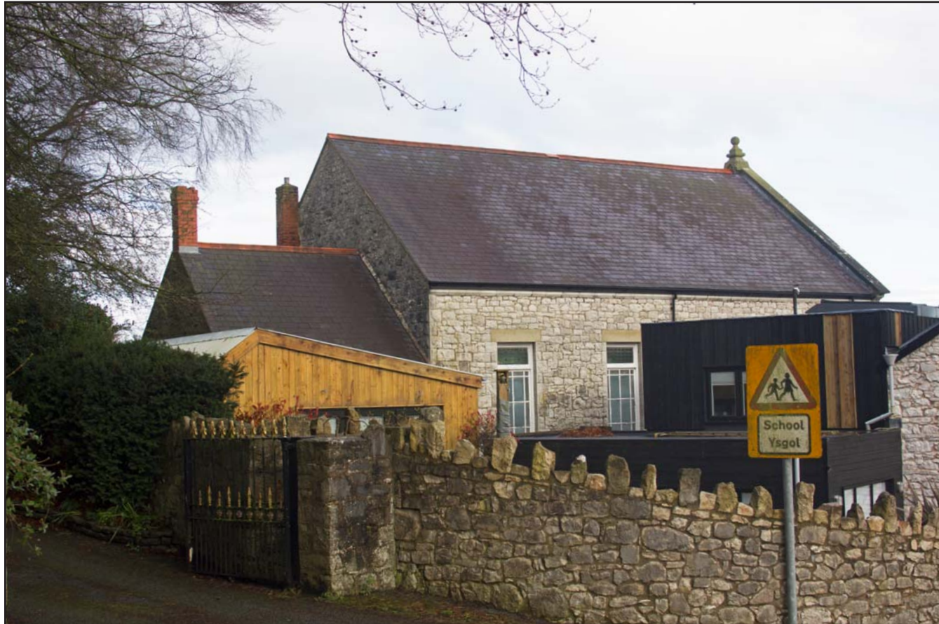
Plate 12: Oblique shot showing southern and eastern elevations of Capel Carmel, Carmel Road, Carmel, Flintshire - from the southeast - no scale
