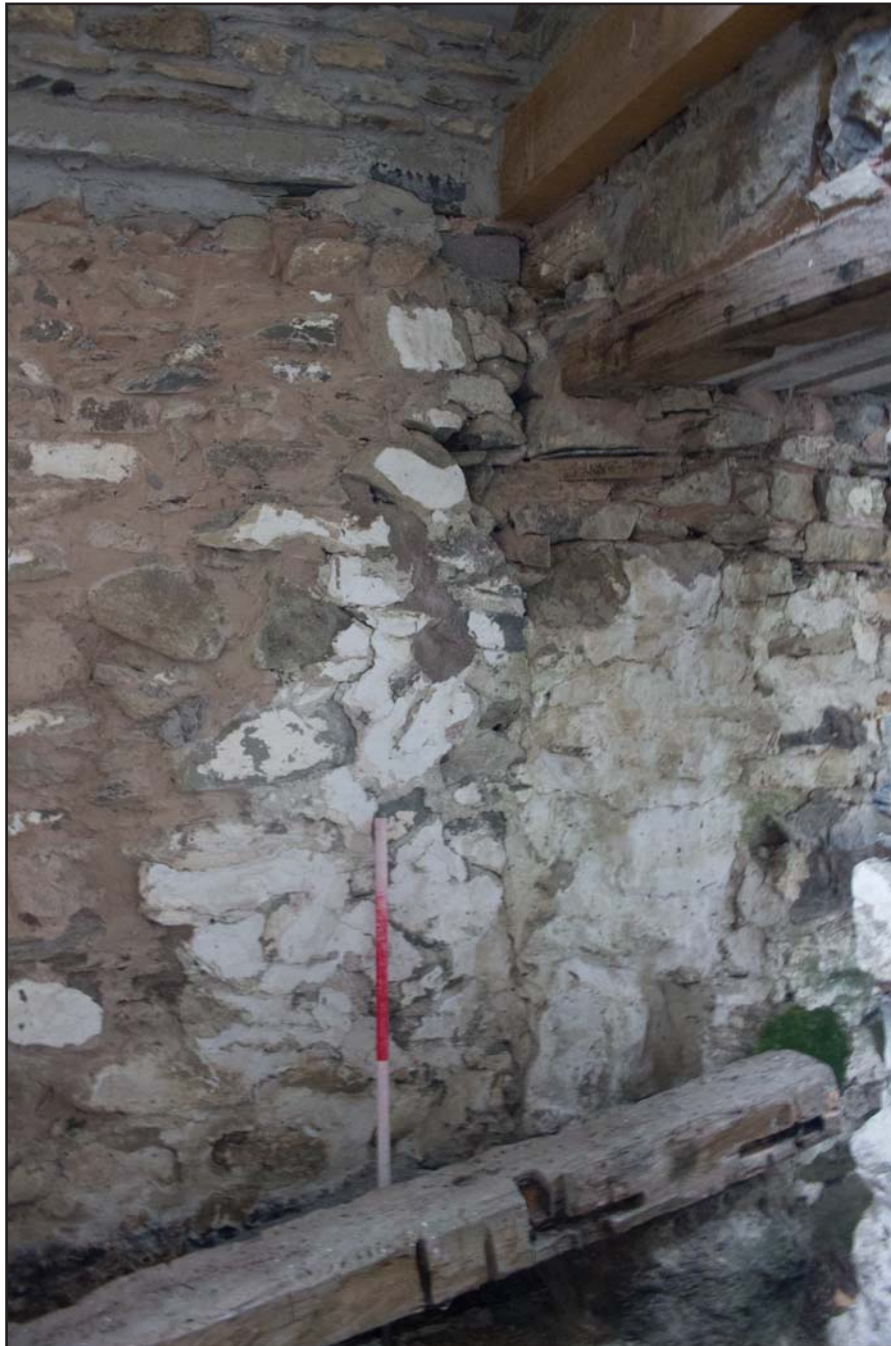
Plate 36: Internal shot, northwest wall (secondary phase room) abuts with former gable (Primary), of the post medieval farmhouse at Penrhyn Garn, Rhydlydan, Pentrefeolas, Conwy - from the south - 1.00m scale
