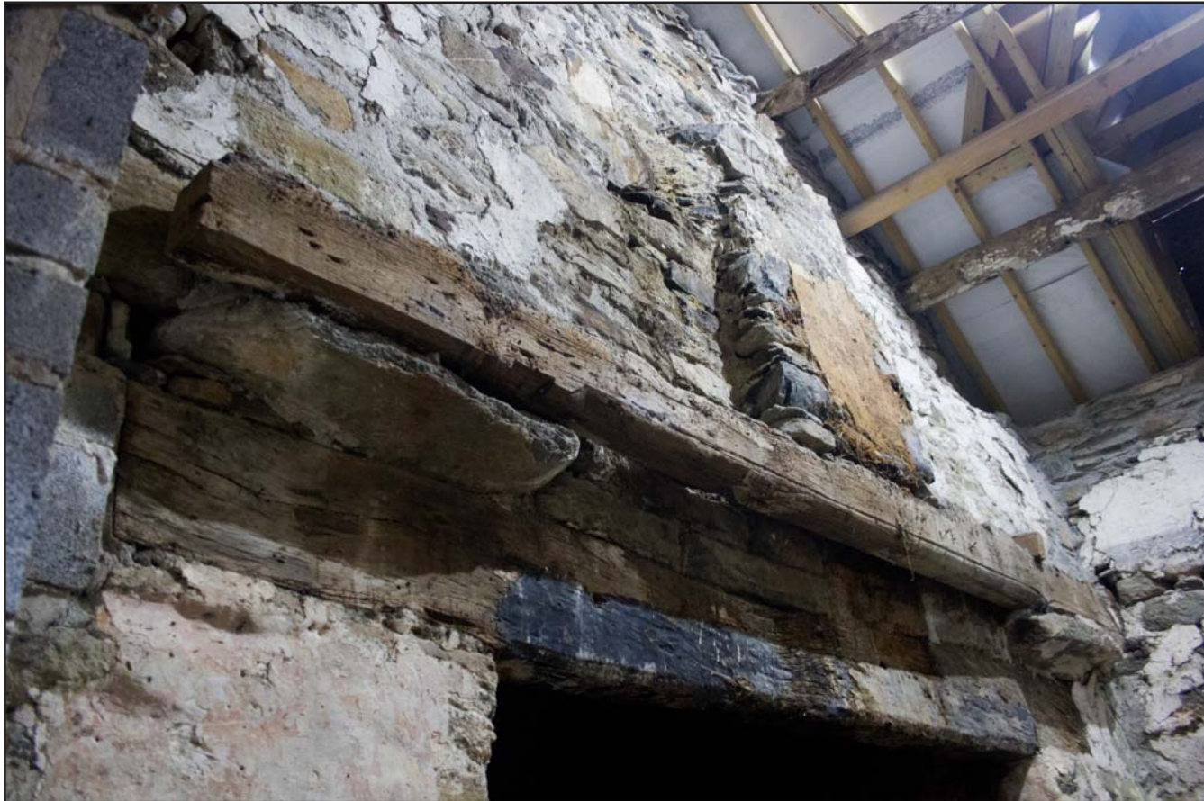
Plate 27: Internal shot, Bressumer Beam, transverse beam with Ovolo Moulding showing stone corbels, First floor fireplace (Primary phase room) of the post medieval farmhouse at Penrhyn Garn, Rhydlydan, Pentrefeolas, Conwy - from the west - no scale
