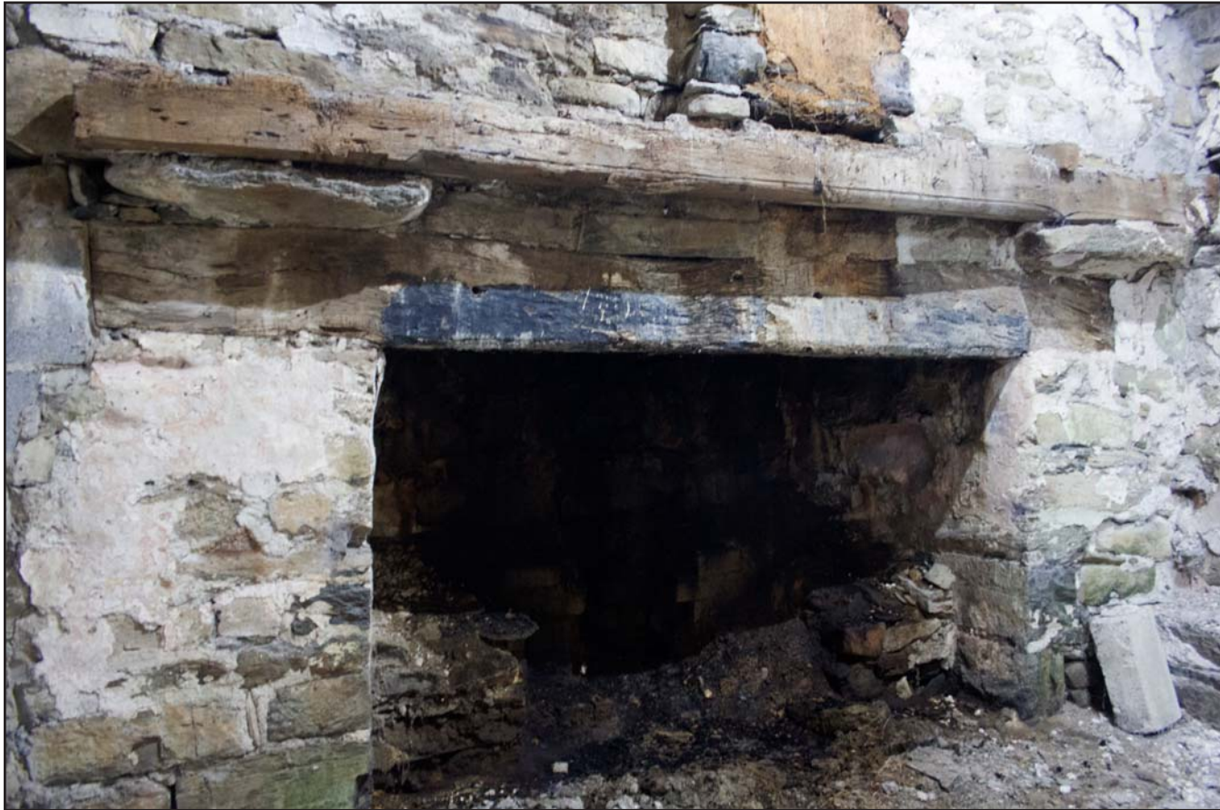
Plate 26: Internal oblique shot, Bressumer Beam, transverse beam with Ovolo Moulding showing stone corbels (Primary phase room) of the post medieval farmhouse at Penrhyn Garn, Rhydlydan, Pentrefeolas, Conwy - from the west - no scale
