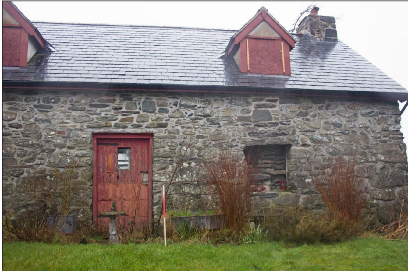
Plate 05: Southeast elevation (right) of the post medieval farmhouse at Penrhyn Garn, Rhydlydan, Pentrefeolas, Conwy - from the southeast - 1.00m scale
