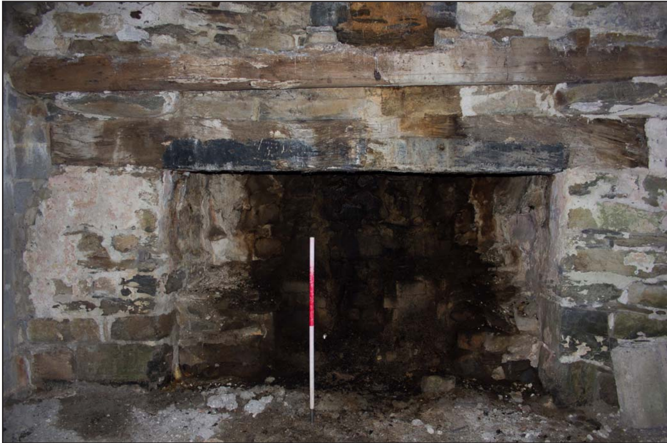
Plate 25: Internal shot, Fireplace with Bressumer Beam, (Primary phase room) of the post medieval farmhouse at Penrhyn Garn, Rhydlydan, Pentrefeolas, Conwy - from the southwest - 1.00m scale
