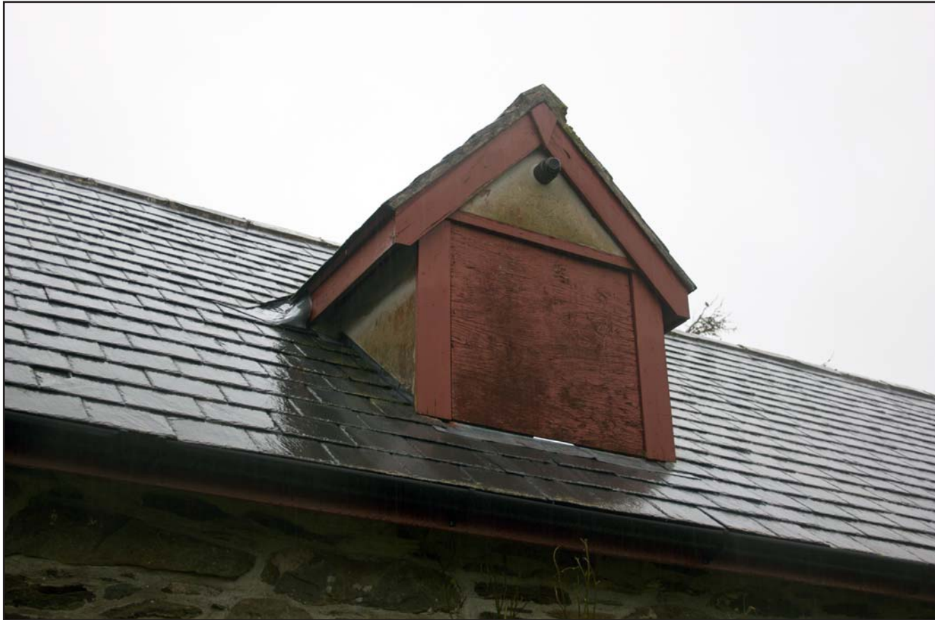
Plate 04: Modern gable fronted dormer in modern roof construction at of the post medieval farmhouse at Penrhyn Garn, Rhydlydan, Pentrefeolas, Conwy - from the south - no scale
