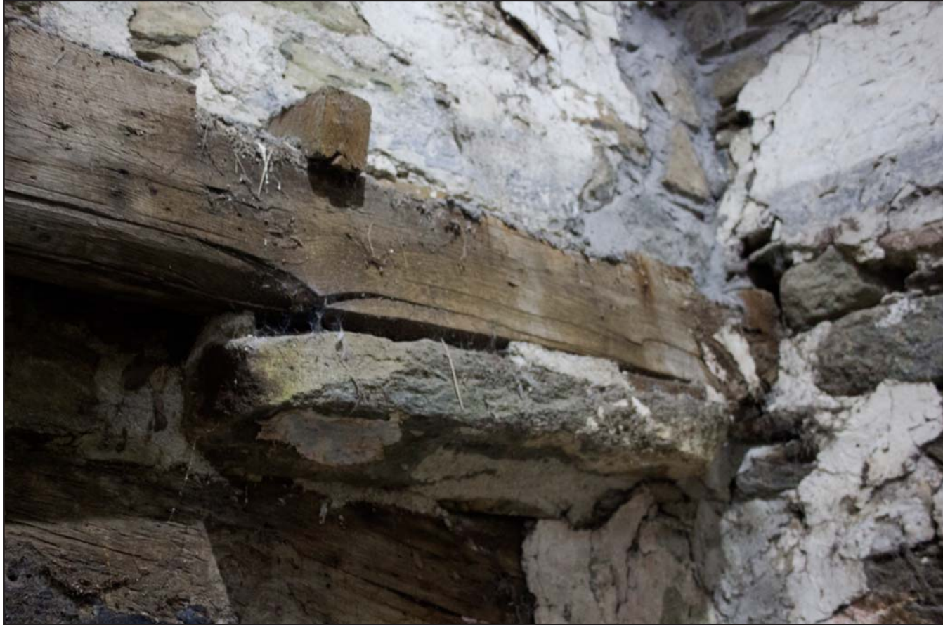
Plate 29: Internal shot, stone corbel (right) supporting Ovolo moulded transverse beam (Primary phase room) of the post medieval farmhouse at Penrhyn Garn, Rhydydan, Pentrefeolas, Conwy - from the east - no scale
