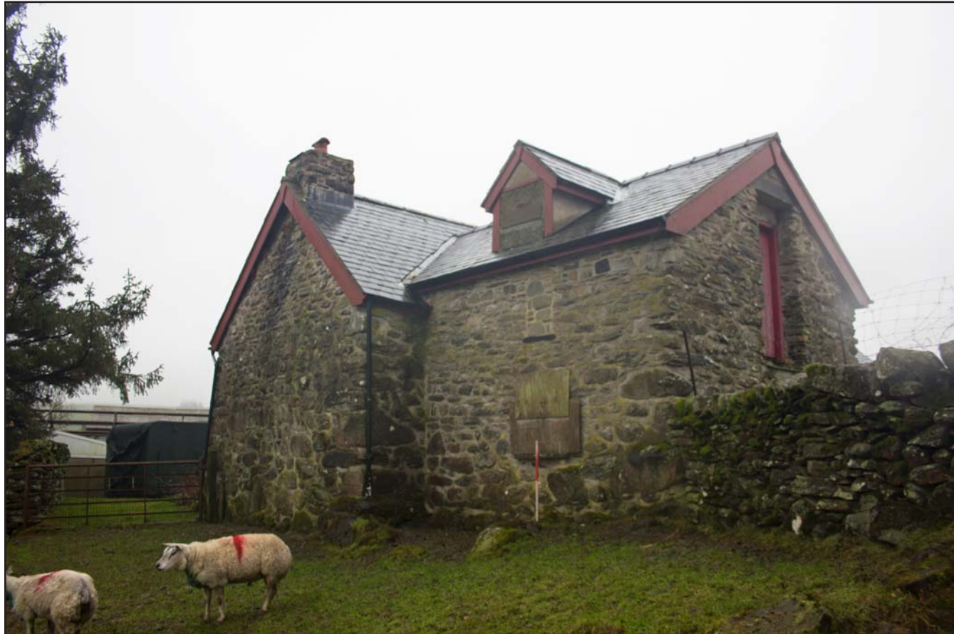
Plate 11: Northeast and southeast elevations (oblique) of the post medieval farmhouse at Penrhyn Garn, Rhydlydan, Pentrefeolas, Conwy - from the north - 1.00m scale
