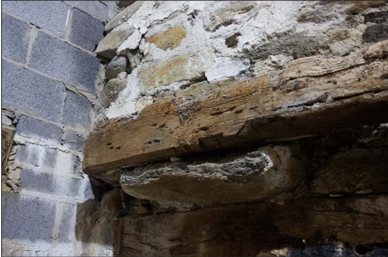
Plate 30: Internal shot, stone corbel (left) supporting Ovolo moulded transverse beam (Primary phase room) of the post medieval farmhouse at Penrhyn Garn, Rhydlydan, Pentrefeolas, Conwy - from the east - no scale
