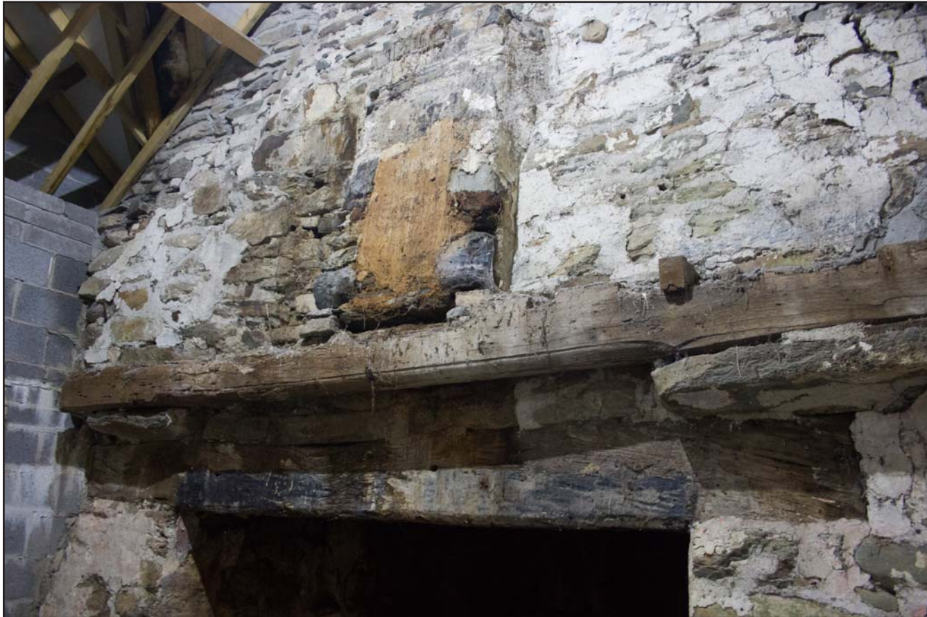
Plate 28: Internal shot, Bressumer Beam, transverse beam with Ovolo Moulding showing stone corbels, First floor fireplace (Primary phase room) of the post medieval farmhouse at Penrhyn Garn, Rhydlydan, Pentrefeolas, Conwy - from the south - no scale
