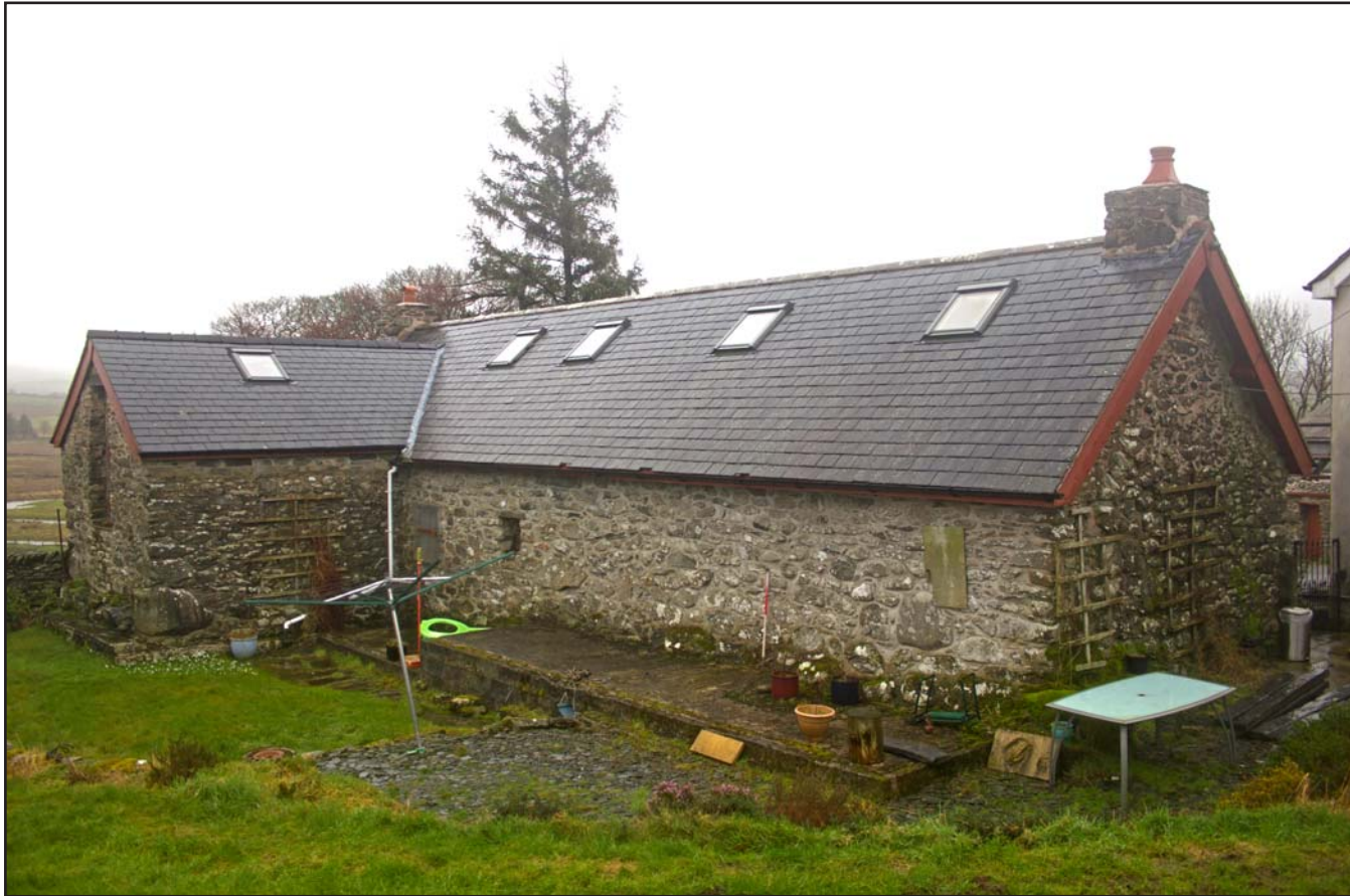
Plate 18: Northwest and southwest elevations (oblique) of the post medieval farmhouse at Penrhyn Garn, Rhydlydan, Pentrefeolas, Conwy - from the west - 1.00m scale
