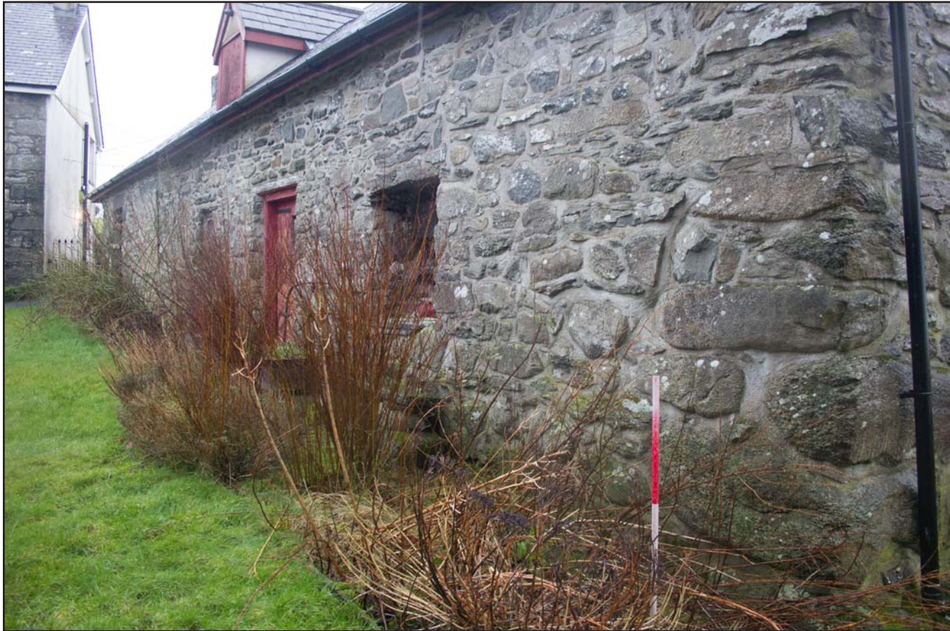
Plate 08: Southeast elevation (oblique) of the post medieval farmhouse at Penrhyn Garn, Rhydlydan, Pentrefeolas, Conwy - from the east - 1.00m scale
