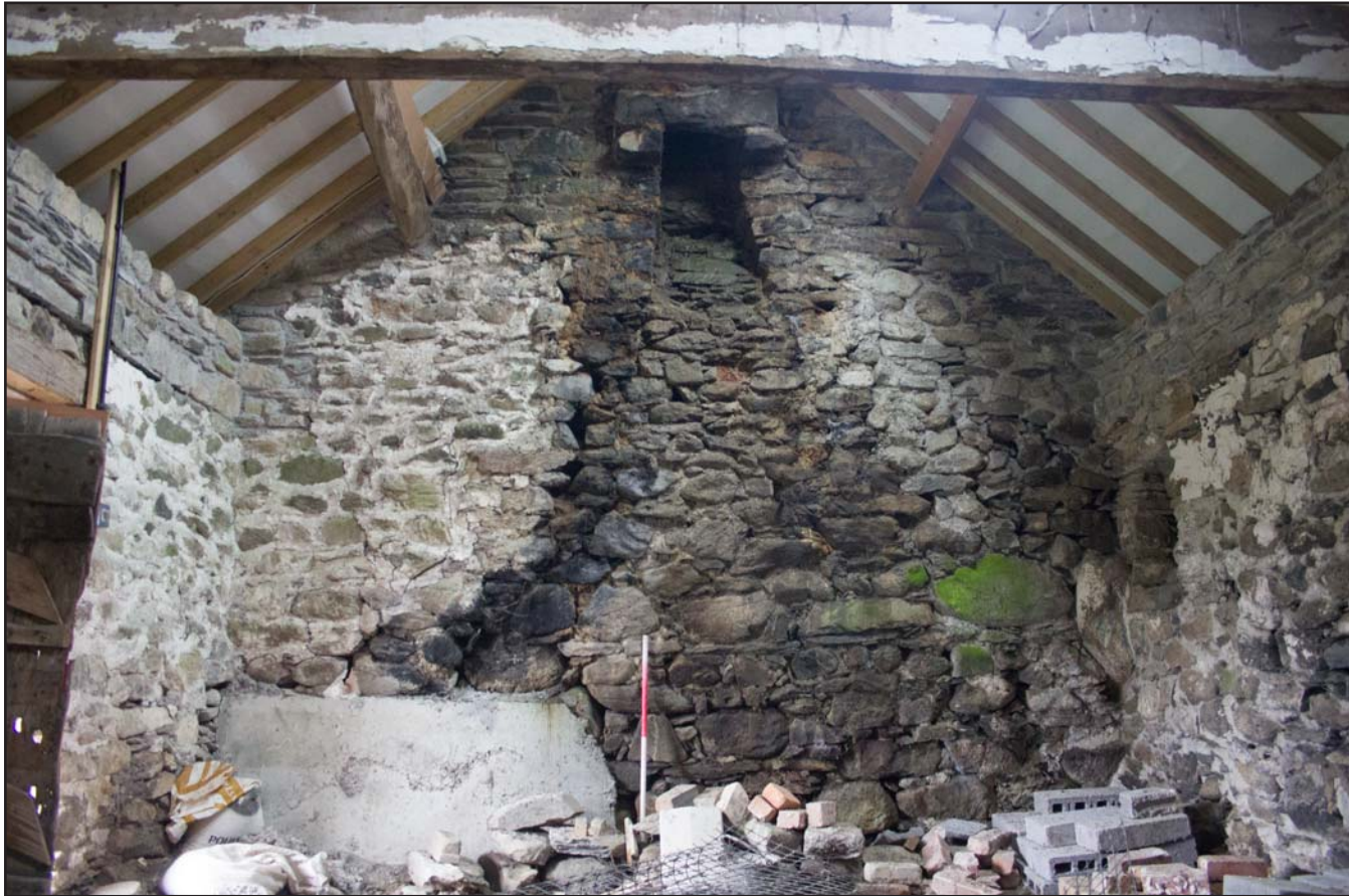
Plate 33: Internal shot, southwest elevation, (secondary, southwest extension), location of former chimney, within the post medieval farmhouse at Penrhyn Garn, Rhydlydan, Pentrefeolas, Conwy - from the northeast - 1.00m scale
