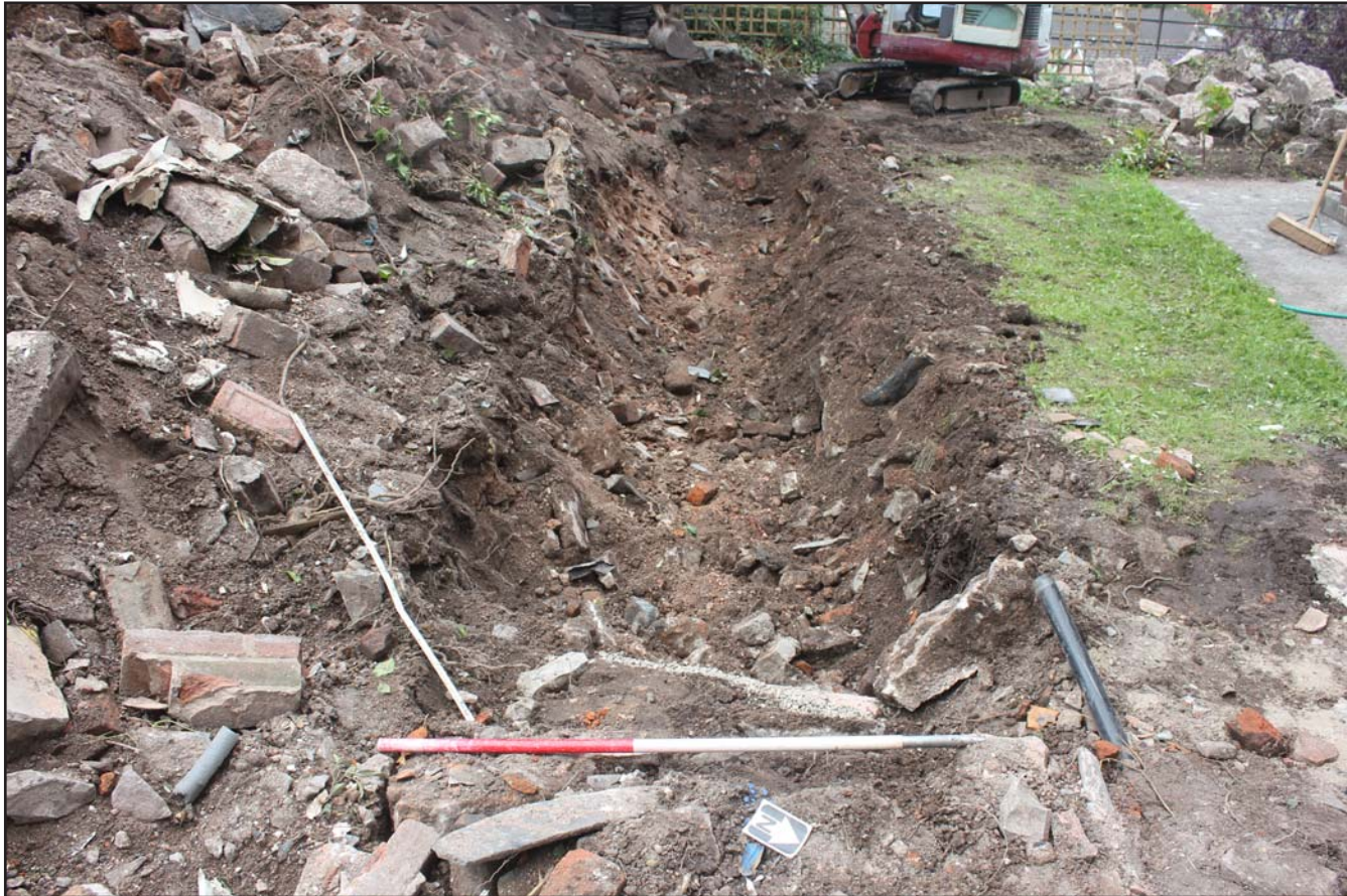
Plate 06: Post excavation shot of trench, on land at Crannog, Prior Street, Ruthin, Denbighshire - from the east - 1.00m scale
