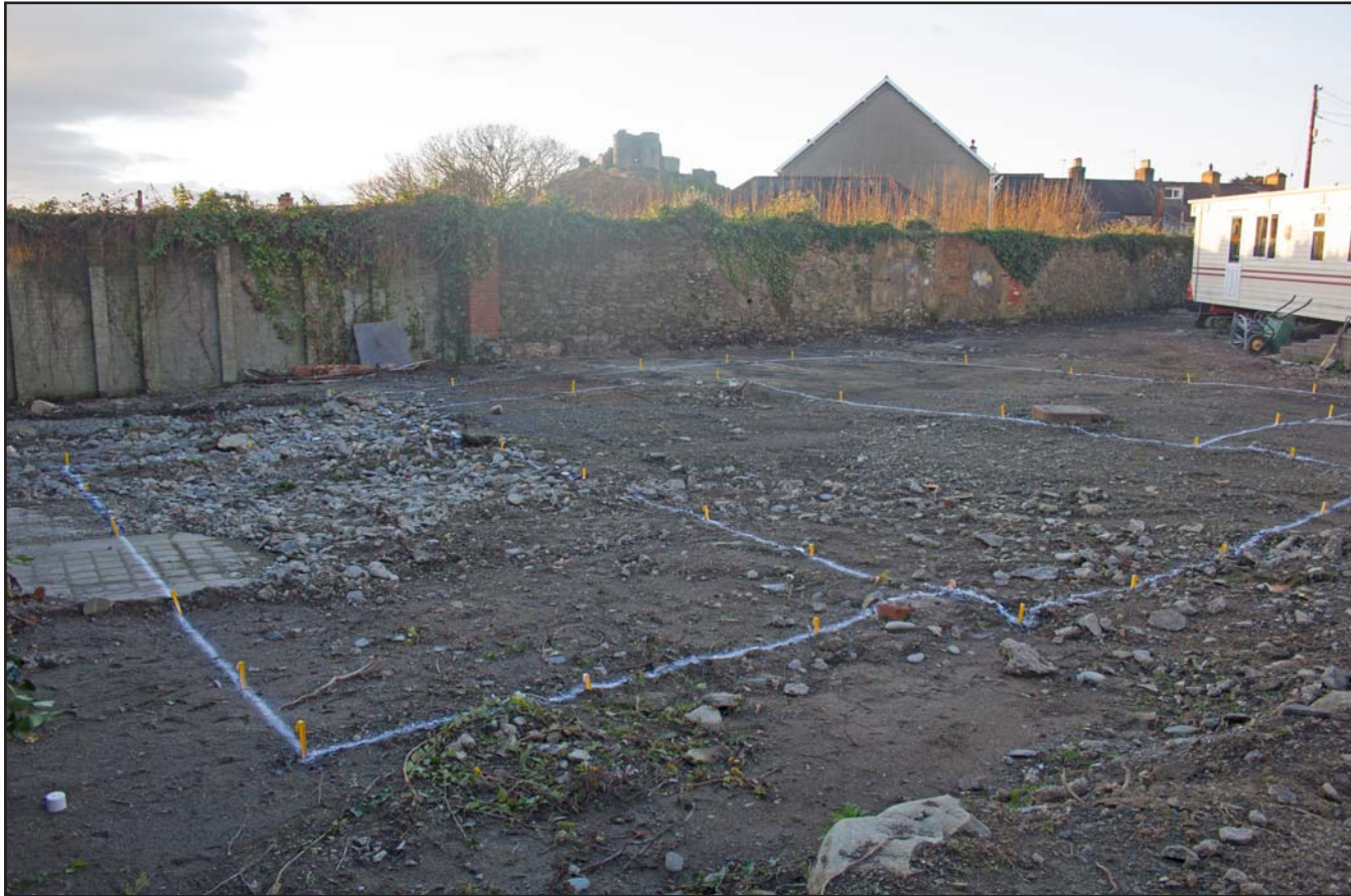
Plate 05: Pre excavation shot of site, Former Prince of Wales Car Park, High Street, Criccieth - from the northeast - 2.00m scale
