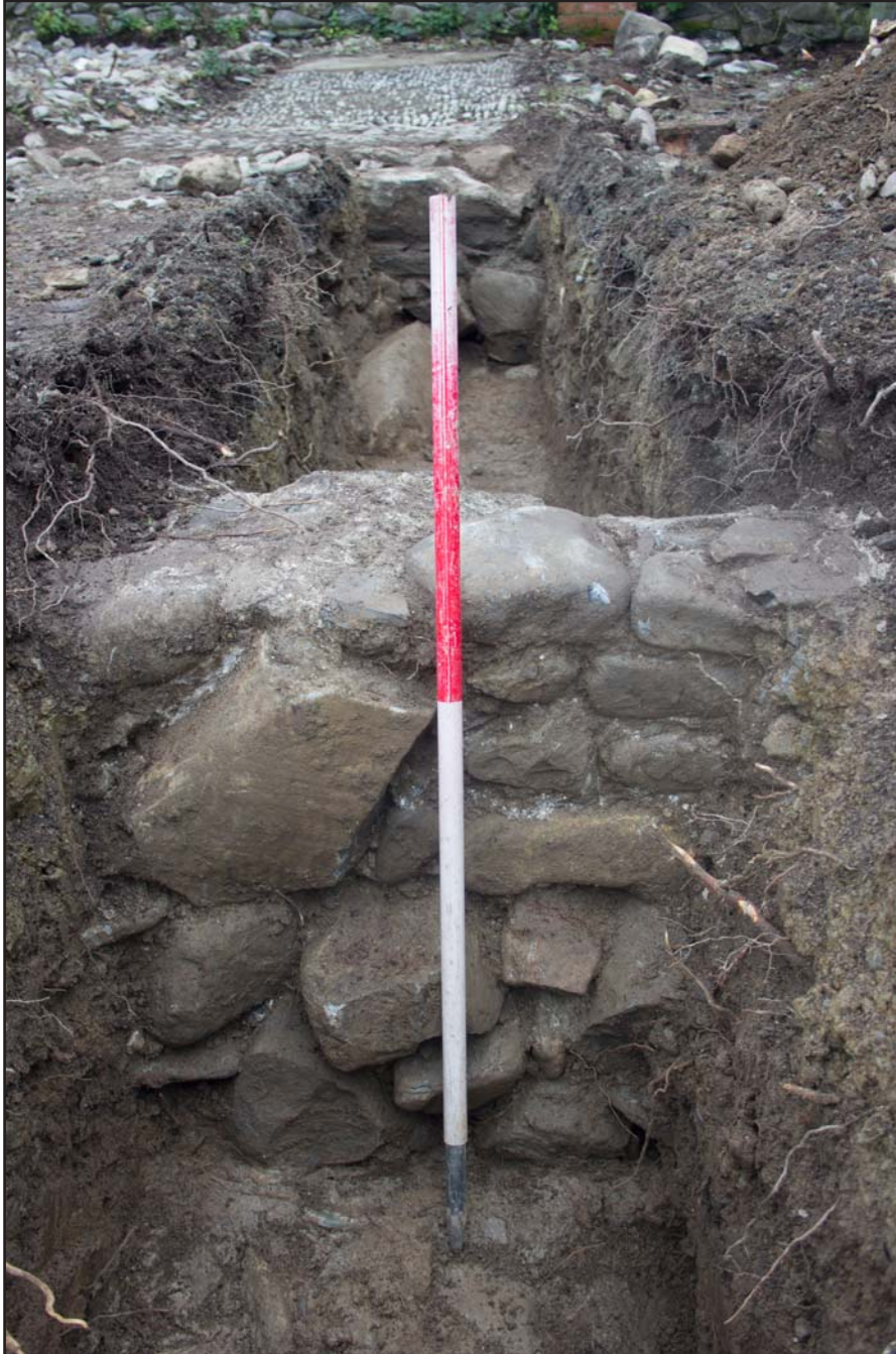
Plate 14: Wall foundation (1003) elevation shot, at Former Prince of Wales Car Park, High Street, Criccieth - from the west - 1.00m scale
