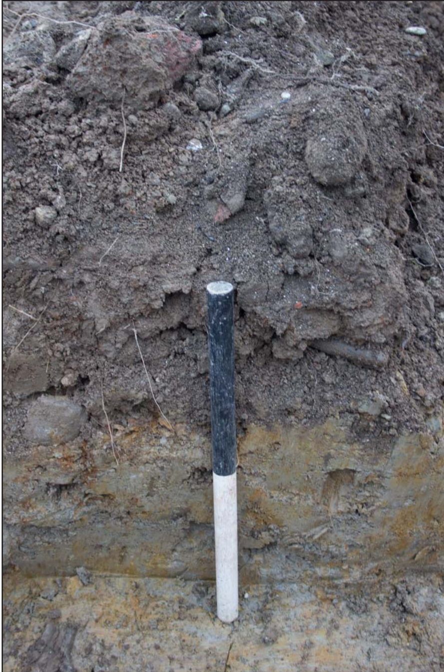
Plate 34: Trench D section shot, at Former Prince of Wales Car Park, High Street, Criccieth - from the south - 0.50m scale
