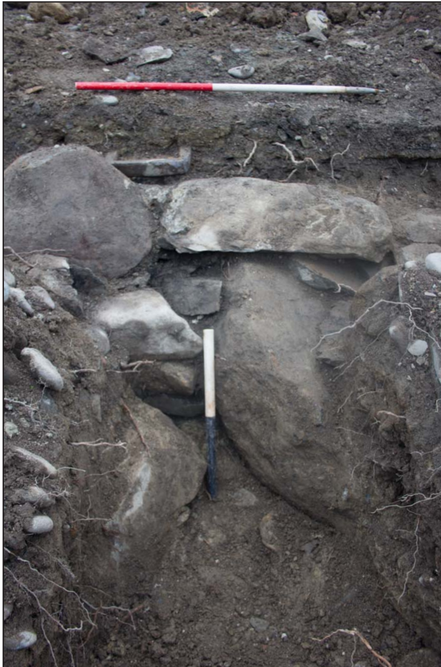
Plate 24: Wall foundation (1002) in elevation (centre), at Former Prince of Wales Car Park, High Street, Criccieth - from the south - 1.00m scale
