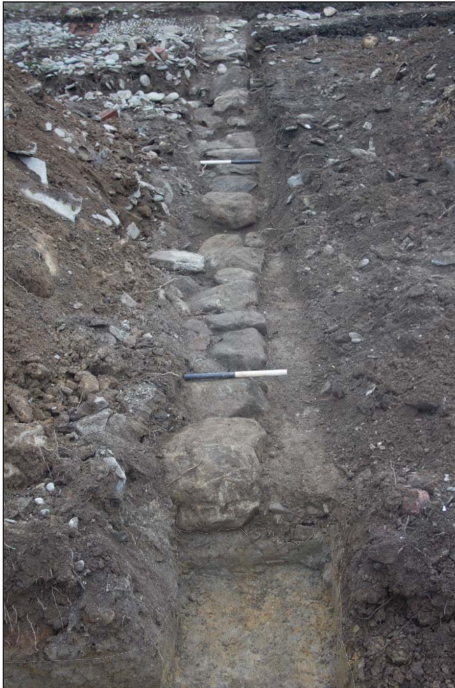
Plate 20: Wall foundation (1002) in plan, at Former Prince of Wales Car Park, High Street, Crickieth - from the north - (2x) 0.50m scale
