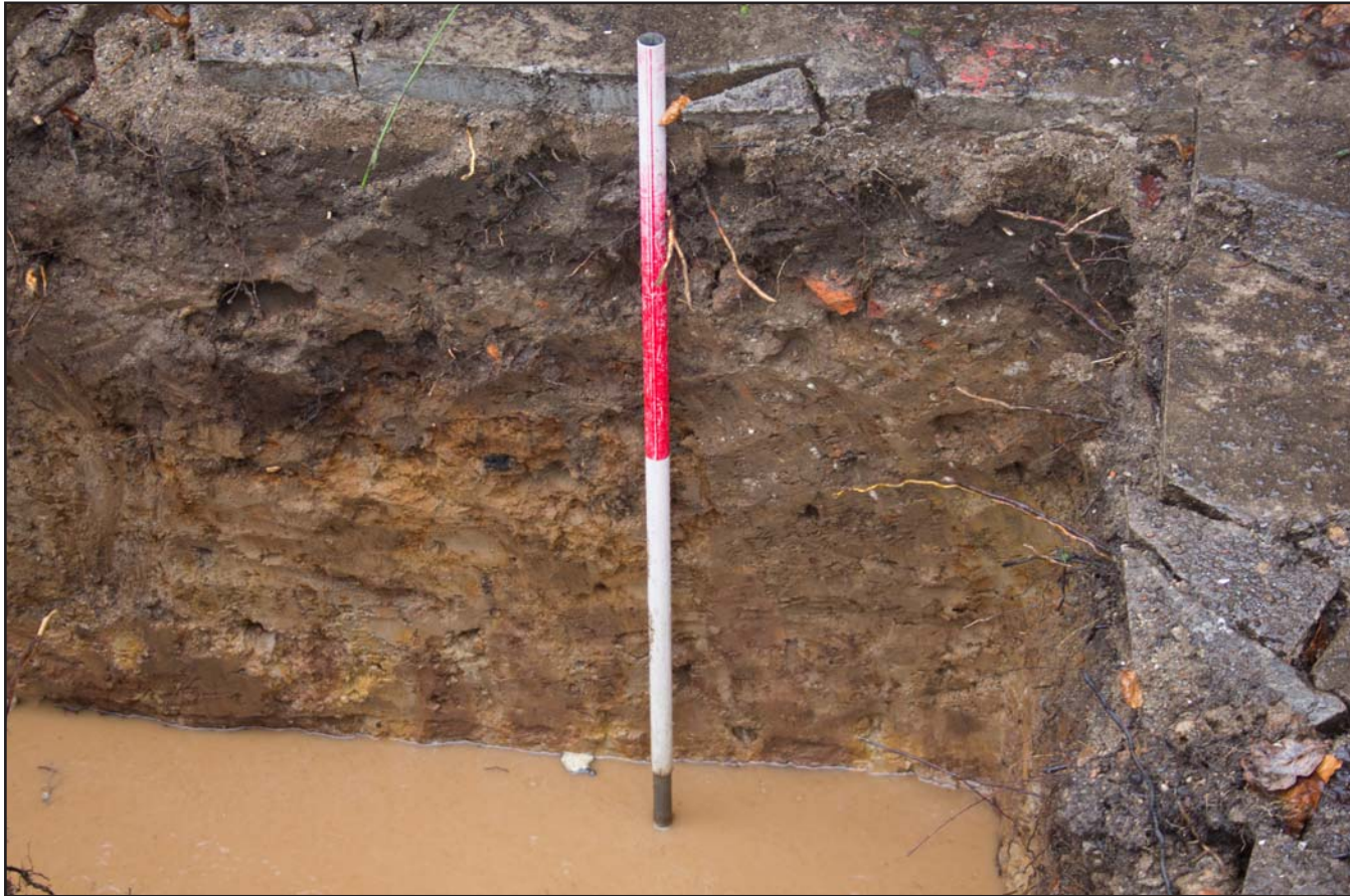
Plate 14: Section of north western trench (rear extension), at no 4. Oaklands Avenue, Rhosnesney, Wrexham - from the southeast - 1.00m scale
