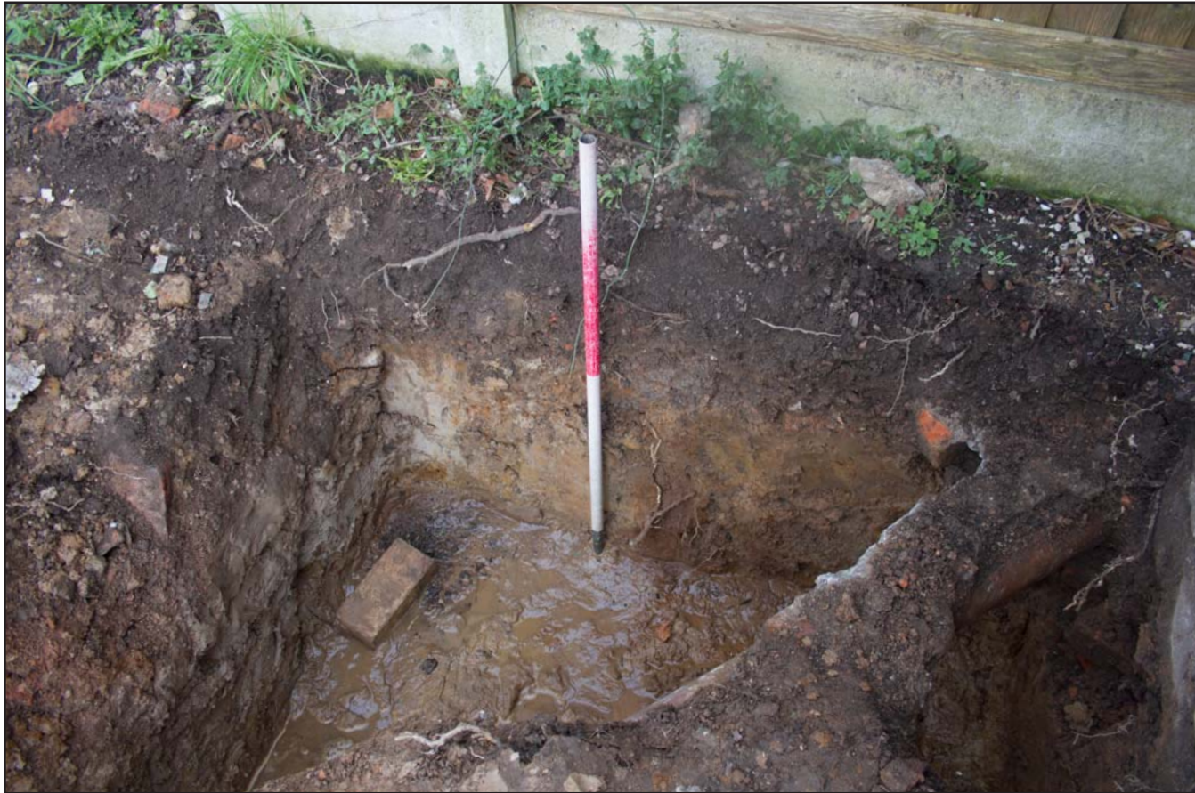
Plate 07: Section of SW trench (front extension), at no 4. Oaklands Avenue, Rhosnesney, Wrexham - from the northeast - 1.00m scale
