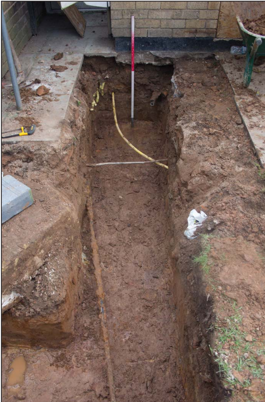
Plate 05: Post excavation shot of NE trench (front extension), at no 4. Oaklands Avenue, Rhosnesney, Wrexham - from the southeast - 1.00m scale
