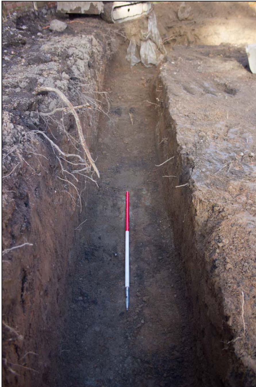
Plate 05: Rear extension western N-S trench, from the south. Scale 1.0m.
