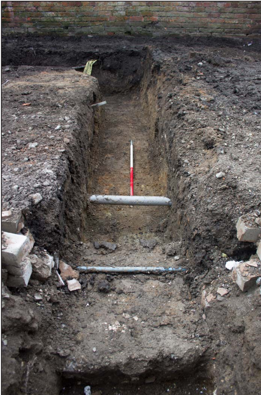
Plate 13: Front extension western N-S trench, from the north. Scale 1.0m.
