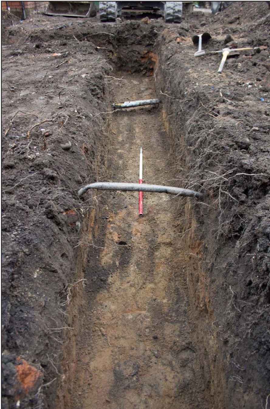
Plate 15: Front extension eastern N-S trench, from the south. Scale 1.0m.
