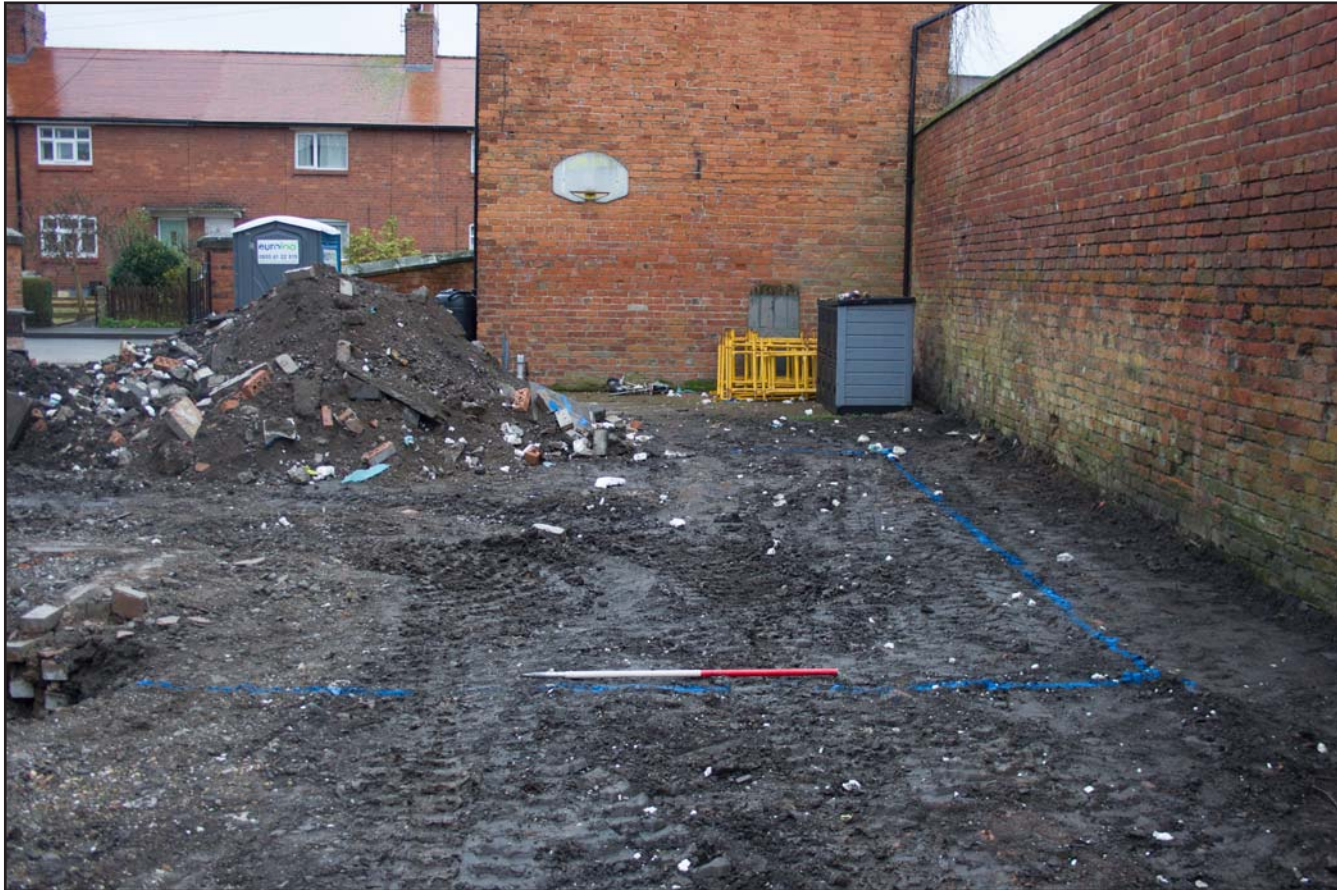
Plate 10: Pre-excitation photograph of front extension footprint, from the west. Scale 1.0m.
