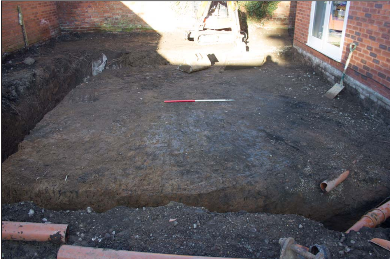
Plate 02: Post-excitation photograph of rear extension footprint, from the south. Scale 1.0m.
