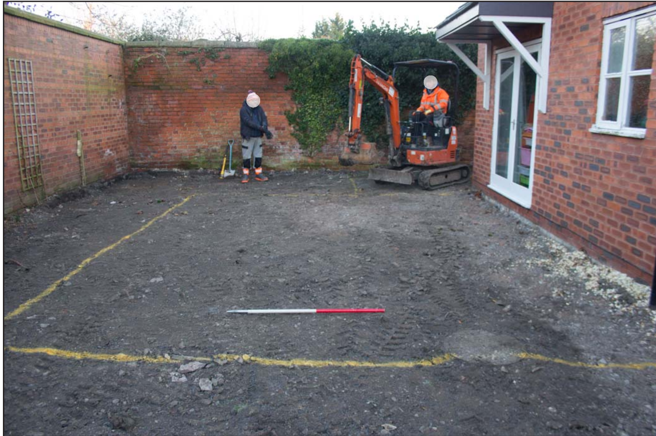
Plate 01: Pre-excitation photograph of rear extension footprint, from the south. Scale 1.0m.
